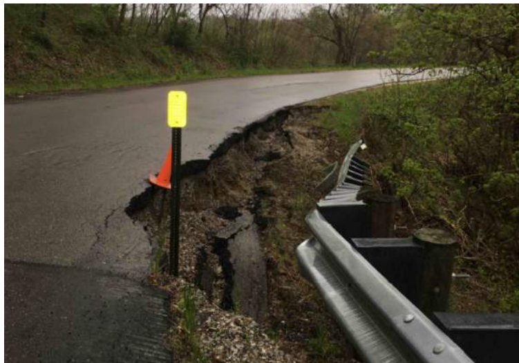
View of Roadway Embankment Looking West Across the Slip Area
