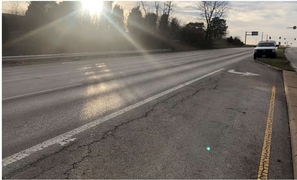
Photograph 1: Overall Pavement Condition of Existing SR-725
