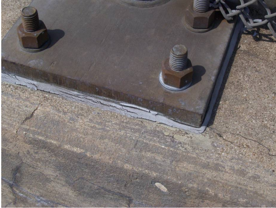
Photo No. 7: Fence mount on top of guard rails.
