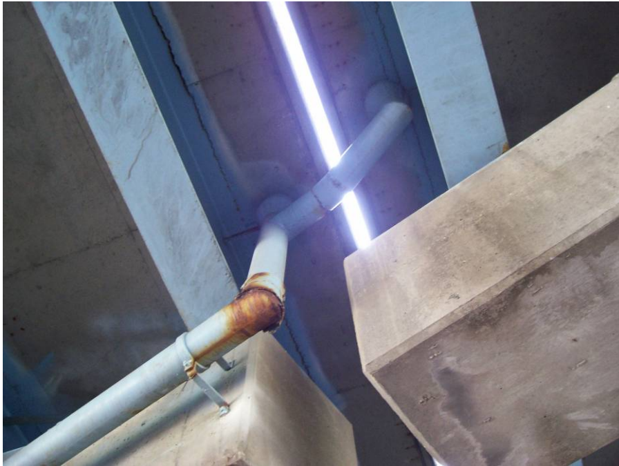
Photo No. 4: Underside of deck drains.
