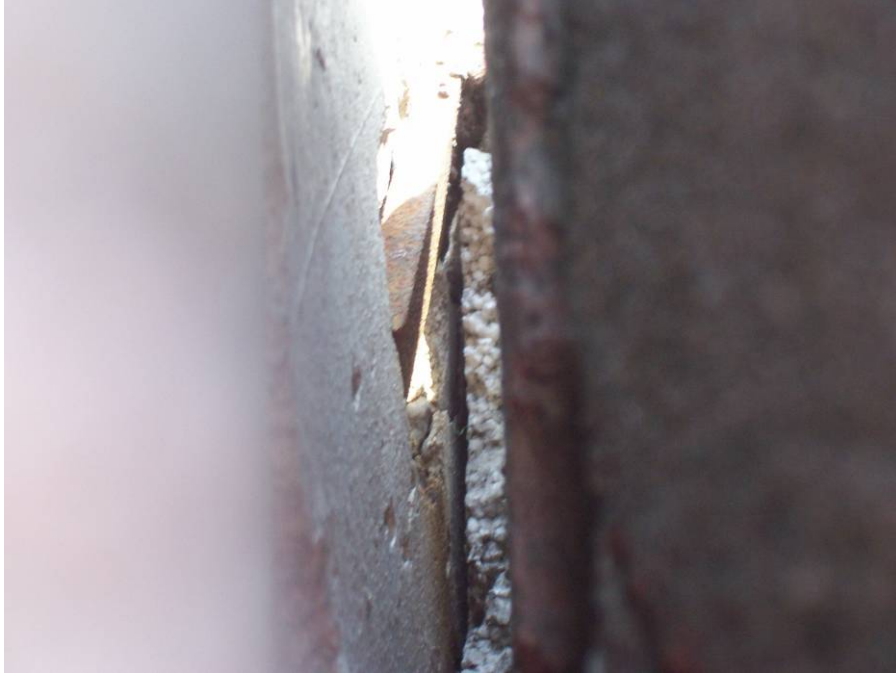
Photo No. 5: Styrofoam inside expansion joint.
