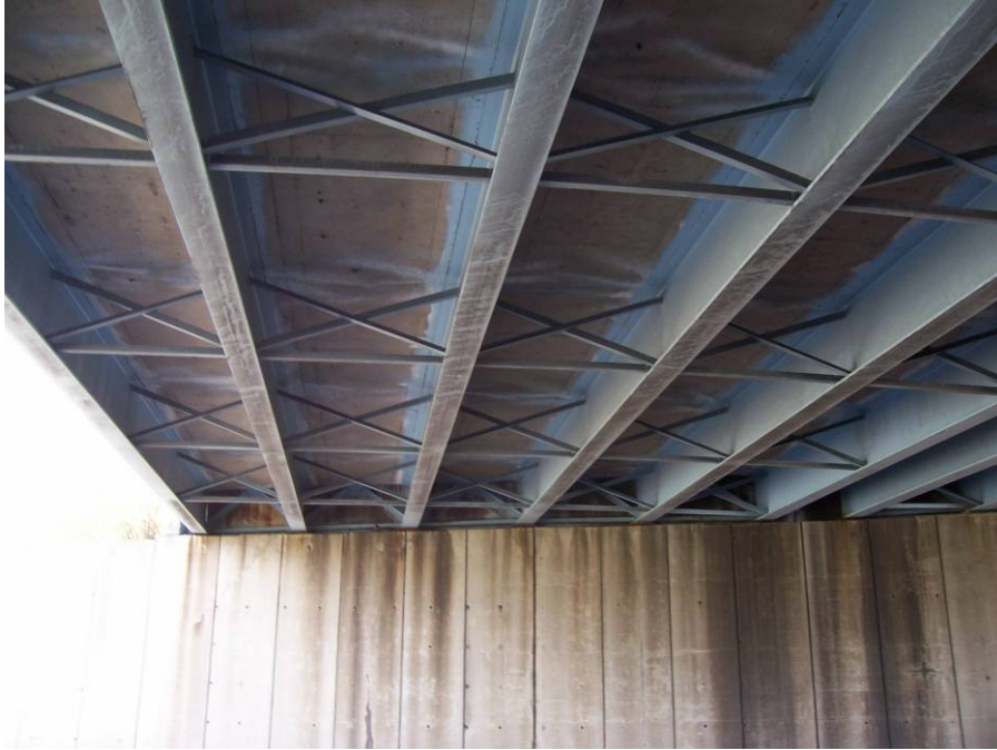
Photo No. 3: Under side of concrete deck and steel support beams.
