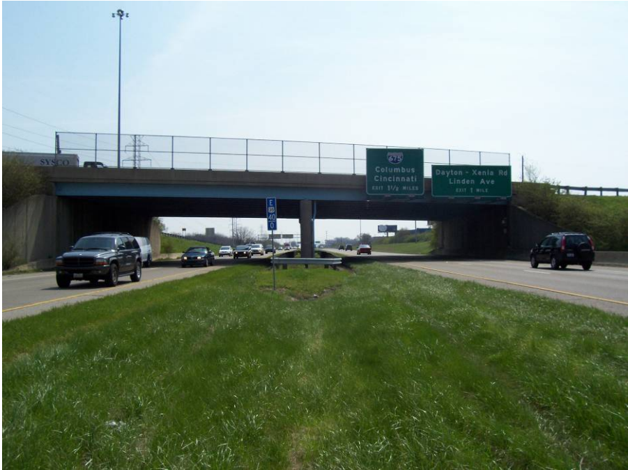
Photo No. 1: View of bridge from the west.
