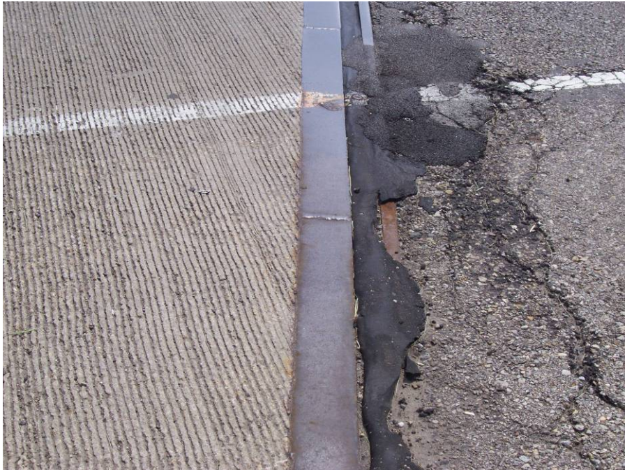
Photo No. 6: Detail of top side of steel expansion joint.
