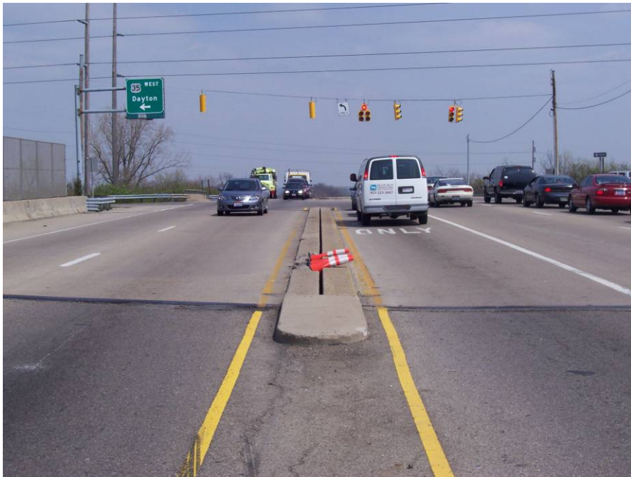
Photo No. 8: Concrete deck and expansion joint.
