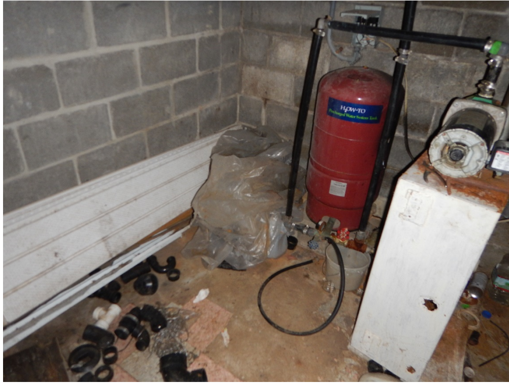
Photo 6: HA-7 and HA-8: Gray and Pink 9x9 floor tile, located in furnace room of basement only.
