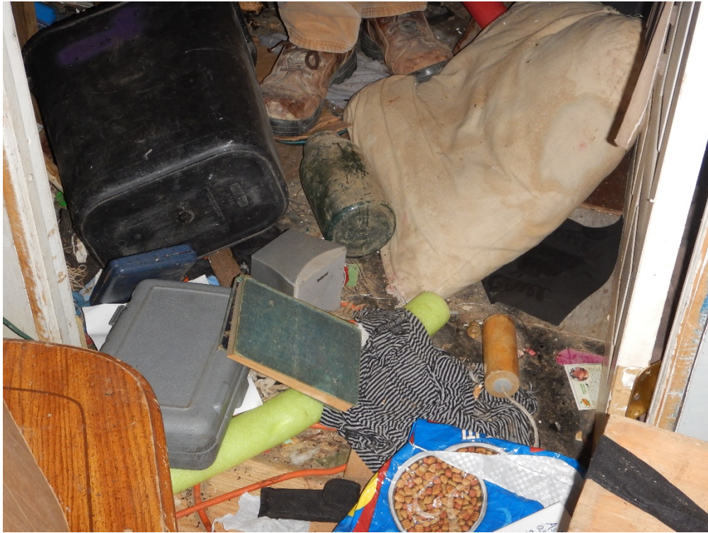
Photo 3: HA-4: Asphalt flooring located in Room #1 only.
