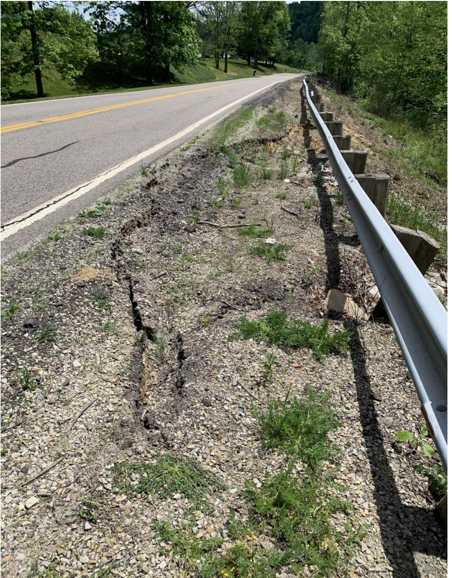
Image provided by ODOT (File Date 12/2022)
