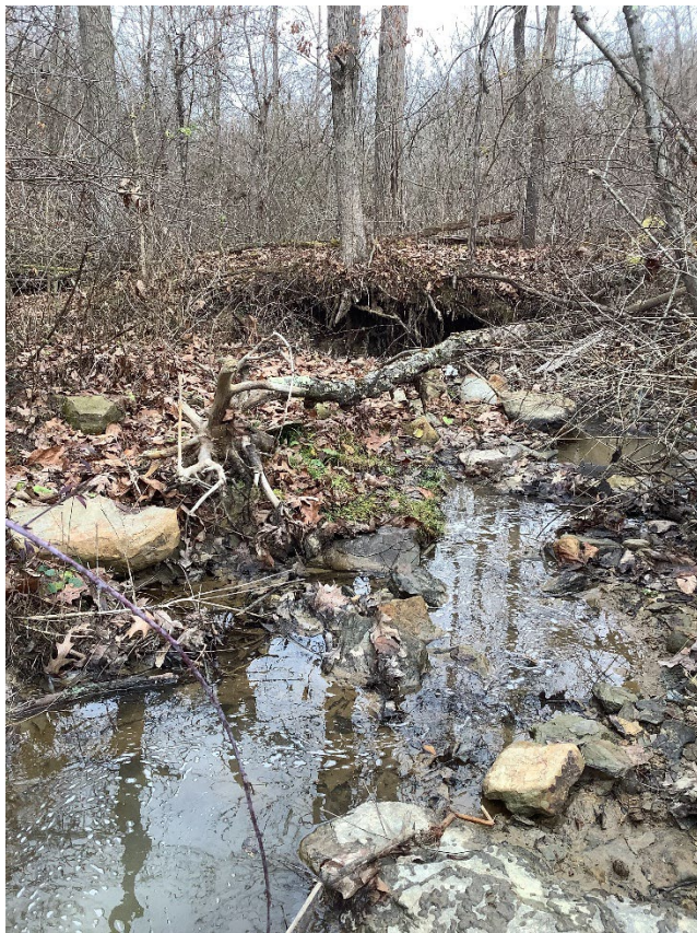
Photo 9 – Facing north, downstream from culvert outlet
