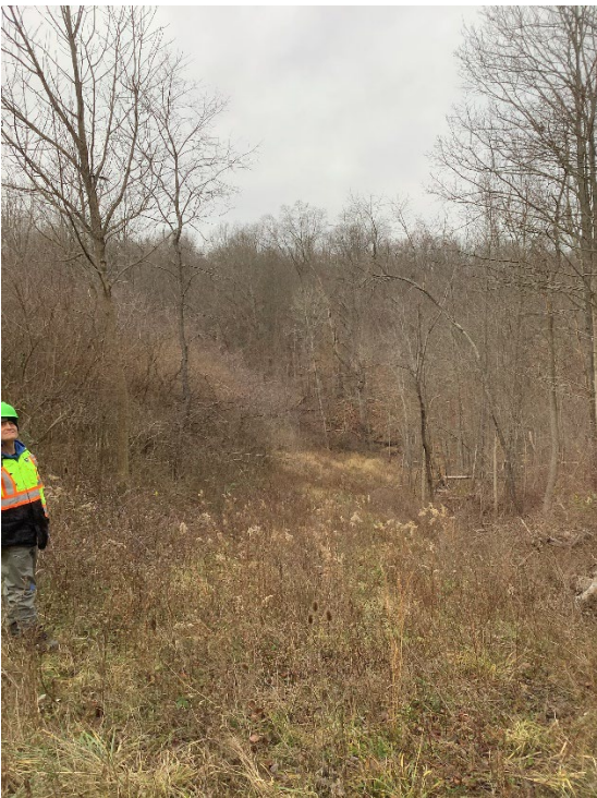
Photo 2 – mid-slope facing west – route construction will bring in equipment – clear of trees
