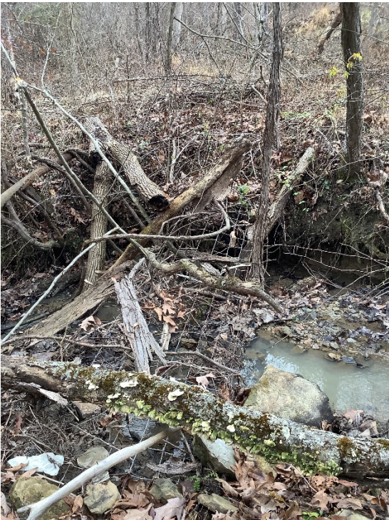
Photo 13 – ROW fence and edge of construction limits for the project
