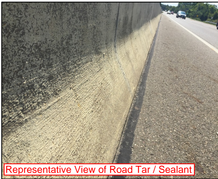
Representative View of Parapet Wall Expansion Joint
