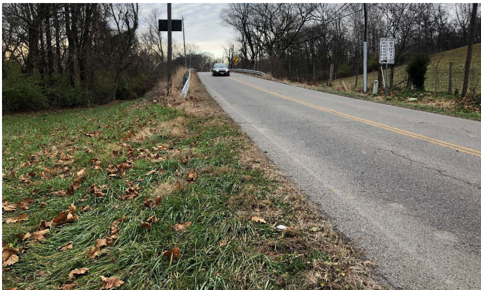
Photograph 5: Drainage Ditches on Both Sides of Roadway
