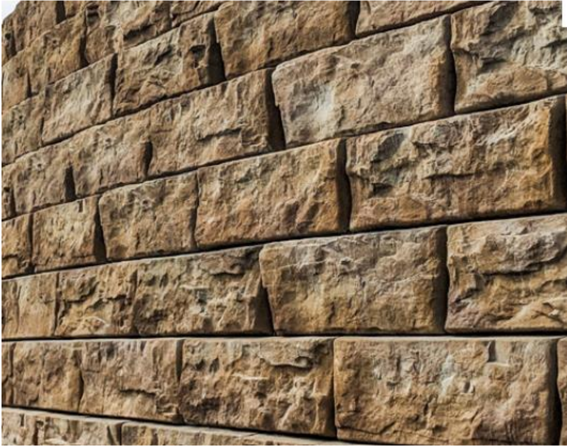
Large Block retaining wall under US 35 bridge
