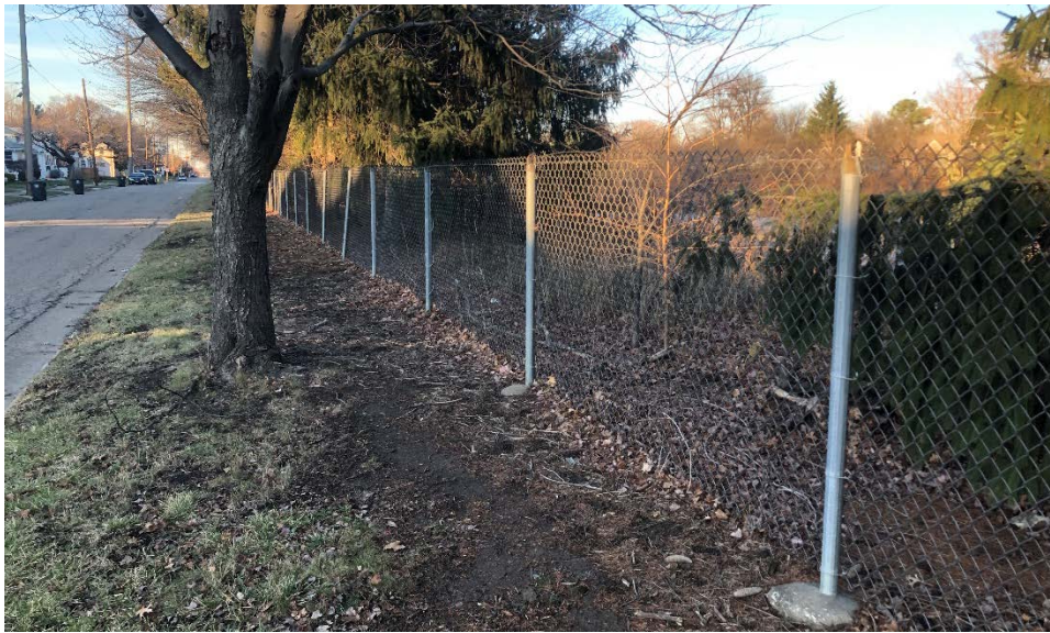
Photograph 7: Slope between Burkhardt Ave. and IR-77
