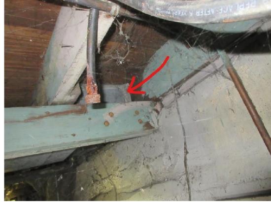
459 Blinn St – Basement
