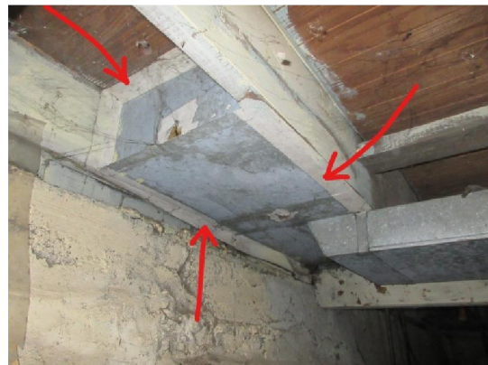
459 Blinn St – Basement
