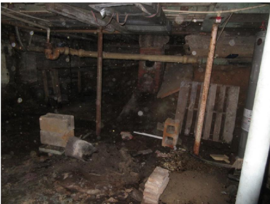
459 Blinn St – Basement
