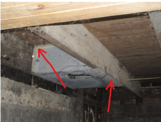
459 Blinn St – Basement
