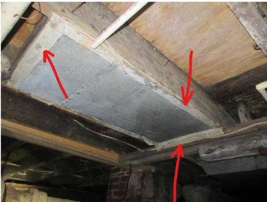
459 Blinn St – Basement
