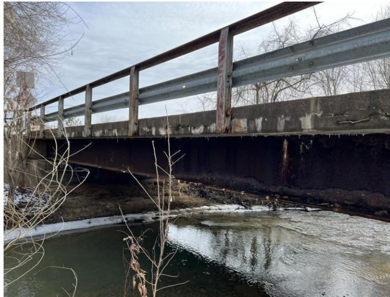
Photograph 10 Overall Bridge Deck Condition
