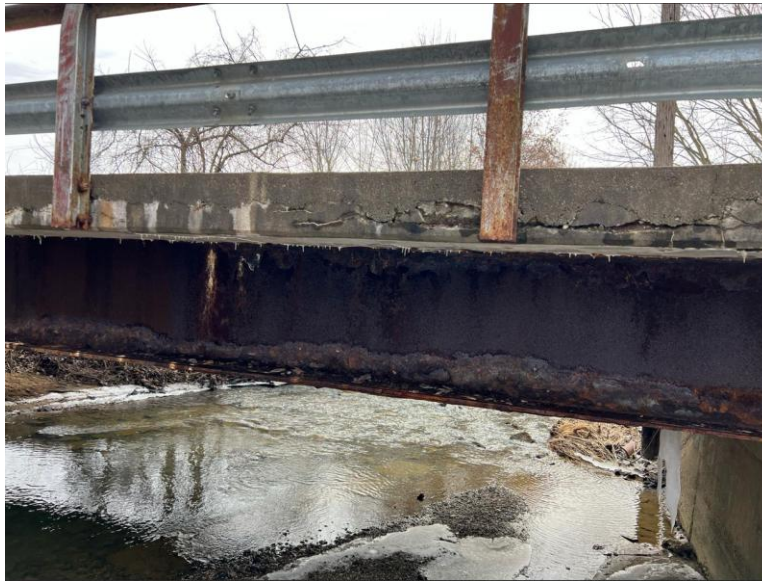
Photograph 3 Corrosion and Section Loss at Main Support Beams
