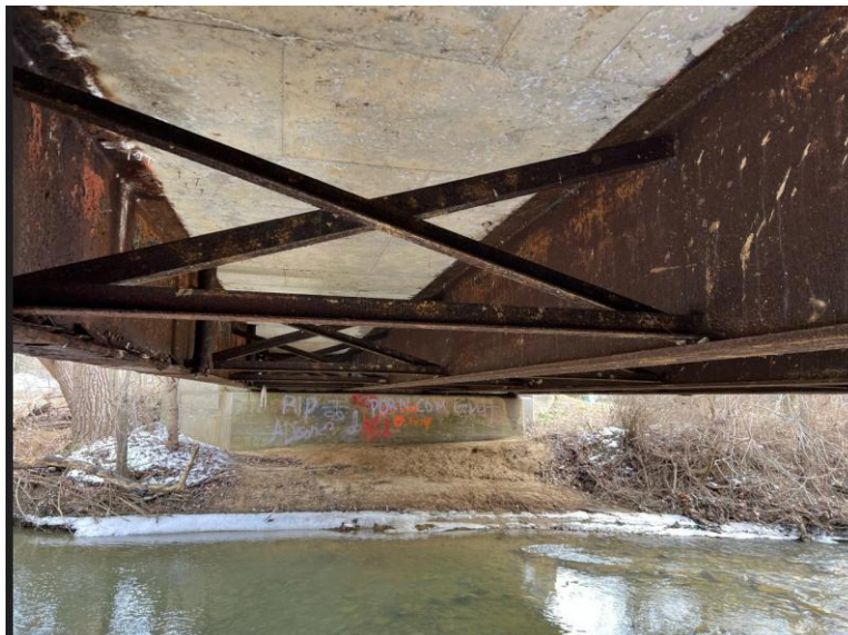
Photograph 3 Corrosion and Section Loss at Main Support Beams
