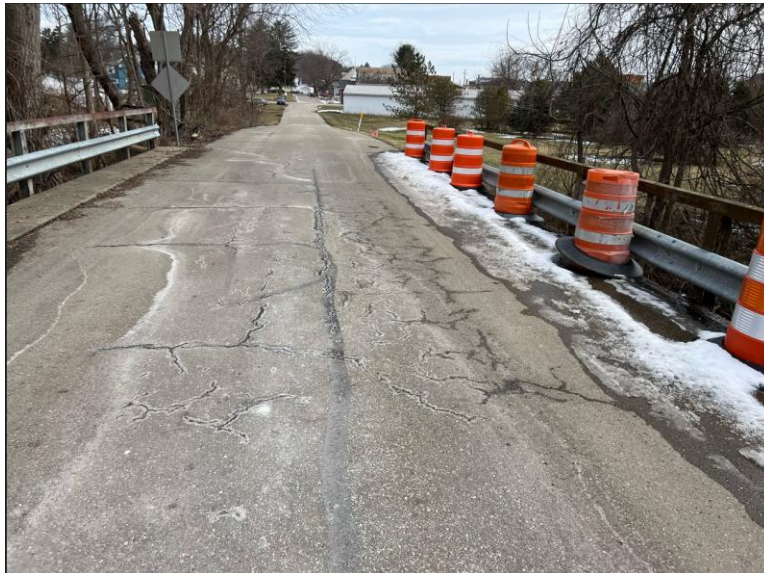
Photograph 9 Overall Condition of Asphalt Wearing Course
