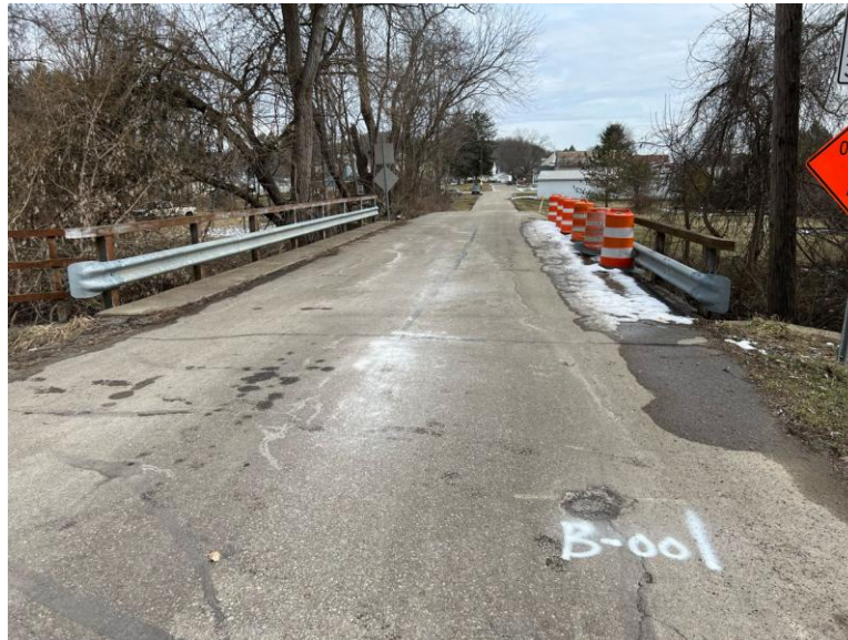
Photograph 1 Overall Bridge View
