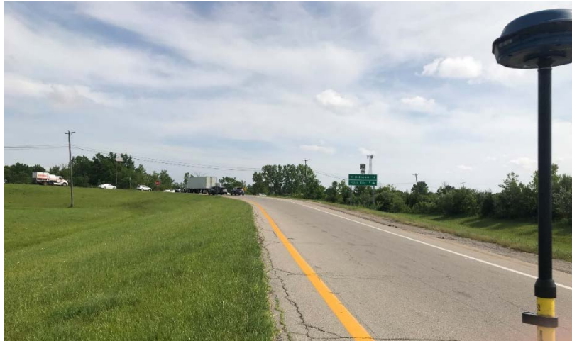
Photograph 3: Pavement condition and embankment slope along Ramp D
