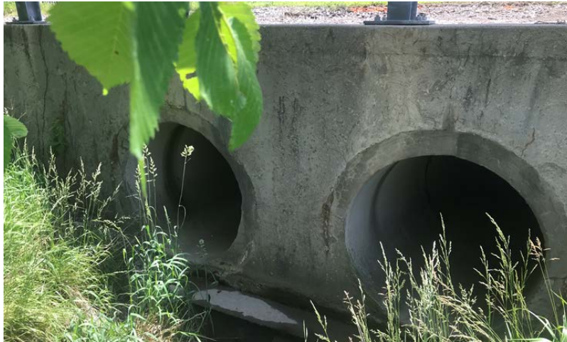
Photograph 4: Industrial Parkway Culvert
