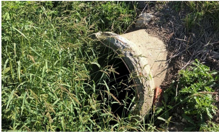
Photograph 6: Inlet of Culvert UNI-42-7.661
