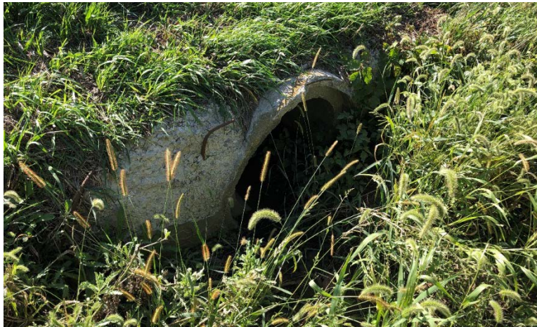
Photograph 4: Outlet of Culvert UNI-42-7.048
