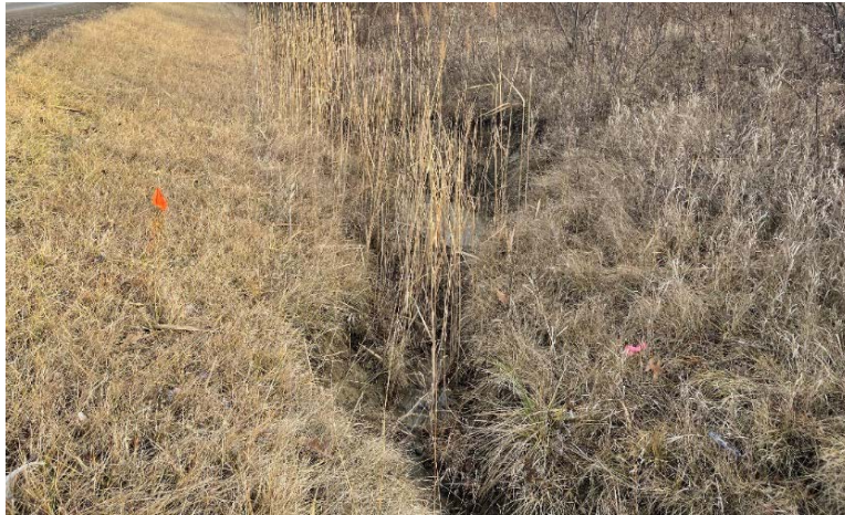
Photograph 2: Signs of Standing Water in Drainage Ditches
