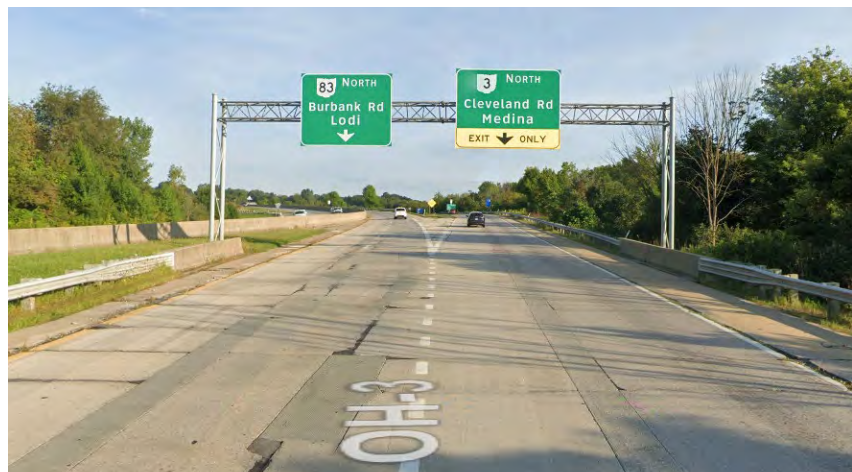
Figure 3 - Google Street View Image of SR-3 northbound Exit Signage
