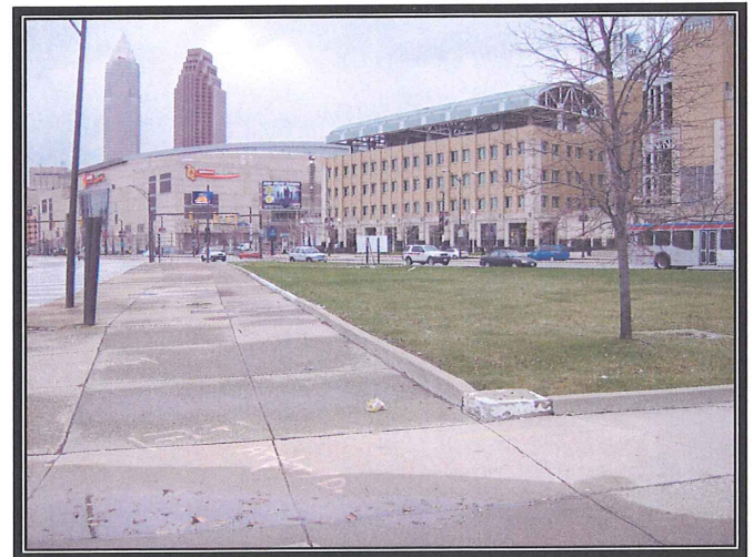
Photograph 4 View looking northwest at the Property from the southernmost point of the Property.
