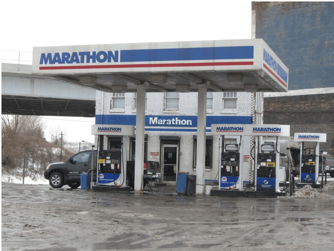
TO-2. North Elevation, Looking South.
