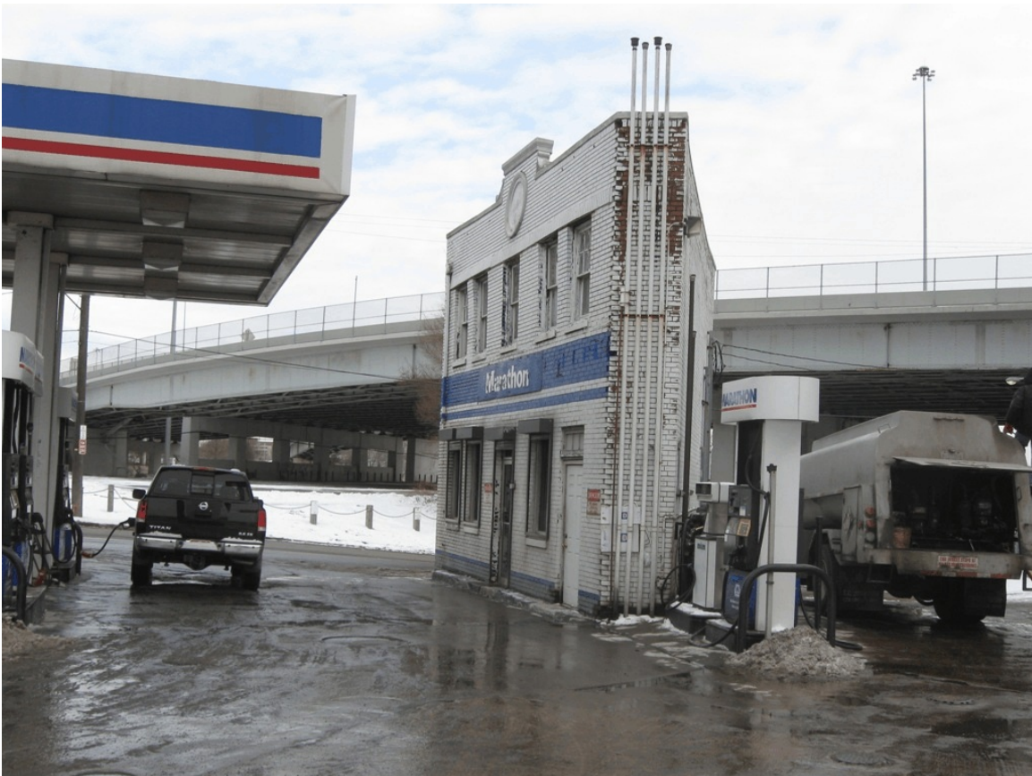
TO-3. West Corner of Filling Station, Looking East.
