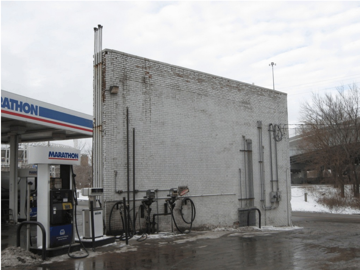
TO-4. South (Rear) Elevation, Looking Northwest.
