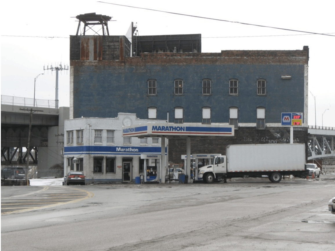
TO-1. General Overview Looking South from Corner of Central Viaduct and Commercial Road.
