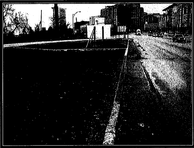
Photograph 9 View looking northwest at the northwestern corner of the Property.
