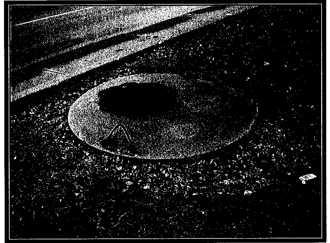
Photograph 8 View of a water meter located centrally along the northeastern border of the Property.
