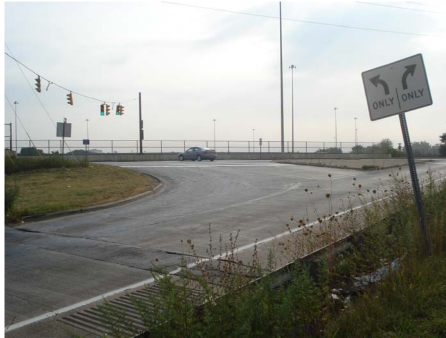
Broadway @ IR-490 EB Exit Ramp Looking East
