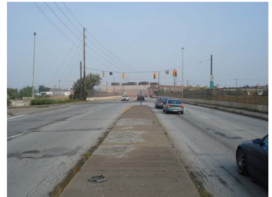
Broadway @ IR-490 EB Exit Ramp Looking Northwest
