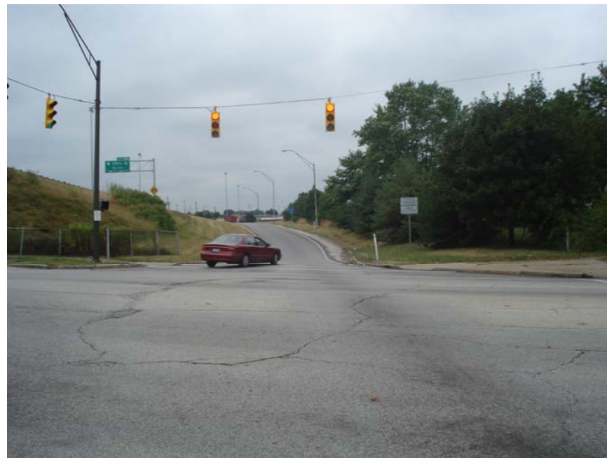
West @ I-90 Westbound On-Ramp Looking West
