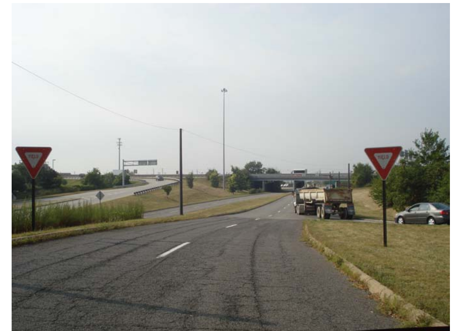
East 14th @ IR-77 NB Exit Ramp terminal Looking South
