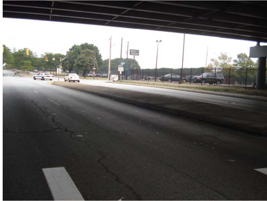
East 30th under IR-77 Looking North
