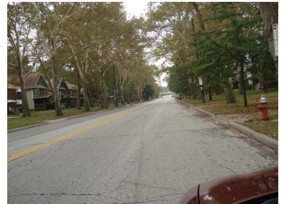
West between Western and Madison Looking South
