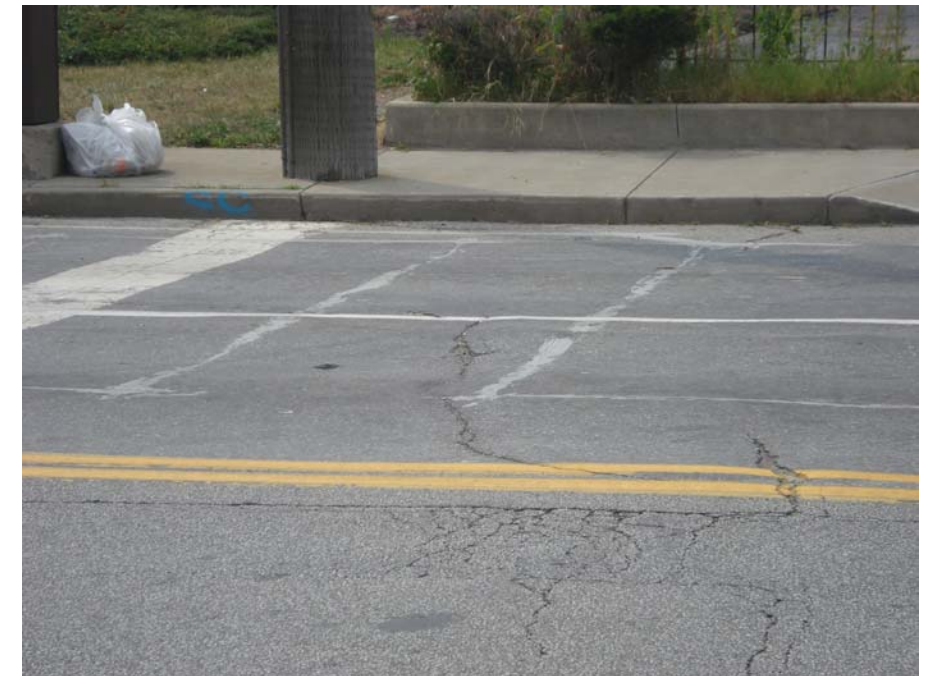
Carnegie @ East 18th Looking West (southbound approach)
