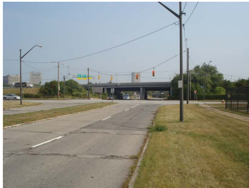
East 14th @ Orange Looking North
