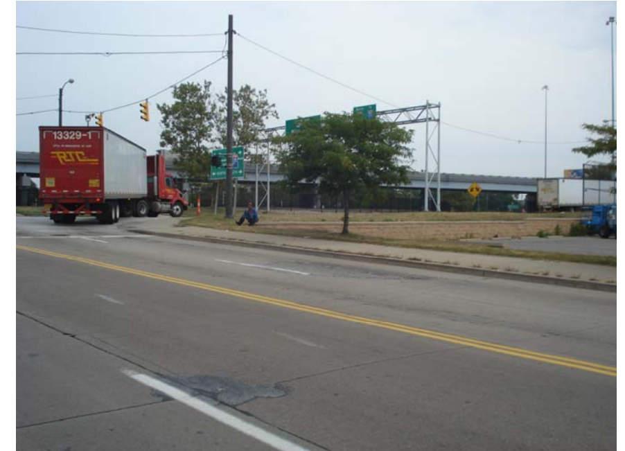
East 30th @ Orange Looking North
