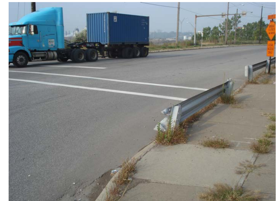
Broadway @ East 37th / Rockefeller Looking West towards IR-490 WB Entrance Ramp
