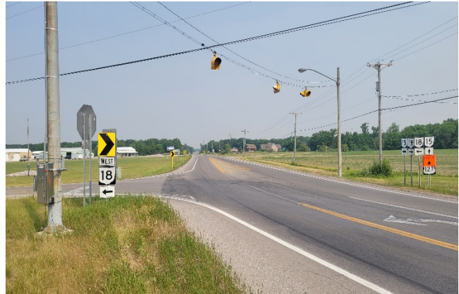
Photo 1 – Intersection Looking West
