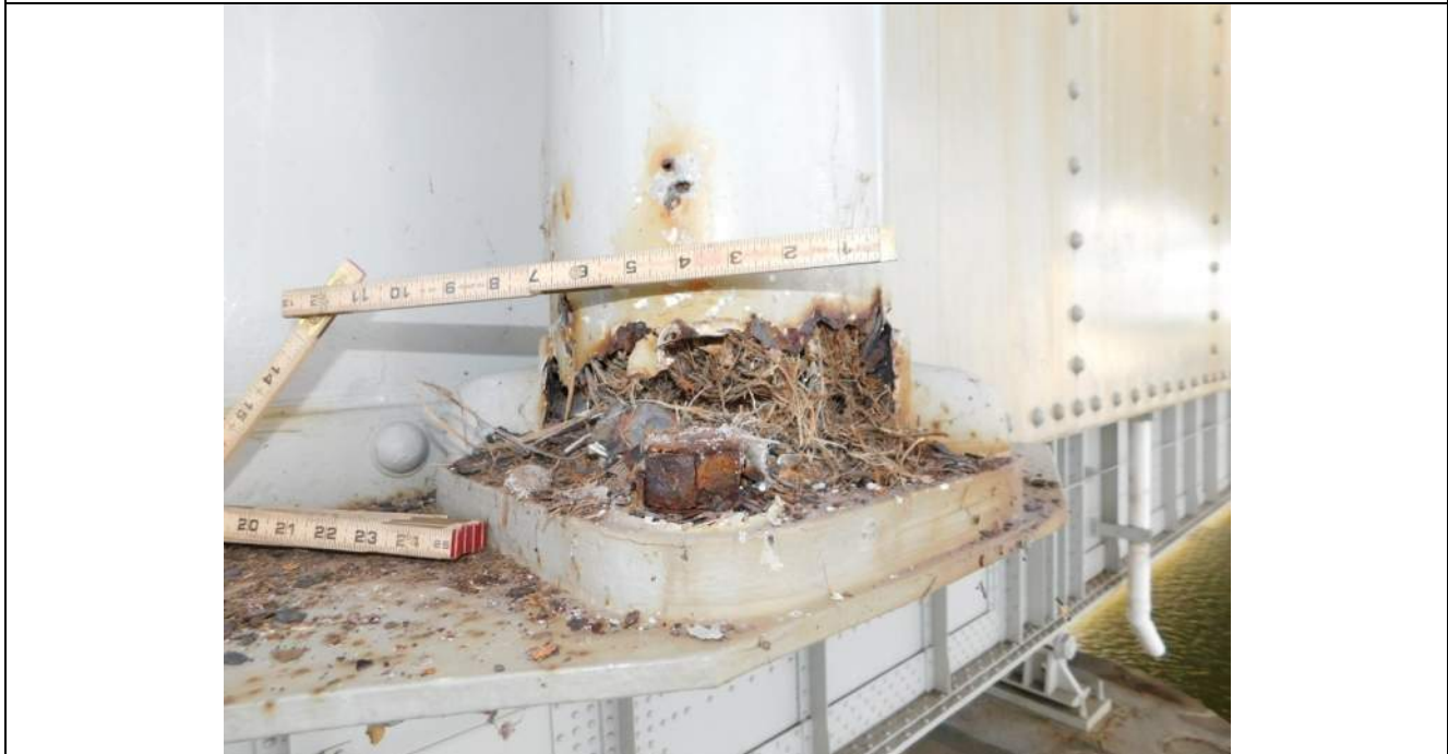
Photo S-320 - [Span 3] -East side light pole at Floorbeam 25S, holes in base of pole around 75% of perimeter, detail view, Looking North
