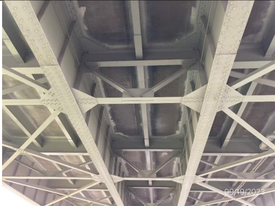
Photo S-171 - [Span 9] -Span framing and underside general view, Looking North
