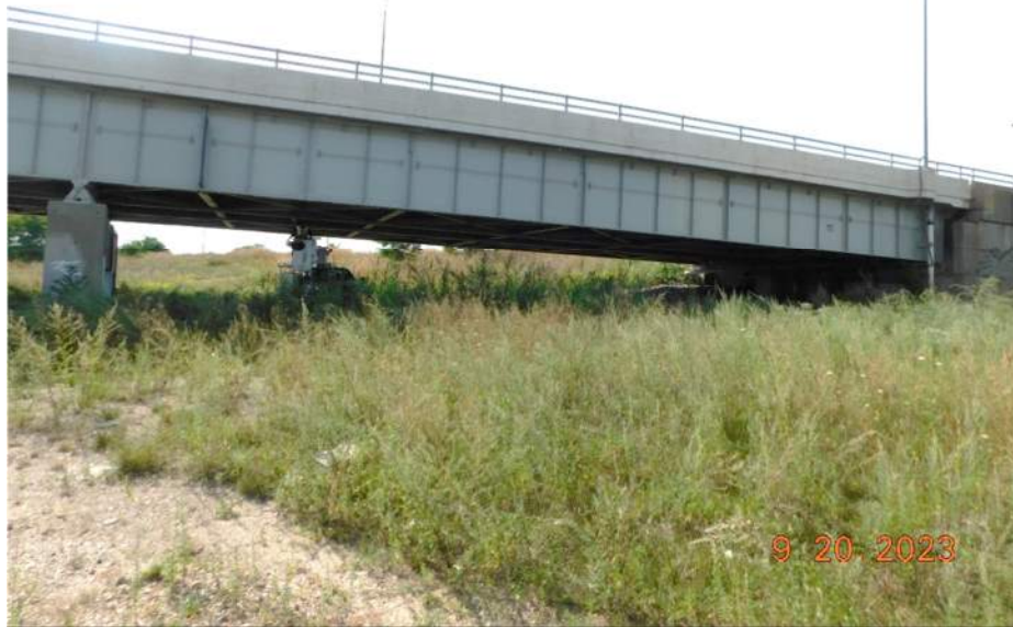
Photo S-81 - [Span 10] -East fascia, general view, Looking West
