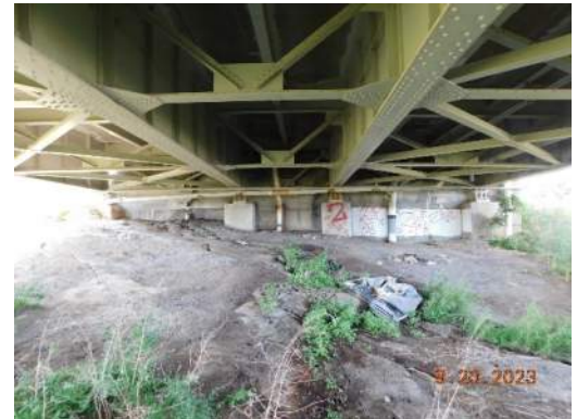
North abutment columns and backwall
