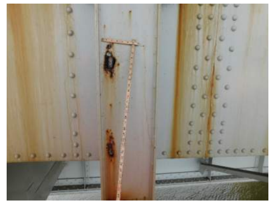
Span 6 East fascia support, holes at south post base web plate
