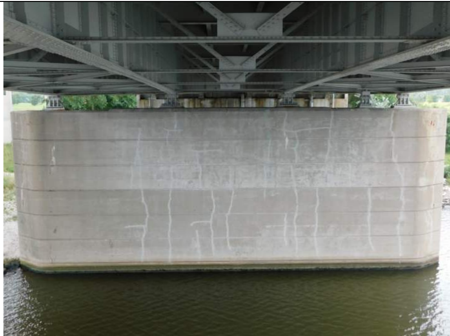
Photo S-286 - [Pier 1] -Pier North face, general view, Looking South
