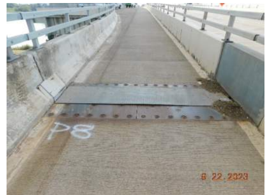
Pier 8 expansion joint at mixed-use trail
