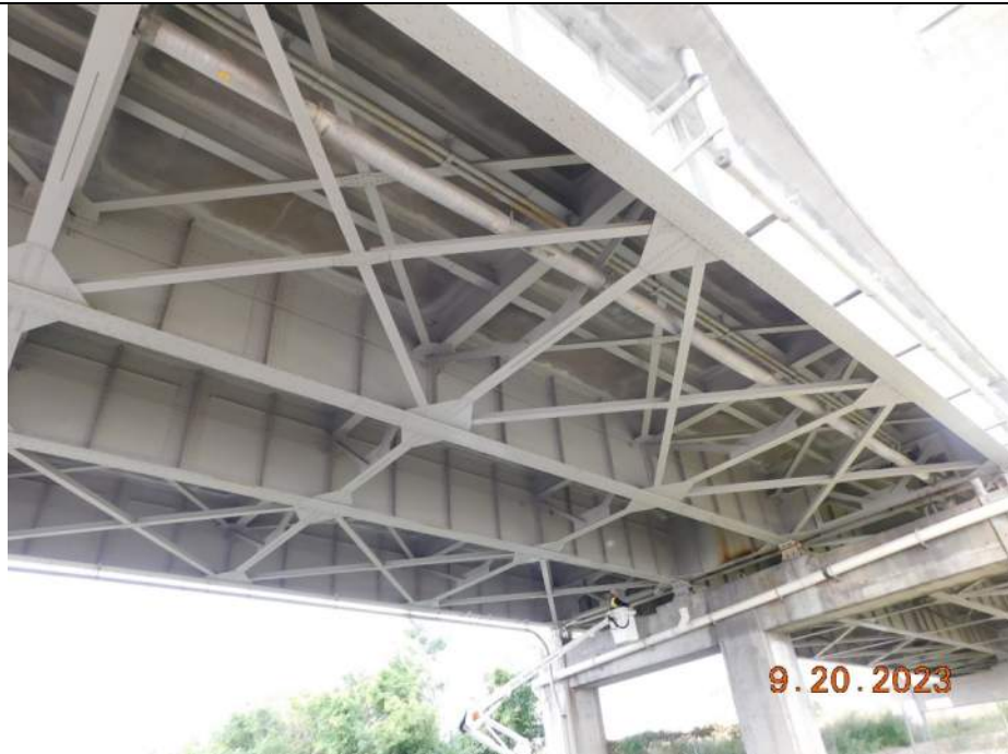
Photo S-170 - [Span 8] -Span framing and underside general view, Looking Northwest
