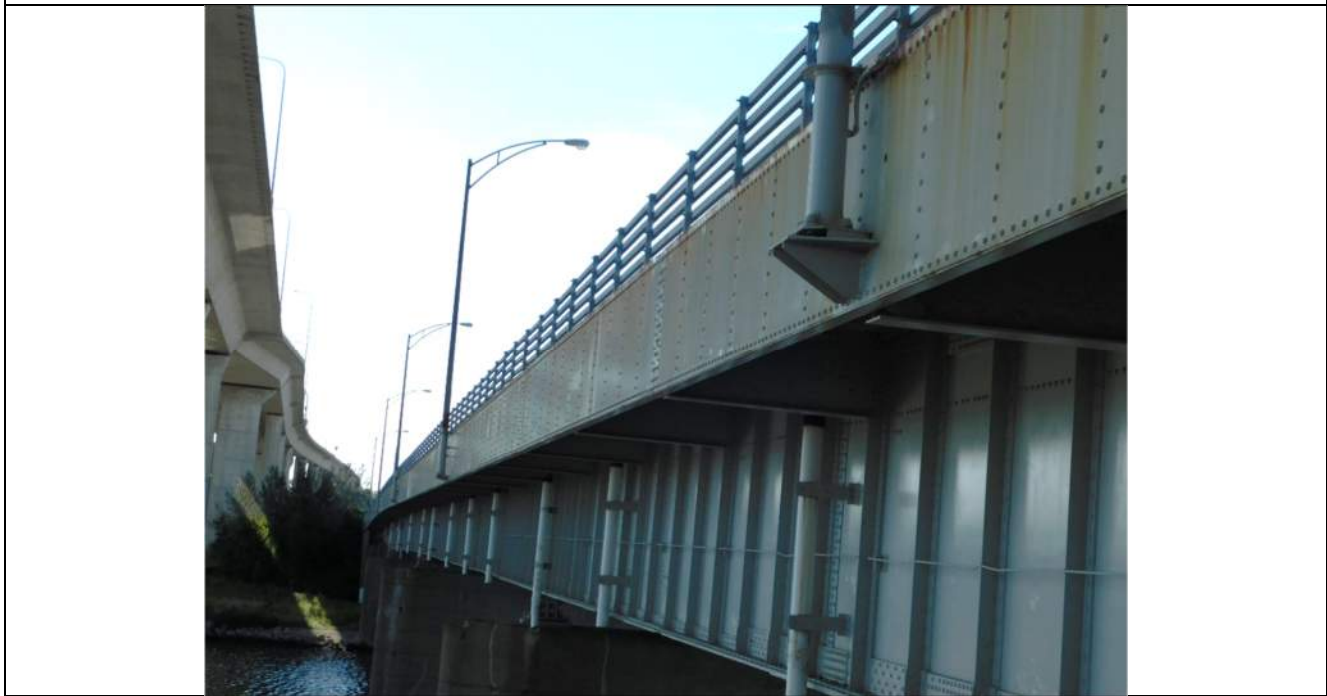
Photo S-72 - [Span 4] -East fascia and framing, general view, Looking Southwest
