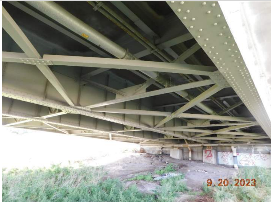
Photo S-172 - [Span 10] -Span framing and underside general view, Looking Northwest
