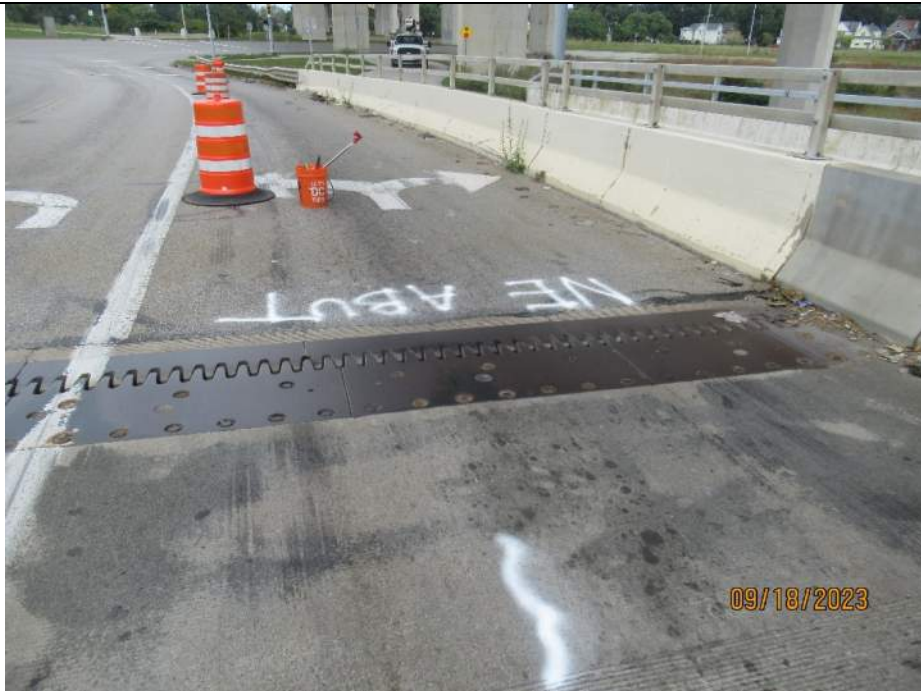
Photo S-14 - [North Approach] -Roadway approach pavement, NB lanes, Looking North
