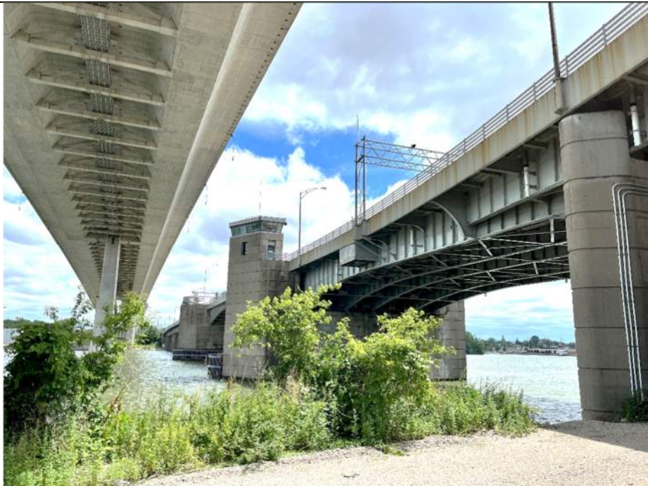
Photo S-2 - [North shoreline] -Structure East elevation, Looking Southwest
