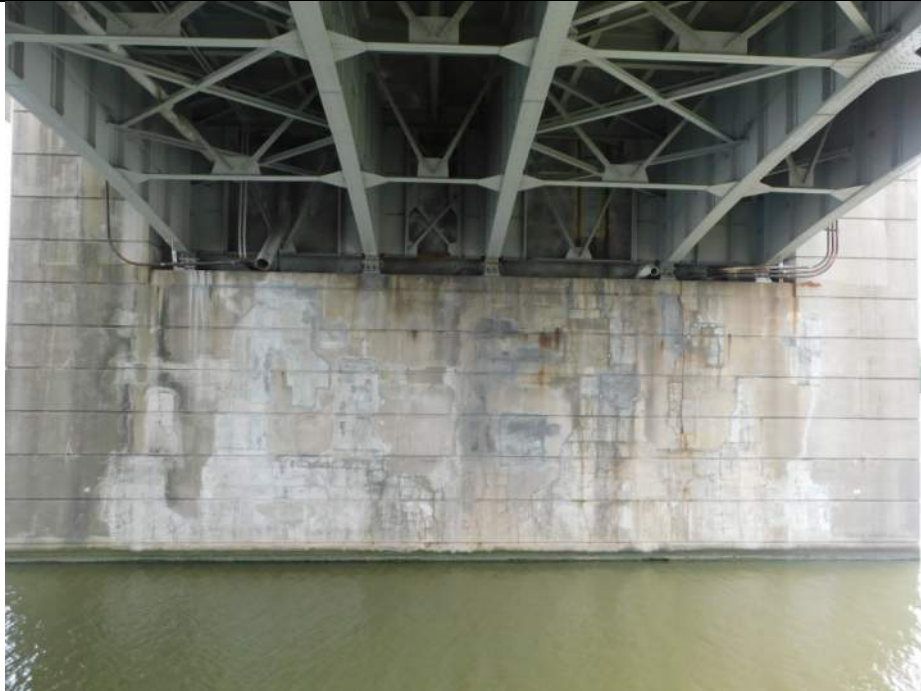
Photo S-301 - [Pier 5] -Pier North face, general view, Looking South
