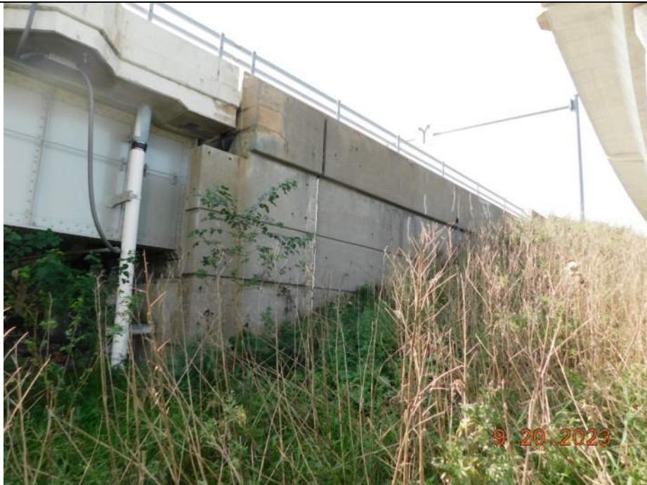
Photo S-284 - [North Abutment] -Abutment East wingwall, Looking North
