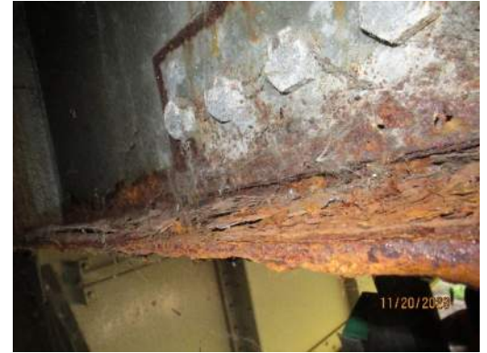
Span 10 FB11s at North abutment, BF SL
