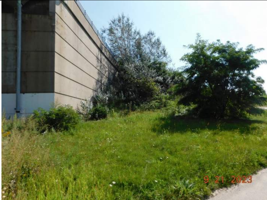
Photo S-29 - [South Approach] -Southwest approach slope, general view, Looking Southwest
