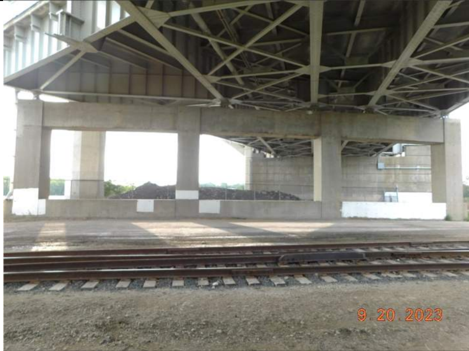
Photo S-309 - [Pier 7] -Pier North face, general view, Looking South
