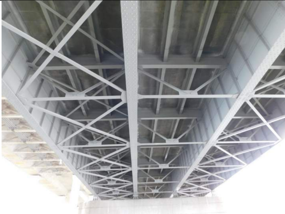
Photo S-163 - [Span 3] -Span framing and underside general view, Looking South
