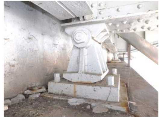
Pier 4 (south side) Rocker Bearing 2W
