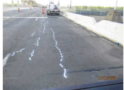
Span 4 deck surface, SB lanes
