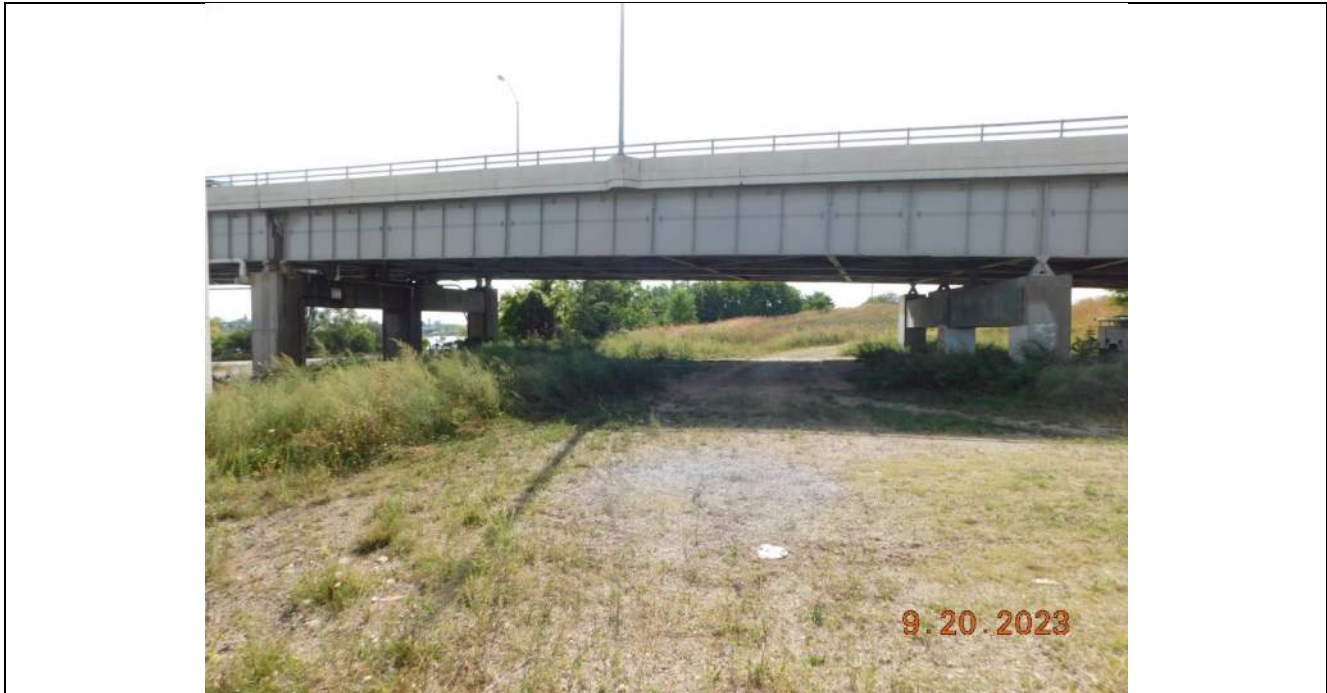
Photo S-79 - [Span 9] -East fascia, general view, Looking West
