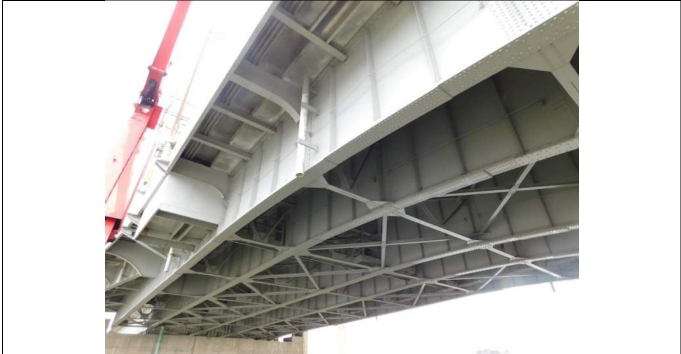
Photo S-167 - [Span 6] -Span framing and underside general view, Looking Northeast
