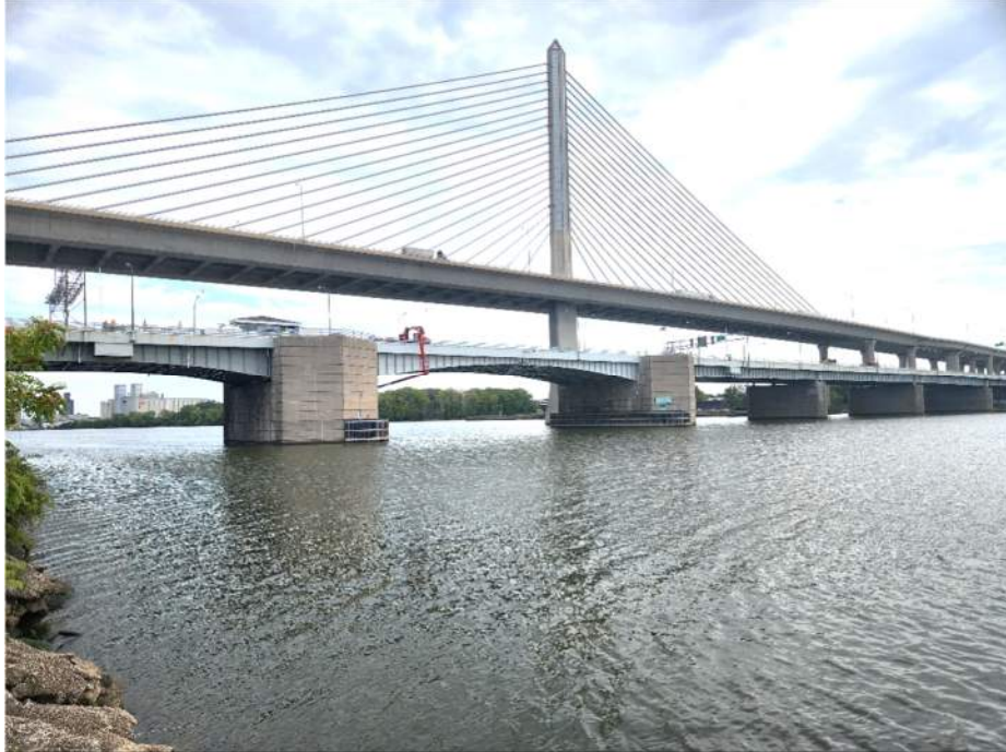
Photo S-1 - [North shoreline] -Structure West elevation, Looking Southeast
