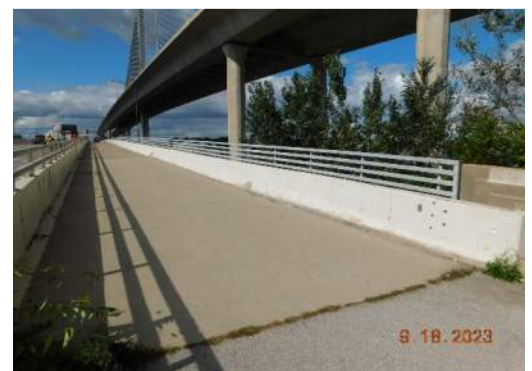
Southeast sidewalk / trail barrier & railing
