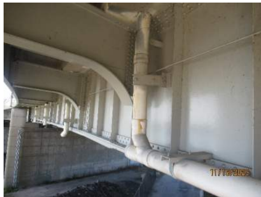
Span 7 drainage downspouts and piping
