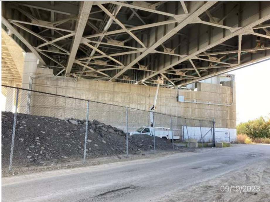
Photo S-306 - [Pier 6] -Pier North face, general view, Looking South
