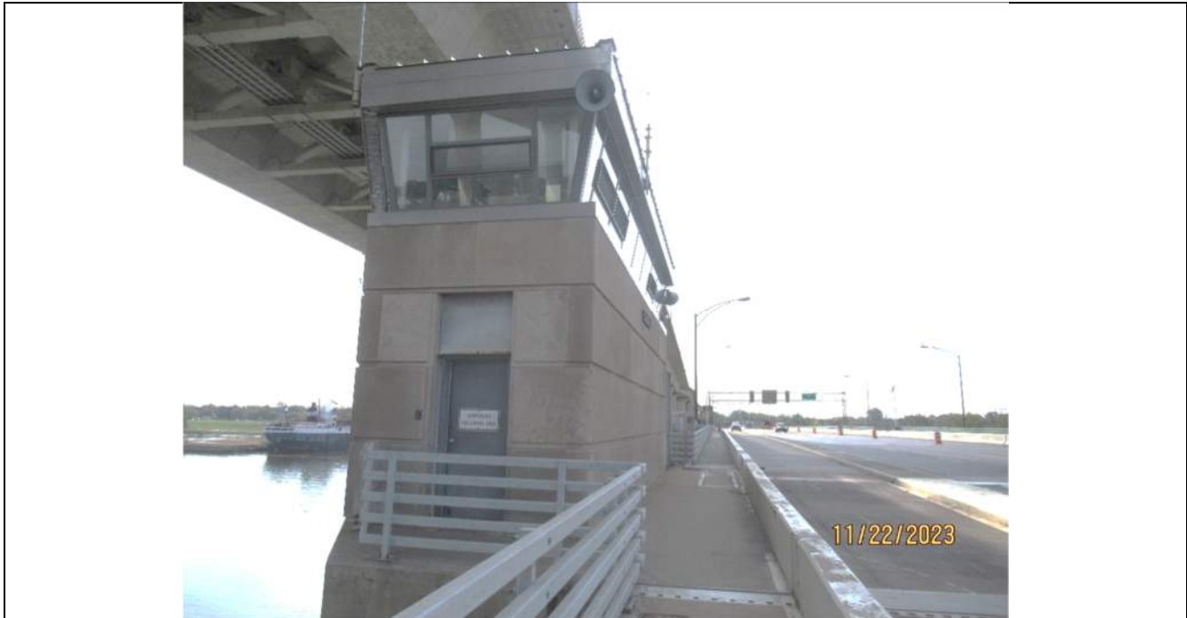
Photo S-371 - [Control House Exterior] -North side and access from roadway level, general view, Looking South
