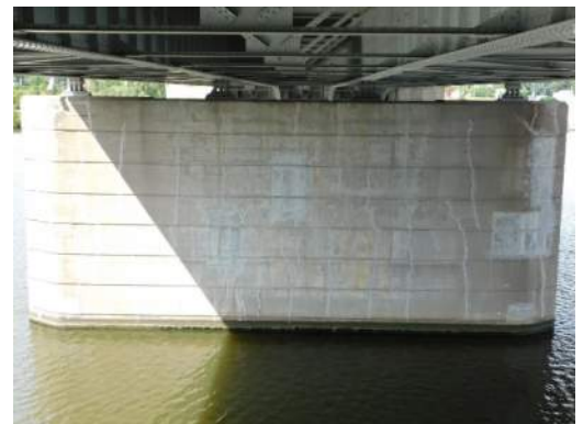
Pier 3 South face, crack and patch repairs
