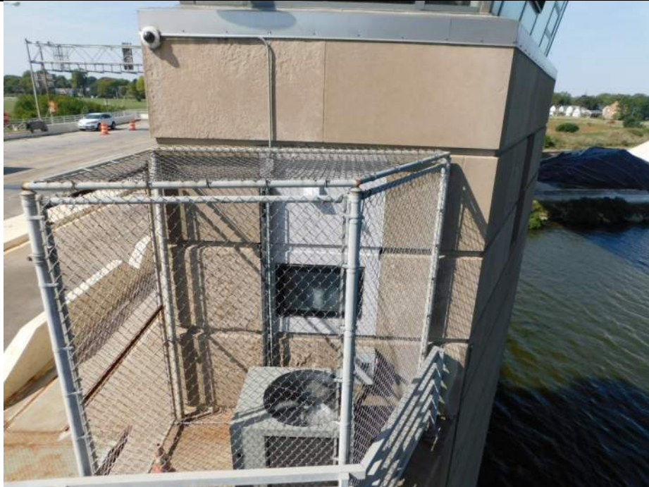
Photo S-373 - [Control House Exterior] -Mechanical cage general view, Looking North
