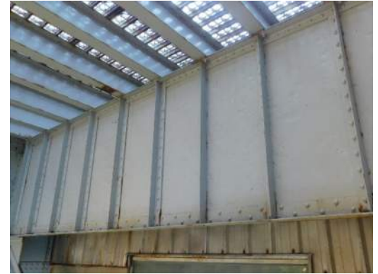
Span 5 South leaf, FB7s web SL throughout
