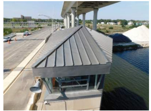
Pier 5 Operator house roof in good condition
