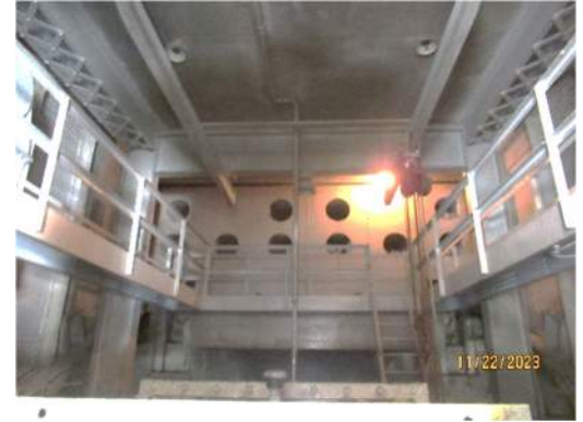
Pier 5 upper catwalks and counterweight pockets, general view at G1W-G2W
