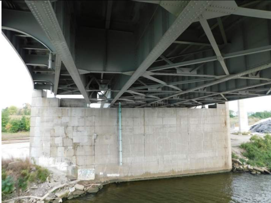
Photo S-305 - [Pier 6] -Pier South face, general view, Looking North
