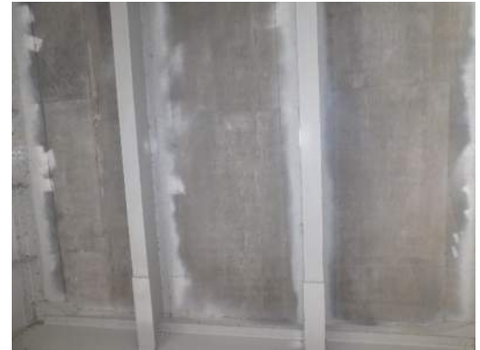
Span 2 deck underside typical general view
