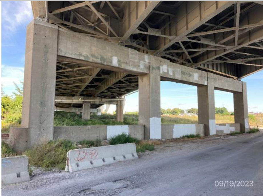
Photo S-308 - [Pier 7] -Pier South face, general view, Looking North
