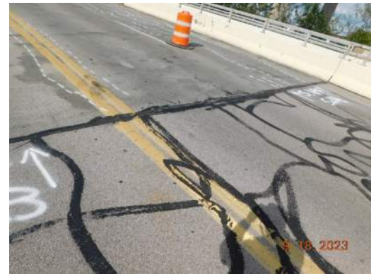
South approach pavement to slab, NB lanes
