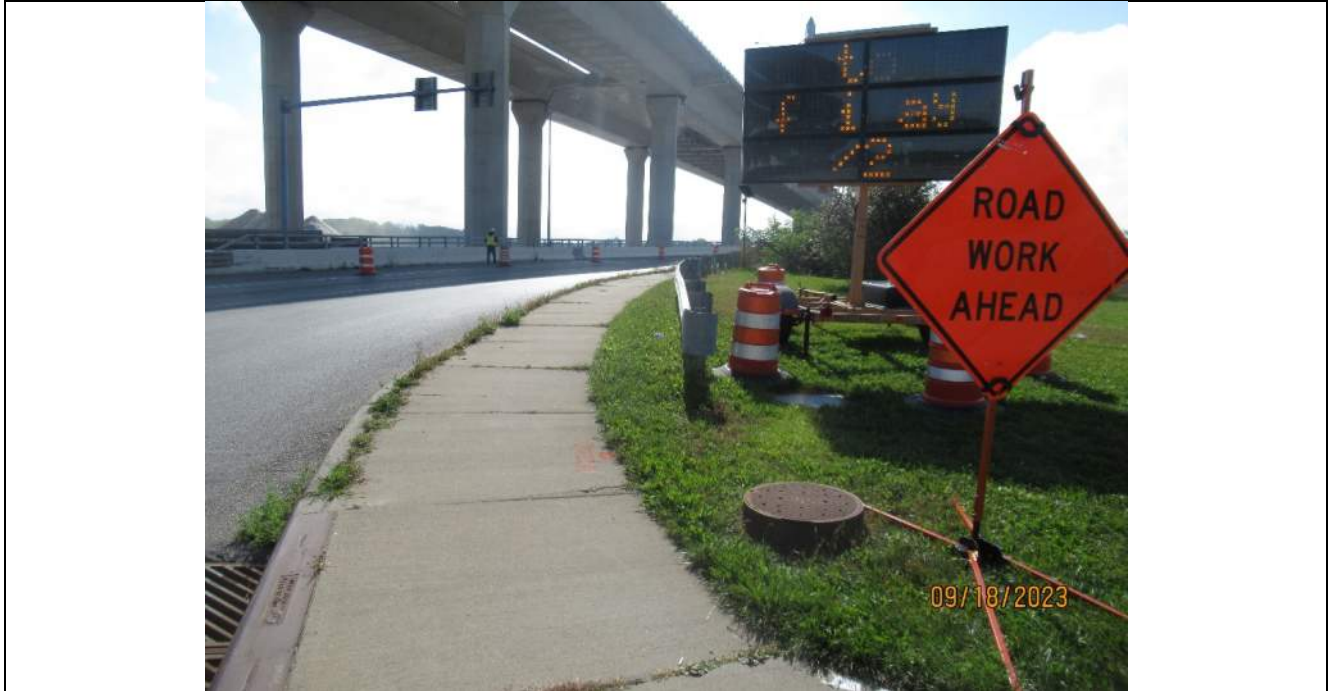
Photo S-23 - [North Approach] -Northwest guard railing, Looking South
