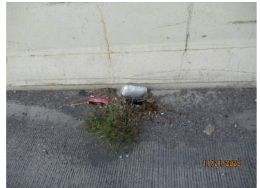
Span 3 drainage scupper at west barrier
