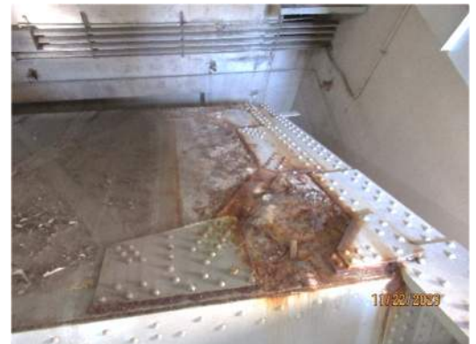
Pier 5, counterweight top at east side
