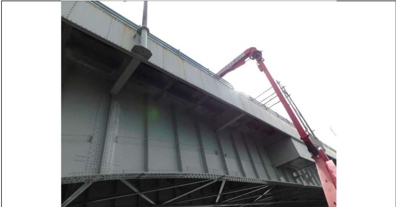
Photo S-71 - [Span 4] -West fascia and framing, general view, Looking Southeast
