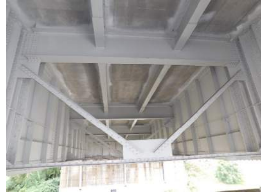
Span 1 typical interior framing
