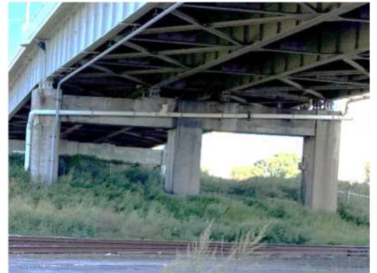
Pier 8, South face general view
