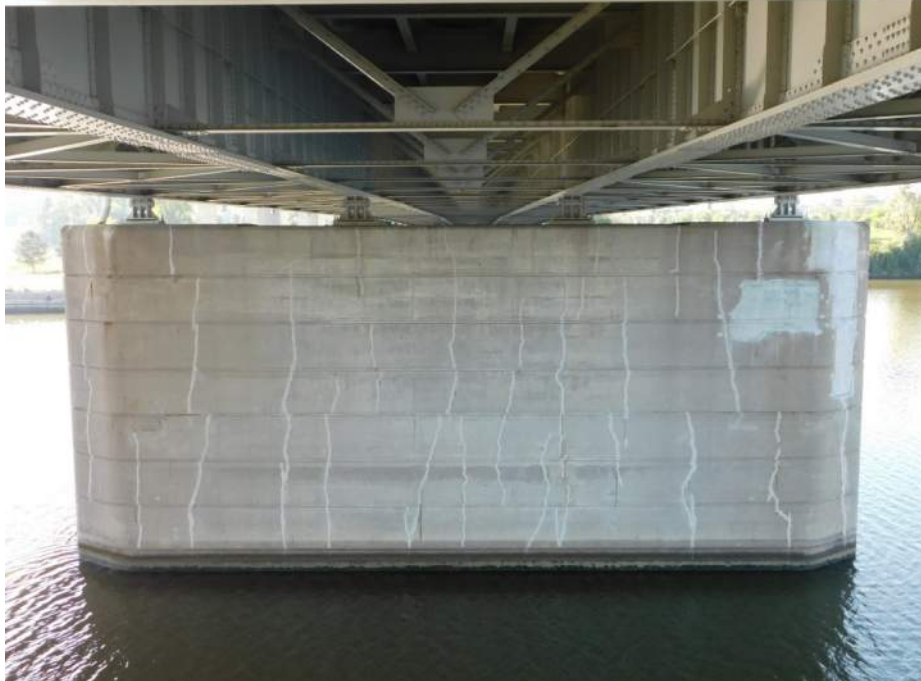
Photo S-291 - [Pier 3] -Pier North face, general view, Looking South
