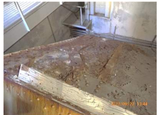
Pier 4, counterweight top at east side
