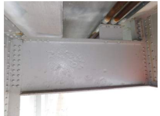
Span 3 West exterior FB20s web SL
