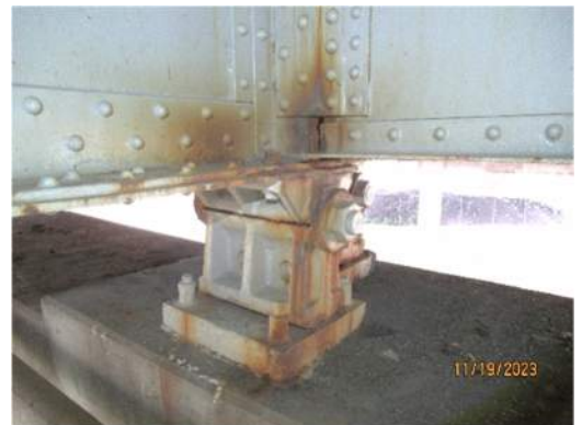
Pier 8 Rocker Bearing 3W (Span 9 side)
