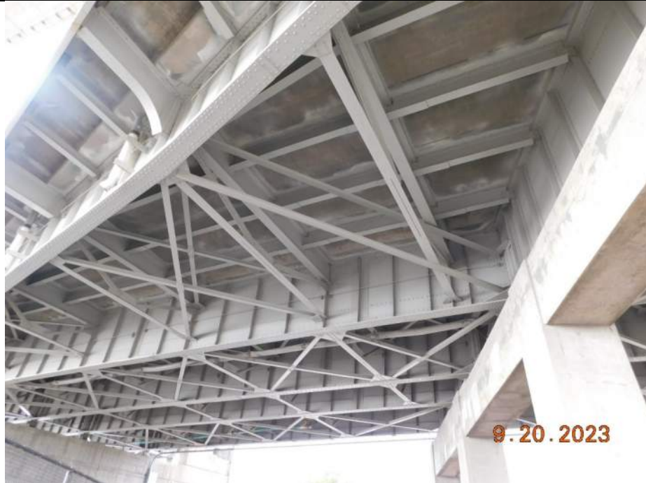
Photo S-169 - [Span 7] -Span framing and underside general view, Looking Southwest
