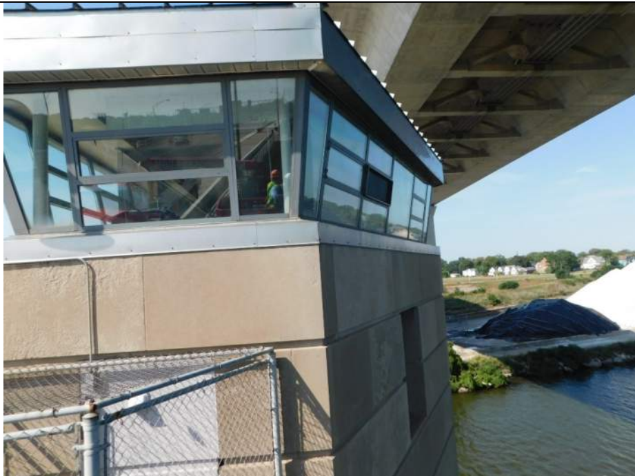
Photo S-374 - [Control House Exterior] -East windows general view, Looking North
