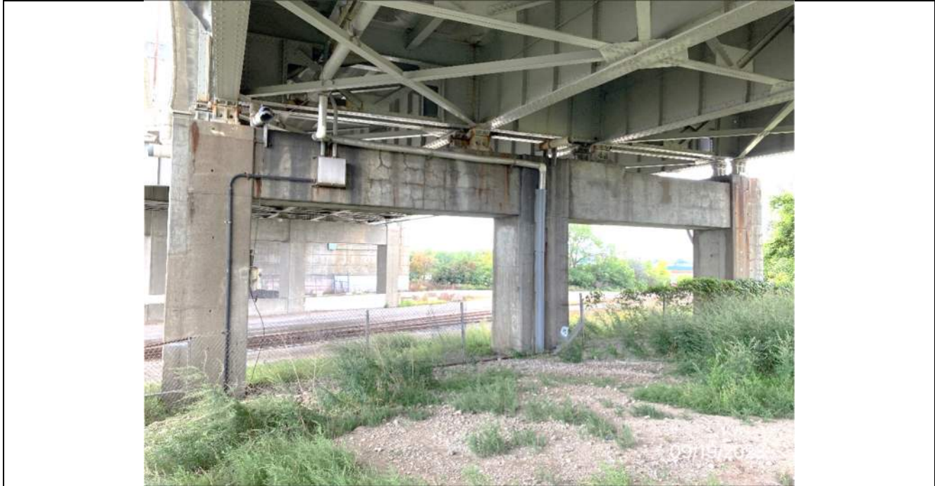
Photo S-311 - [Pier 8] -Pier North face, general view, Looking South
