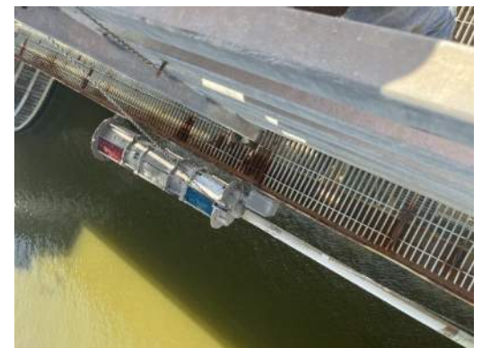
Photo E23: Southeast Navigation Light
