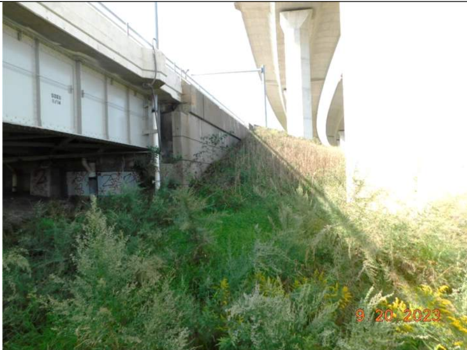
Photo S-32 - [North Approach] -Northeast approach slope, general view, Looking North
