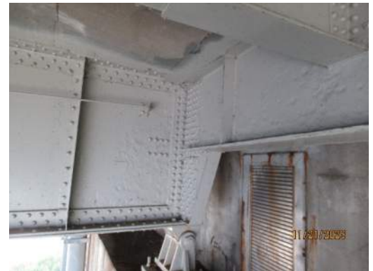
Span 1 Girder 4W west face SL at abutment
