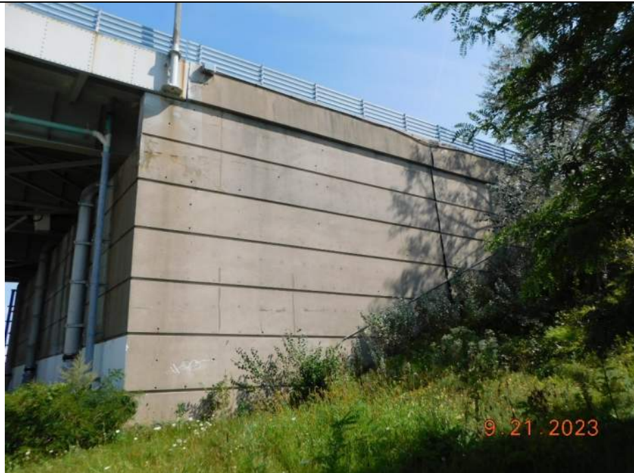
Photo S-276 - [South Abutment] -Abutment West wingwall, Looking Southeast
