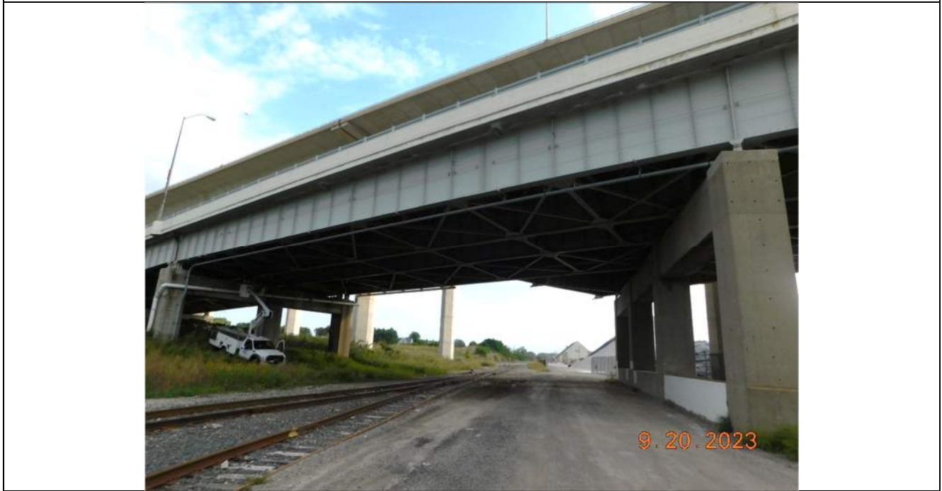
Photo S-76 - [Span 8] -West fascia, general view, Looking East
