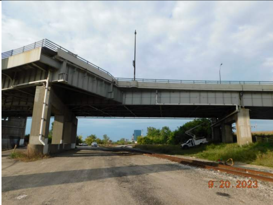
Photo S-77 - [Span 8] -East fascia, general view, Looking West
