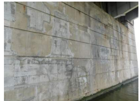
Pier 5 North face detail view, center to west
