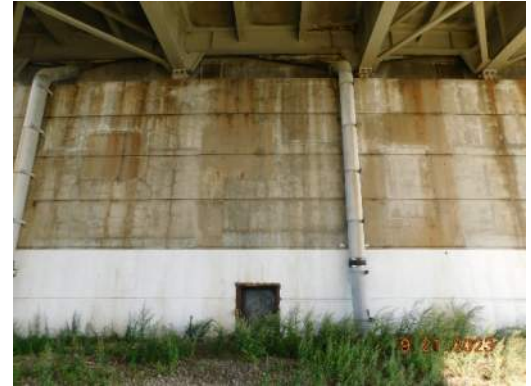
South abutment stem wall, middle section
