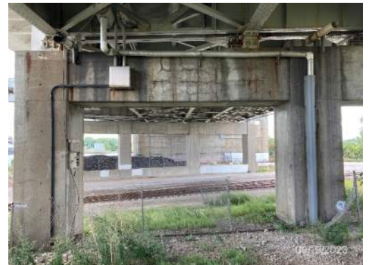
Pier 8 drainage troughs and piping
