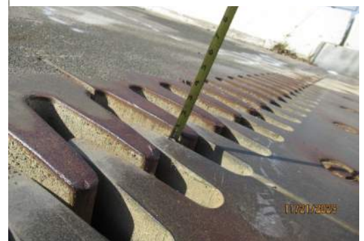
South abutment finger joint, SB right lane
