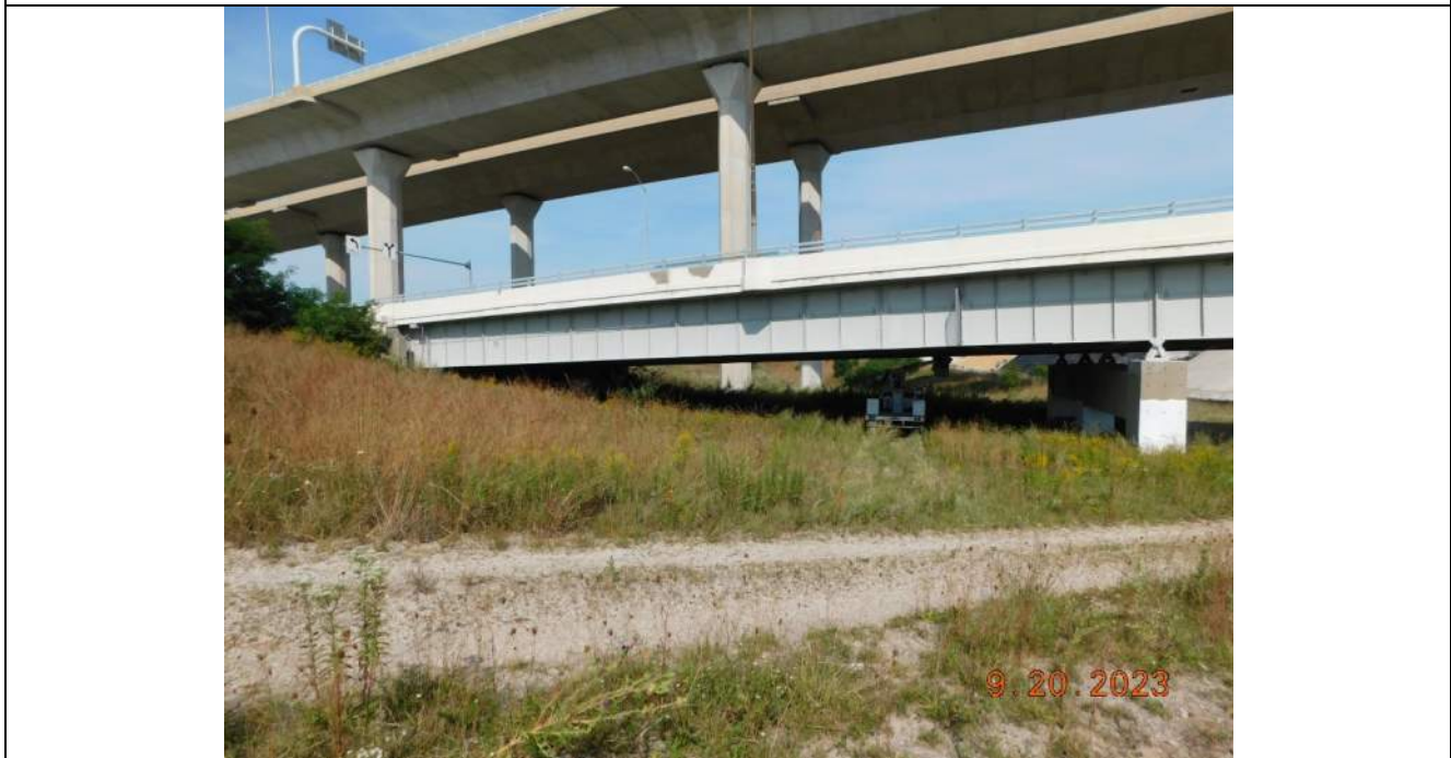
Photo S-80 - [Span 10] -West fascia, general view, Looking East
