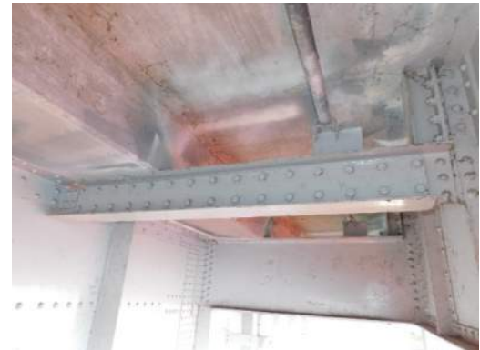
Span 6 East sidewalk repair between FB1s and FB2s
