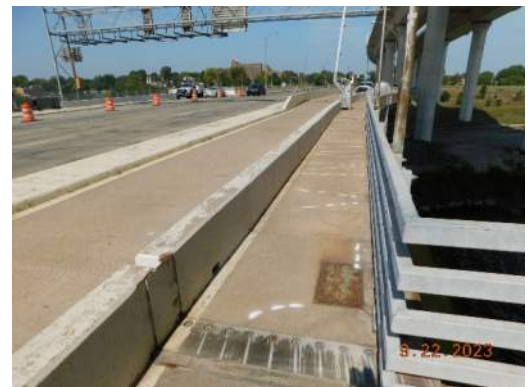
Span 6 East sidewalk
