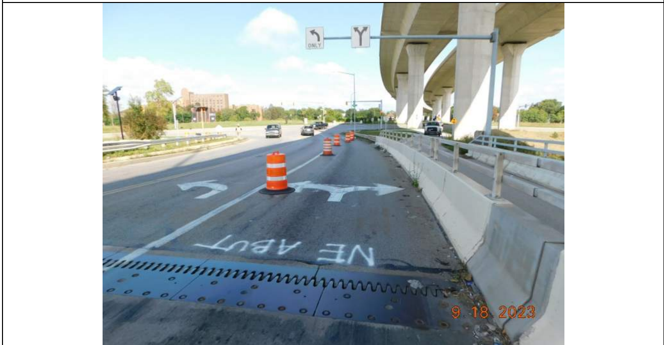
Photo S-8 - [North Approach] -View off of structure, Looking North
