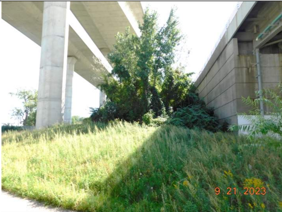
Photo S-30 - [South Approach] -Southeast approach slope, general view, Looking South
