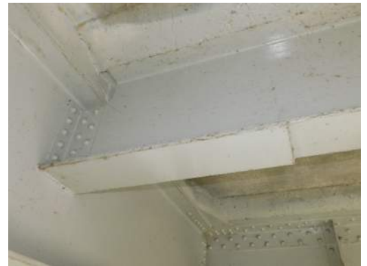
Span 2 Stringer 6W at FB15s typical connection
