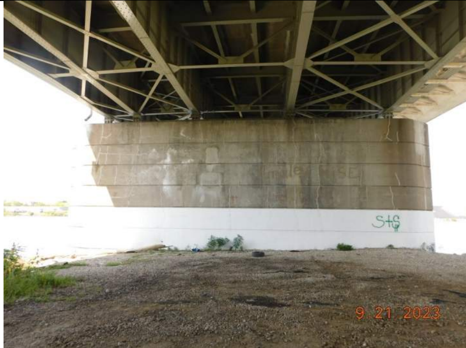
Photo S-285 - [Pier 1] -Pier South face, general view, Looking North
