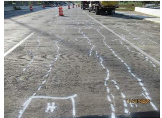
South approach concrete slab, SB lanes
