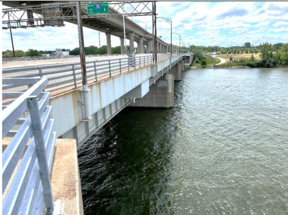
Photo S-4 - [Span 3W] -Feature Under - Maumee River, West side Looking South
