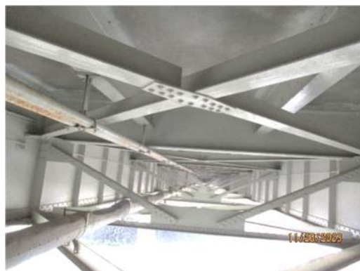
Span 9 typical bracing in good condition
