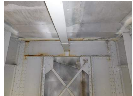
Span 6 FB0s at Pier 5, web SL and holes
