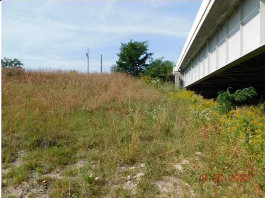
Photo S-31 - [North Approach] -Northwest approach slope, general view, Looking North
