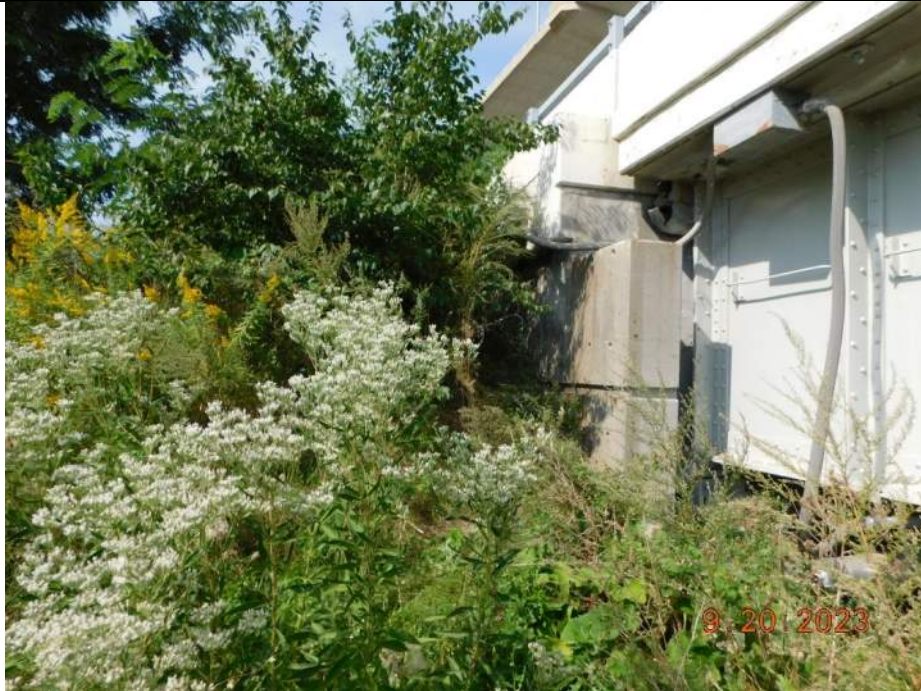
Photo S-283 - [North Abutment] -Abutment West wingwall, Looking North
