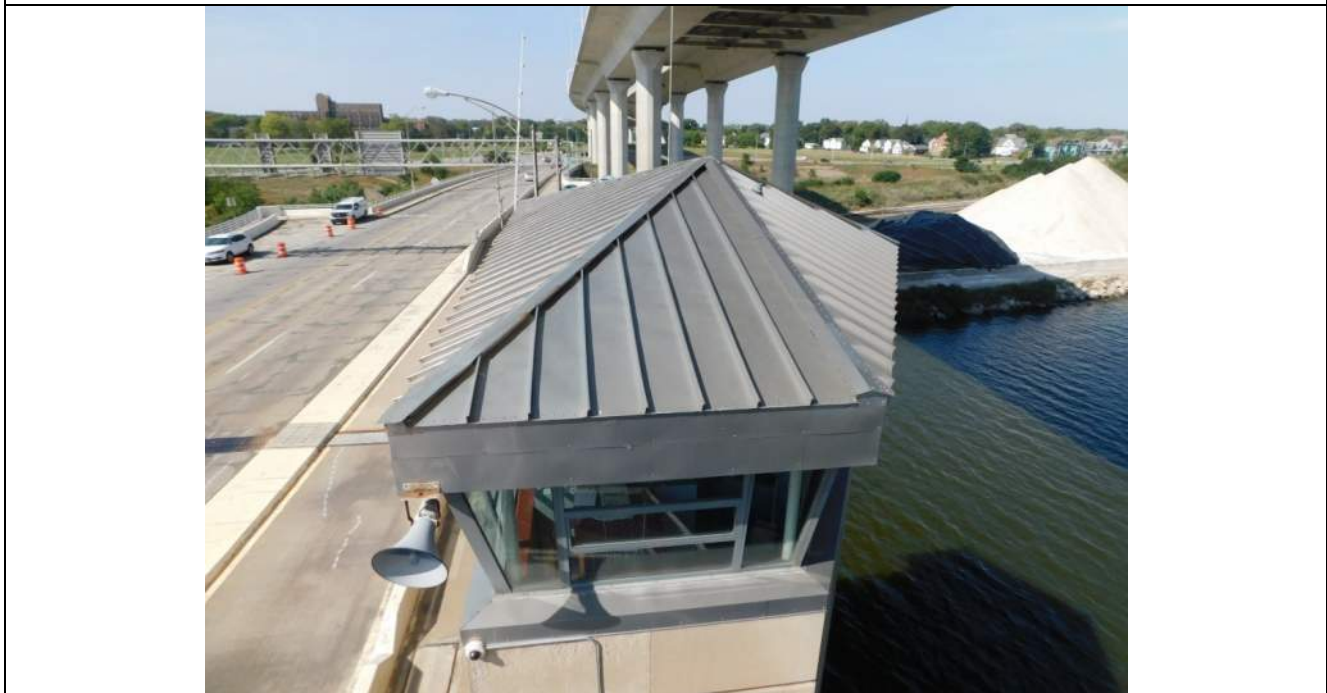
Photo S-372 - [Control House Exterior] -Roof general view, Looking North
