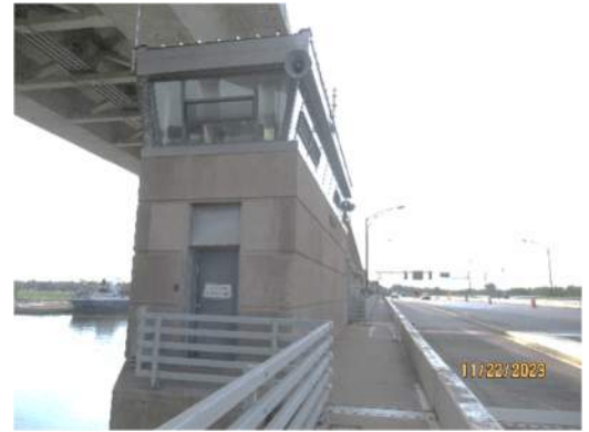
Pier 5, Operator house and roadway access
