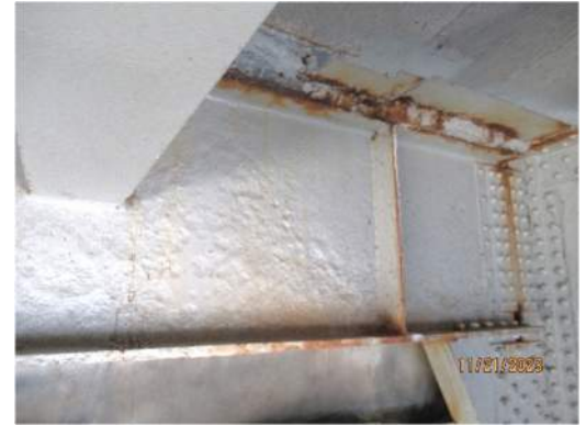
Span 1 FB0s at South abutment, web SL
