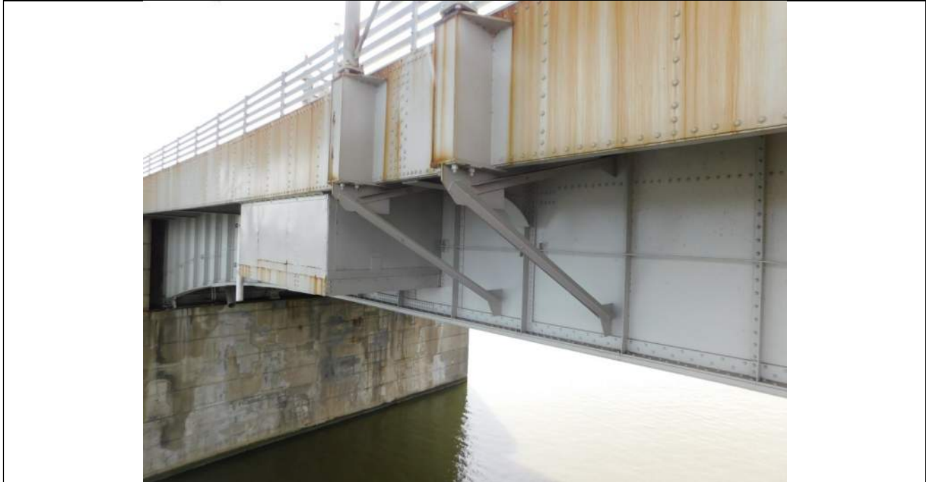
Photo S-73 - [Span 6] -East fascia and framing, general view, Looking Southwest
