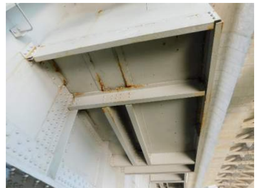
Span 4 East side swing gate support & housing at G4W
