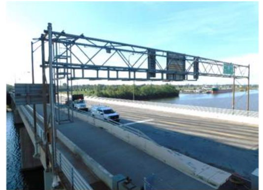
Span 4 sign gantry north elevation
