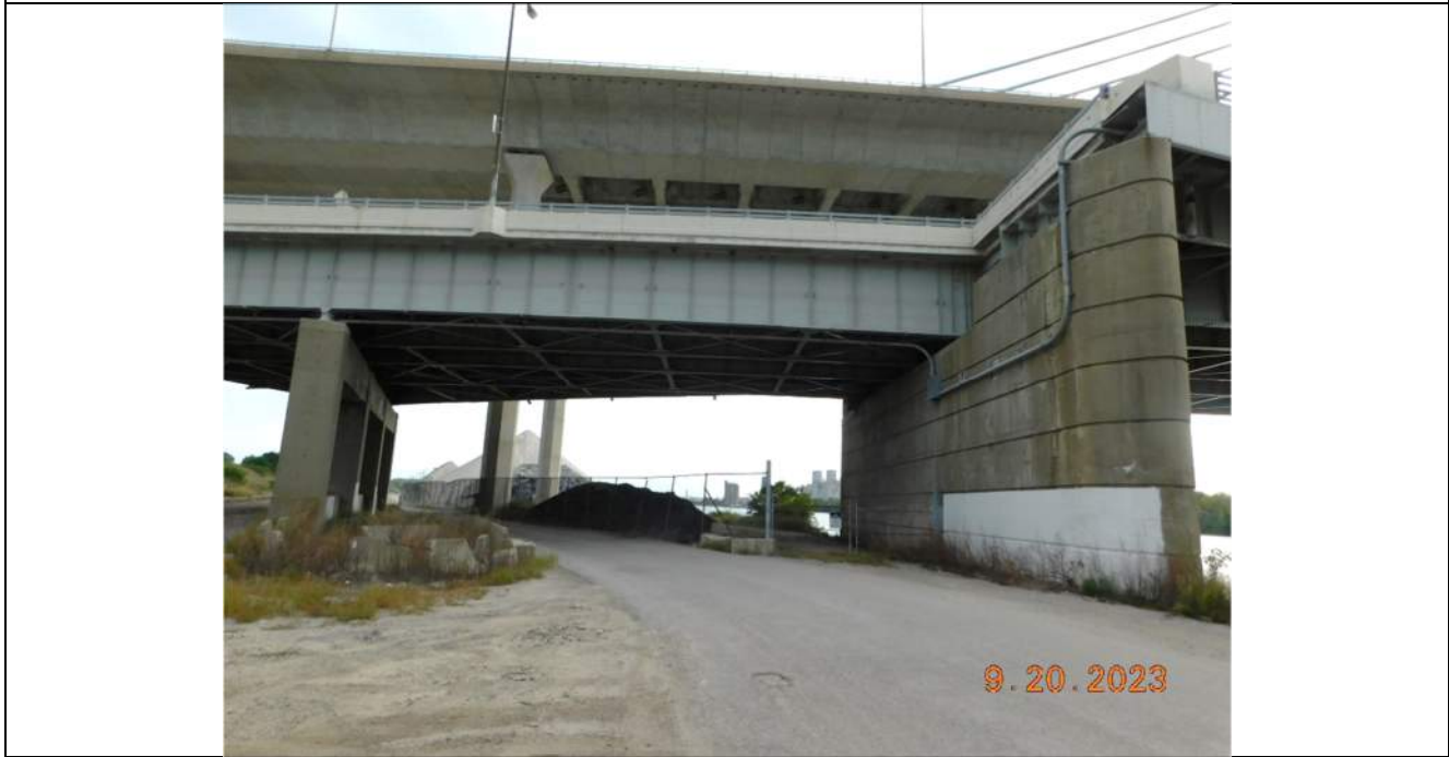
Photo S-74 - [Span 7] -West fascia, general view, Looking East
