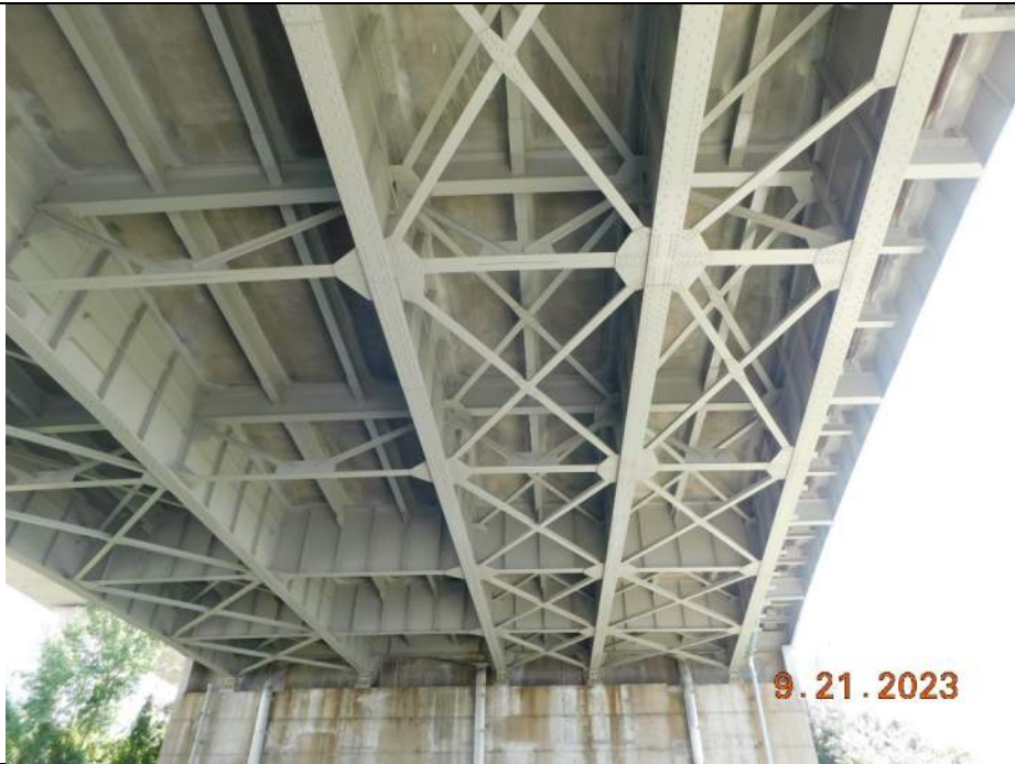
Photo S-162 - [Span 1] -Span framing and underside general view, Looking North
