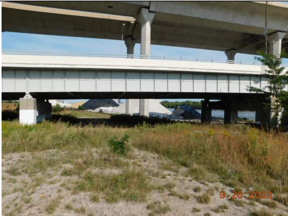
Photo S-78 - [Span 9] -West fascia, general view, Looking East
