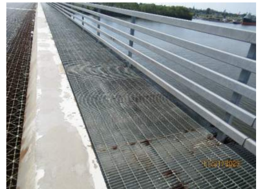
Span 5 North leaf West sidewalk
