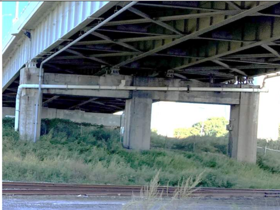
Photo S-310 - [Pier 8] -Pier South face, general view, Looking North
