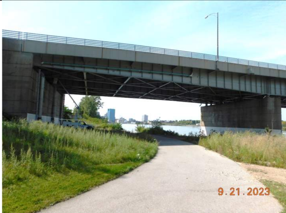
Photo S-69 - [Span 1] -East fascia, general view, Looking West
