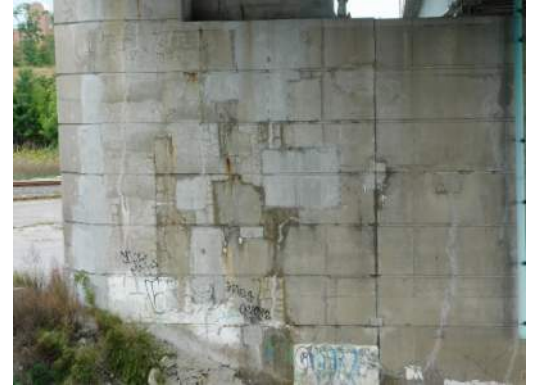
Pier 6, South side detail view, West side
