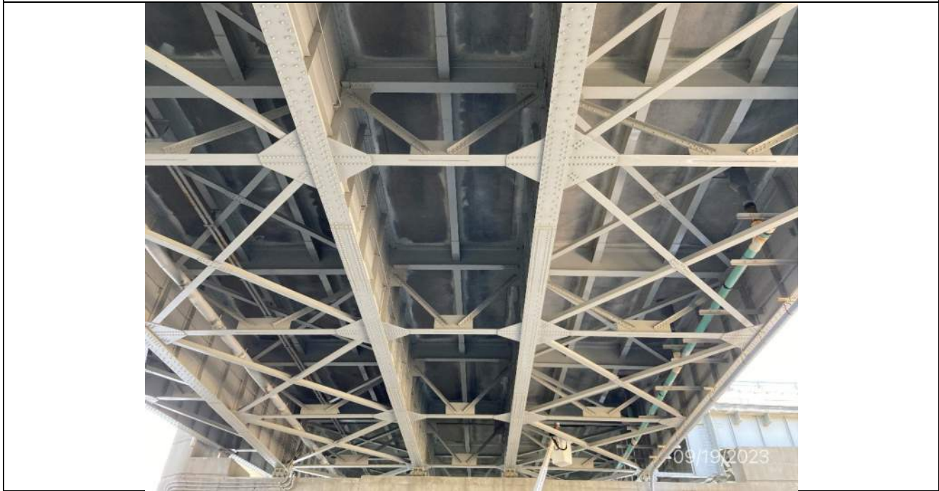
Photo S-168 - [Span 7] -Span framing and underside general view, Looking South
