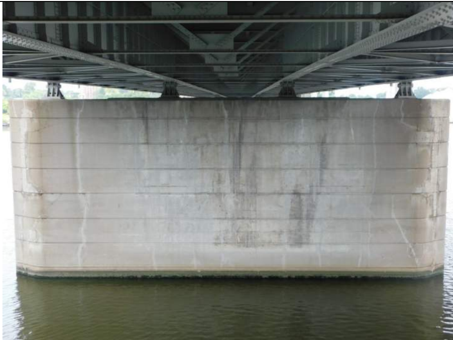
Photo S-288 - [Pier 2] -Pier South face, general view, Looking North
