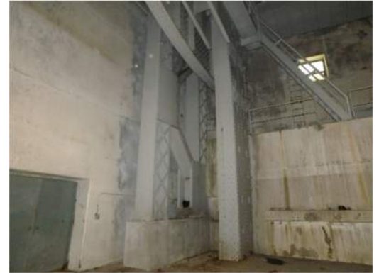
Pier 4 Trunnion Tower 1W lower portion
