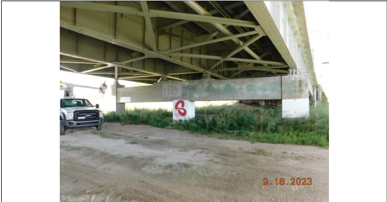
Photo S-313 - [Pier 9] -Pier South face, general view, Looking North
