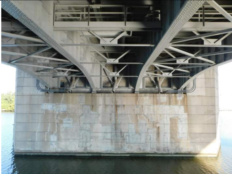
Photo S-293 - [Pier 4] -Pier South face, general view, Looking North
