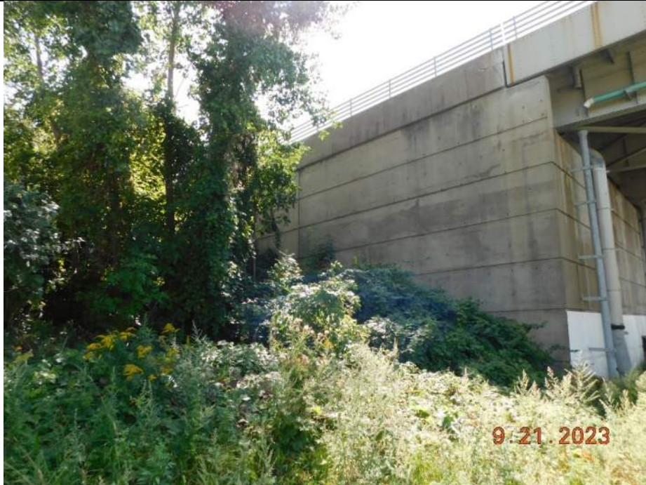
Photo S-277 - [South Abutment] -Abutment East wingwall, Looking Southwest
