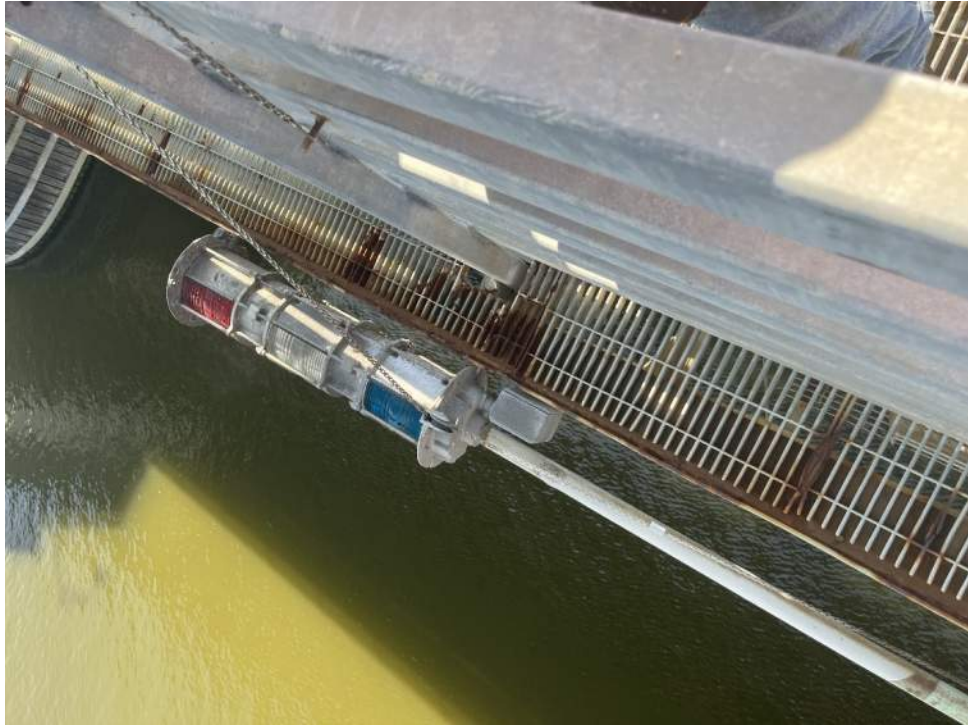
Photo E-23: Southeast Navigation Light
