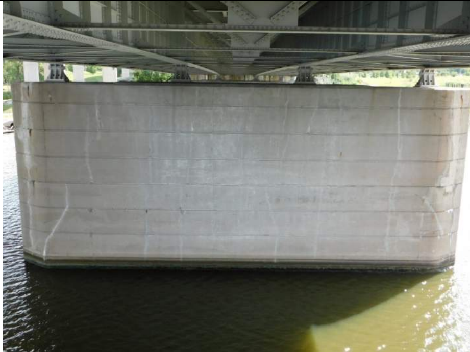
Photo S-289 - [Pier 2] -Pier North face, general view, Looking South
