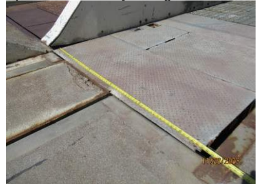
Span 5 South leaf East sidewalk joint cover at rear break joint
