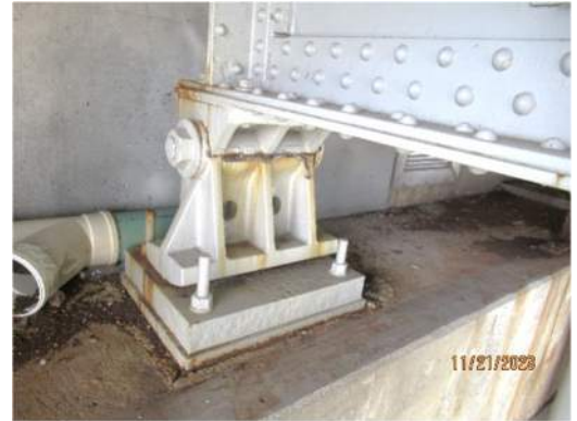
South abutment Rocker Bearing 4W
