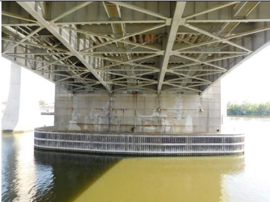
Photo S-294 - [Pier 4] -Pier North face, general view, Looking South
