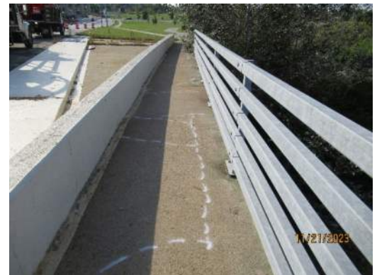
Southwest sidewalk, barrier, railing
