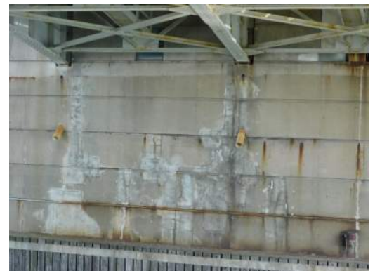
Pier 4 North face detail view, East side
