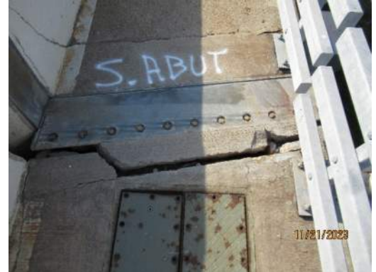
South abutment joint, West sidewalk
