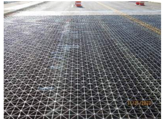
Grid deck north leaf, SB lanes
