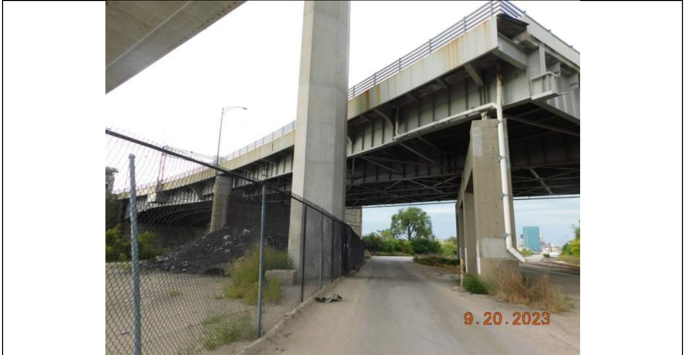
Photo S-75 - [Span 7] -East fascia, general view, Looking West
