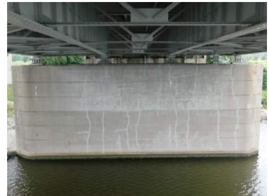
Pier 1 North face, crack repairs throughout
