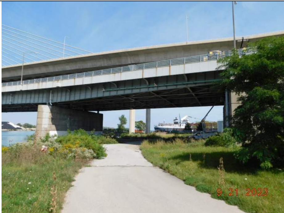
Photo S-68 - [Span 1] -West fascia, general view, Looking East
