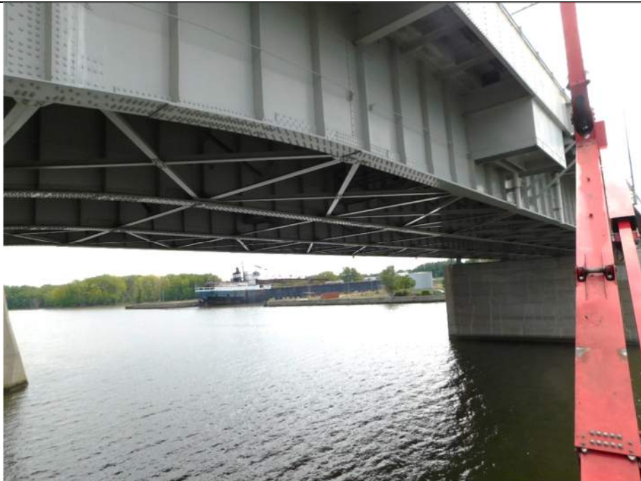
Photo S-164 - [Span 4] -Span framing and underside general view, Looking Southeast
