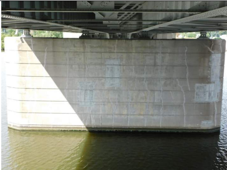
Photo S-290 - [Pier 3] -Pier South face, general view, Looking North
