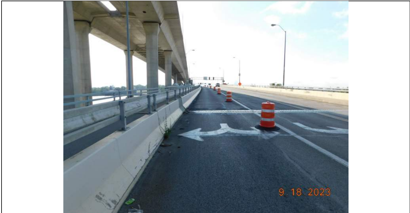
Photo S-7 - [North Approach] -View onto structure from North Approach, Looking South
