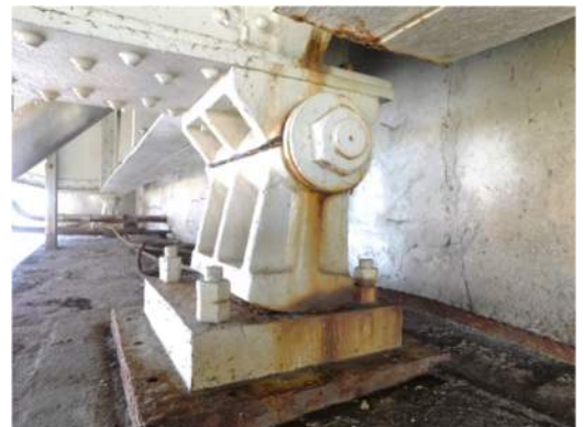
Pier 5 (north side) Rocker Bearing 3W
