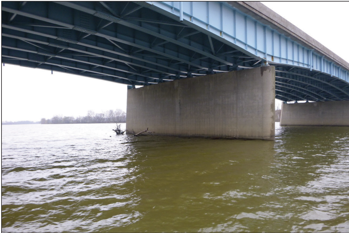
Photograph No. 16: View of the South Face of Pier 4, Looking Northwest.
