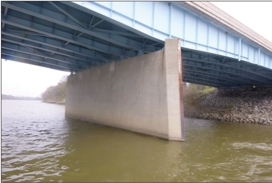
Photograph No. 17: View of the North Face of Pier 5, Looking Southeast.
