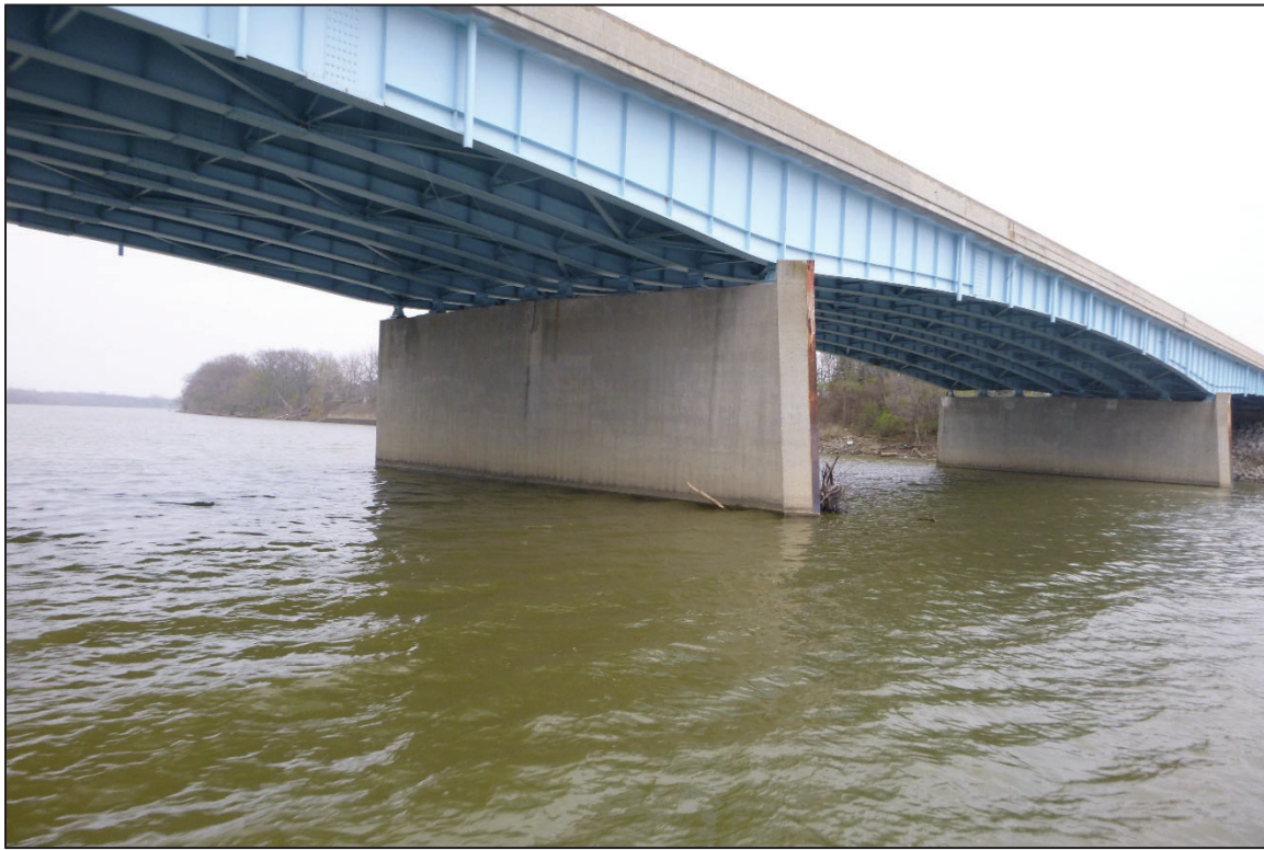
Photograph No. 15: View of the North Face of Pier 4, Looking Southeast.
