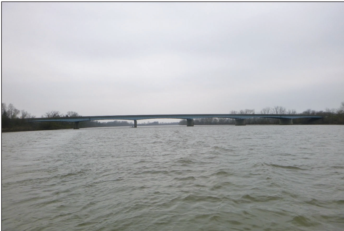
Photograph No. 2: Overall View of Structure No. 3500578 (HEN-6-1650), Looking West.
