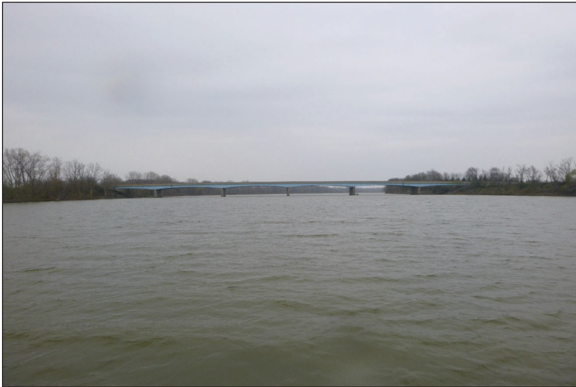
Photograph No. 1: Overall View of Structure No. 3500578 (HEN-6-1650), Looking East.
