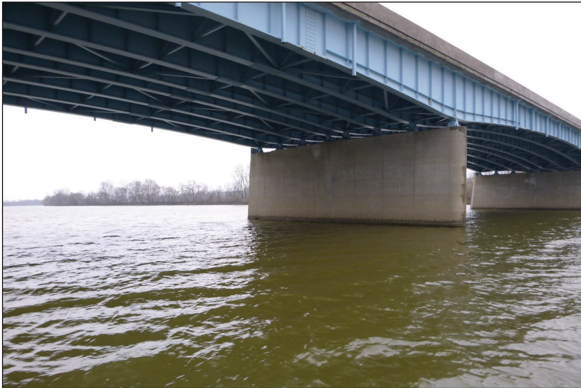
Photograph No. 14: View of the South Face of Pier 3, Looking Northwest.
