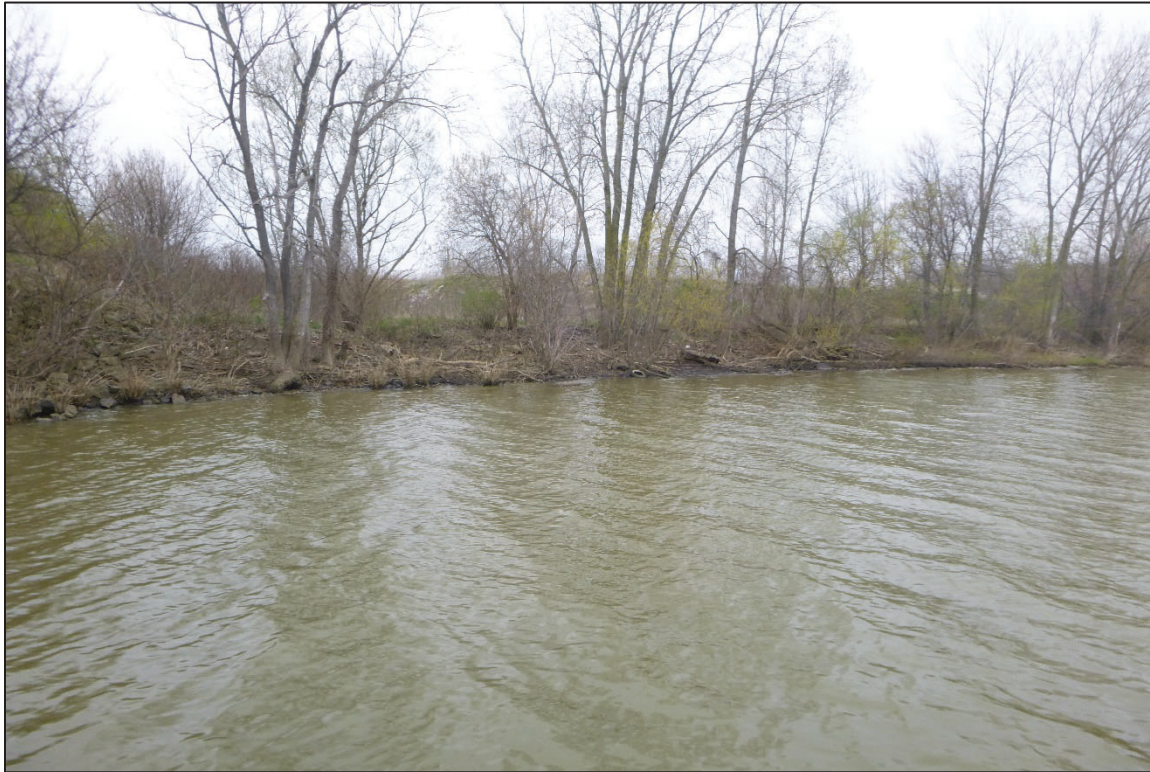
Photograph No. 5: View of the North Embankment Downstream of the Structure, Looking Northeast.
