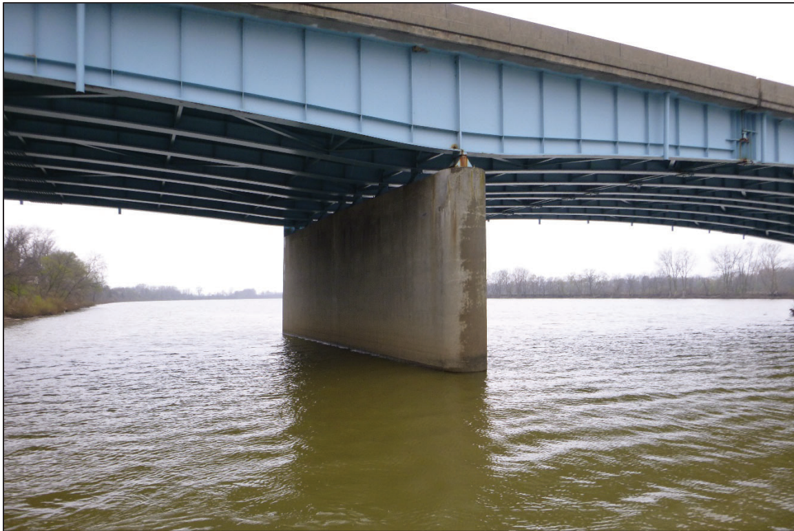
Photograph No. 18: View of the South Face of Pier 5, Looking Northwest.
