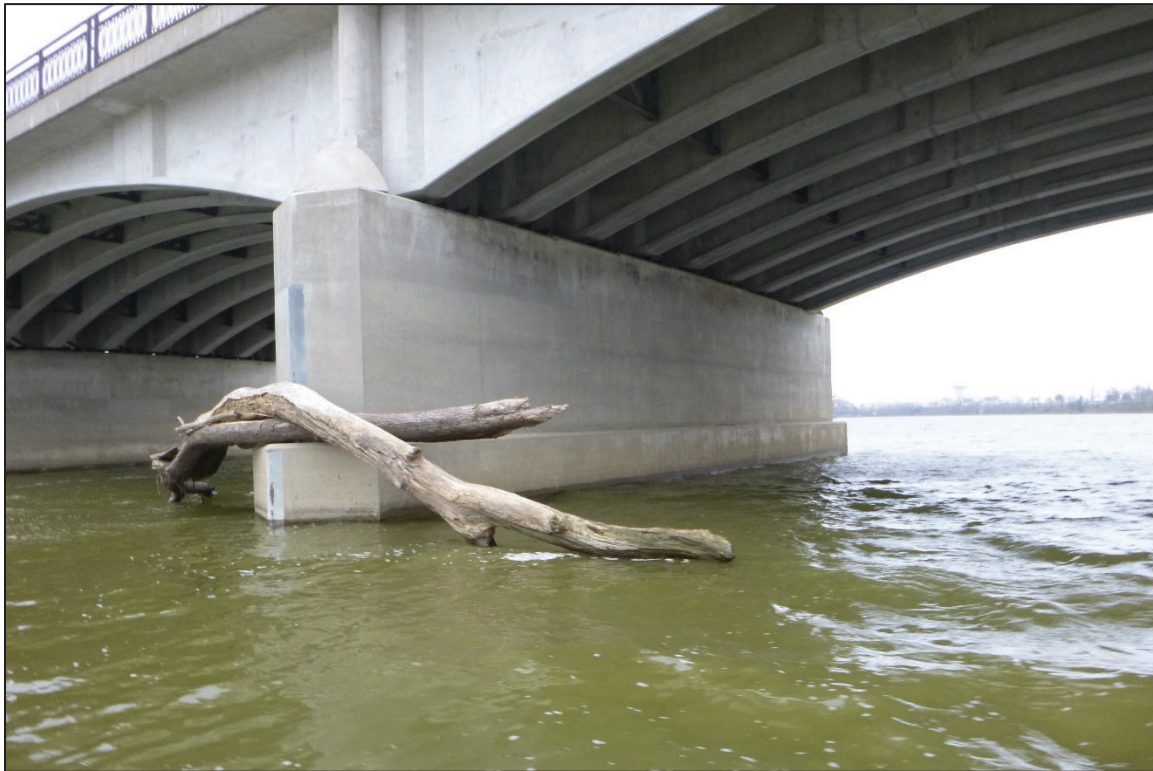
Photograph No. 12: View of the South Face of Pier 2, Looking Northeast.
