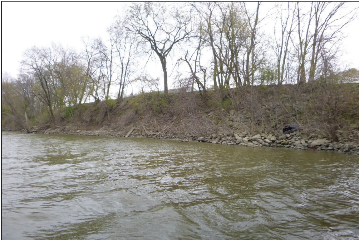
Photograph No. 8: View of the South Embankment Downstream of the Structure, Looking Southeast.
