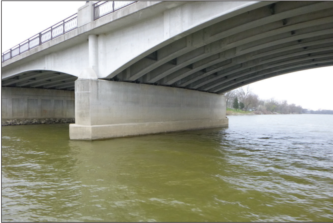
Photograph No. 9: View of the North Face of Pier 1, Looking Southwest.
