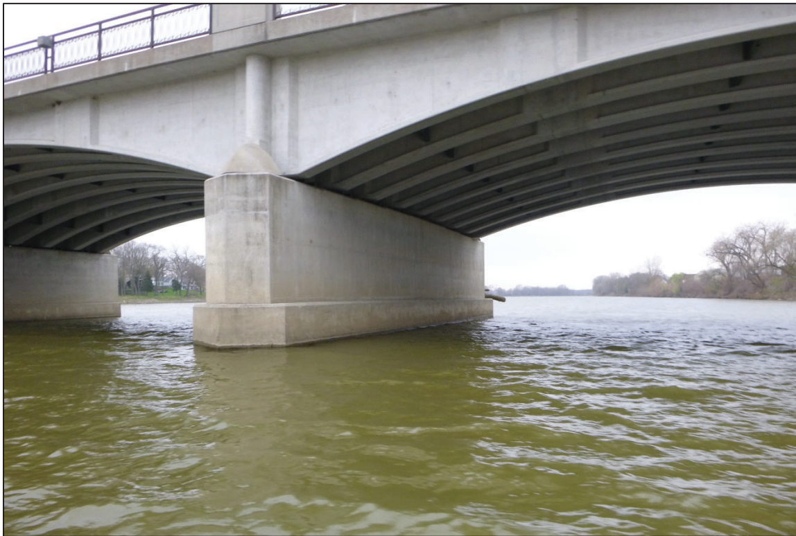
Photograph No. 18: View of the North Face of Pier 5, Looking Southwest.
