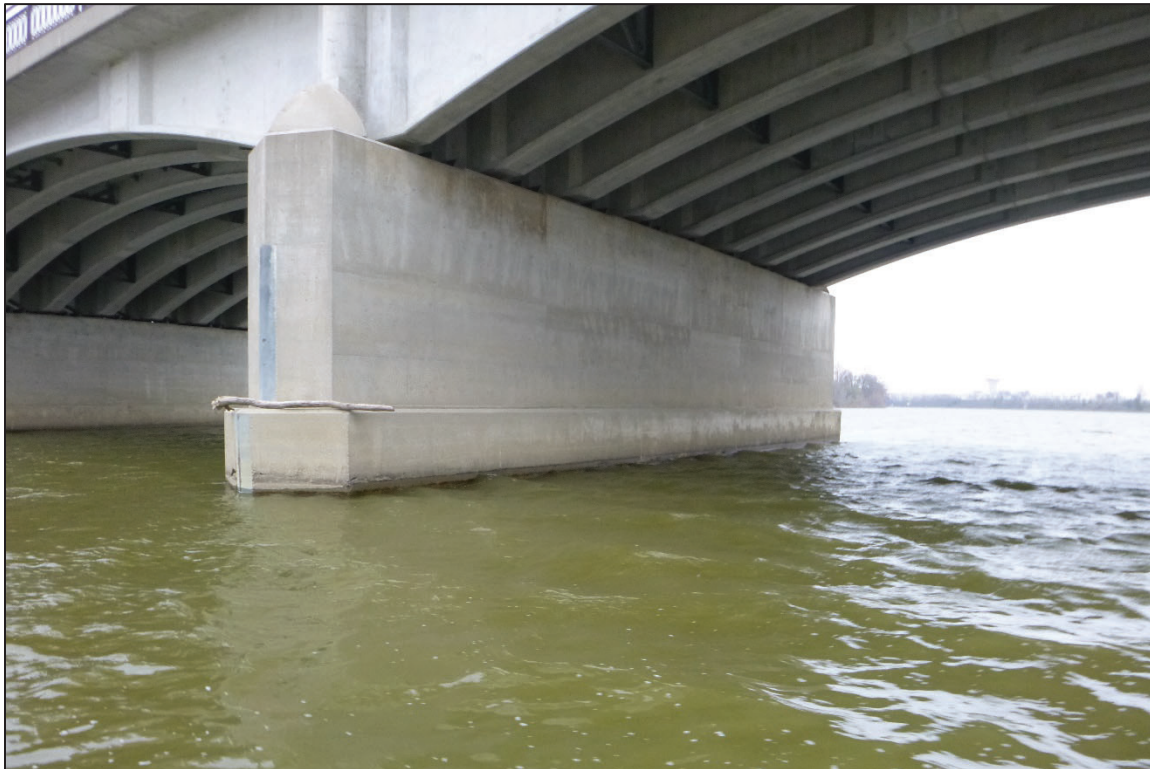
Photograph No. 14: View of the South Face of Pier 3, Looking Northeast.
