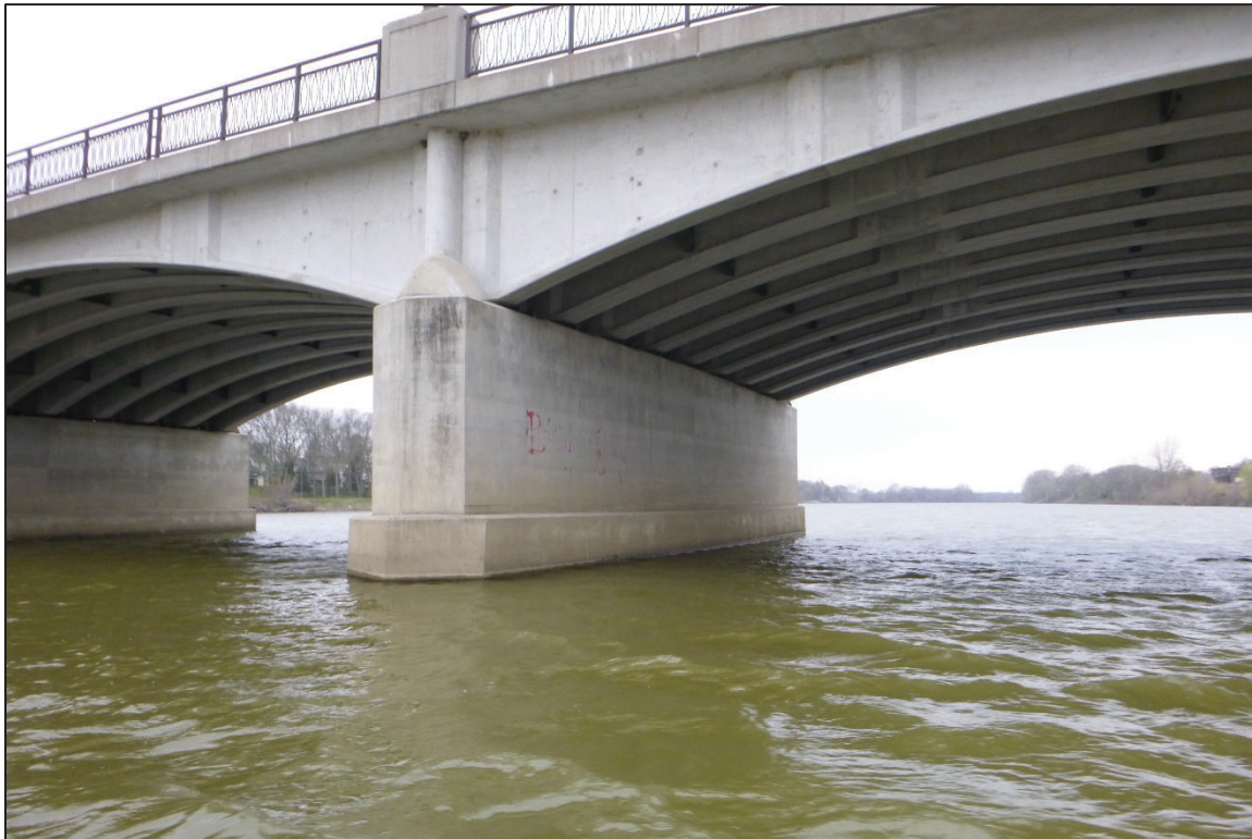
Photograph No. 16: View of the North Face of Pier 4, Looking Southwest.
