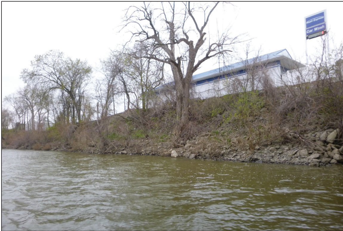
Photograph No. 3: View of the North Embankment Upstream of the Structure, Looking Northwest.
