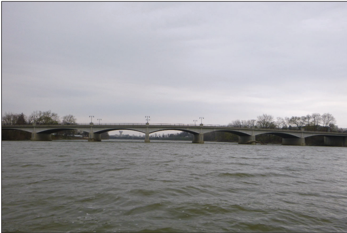
Photograph No. 1: Overall View of Structure No. 3502384 (HEN-108-1561), Looking East.
