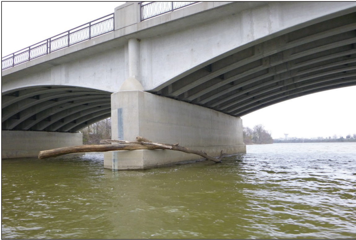
Photograph No. 19: View of the South Face of Pier 5, Looking Northeast.
