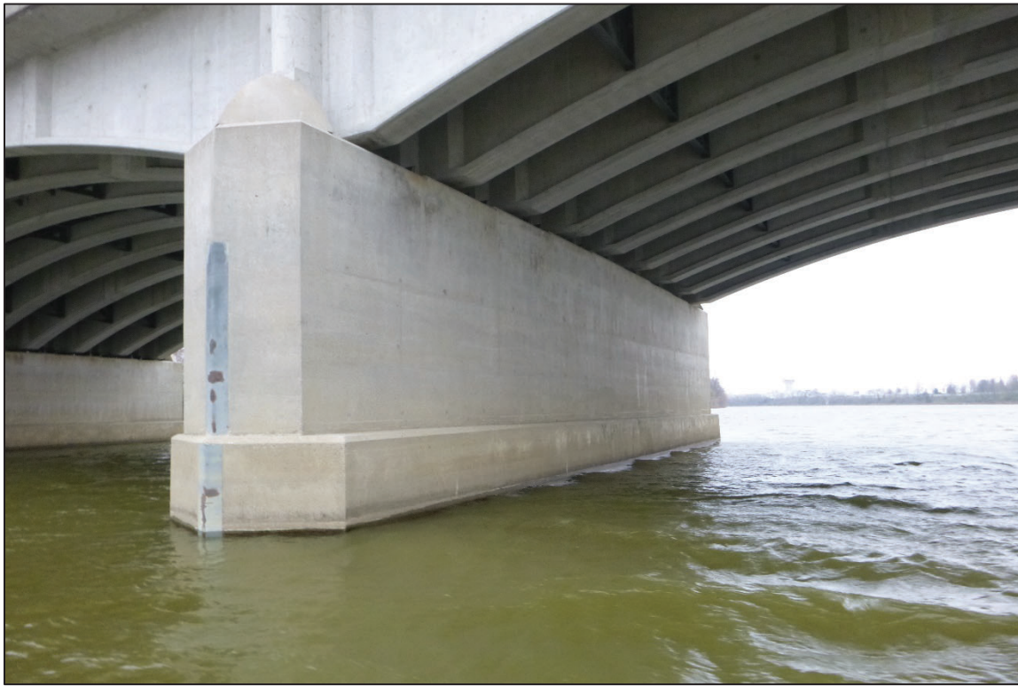
Photograph No. 17: View of the South Face of Pier 4, Looking Northeast.
