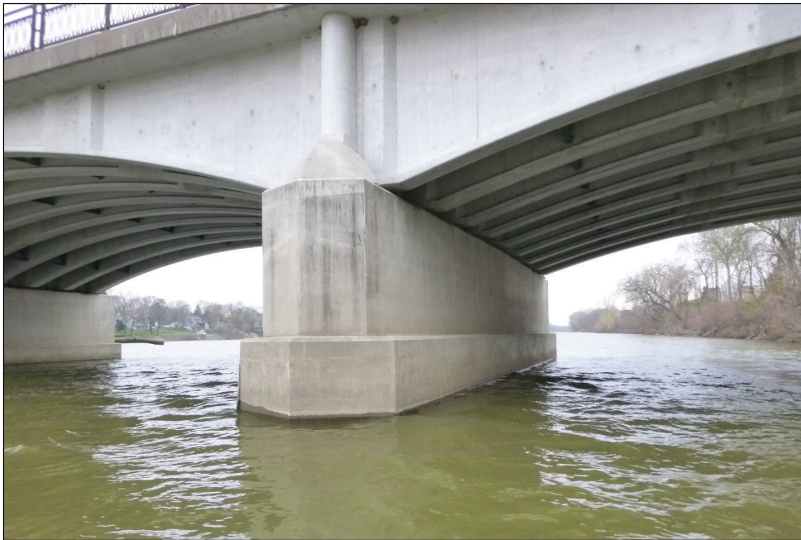
Photograph No. 20: View of the North Face of Pier 6, Looking Southwest.
