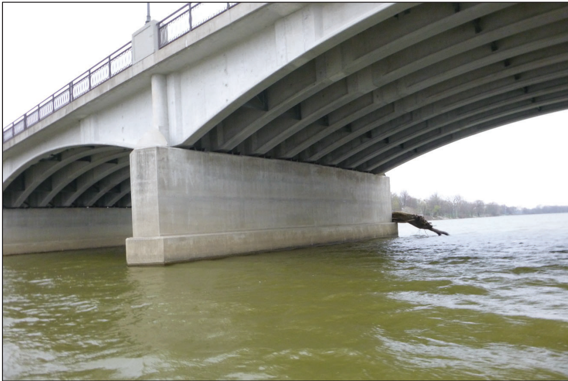
Photograph No. 11: View of the North Face of Pier 2, Looking Southwest.
