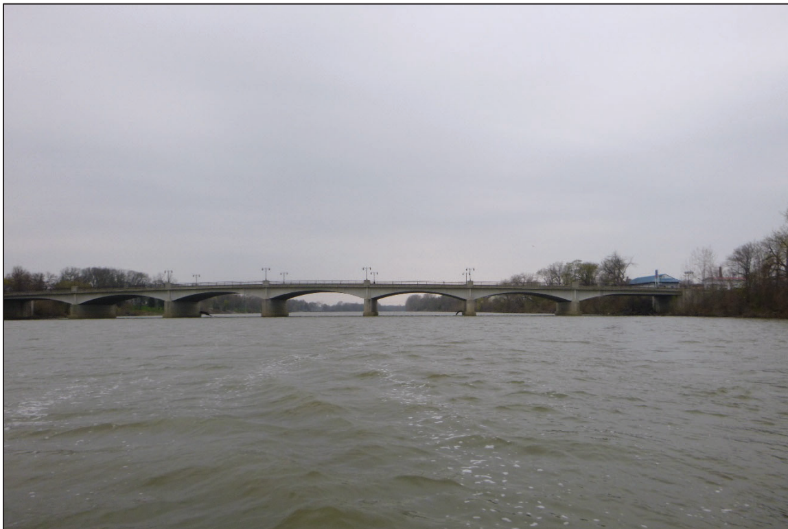
Photograph No. 2: Overall View of Structure No. 3502384 (HEN-108-1561), Looking West.
