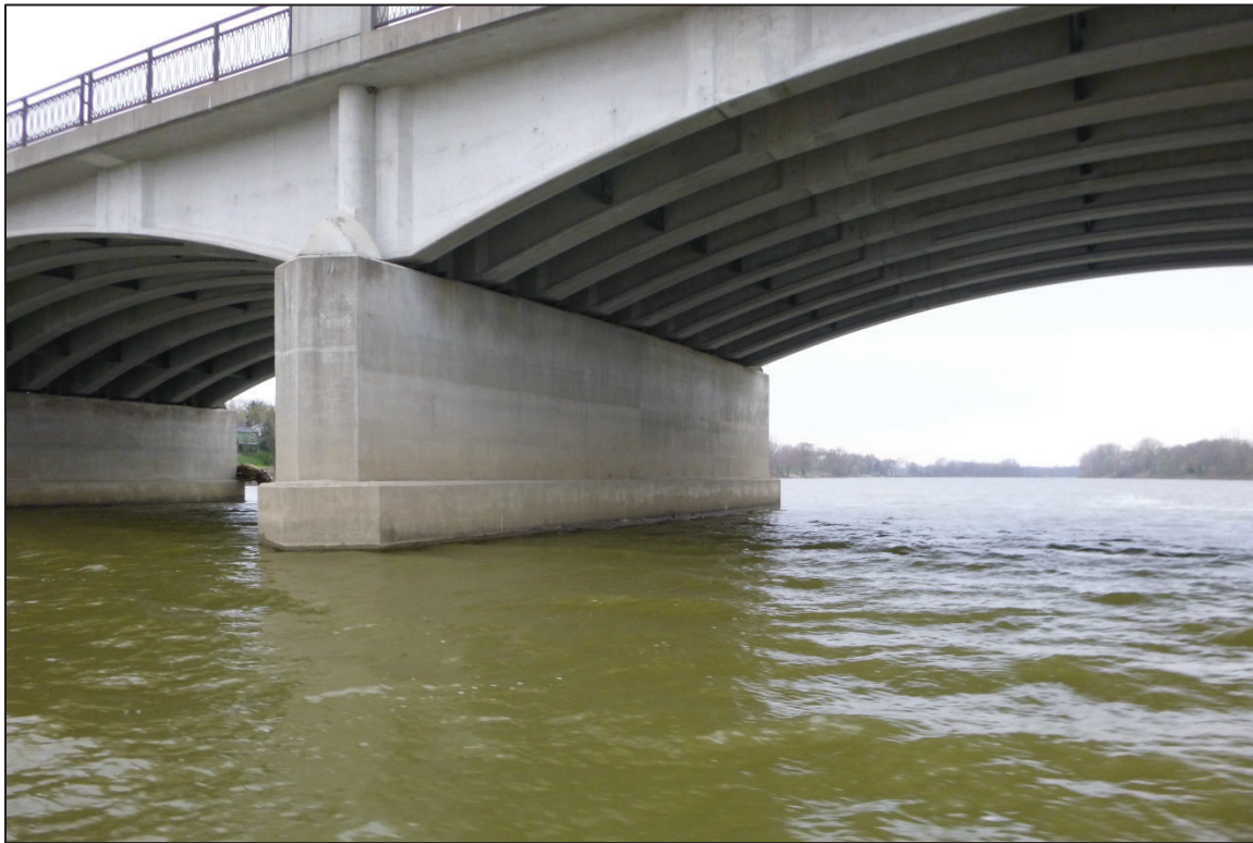
Photograph No. 13: View of the North Face of Pier 3, Looking Southwest.
