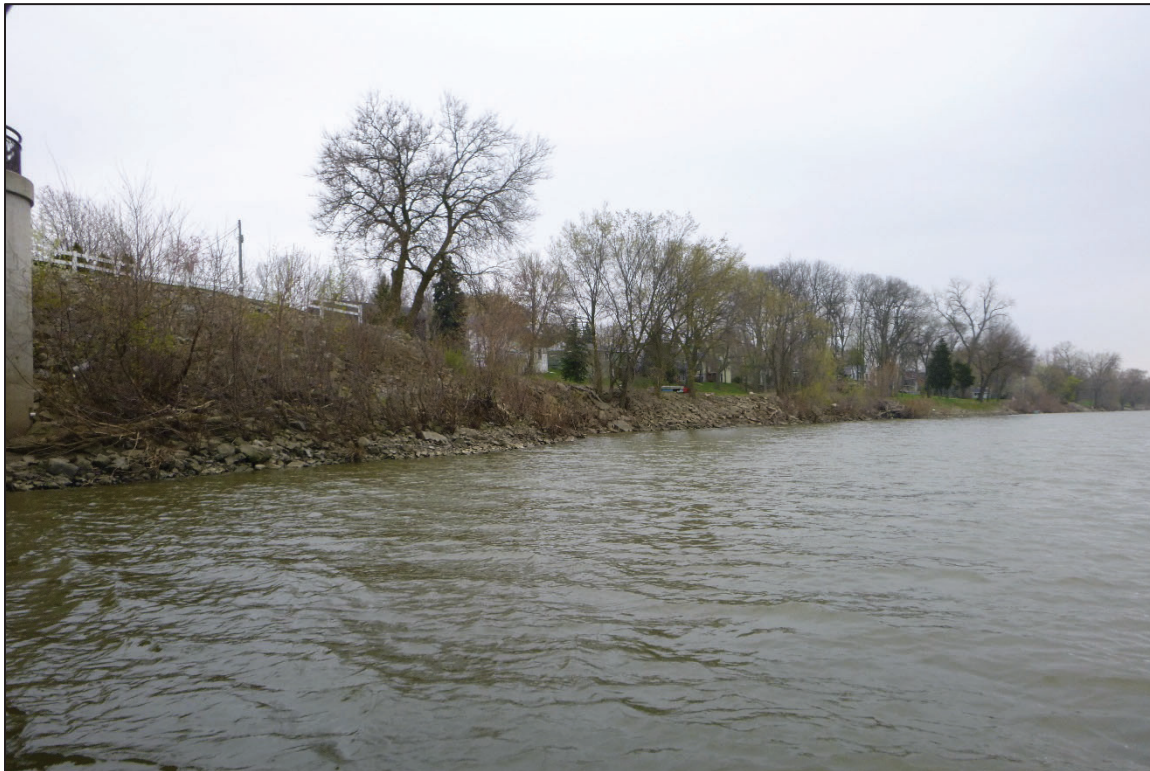
Photograph No. 6: View of the South Embankment Upstream of the Structure, Looking Southwest.
