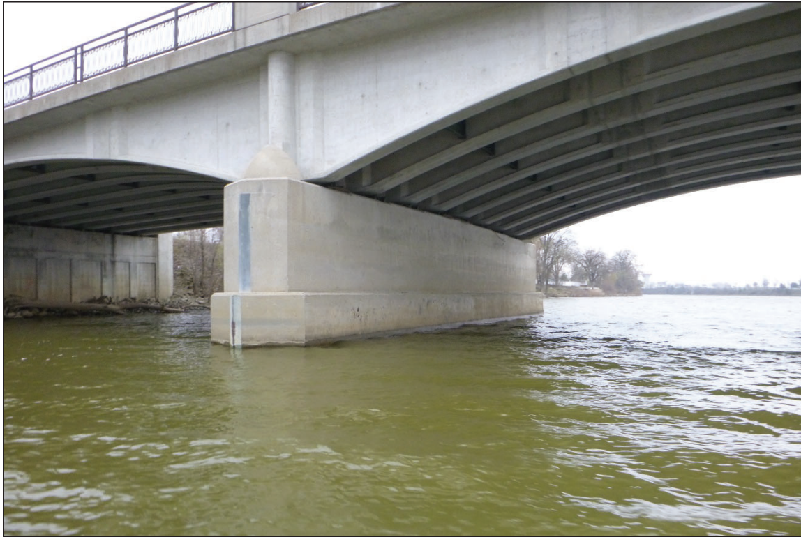
Photograph No. 21: View of the South Face of Pier 6, Looking Northeast.
