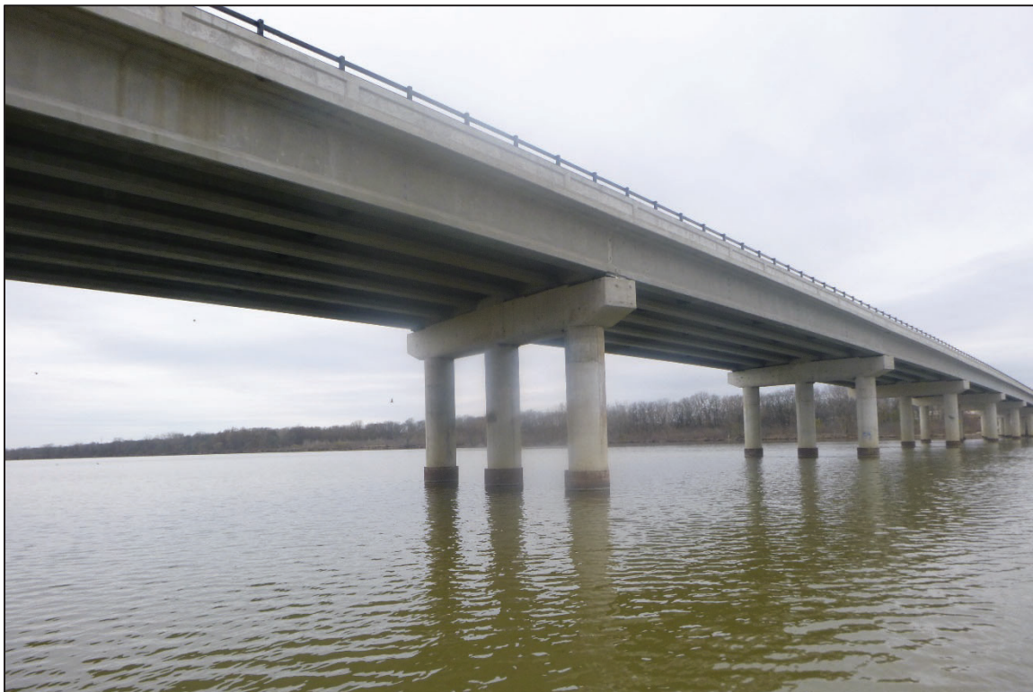
Photograph No. 14: View of the South Face of Bent 3, Looking Northwest.
