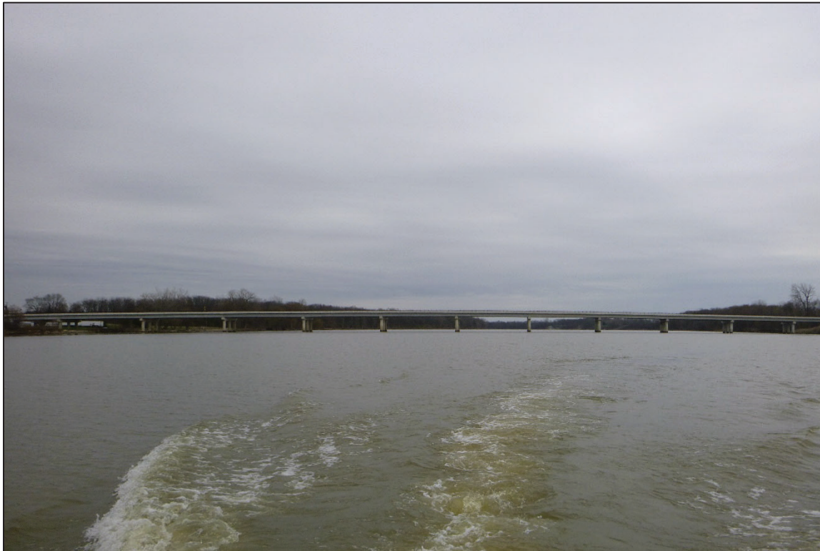
Photograph No. 2: Overall View of Structure No. 3502392 (HEN-109-1820), Looking East.
