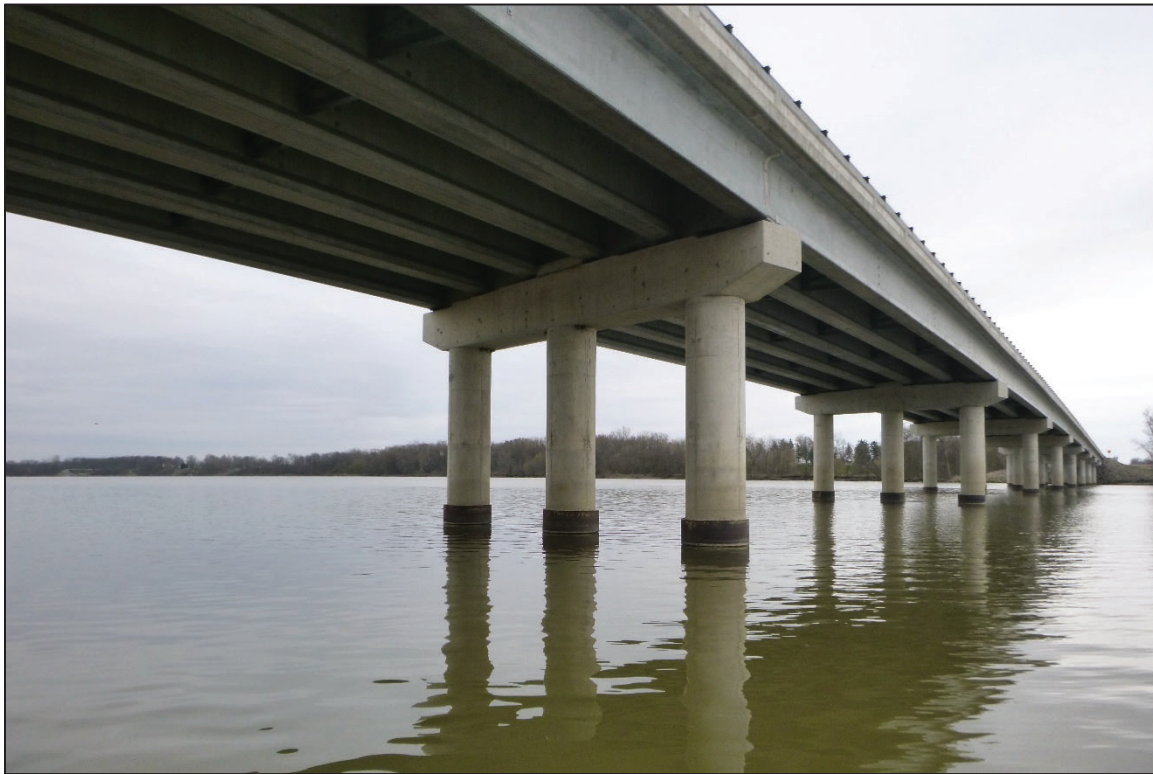
Photograph No. 23: View of the North Face of Bent 8, Looking Southeast.
