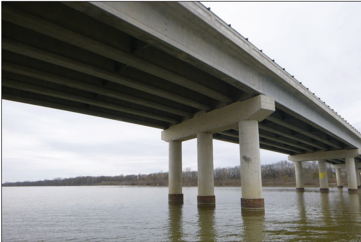
Photograph No. 18: View of the South Face of Bent 5, Looking Northwest.
