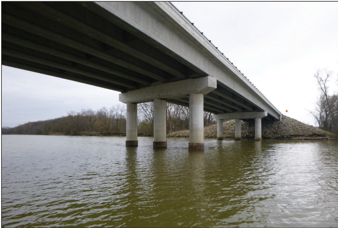
Photograph No. 11: View of the North Face of Bent 2, Looking Southeast.
