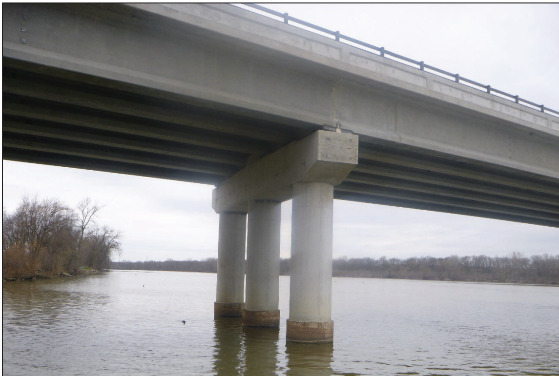
Photograph No. 10: View of the South Face of Bent 1, Looking Northwest.
