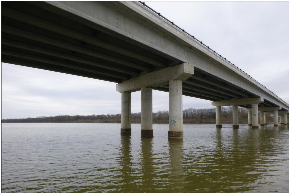
Photograph No. 16: View of the South Face of Bent 4, Looking Northwest.
