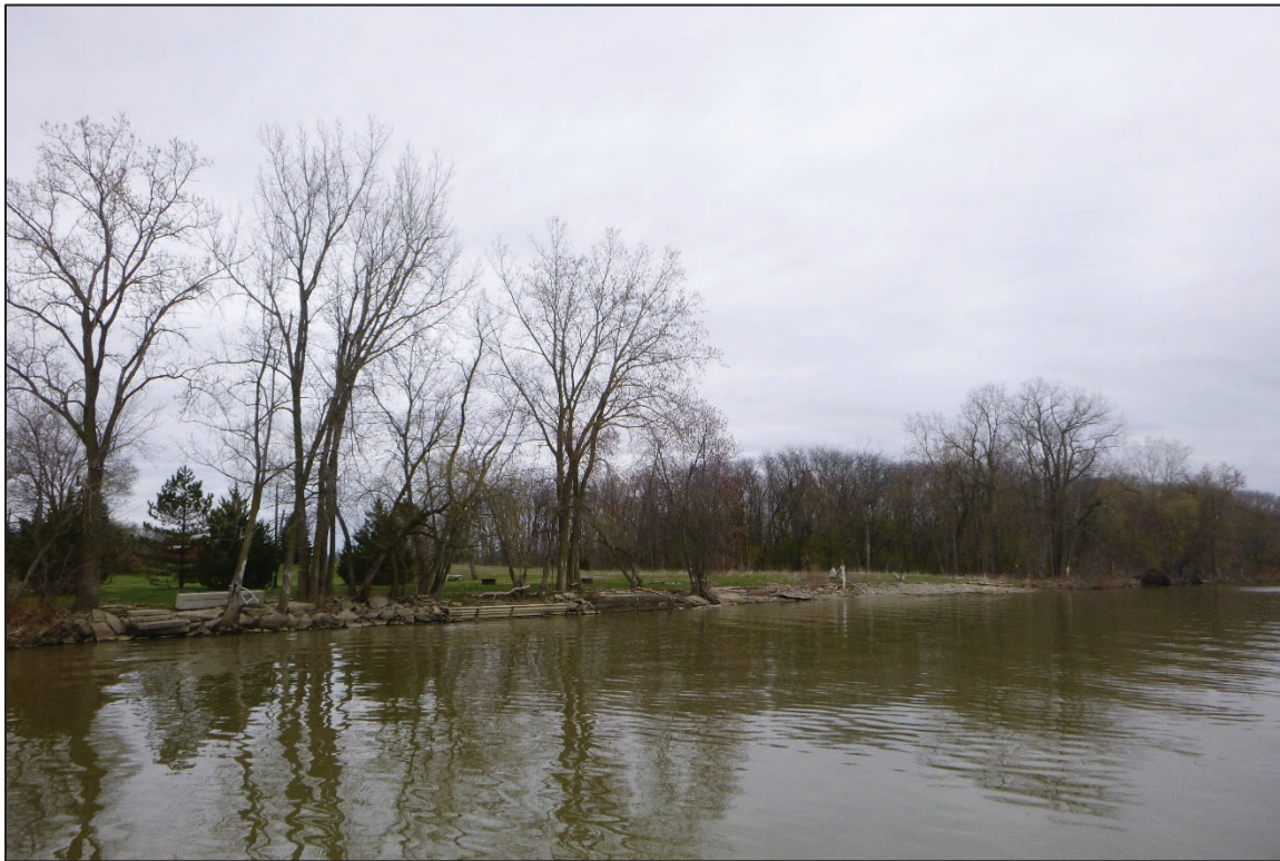
Photograph No. 5: View of the North Embankment Downstream of the Structure, Looking Northeast.
