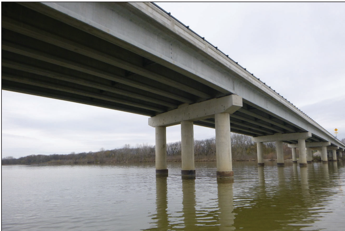
Photograph No. 22: View of the South Face of Bent 7, Looking Northwest.
