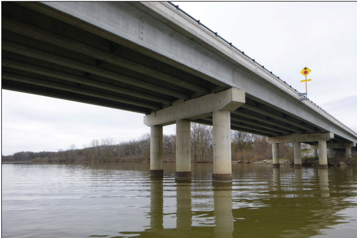
Photograph No. 26: View of the South Face of Bent 9, Looking Northwest.
