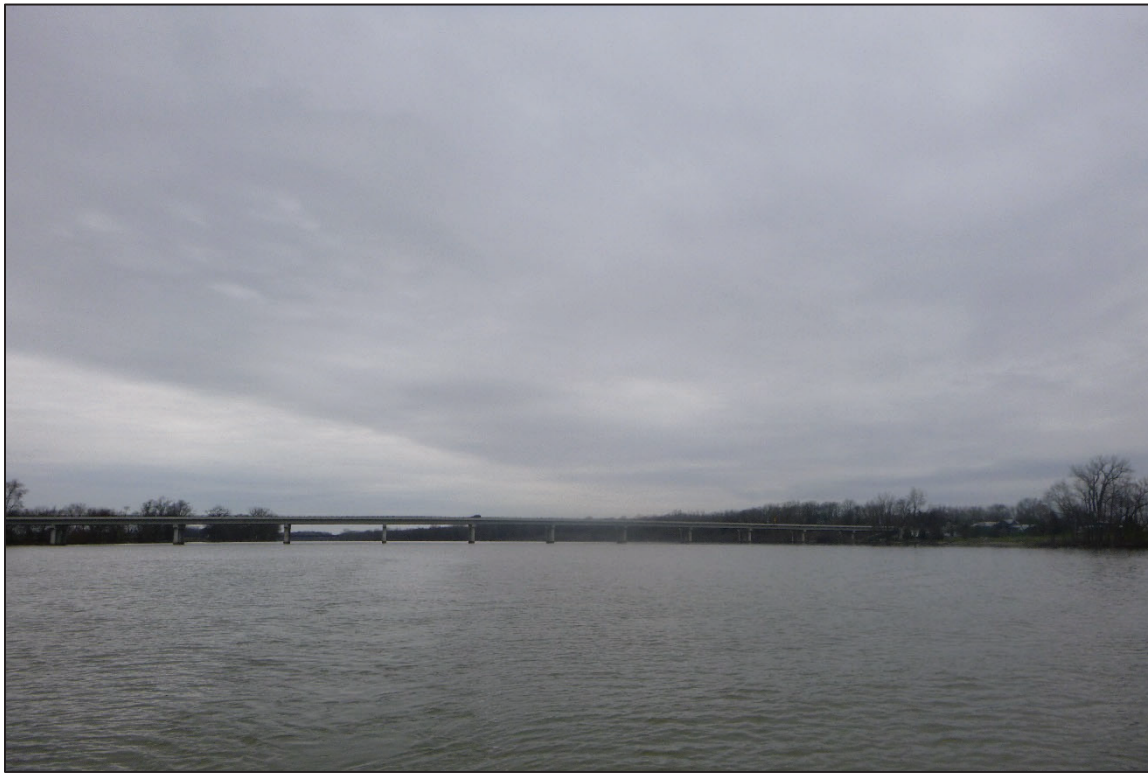
Photograph No. 1: Overall View of Structure No. 3502392 (HEN-109-1820), Looking West.
