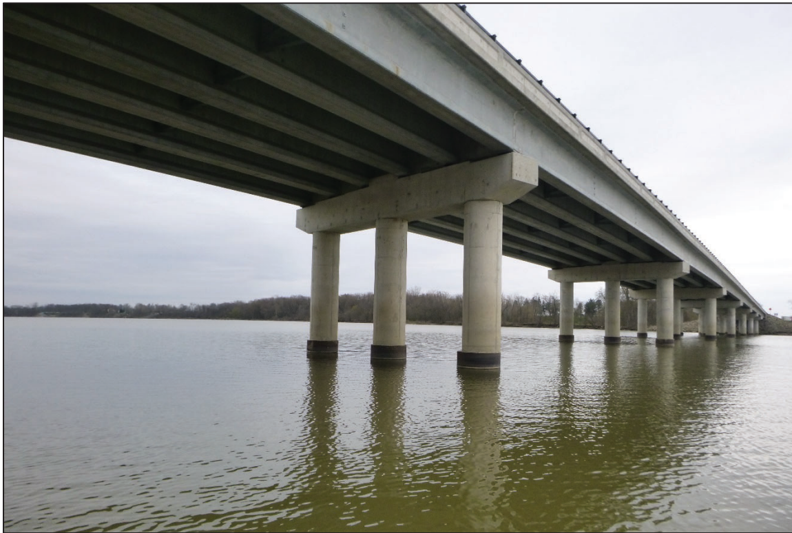
Photograph No. 21: View of the North Face of Bent 7, Looking Southeast.
