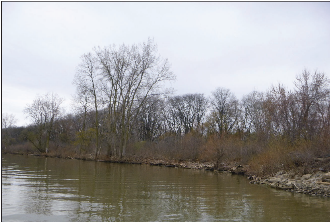
Photograph No. 3: View of the North Embankment Upstream of the Structure, Looking Northwest.
