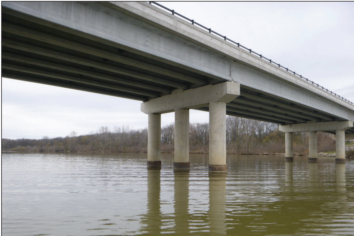
Photograph No. 24: View of the South Face of Bent 8, Looking Northwest.
