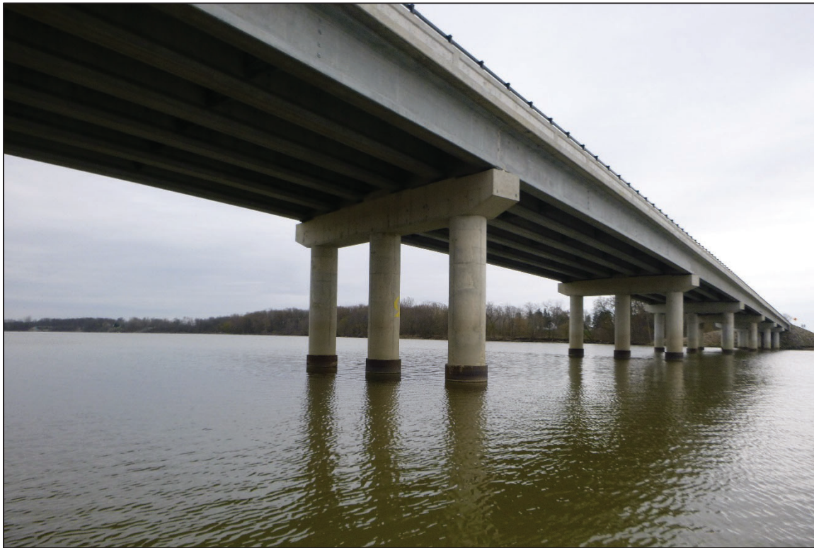
Photograph No. 19: View of the North Face of Bent 6, Looking Southeast.
