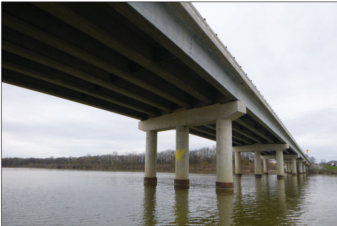
Photograph No. 20: View of the South Face of Bent 6, Looking Northwest.
