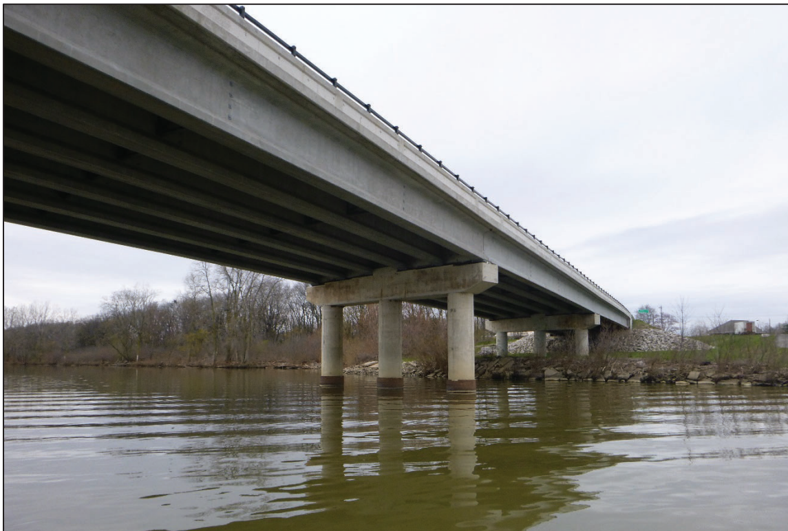
Photograph No. 28: View of the South Face of Bent 10, Looking Northwest.
