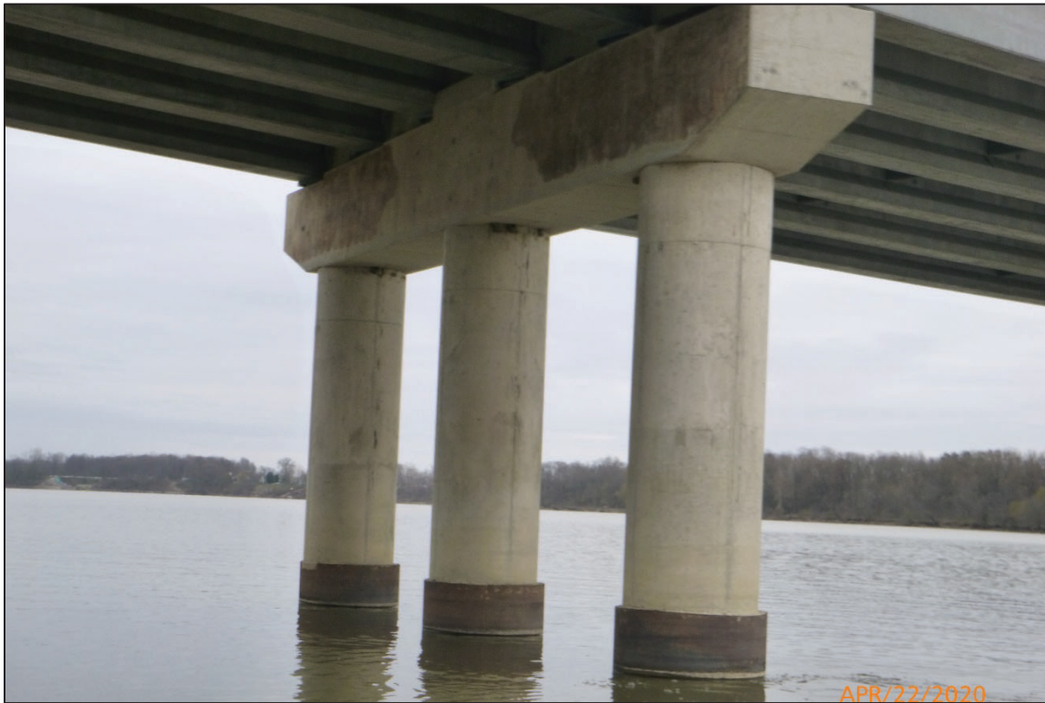
Photograph No. 27: View of the North Face of Bent 10, Looking Southeast.
