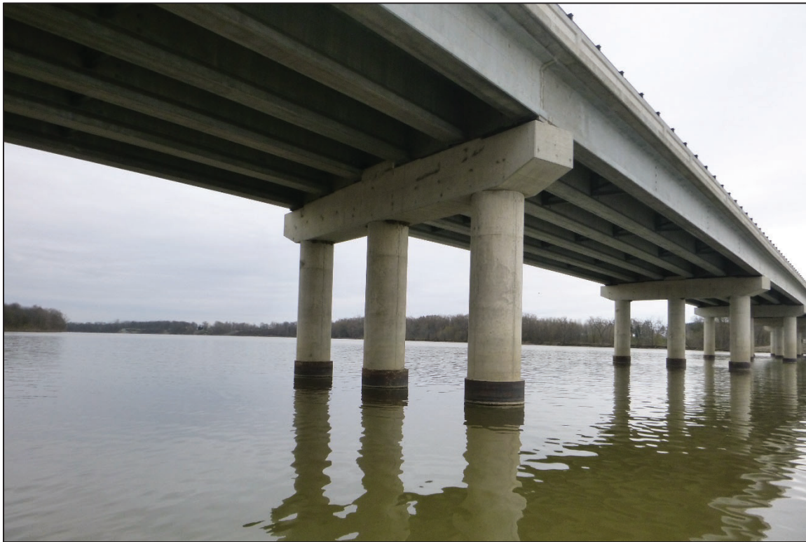
Photograph No. 25: View of the North Face of Bent 9, Looking Southeast.
