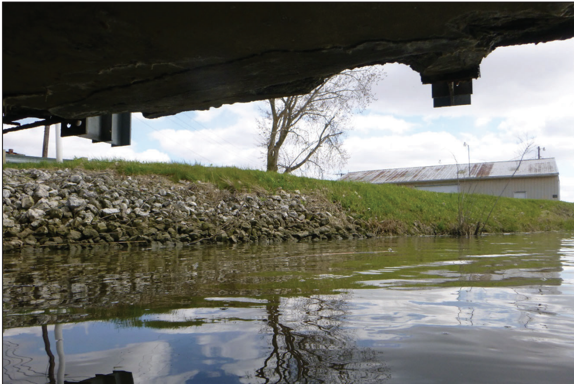
Photograph No. 6: View of the East Embankment Upstream of the Structure, Looking Southeast.
