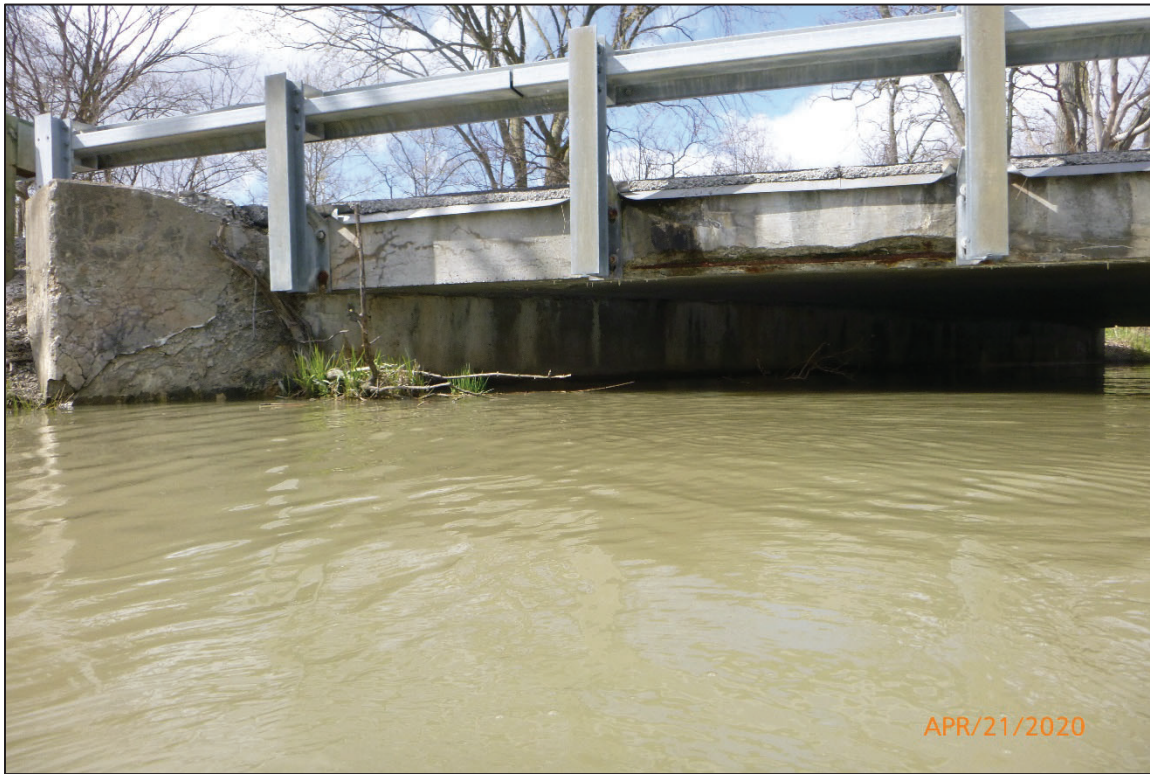
Photograph No. 9: View of the East Face of Abutment 1, Looking Northwest.
