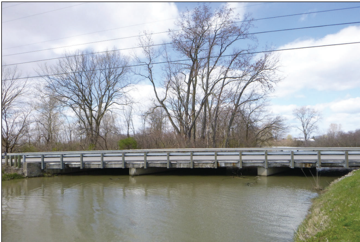
Photograph No. 2: Overall View of Structure No. 4800451 (LUC-2-3175), Looking North.
