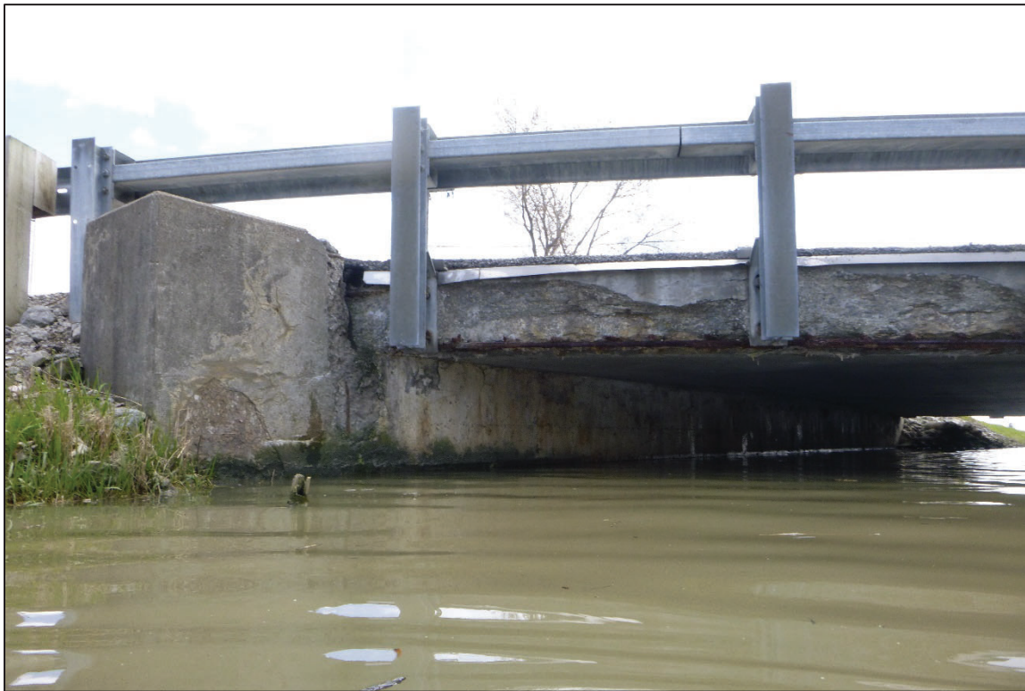
Photograph No. 16: View of the West Face of Abutment 2, Looking Southeast.
