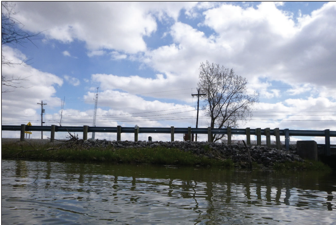
Photograph No. 8: View of the East Embankment Downstream of the Structure, Looking Southeast.
