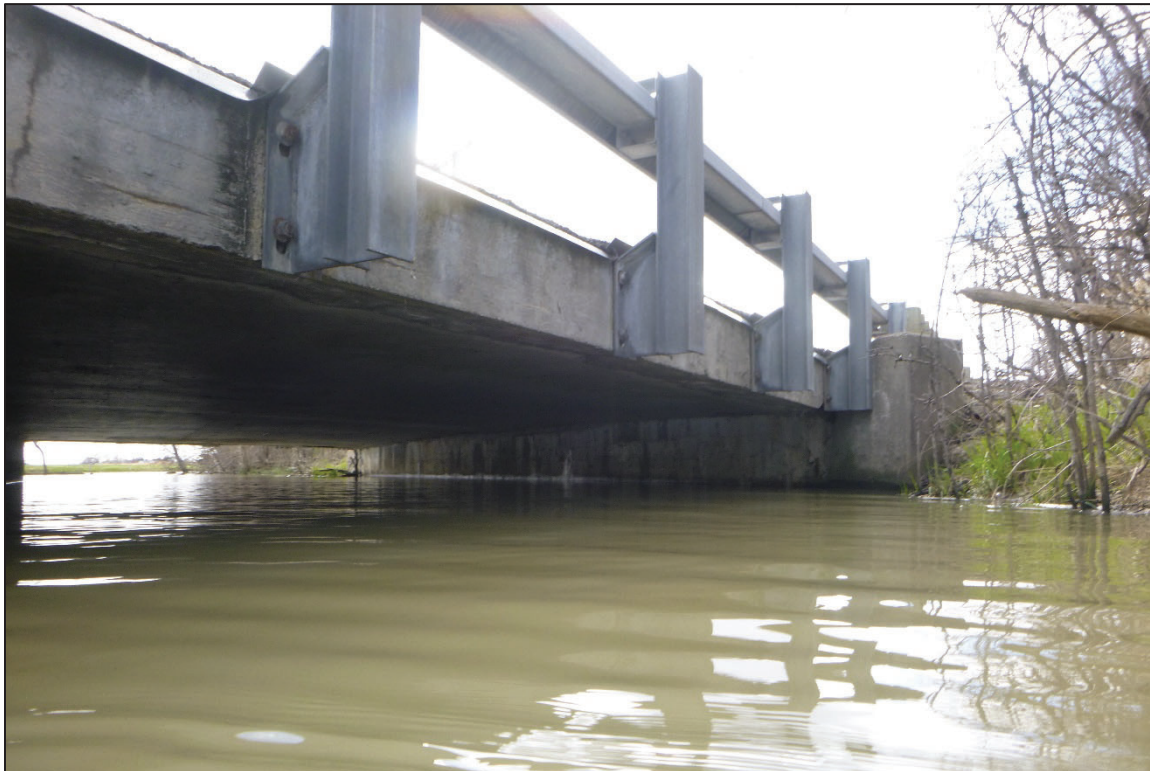
Photograph No. 10: View of the East Face of Abutment 1, Looking Southwest.
