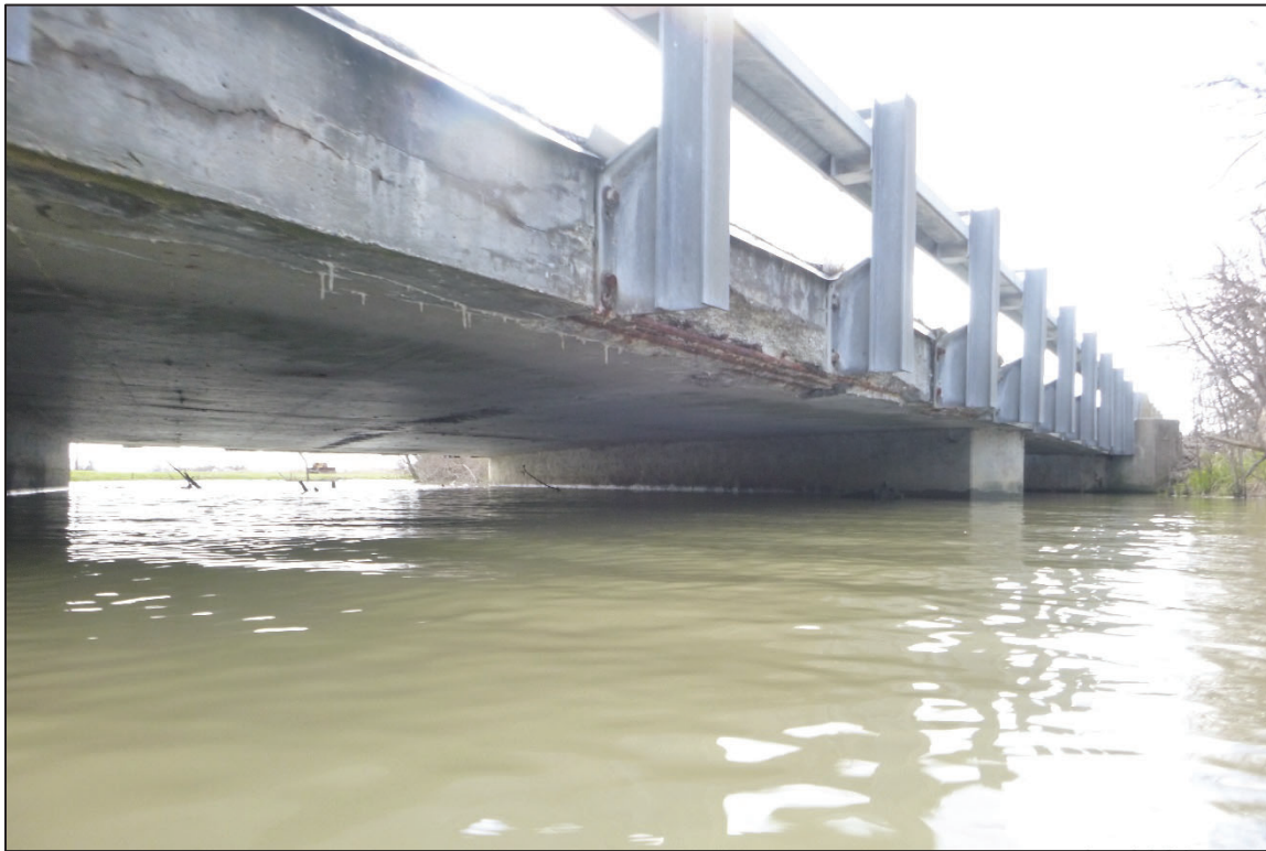
Photograph No. 13: View of the East Face of Bent 1, Looking Southwest.
