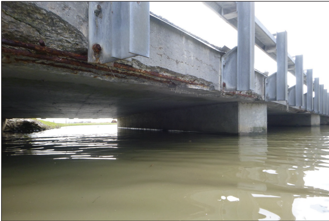
Photograph No. 15: View of the East Face of Bent 2, Looking Southwest.
