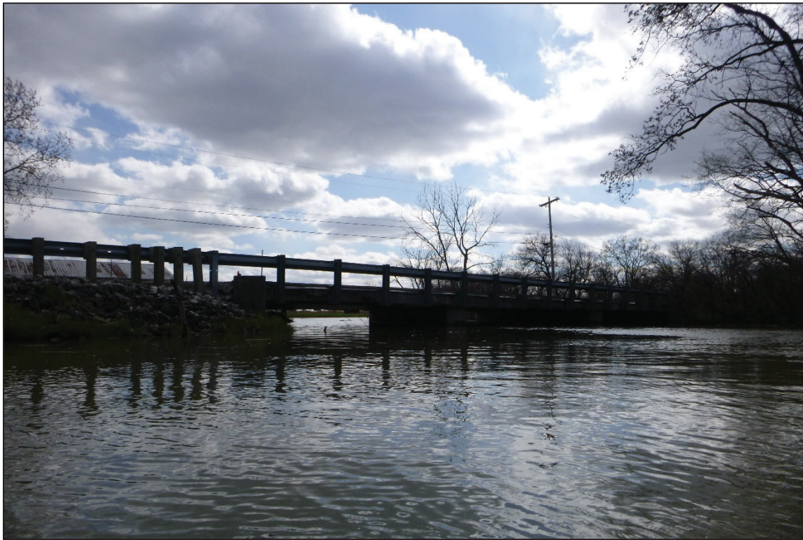
Photograph No. 1: Overall View of Structure No. 4800451 (LUC-2-3175), Looking South.
