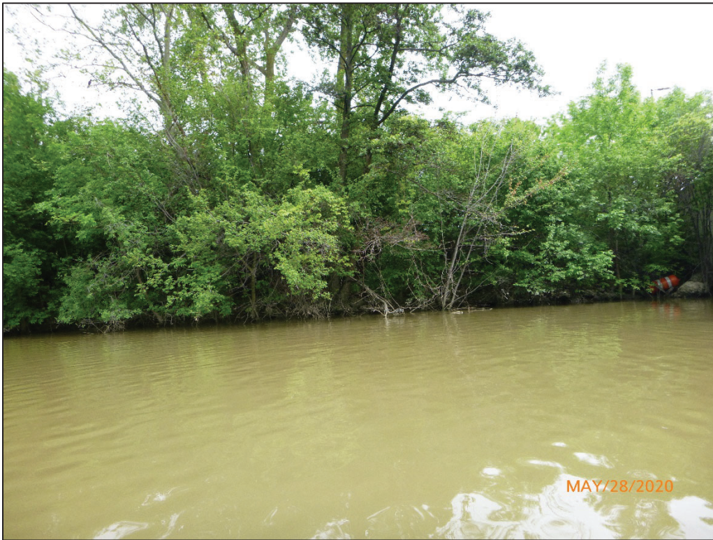
Photograph No. 3: View of the North Embankment Upstream of the Structure, Looking North.
