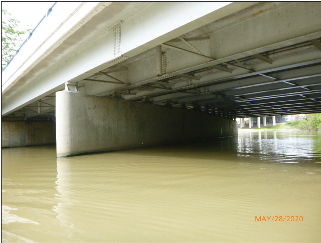
Photograph No. 9: View of the North Face of Pier 1, Looking Southwest.
