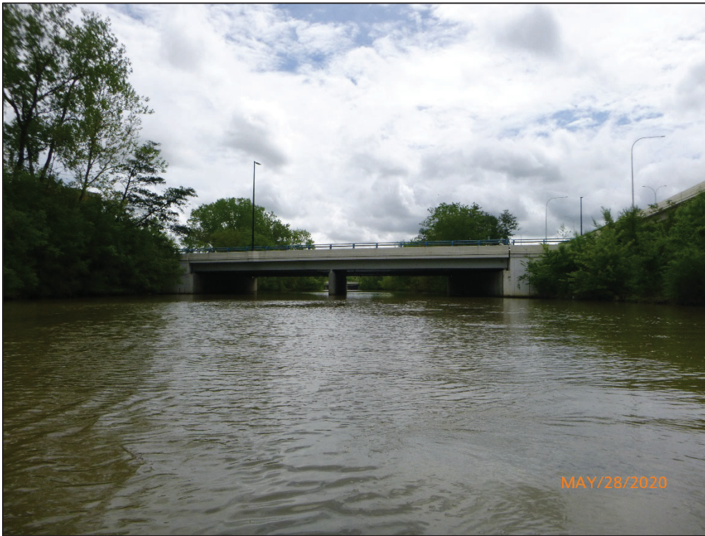
Photograph No. 1: Overall View of Structure No. 4801741 (LUC-24-2656), Looking East.
