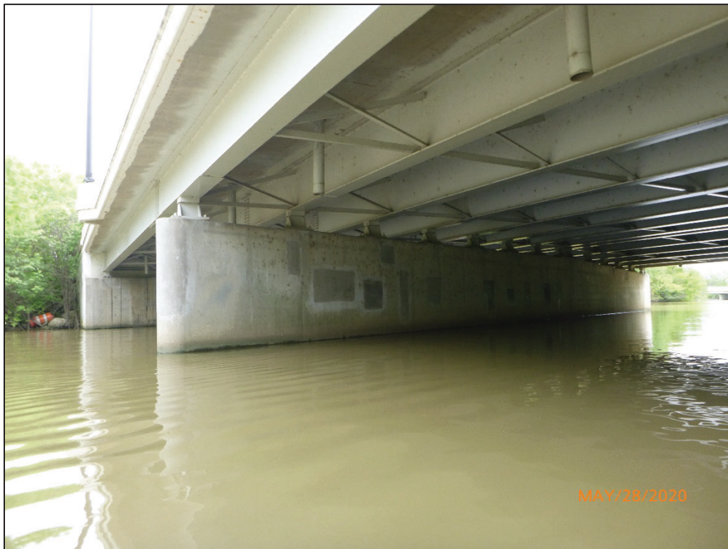
Photograph No. 10: View of the South Face of Pier 1, Looking Northeast.
