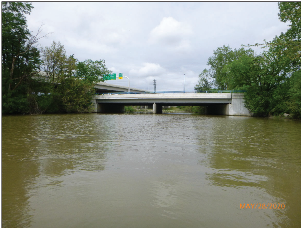
Photograph No. 2: Overall View of Structure No. 4801741 (LUC-24-2656), Looking West.
