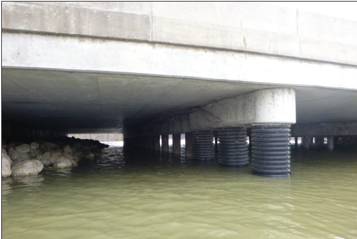
Photograph No. 14: View of the South Face of Bent 1, Looking Northwest.
