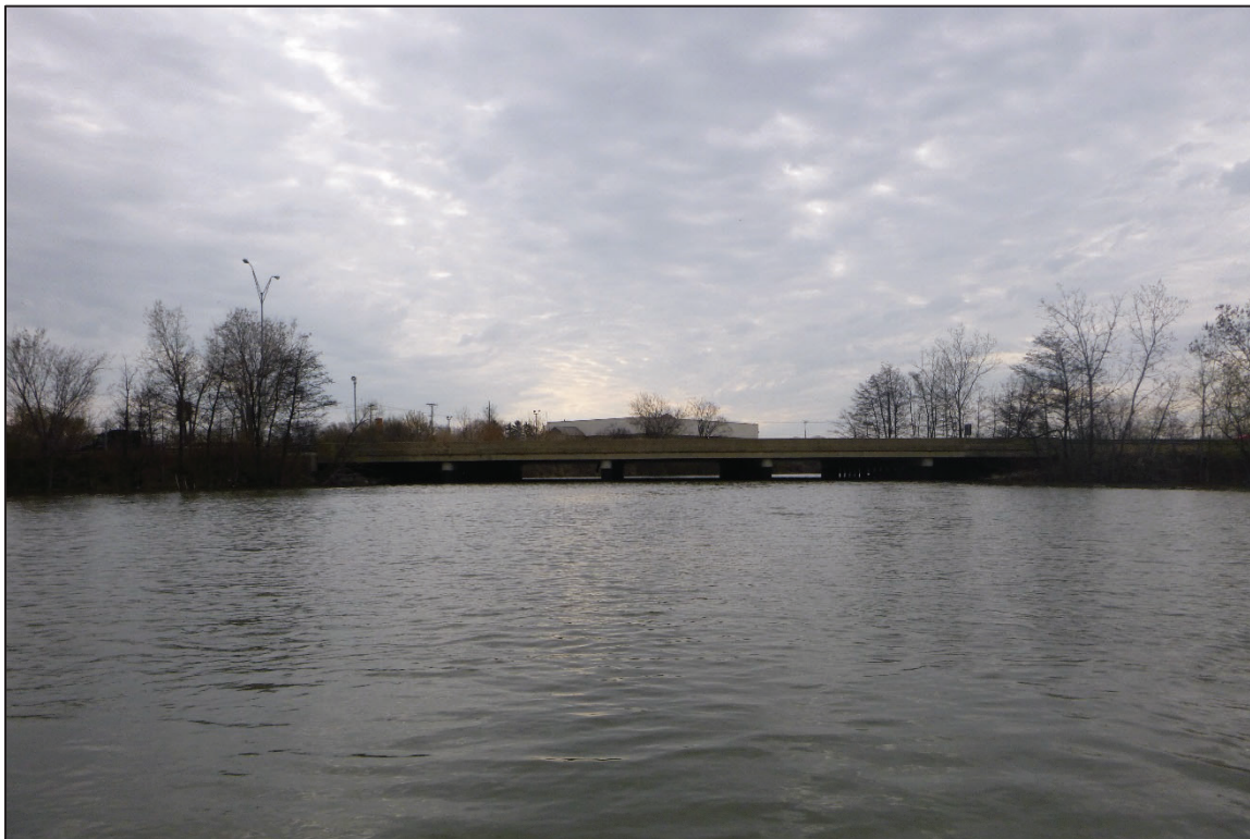
Photograph No. 2: Overall View of Structure No. 4804686 (LUC-75-1013), Looking East.
