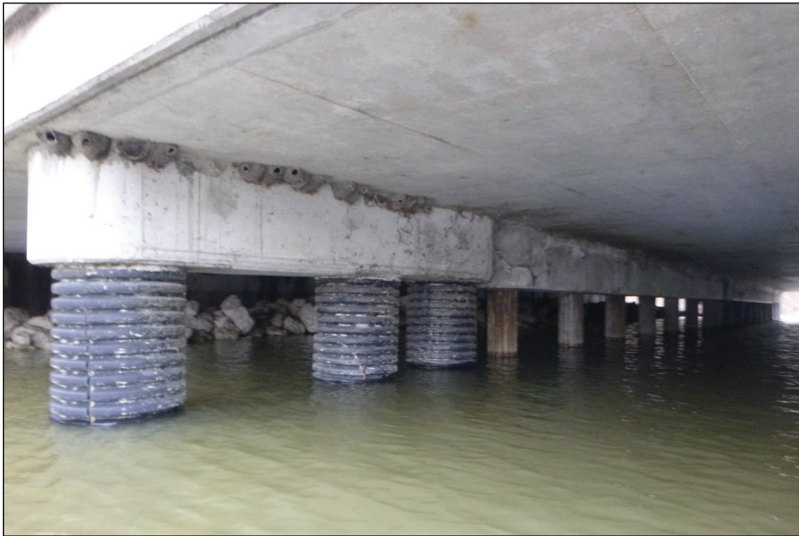
Photograph No. 25: View of the South Face of Bent 4, Looking Northeast.
