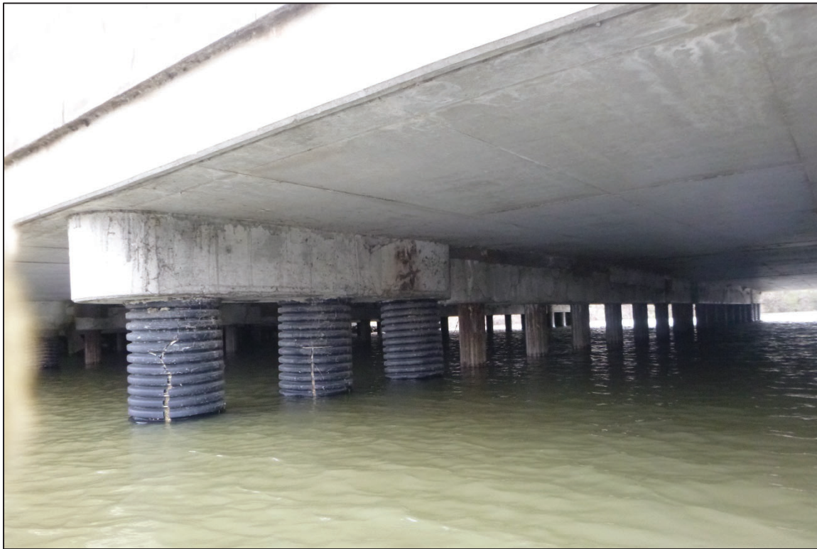
Photograph No. 17: View of the South Face of Bent 2, Looking Northeast.
