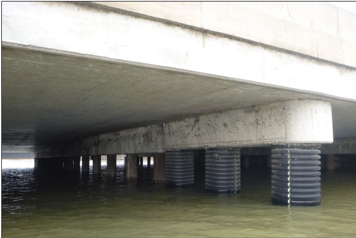
Photograph No. 22: View of the South Face of Bent 3, Looking Northwest.
