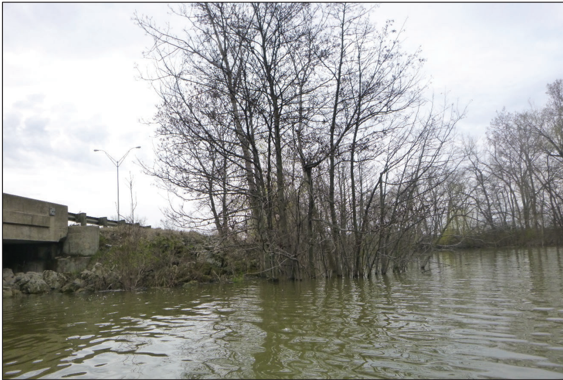
Photograph No. 7: View of the South Embankment Upstream of the Structure, Looking Southeast.
