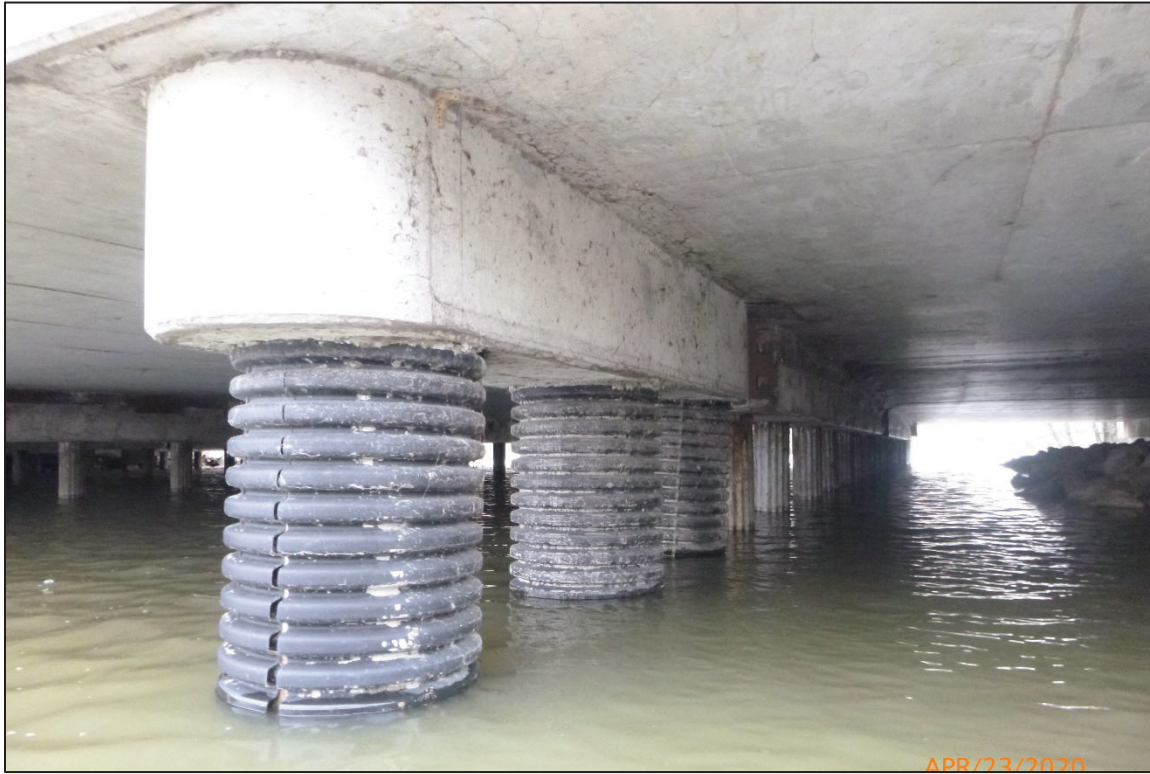
Photograph No. 13: View of the South Face of Bent 1, Looking Northeast.
