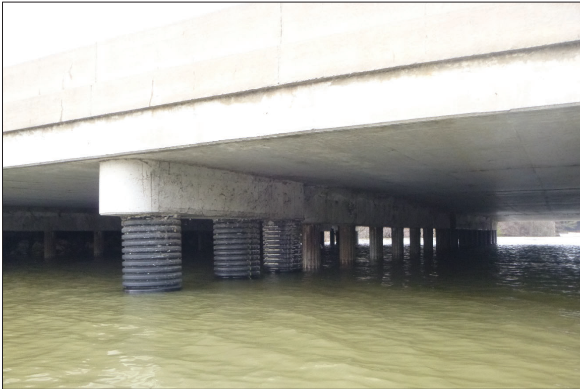
Photograph No. 16: View of the North Face of Bent 2, Looking Southwest.
