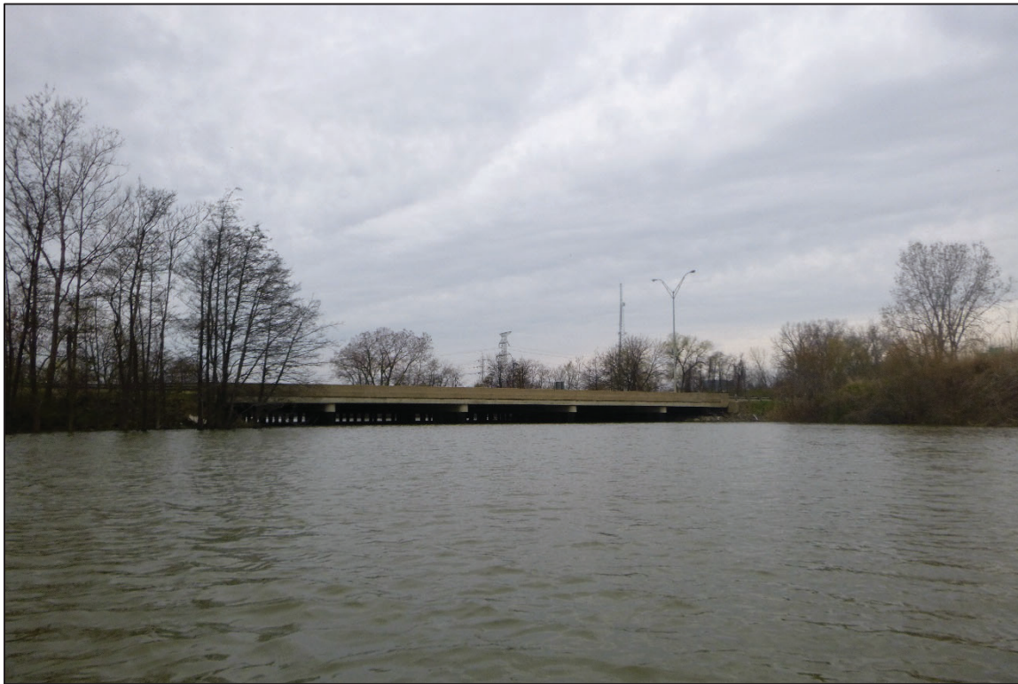
Photograph No. 1: Overall View of Structure No. 4804686 (LUC-75-1013), Looking West.
