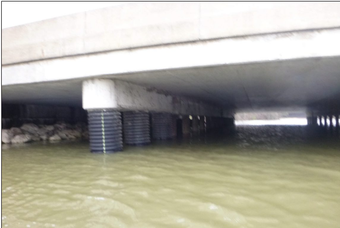
Photograph No. 12: View of the North Face of Bent 1, Looking Southwest.
