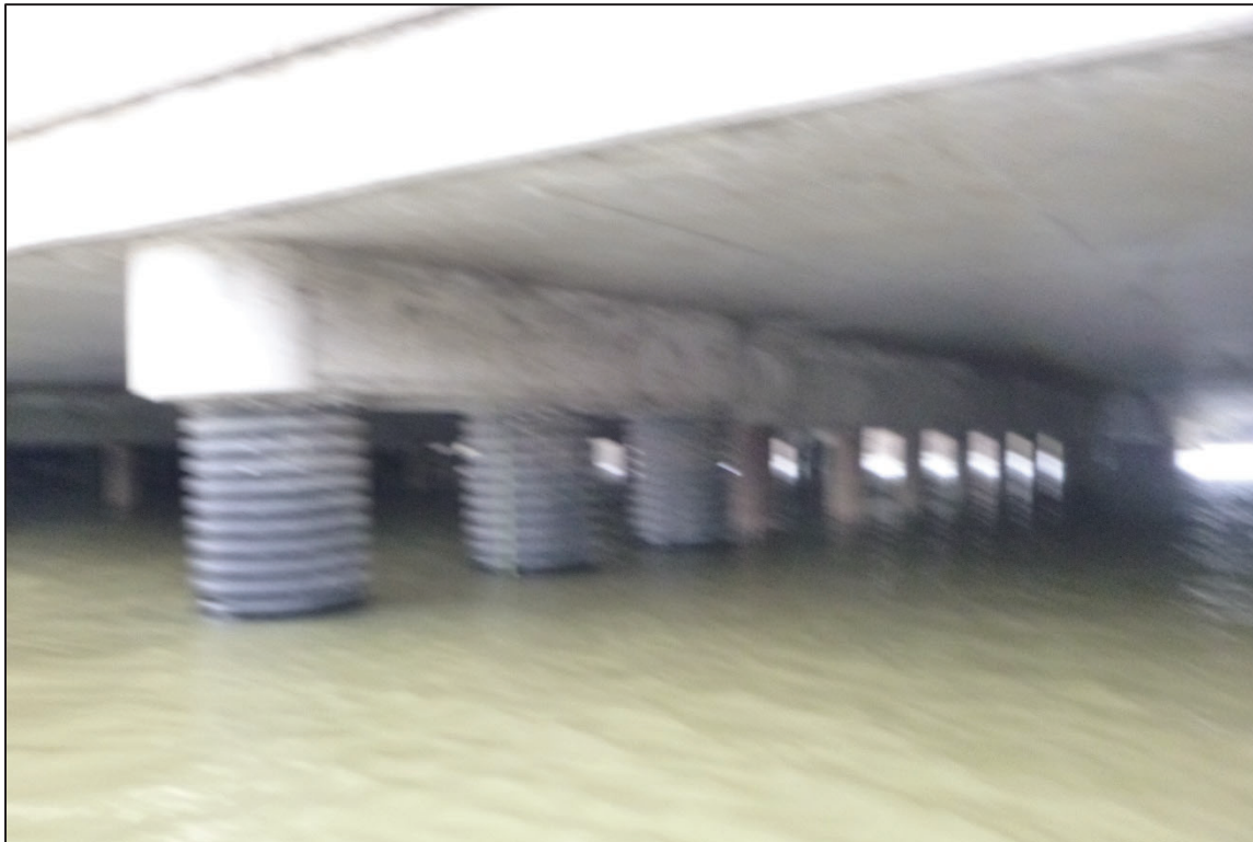
Photograph No. 20: View of the North Face of Bent 3, Looking Southwest.
