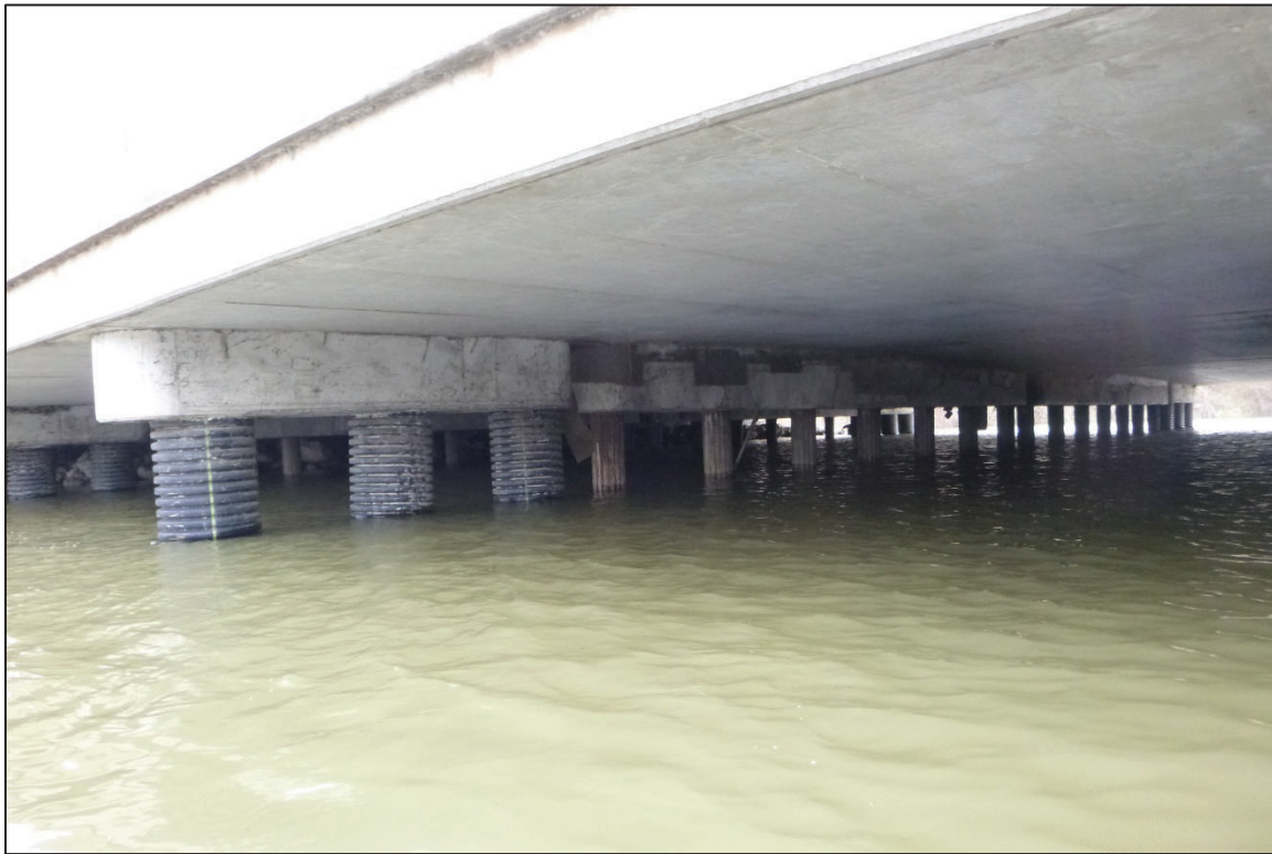
Photograph No. 21: View of the South Face of Bent 3, Looking Northeast.
