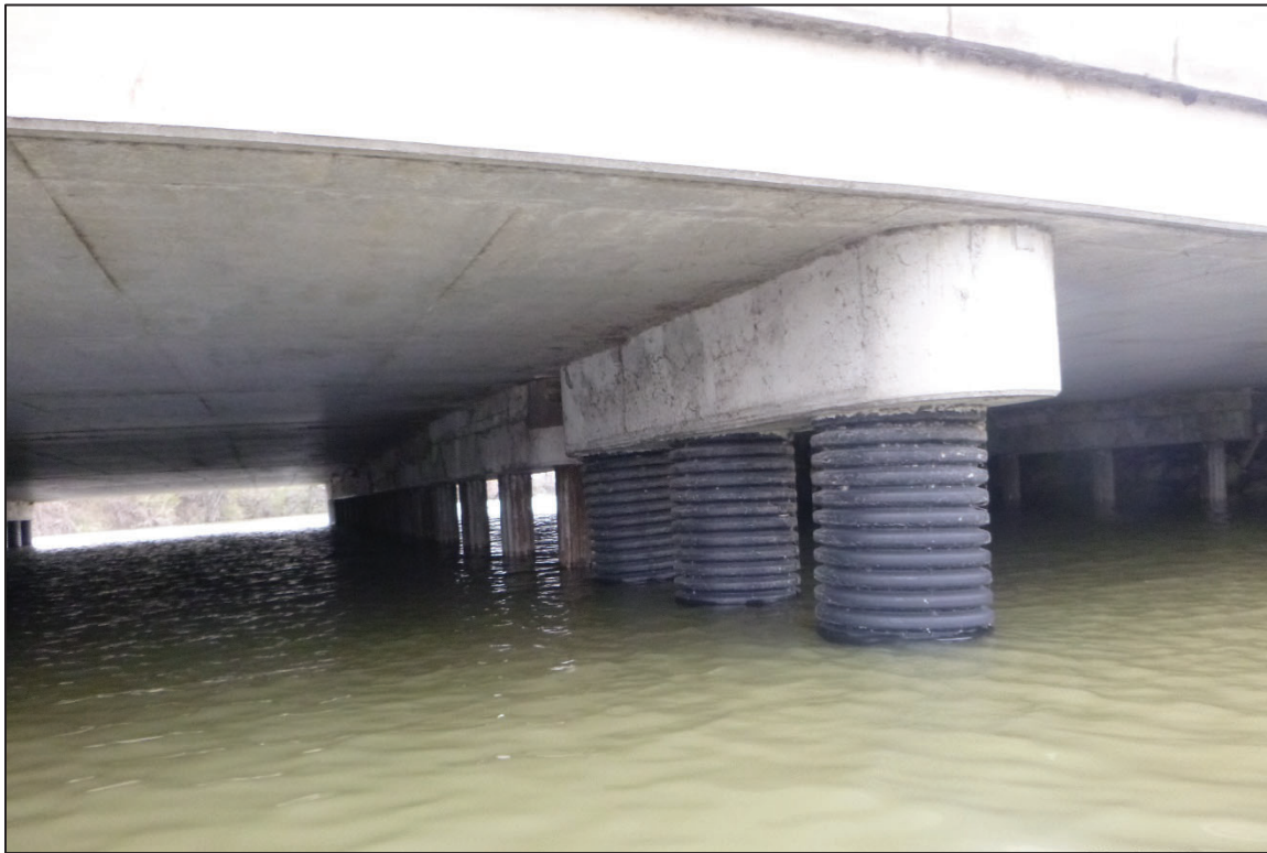
Photograph No. 15: View of the North Face of Bent 2, Looking Southeast.
