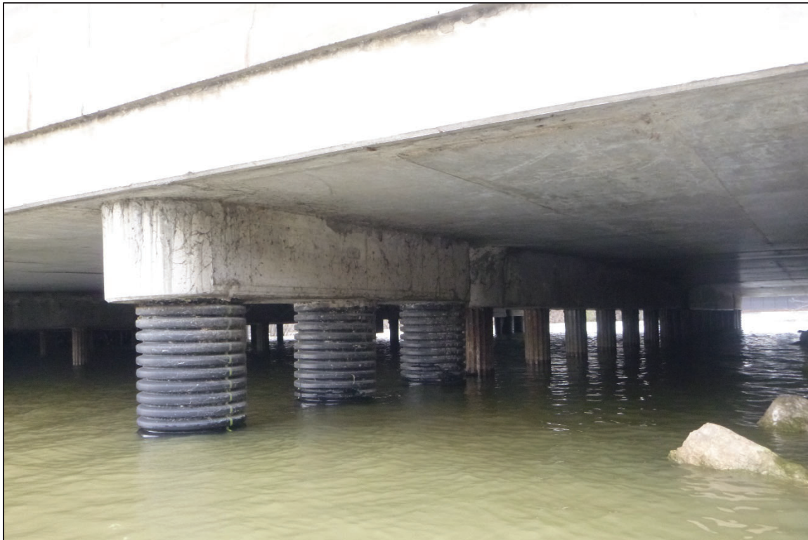
Photograph No. 24: View of the North Face of Bent 4, Looking Southwest.
