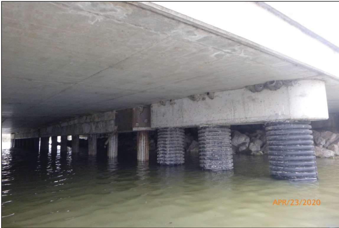
Photograph No. 11: View of the North Face of Bent 1, Looking Southeast.
