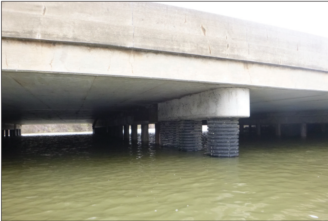
Photograph No. 19: View of the North Face of Bent 3, Looking Southeast.
