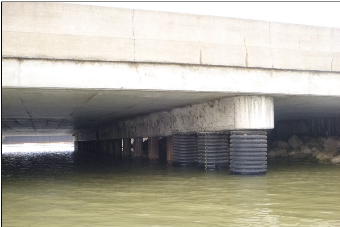
Photograph No. 26: View of the South Face of Bent 4, Looking Northwest.
