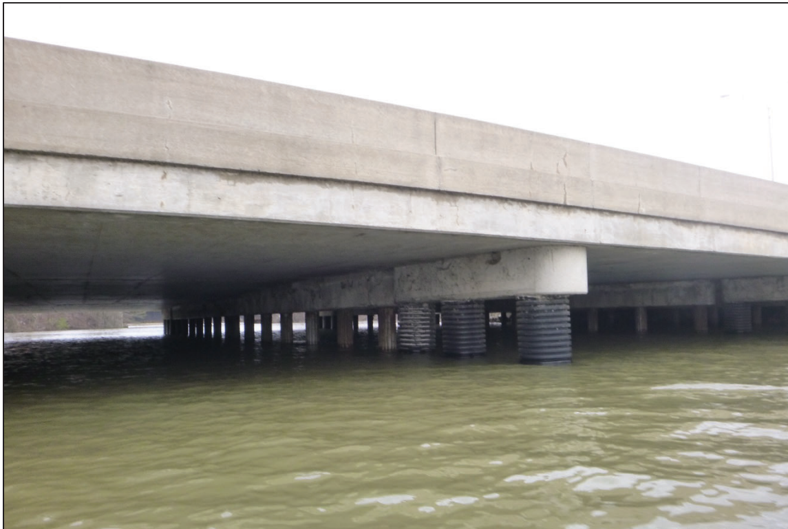
Photograph No. 18: View of the South Face of Bent 2, Looking Northwest.
