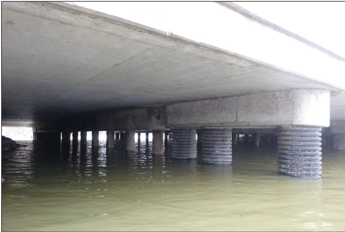
Photograph No. 23: View of the North Face of Bent 4, Looking Southeast.
