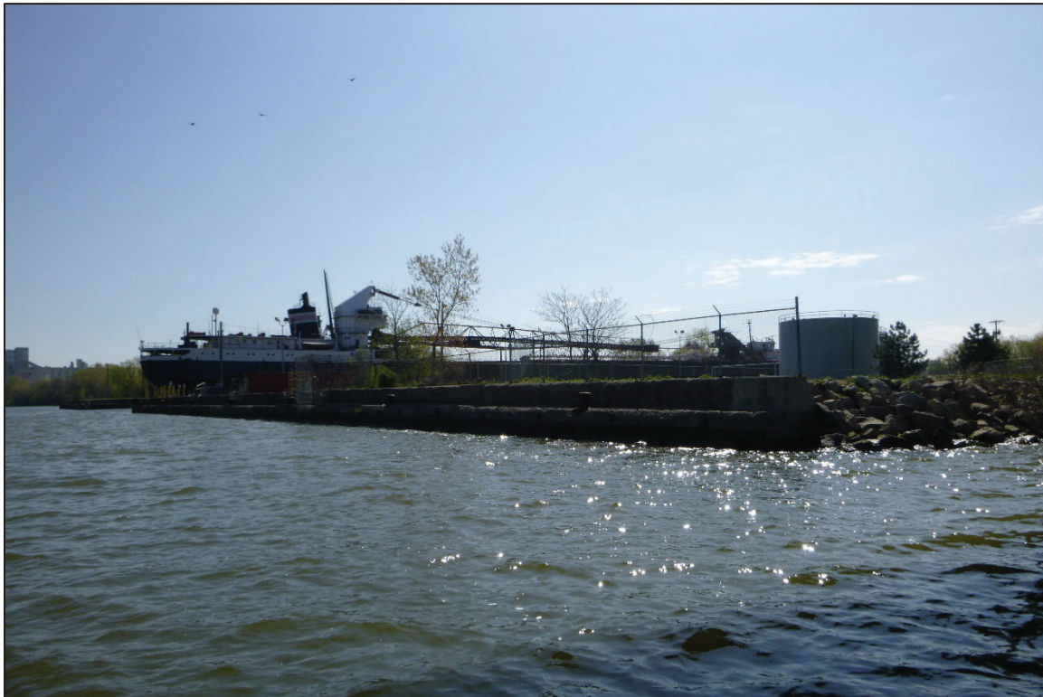
Photograph No. 8: View of the Southeast Embankment Downstream of the Structure, Looking East.
