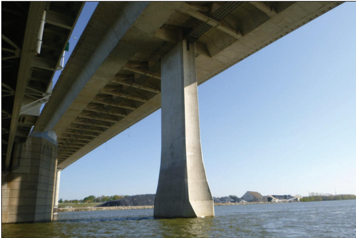
Photograph No. 10: View of the South Face of Pier 28, Looking North.
