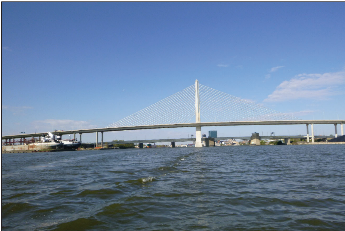
Photograph No. 2: Overall View of Structure No. 4805909 (LUC-280-0346), Looking Southwest.
