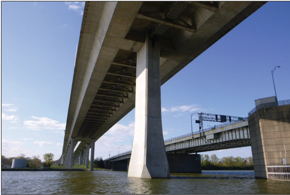
Photograph No. 9: View of the North Face of Pier 28, Looking Southeast.
