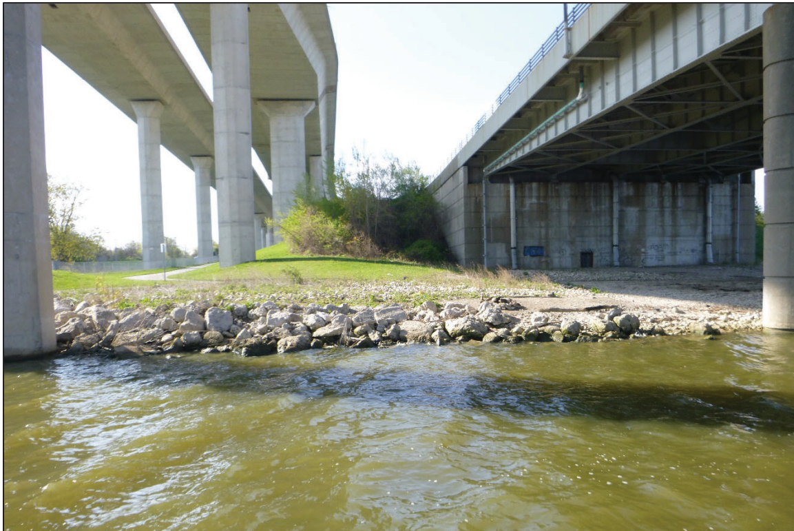
Photograph No. 6: View of the Southeast Embankment Upstream of the Structure, Looking Southeast.
