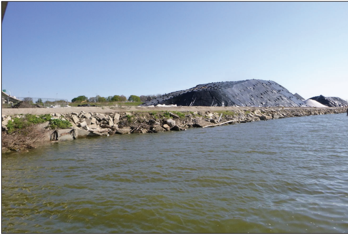
Photograph No. 5: View of the Northwest Embankment Downstream of the Structure, Looking North.
