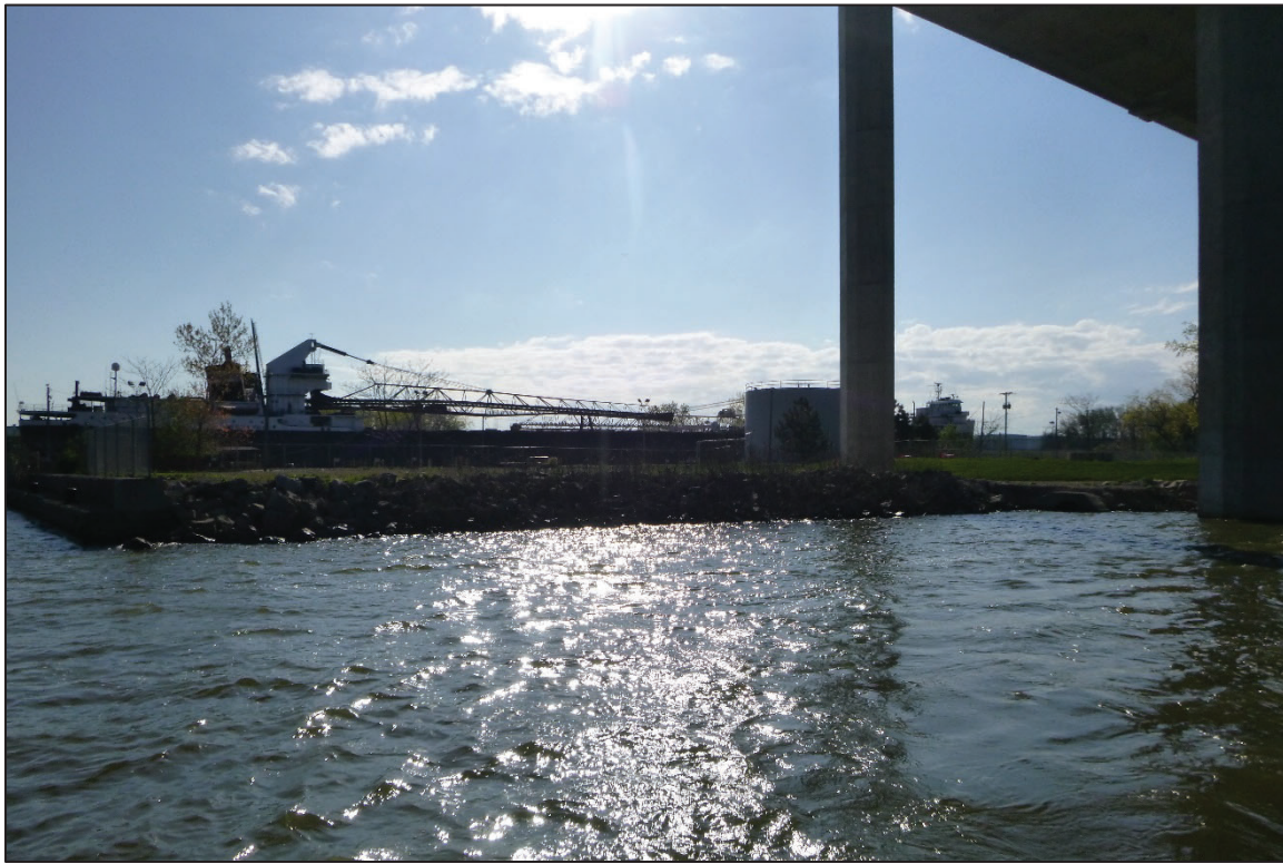
Photograph No. 7: View of the Southeast Embankment at the Structure, Looking East.
