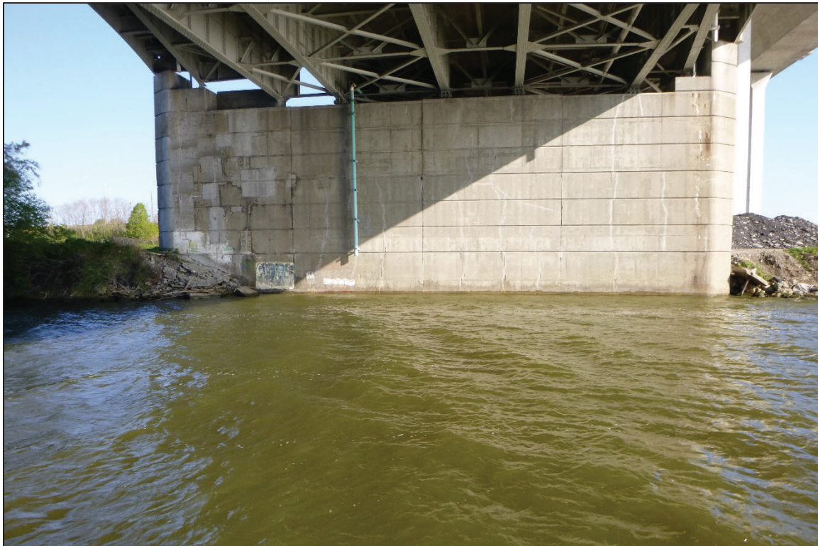
Photograph No. 4: View of the Northwest Embankment at the Structure, Looking Northwest.
