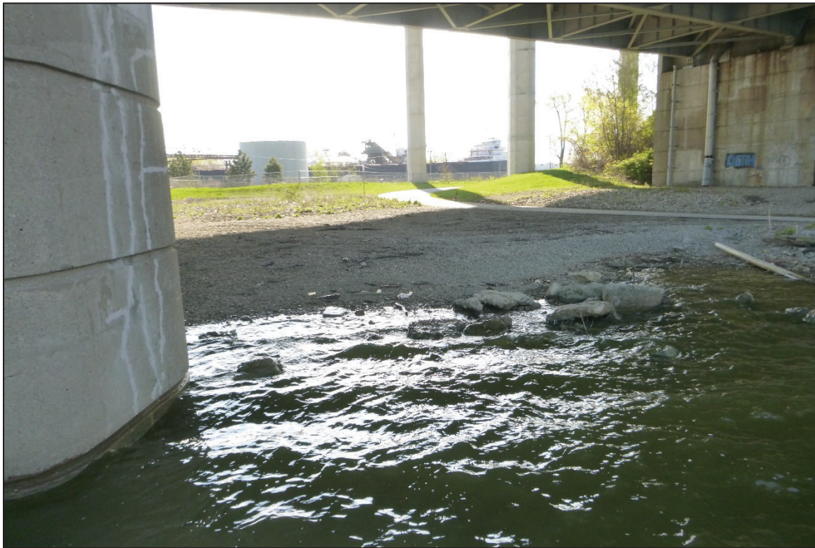
Photograph No. 7: View of the Southeast Embankment at the Structure, Looking East.
