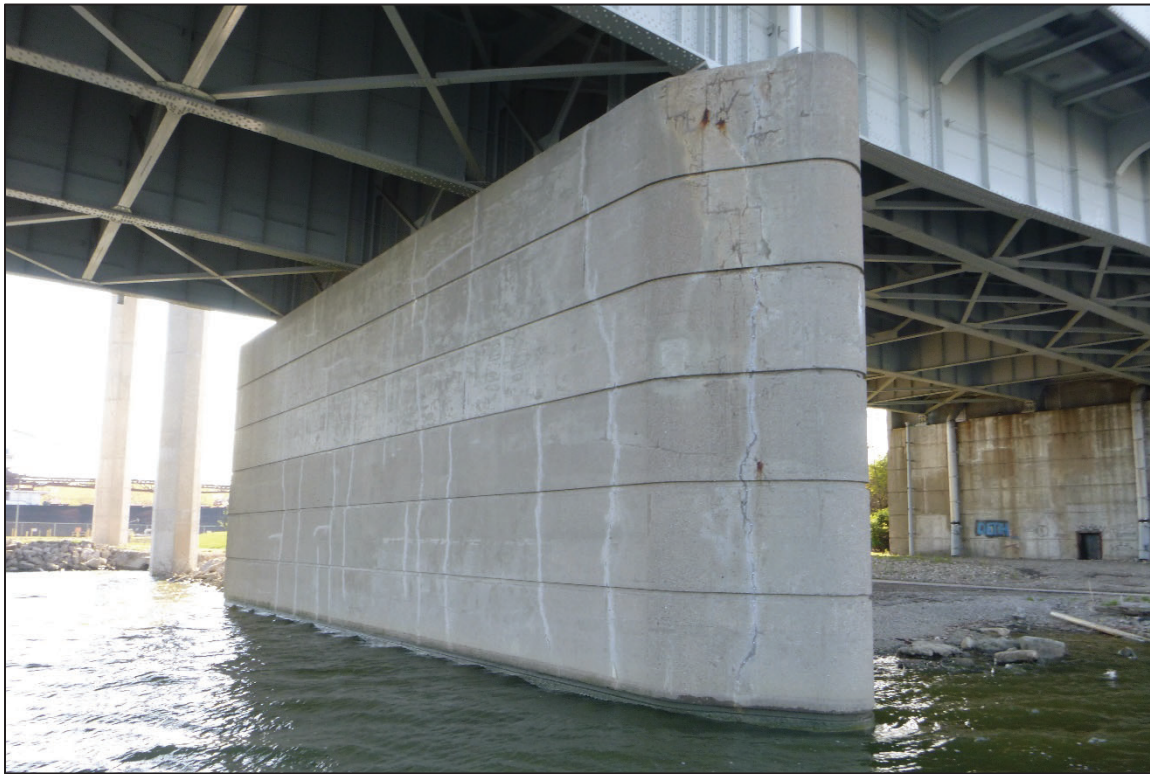
Photograph No. 9: View of the North Face of Pier 1, Looking East.
