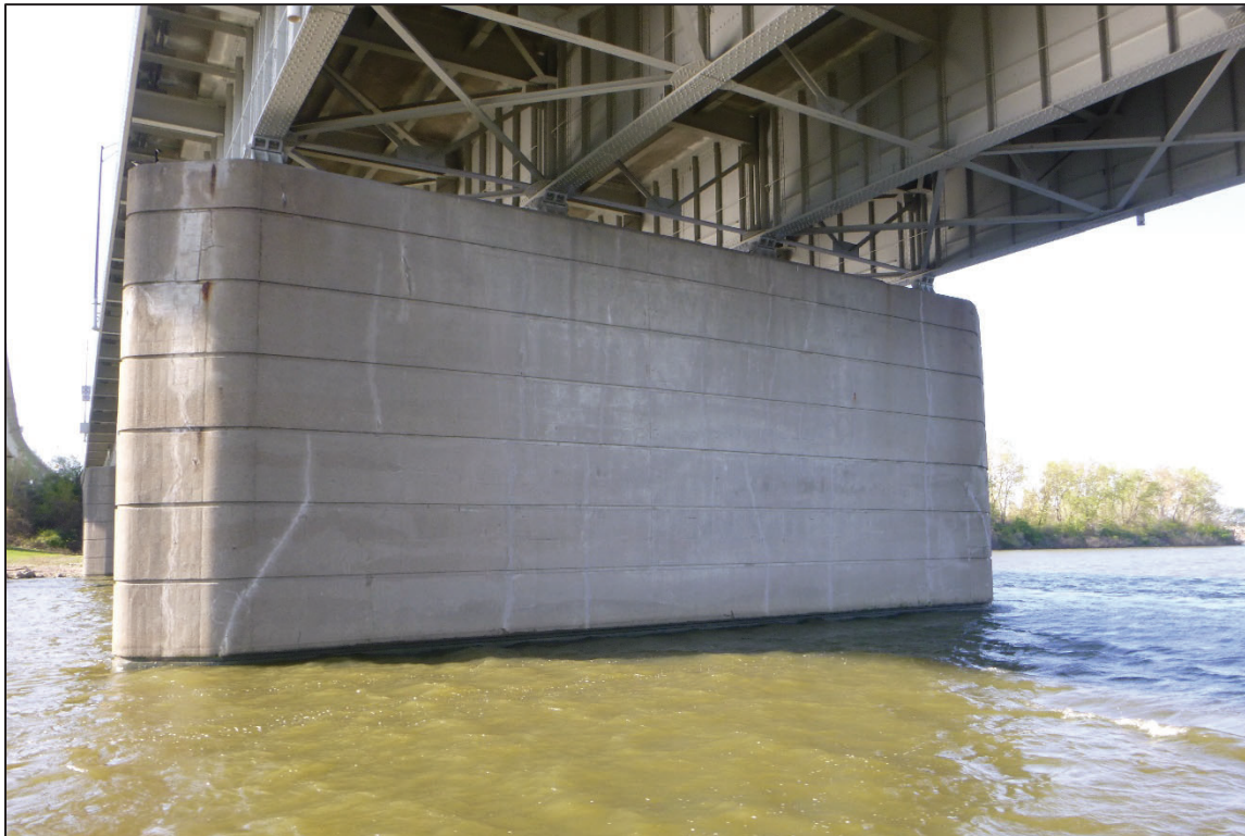
Photograph No. 10: View of the North Face of Pier 2, Looking Southeast.
