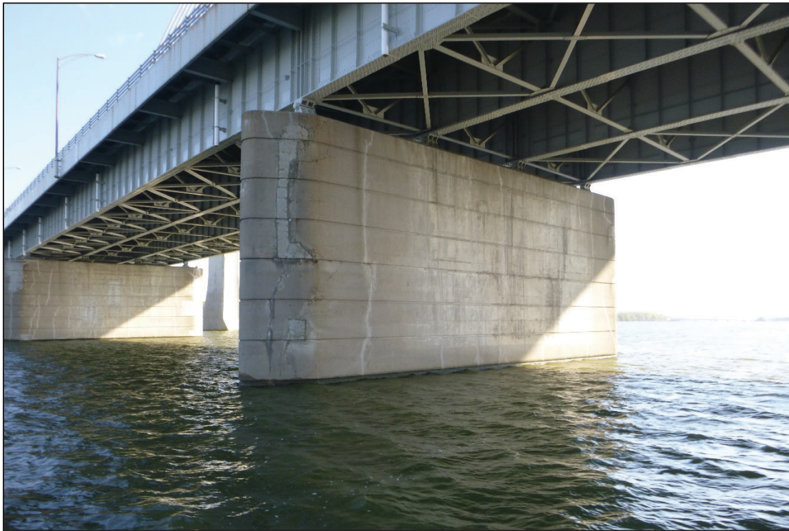
Photograph No. 11: View of the South Face of Pier 2, Looking North.
