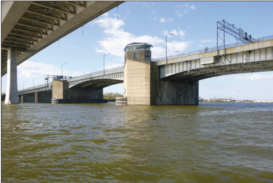
Photograph No. 2: Overall View of Structure No. 4805917 (LUC-65-0535), Looking South.
