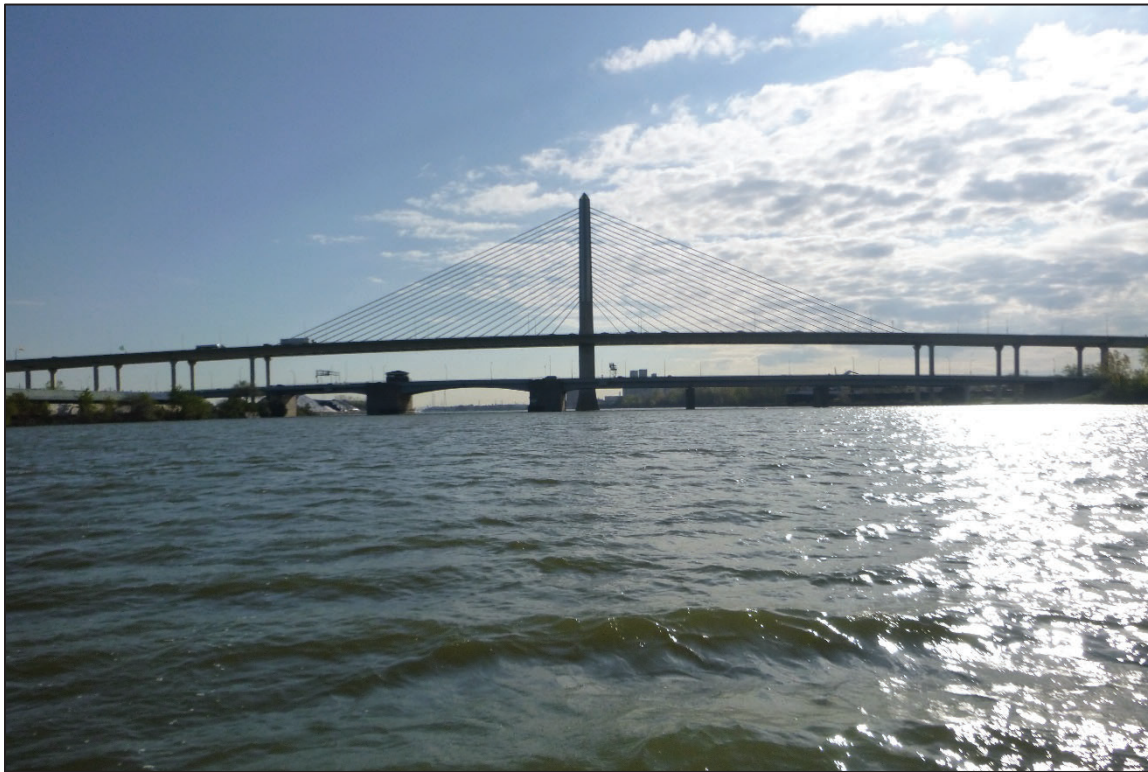
Photograph No. 1: Overall View of Structure No. 4805917 (LUC-65-0535), Looking Northeast.
