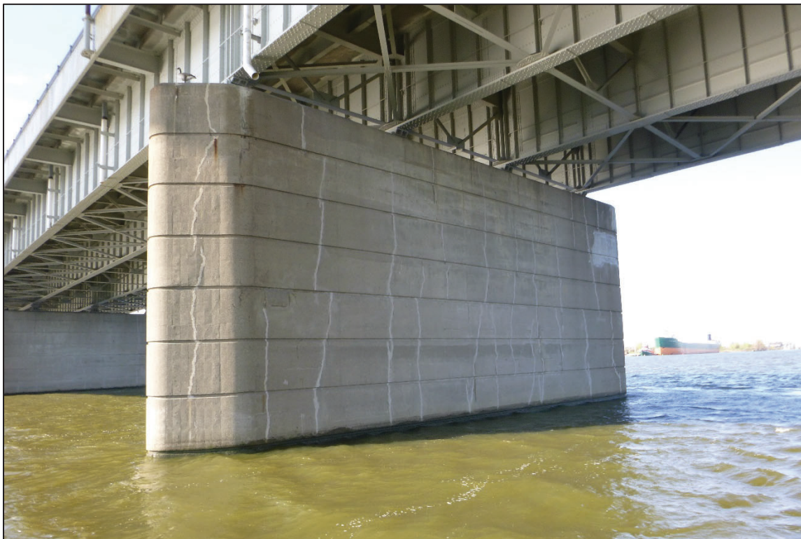
Photograph No. 12: View of the North Face of Pier 3, Looking South.
