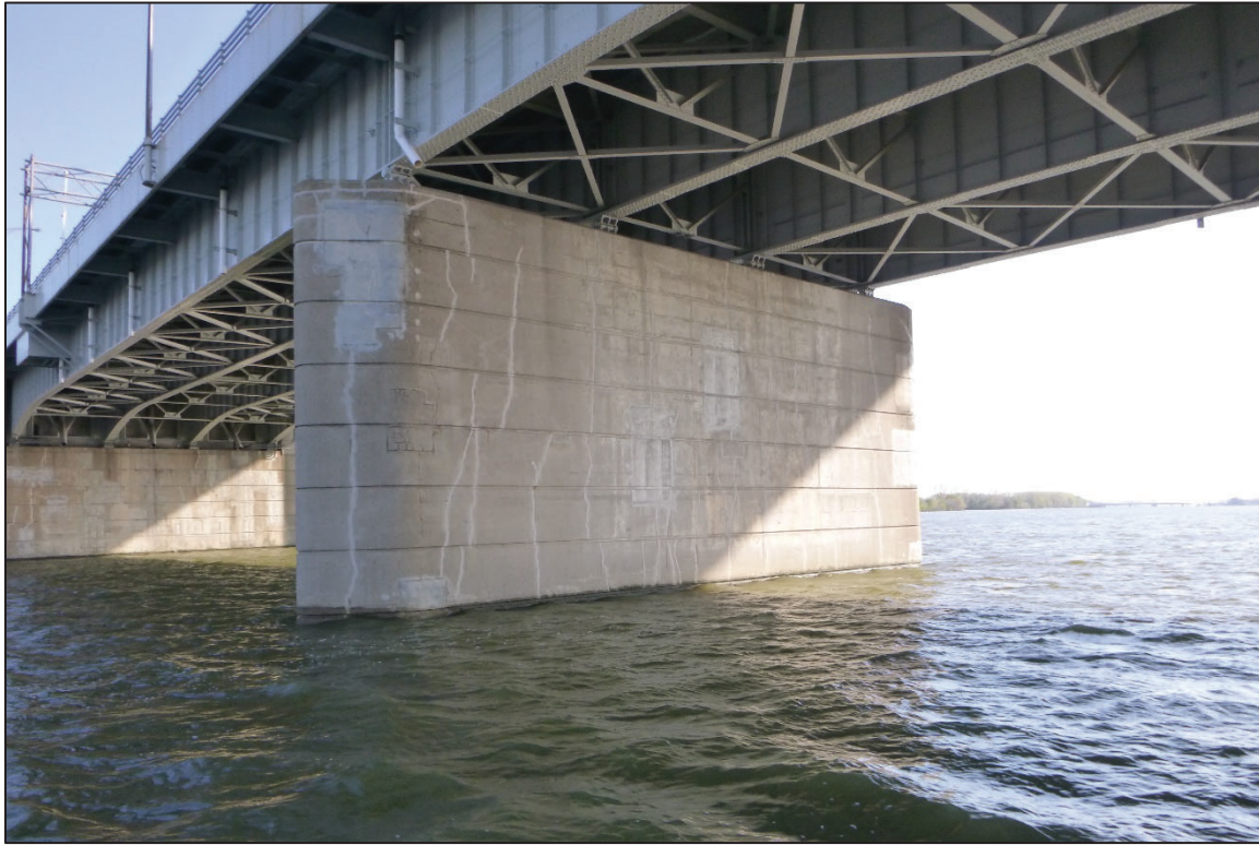
Photograph No. 13: View of the South Face of Pier 3, Looking North.
