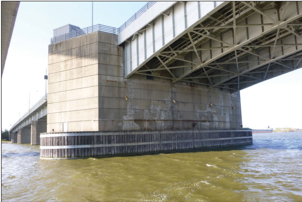
Photograph No. 14: View of the North Face of Pier 4, Looking South.
