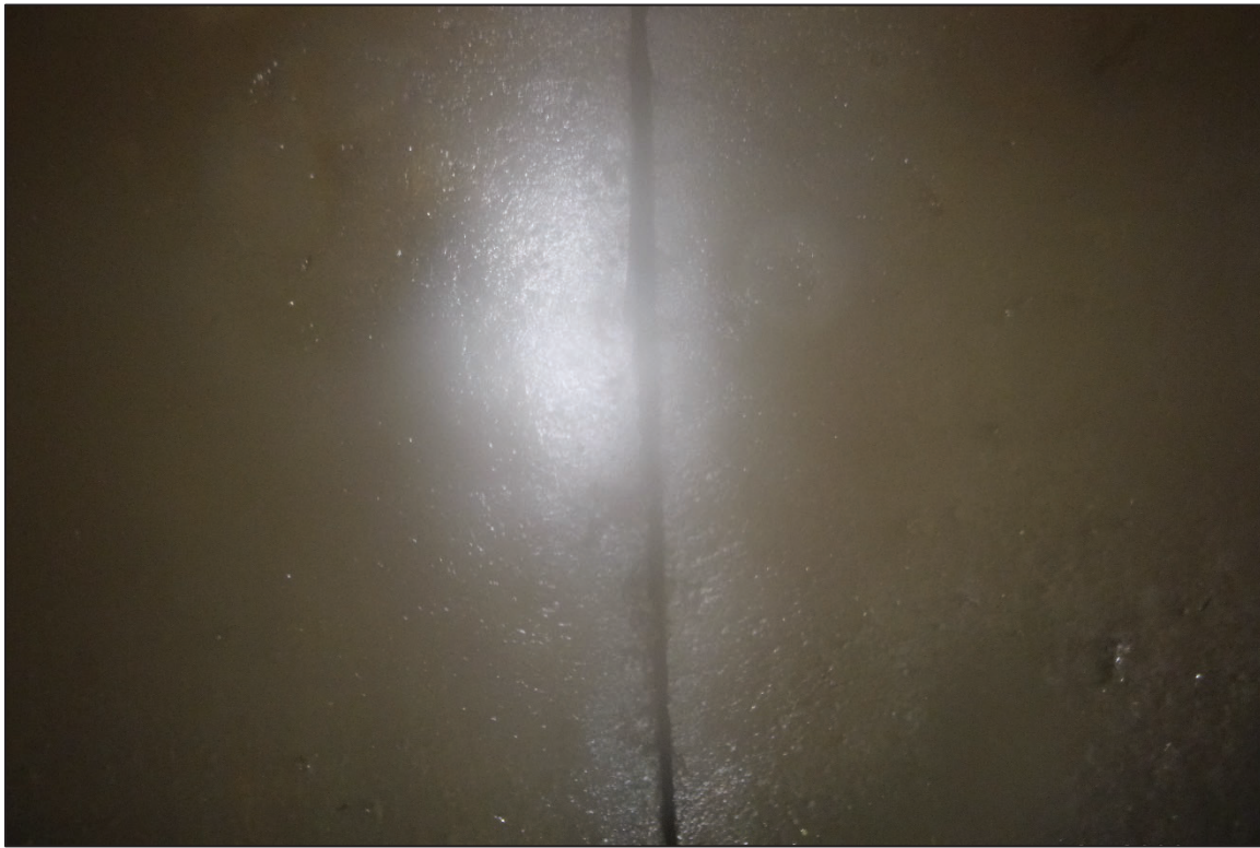
Photograph No. 3: View of the Typical Joint Condition, Looking South.
