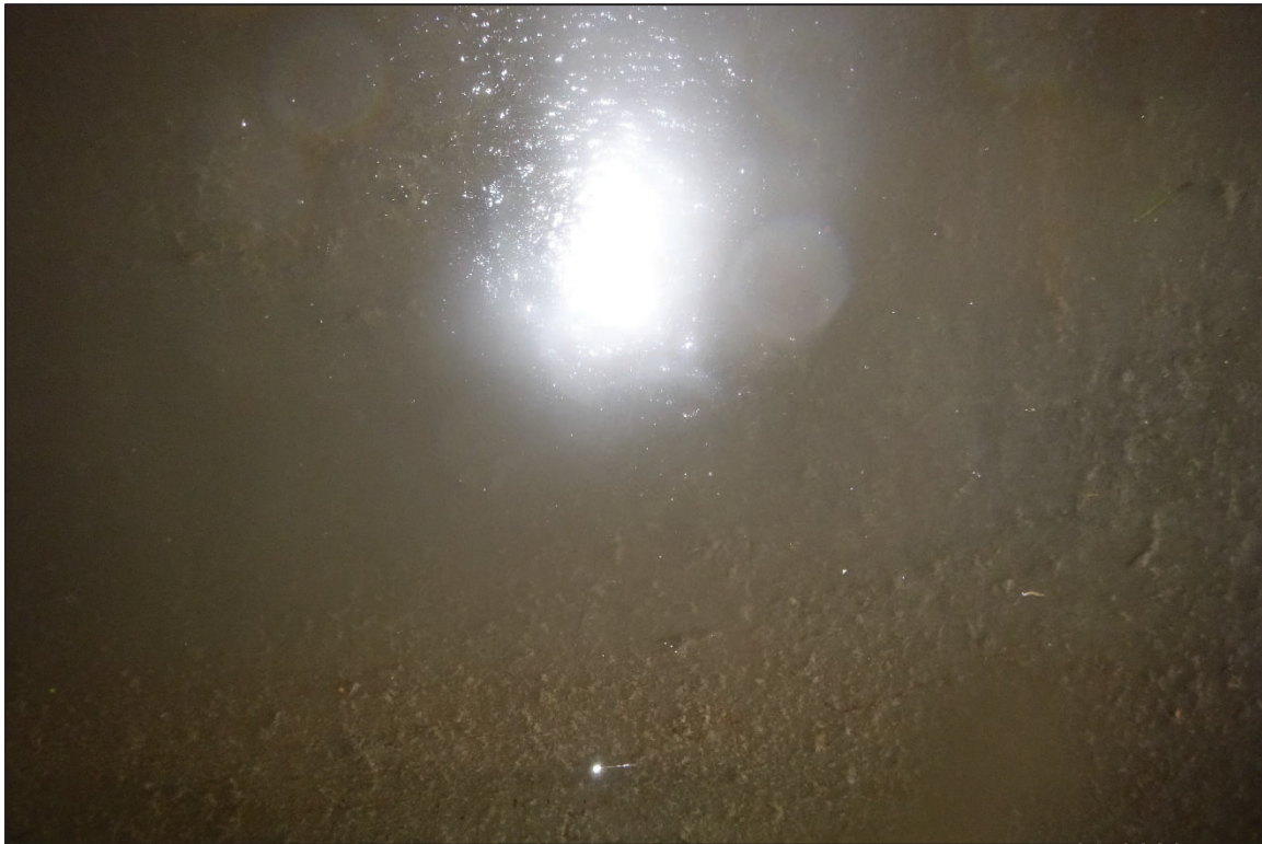
Photograph No. 4: View of the Typical Concrete Condition, Looking South.
