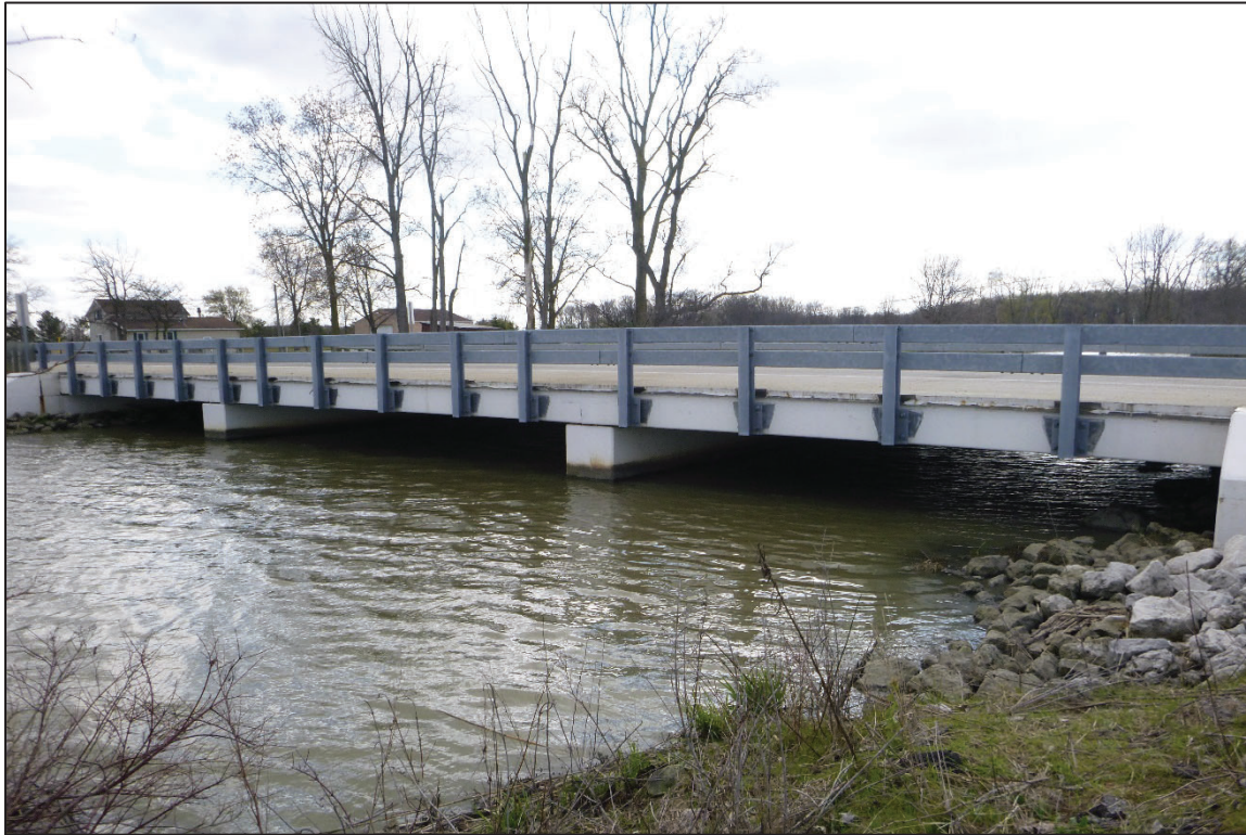
Photograph No. 1: Overall View of Structure No. 6200044 (OTT-2-0016), Looking Southwest.
