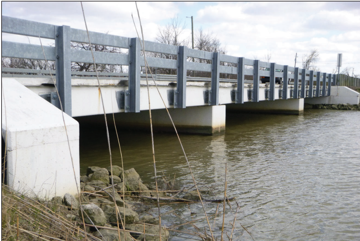
Photograph No. 2: Overall View of Structure No. 6200044 (OTT-2-0016), Looking Southeast.
