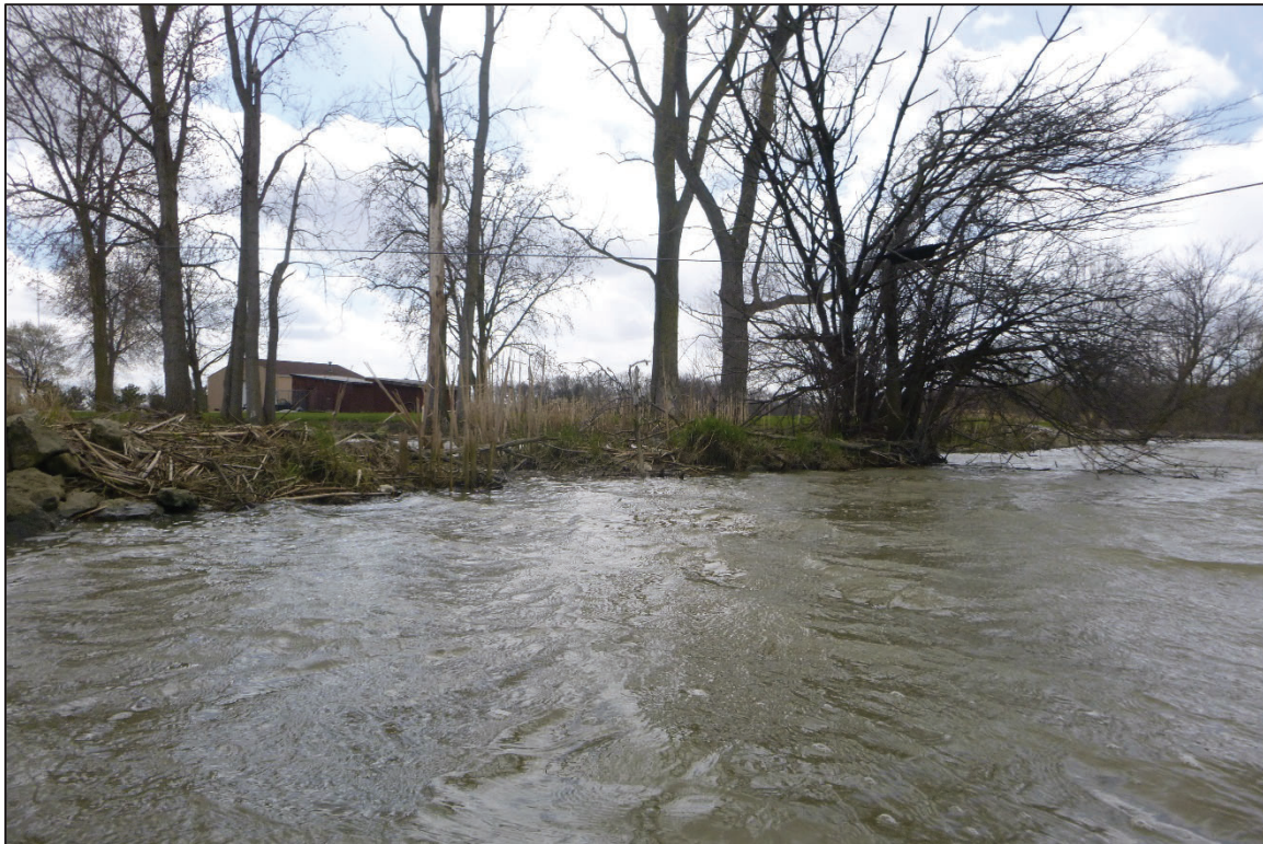
Photograph No. 6: View of the South Embankment Upstream of the Structure, Looking Southwest.
