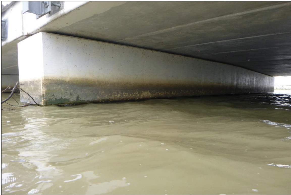
Photograph No. 10: View of the South Face of Bent 1, Looking Northeast.
