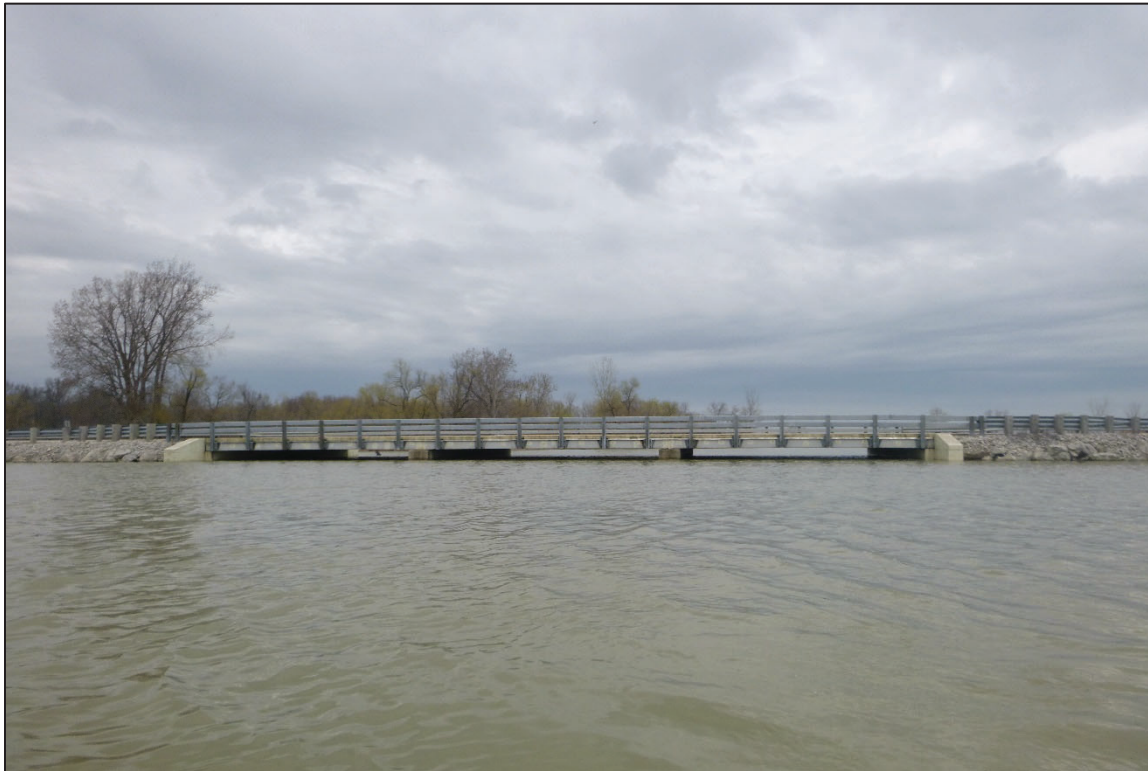
Photograph No. 2: Overall View of Structure No. 6200109 (OTT-2-0667), Looking North.
