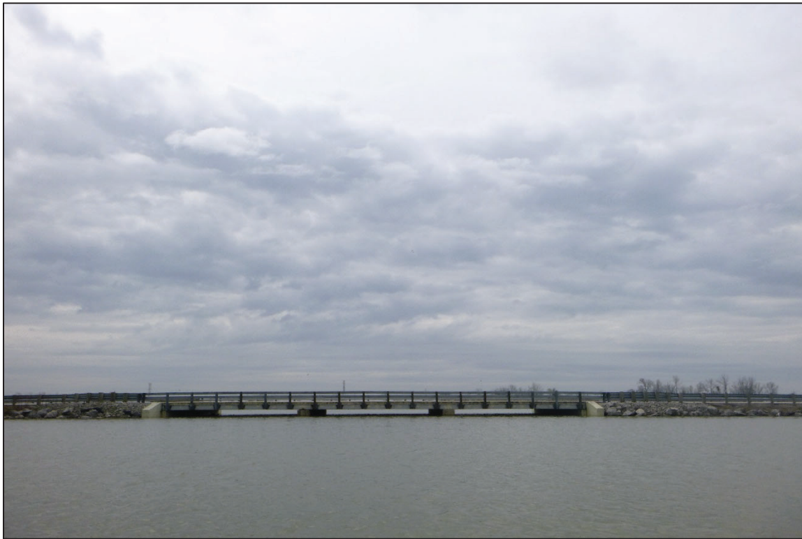
Photograph No. 1: Overall View of Structure No. 6200109 (OTT-2-0667), Looking South.
