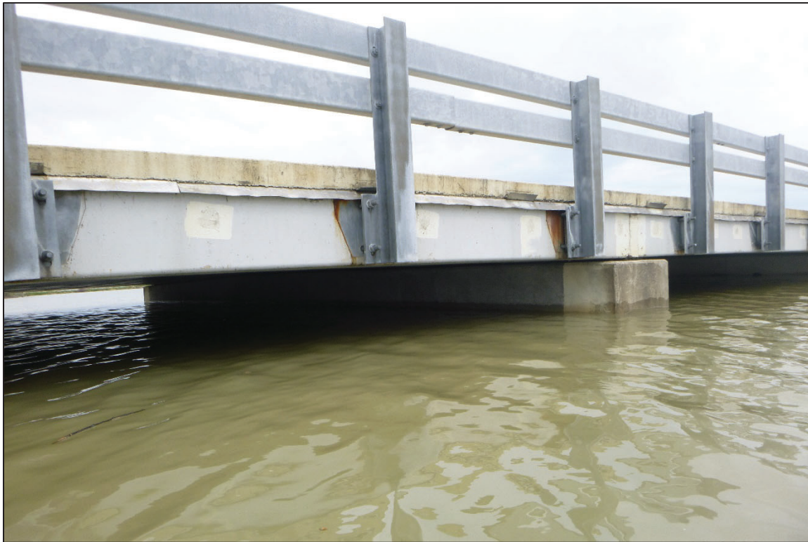
Photograph No. 14: View of the West Face of Bent 2, Looking Northeast.
