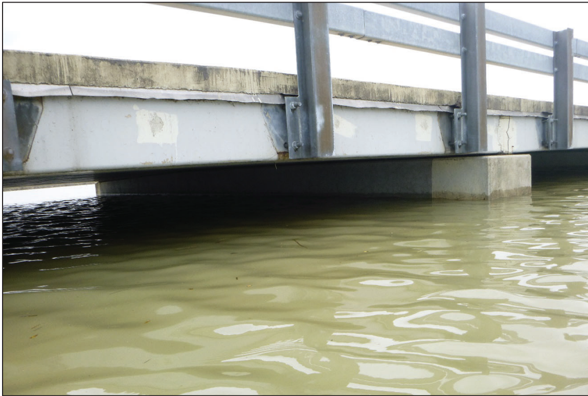
Photograph No. 11: View of the East Face of Bent 1, Looking Southwest.
