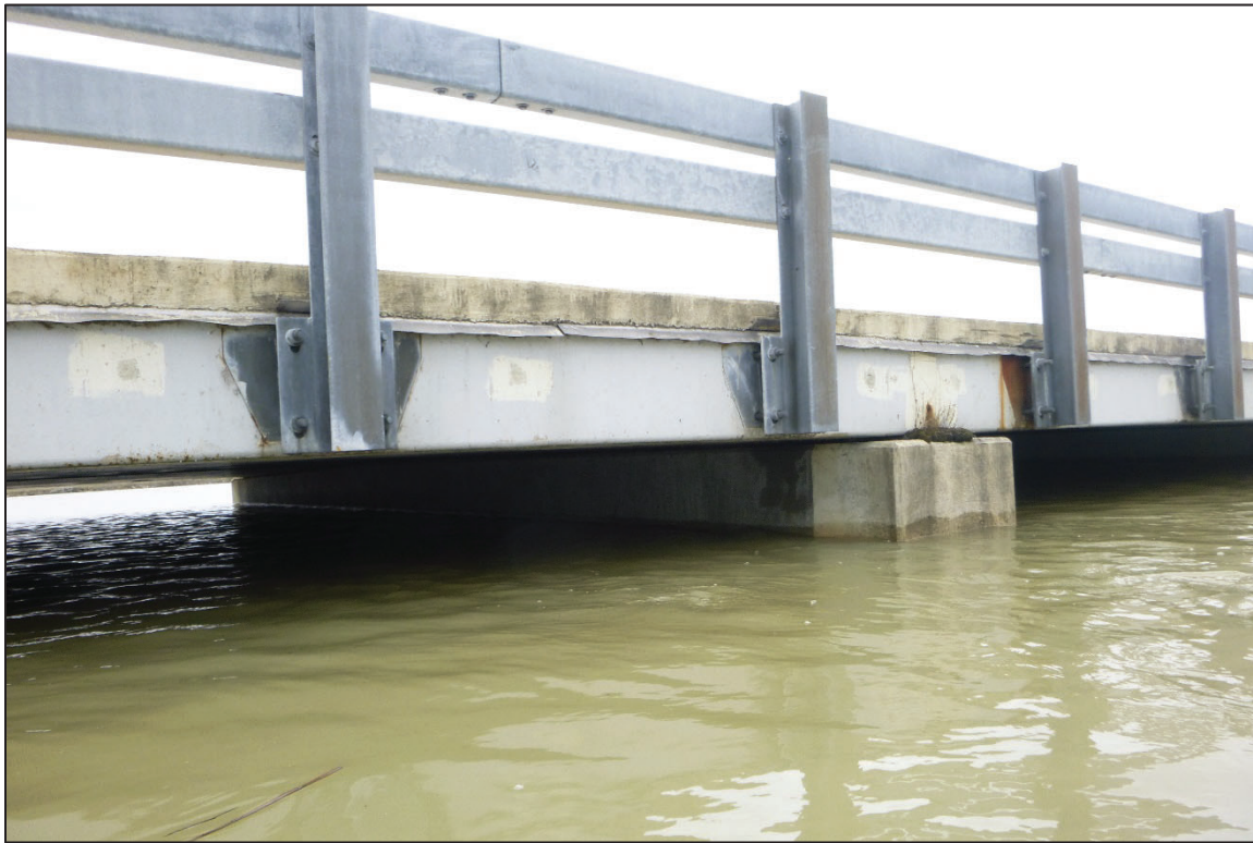
Photograph No. 13: View of the East Face of Bent 2, Looking Southwest.
