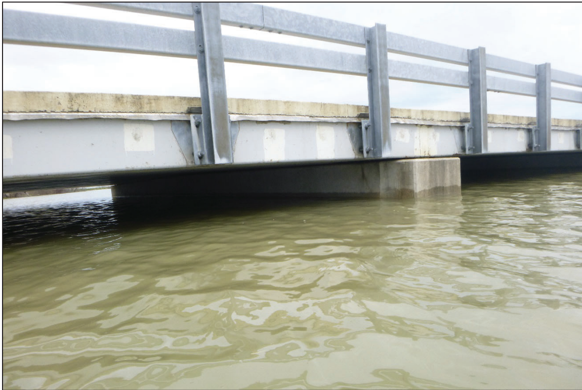
Photograph No. 12: View of the West Face of Bent 1, Looking Northeast.
