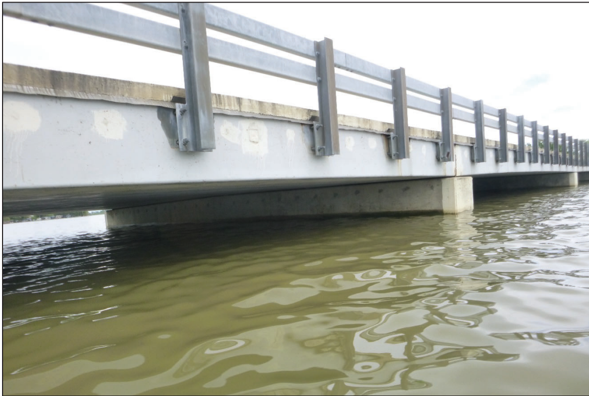
Photograph No. 13: View of the North Face of Bent 3, Looking Southeast.
