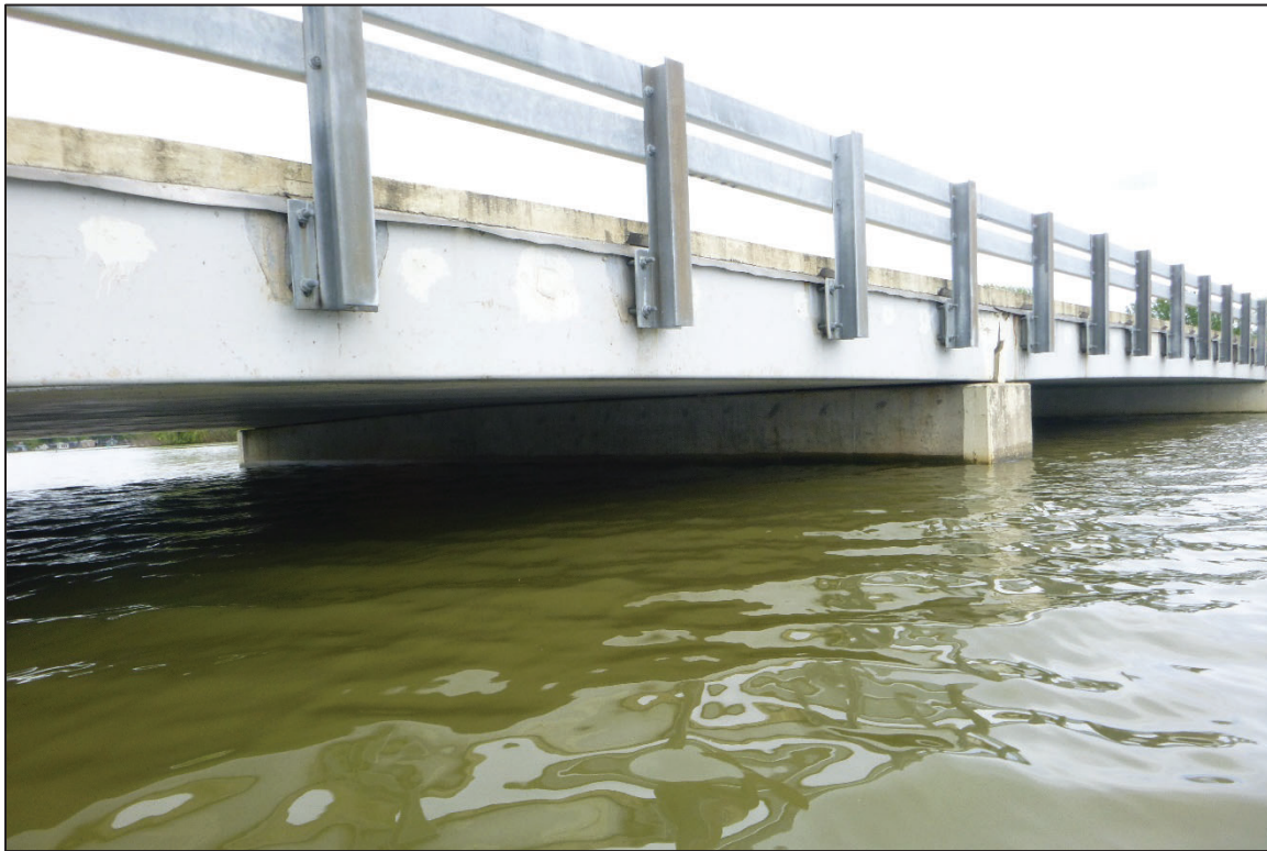
Photograph No. 17: View of the North Face of Bent 5, Looking Southeast.
