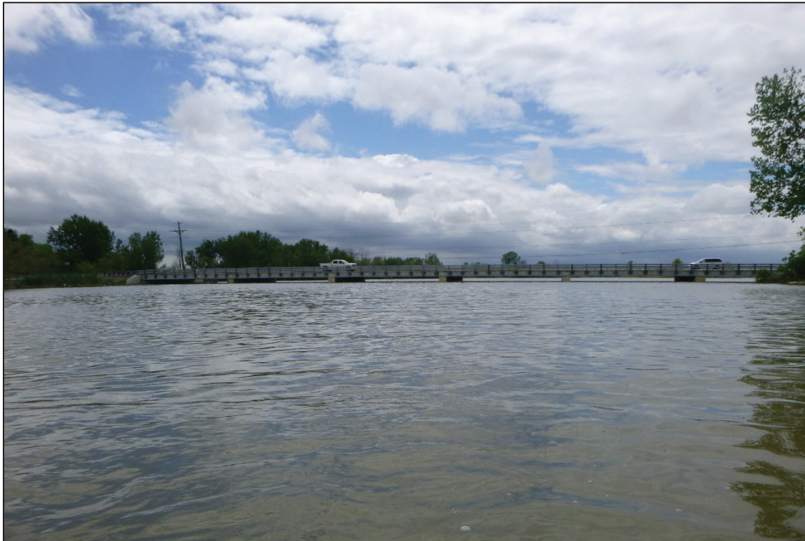
Photograph No. 2: Overall View of Structure No. 6200133 (OTT-2-1079), Looking West.
