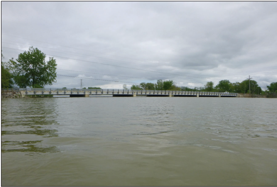
Photograph No. 1: Overall View of Structure No. 6200133 (OTT0201079), Looking East.
