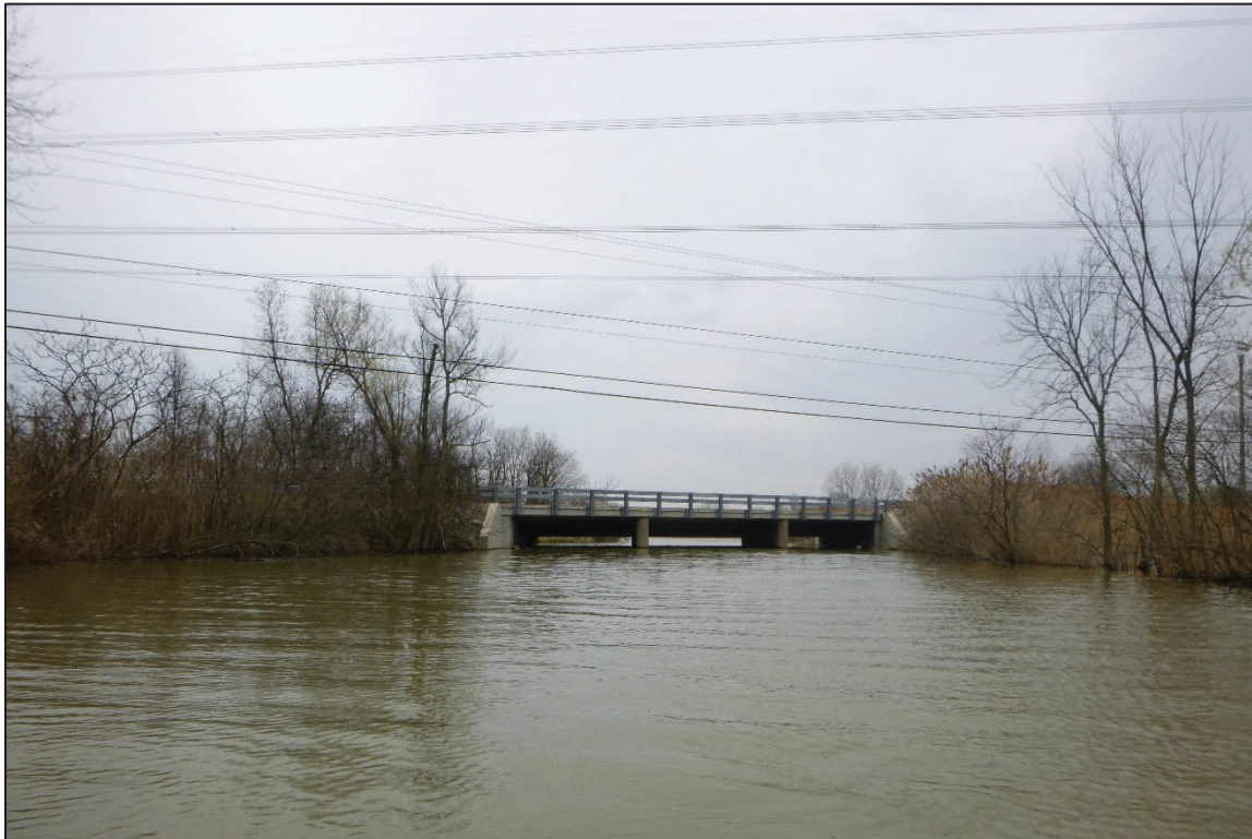
Photograph No. 2: Overall View of Structure No. 6200184 (OTT-2-1312), Looking Northeast.
