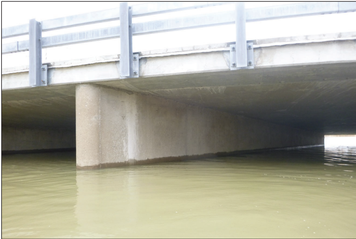
Photograph No. 13: View of the South Face of Pier 2, Looking North.
