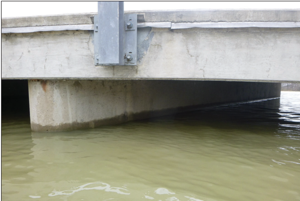
Photograph No. 10: View of the North Face of Pier 1, Looking South.
