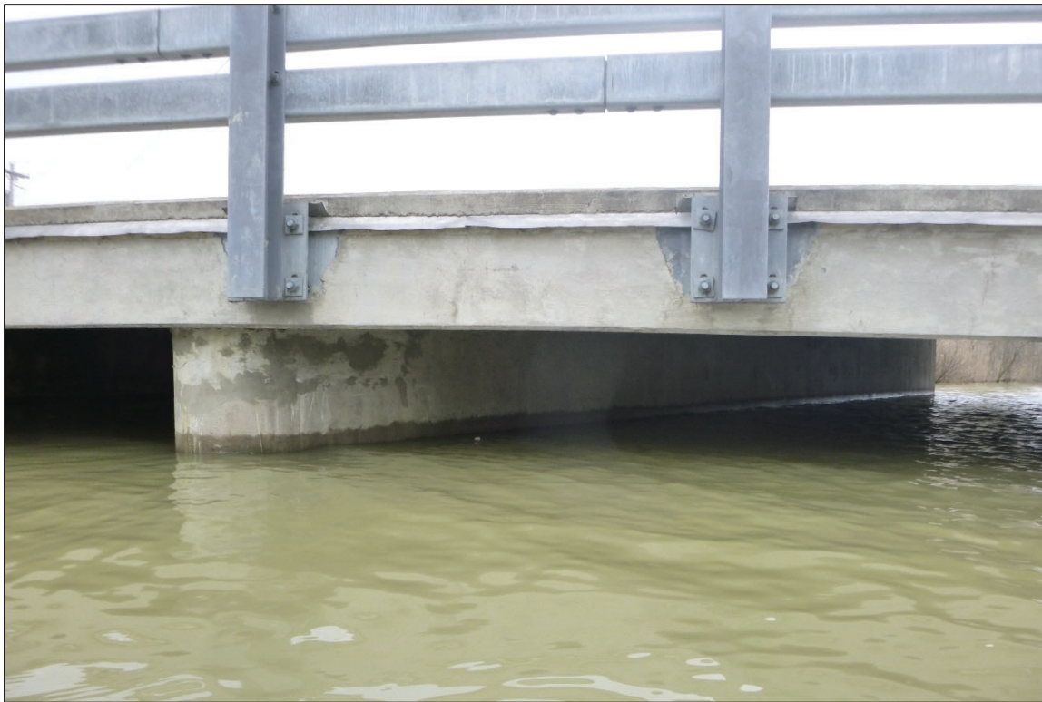
Photograph No. 12: View of the North Face of Pier 2, Looking South.
