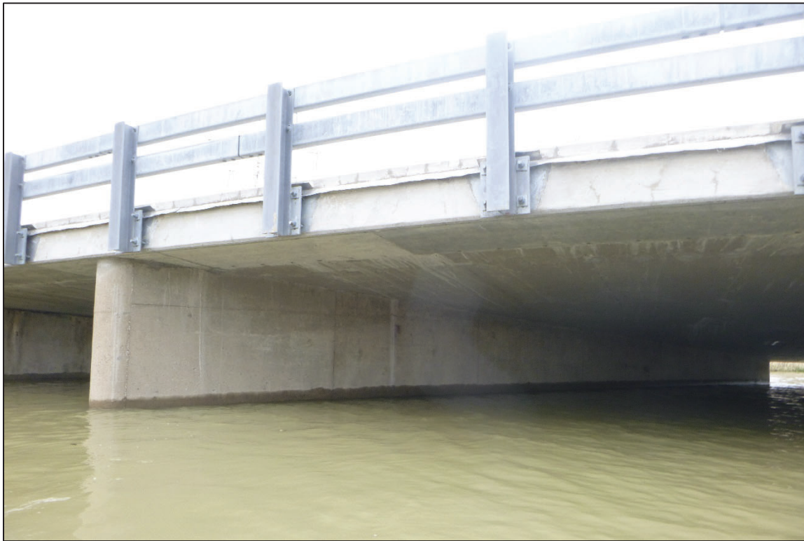
Photograph No. 11: View of the South Face of Pier 1, Looking North.
