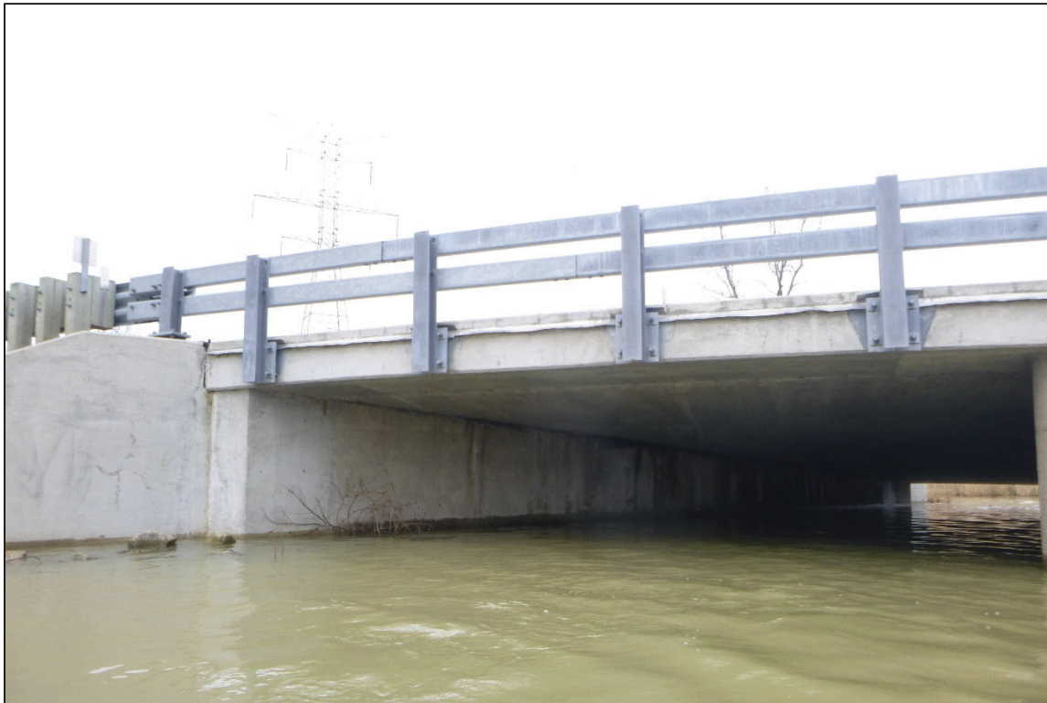
Photograph No. 4: View of the West Embankment at the Structure, Looking North.
