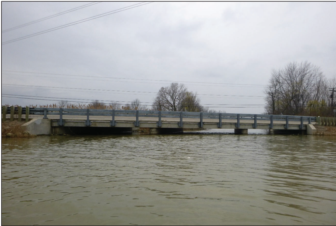
Photograph No. 1: Overall View of Structure No. 6200184 (OTT-2-1312), Looking Southwest.
