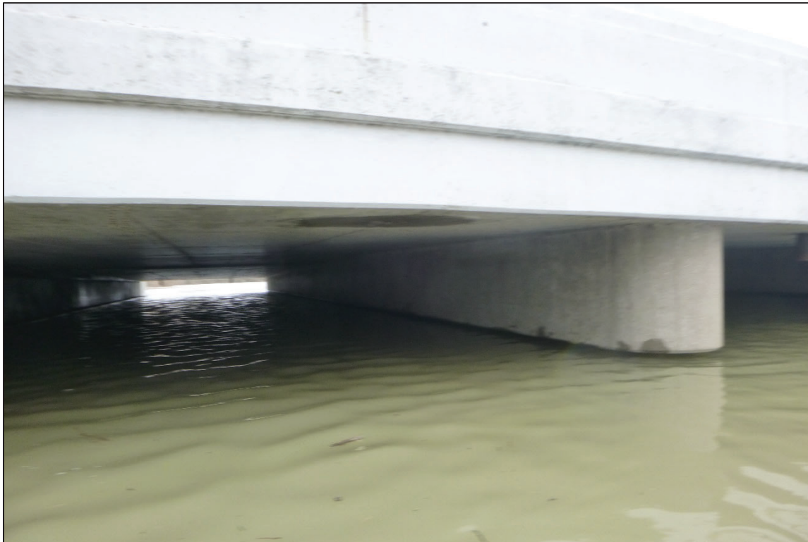
Photograph No. 12: View of the East Face of Bent 2, Looking West.
