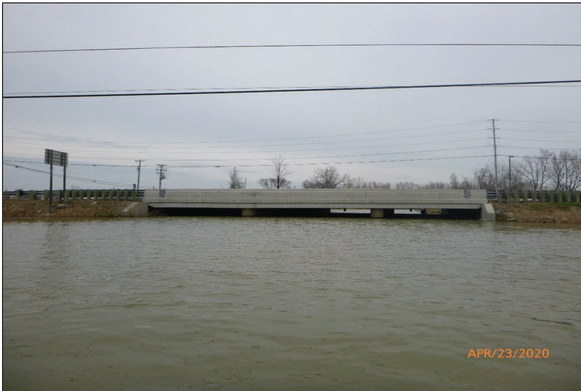
Photograph No. 2: Overall View of Structure No. 6200214 (OTT-2-1654), Looking Northeast.
