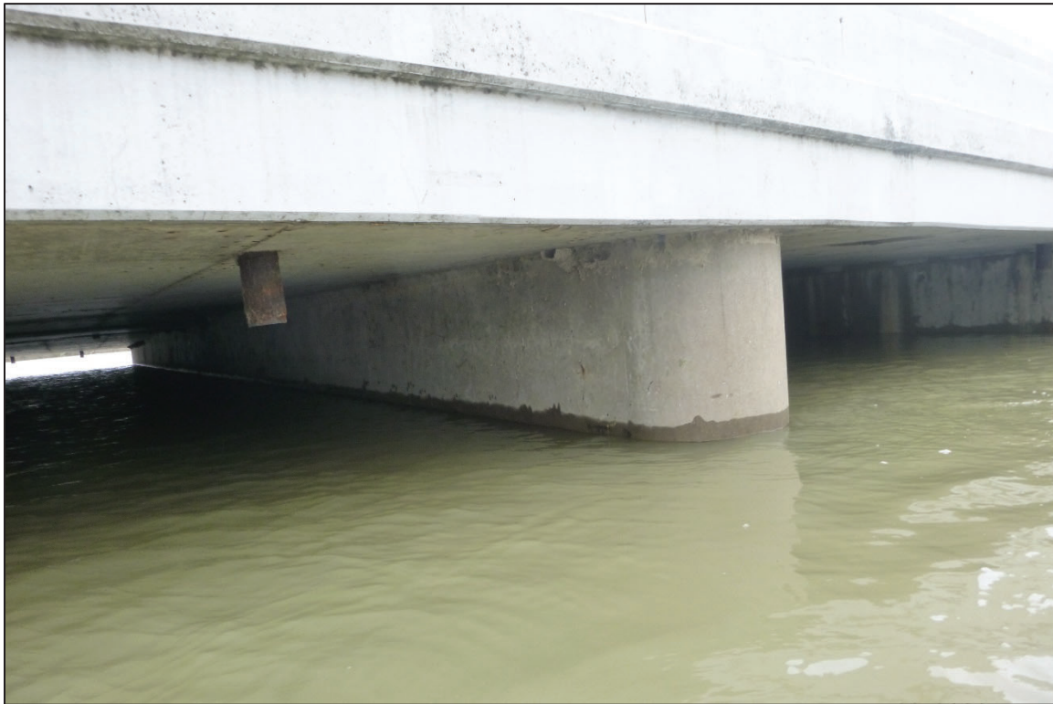
Photograph No. 10: View of the East Face of Bent 1, Looking West.
