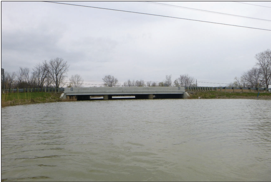
Photograph No. 1: Overall View of Structure No. 6200214 (OTT-2-1654), Looking Southwest.
