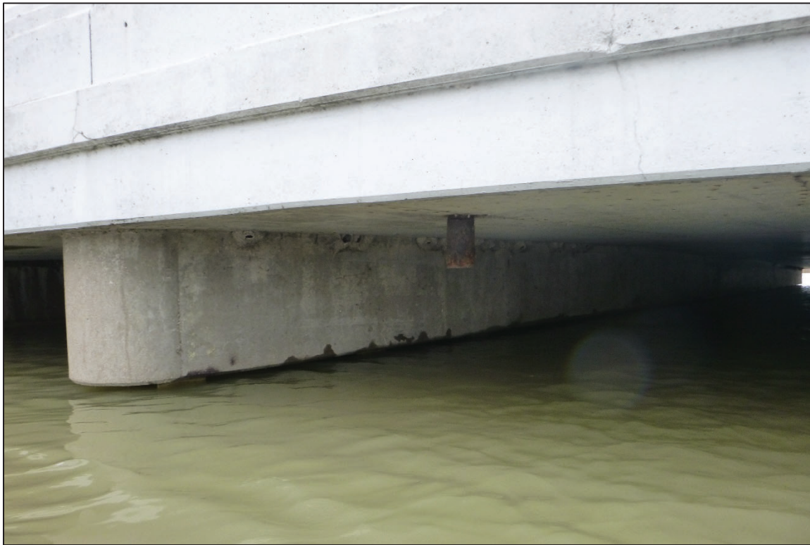
Photograph No. 11: View of the West Face of Bent 2, Looking South.
