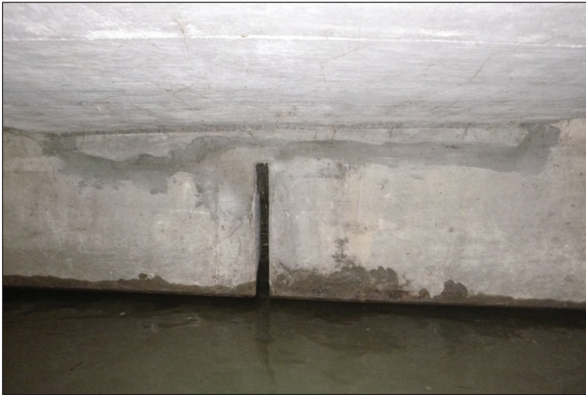
Photograph No. 15: View of the Typical Joint at Bent, Looking West.
