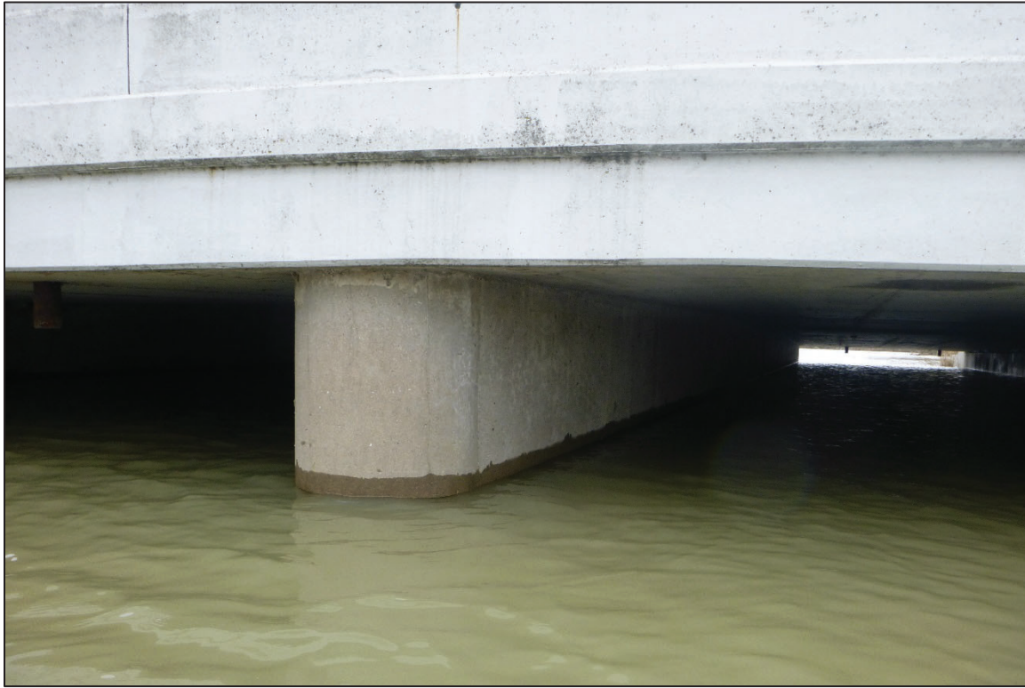
Photograph No. 9: View of the West Face of Bent 1, Looking South.
