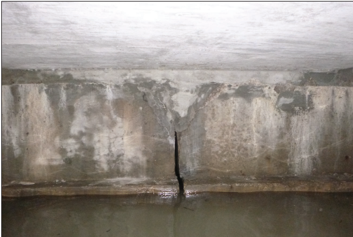
Photograph No. 14: View of the Typical Joint at Abutment, Looking East.
