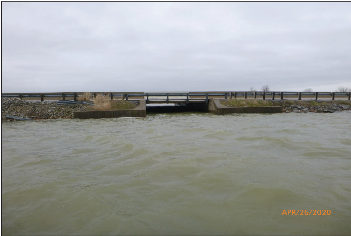
Photograph No. 1: Overall View of Structure No. 6200303 (OTT-2-1810), Looking South.
