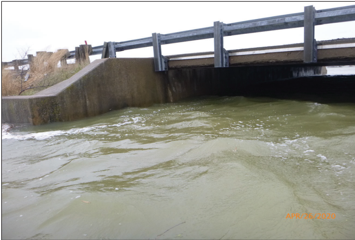
Photograph No. 9: View of the North Corner of Abutment 2, Looking Southeast.
