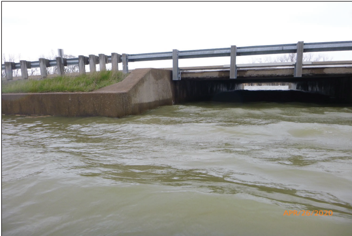
Photograph No. 8: View of the South Corner of Abutment 1, Looking Northwest.
