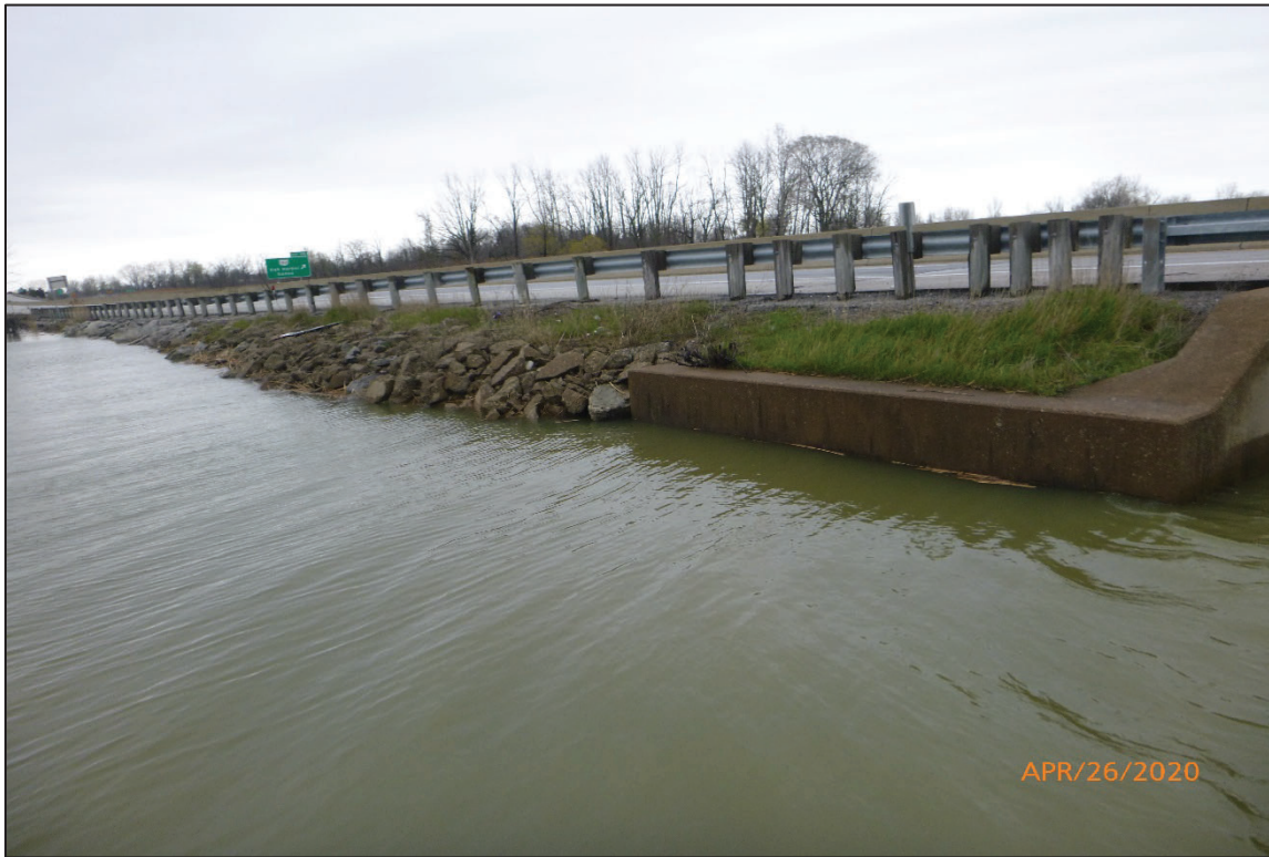
Photograph No. 3: View of the West Embankment Upstream of the Structure, Looking Northwest.
