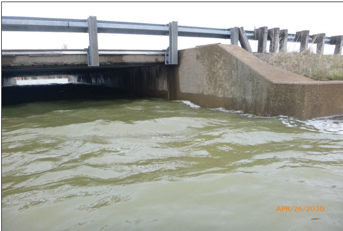
Photograph No. 10: View of the South Corner of Abutment 2, Looking Northeast.
