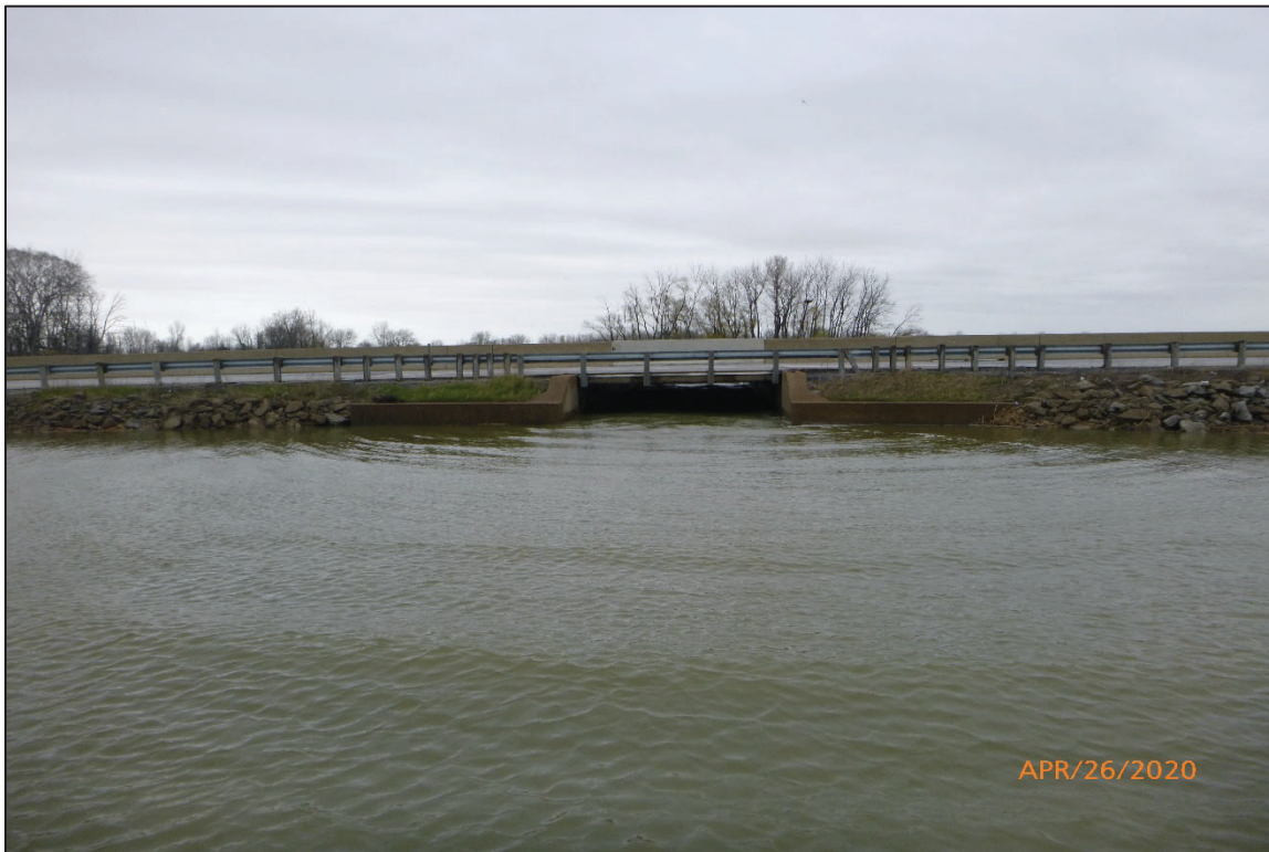
Photograph No. 2: Overall View of Structure No. 6200303 (OTT-2-1810), Looking North.
