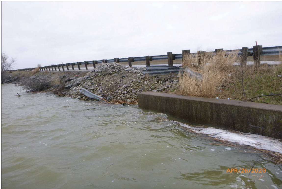
Photograph No. 6: View of the East Embankment Downstream of the Structure, Looking Southeast.
