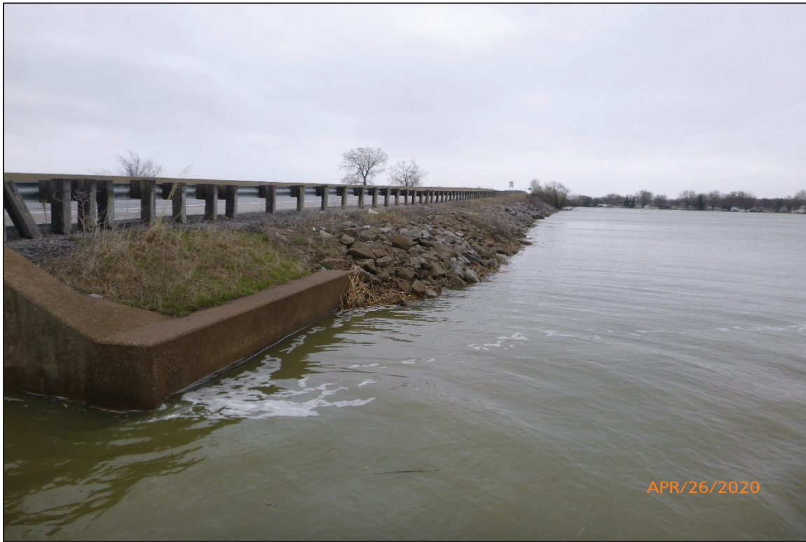
Photograph No. 5: View of the East Embankment Upstream of the Structure, Looking Northeast.
