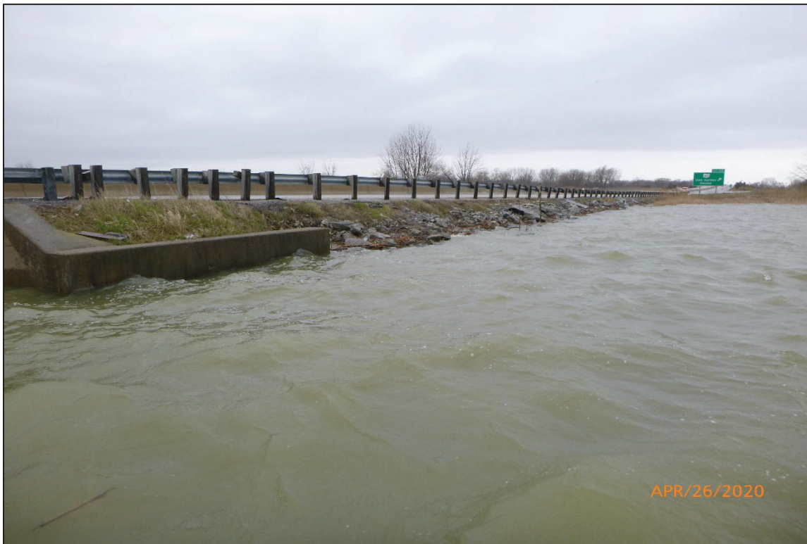
Photograph No. 4: View of the West Embankment Downstream of the Structure, Looking Southwest.
