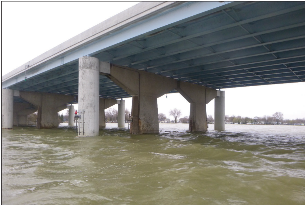
Photograph No. 11: View of the West Face of Pier 2, Looking South.
