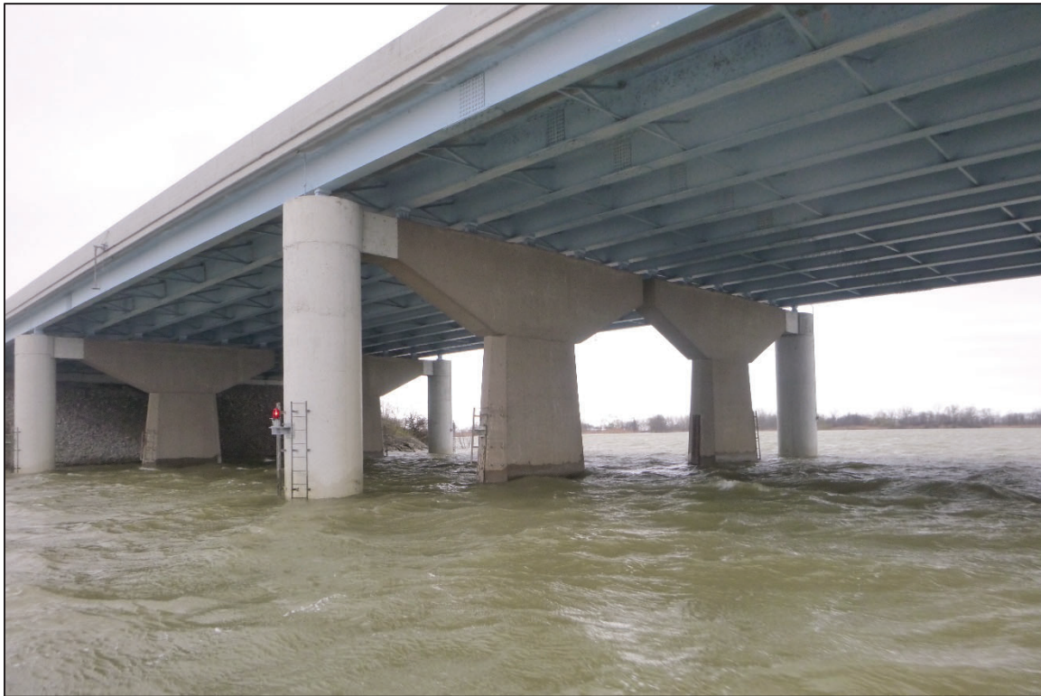
Photograph No. 12: View of the East Face of Pier 2, Looking North.
