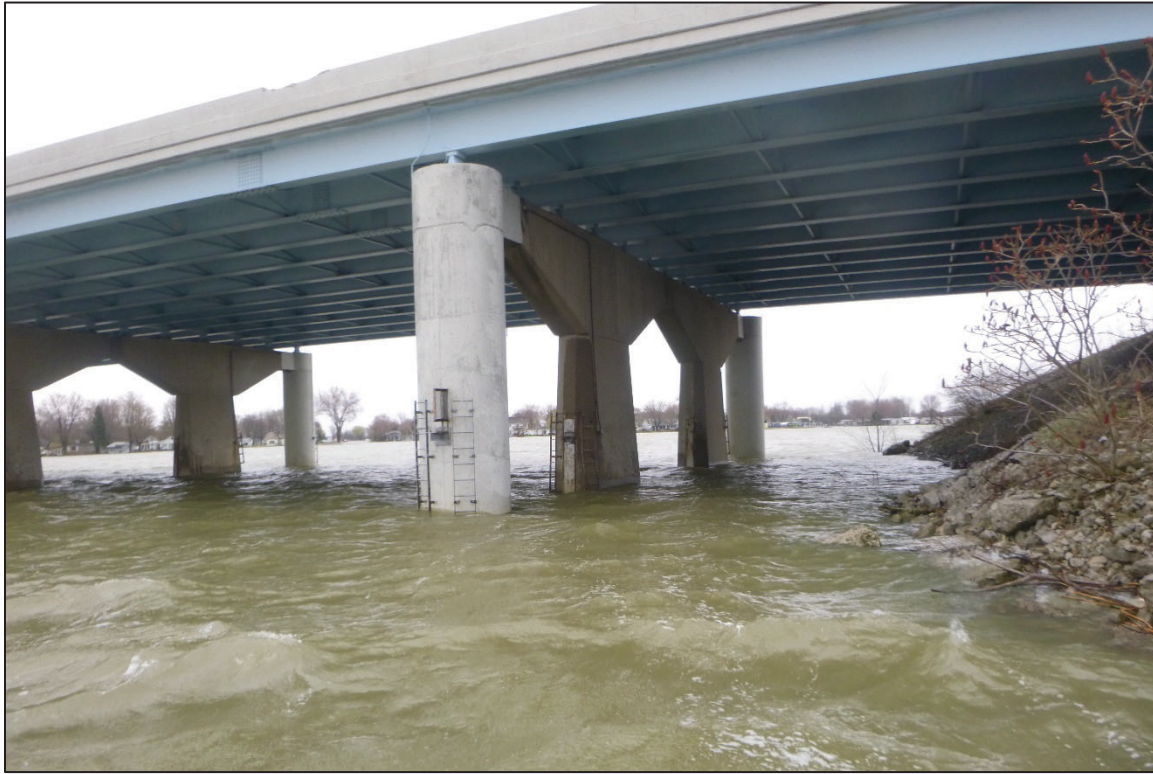
Photograph No. 9: View of the West Face of Pier 1, Looking South.
