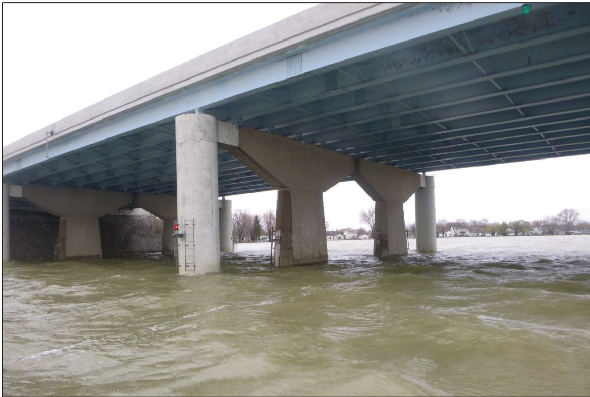
Photograph No. 16: View of the West Face of Pier 4, Looking South.
