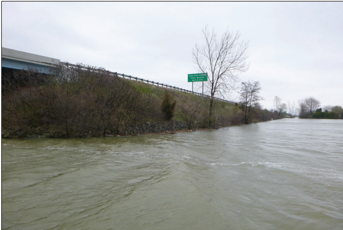
Photograph No. 6: View of the East Embankment Upstream of the Structure, Looking East.
