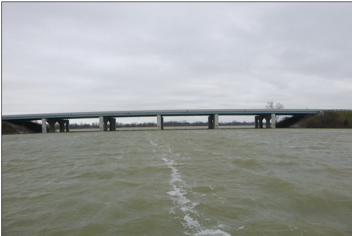
Photograph No. 2: Overall View of Structure No. 6200338 (OTT-2-1830), Looking Northeast.
