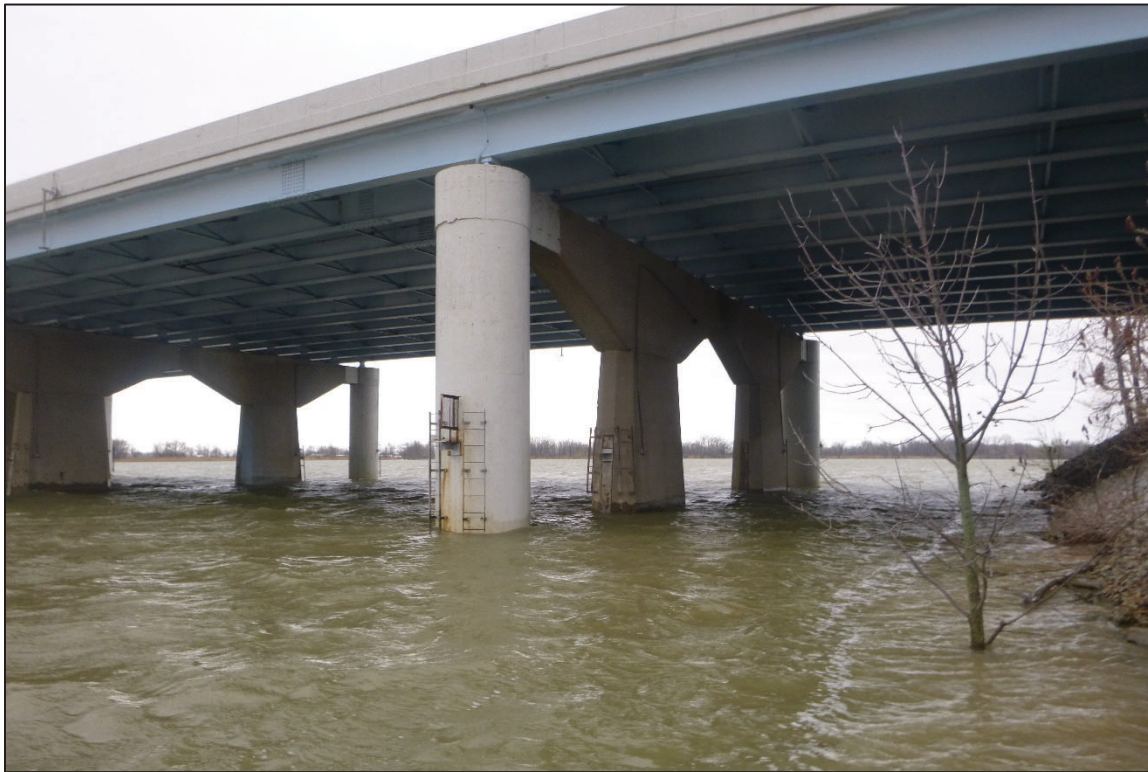
Photograph No. 19: View of the East Face of Pier 5, Looking North.
