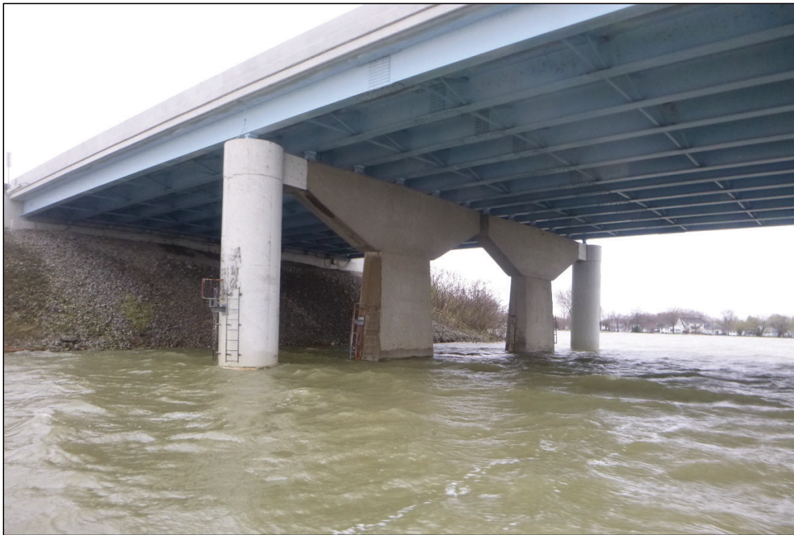
Photograph No. 18: View of the West Face of Pier 5, Looking South.
