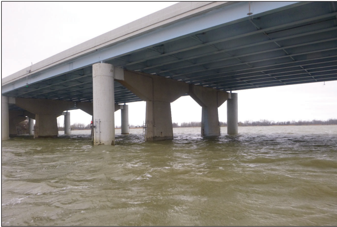
Photograph No. 17: View of the East Face of Pier 4, Looking North.
