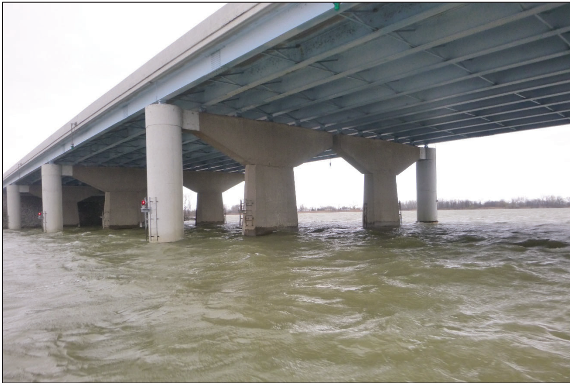
Photograph No. 15: View of the East Face of Pier 3, Looking North.
