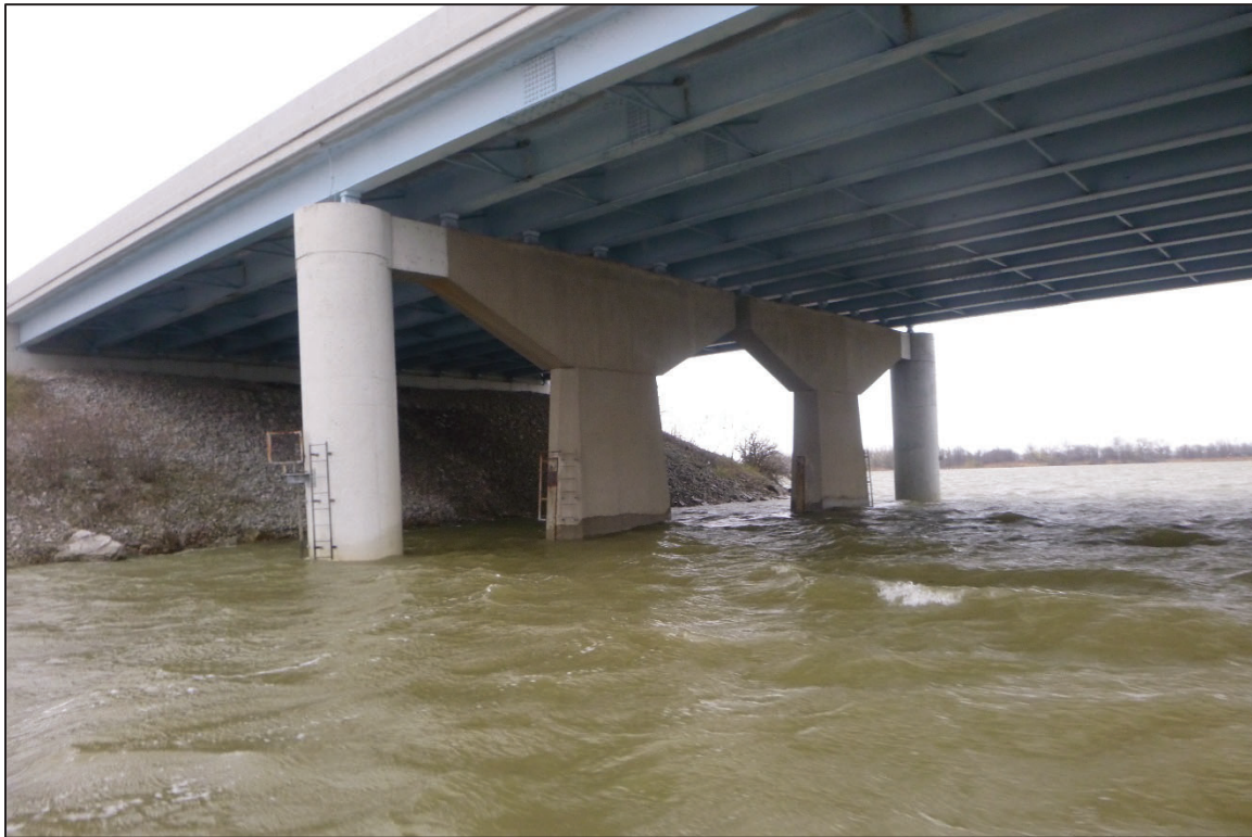
Photograph No. 10: View of the East Face of Pier 1, Looking North.
