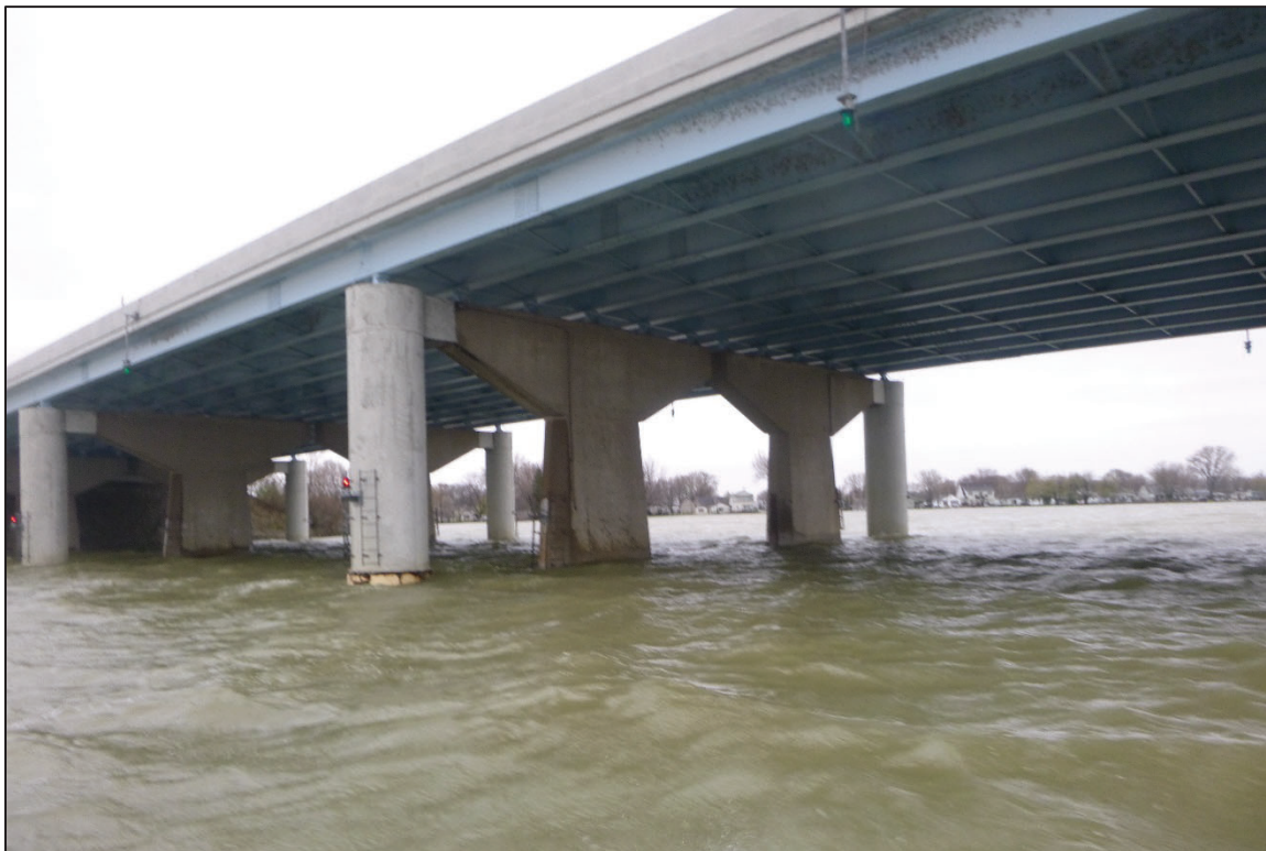
Photograph No. 14: View of the West Face of Pier 3, Looking South.
