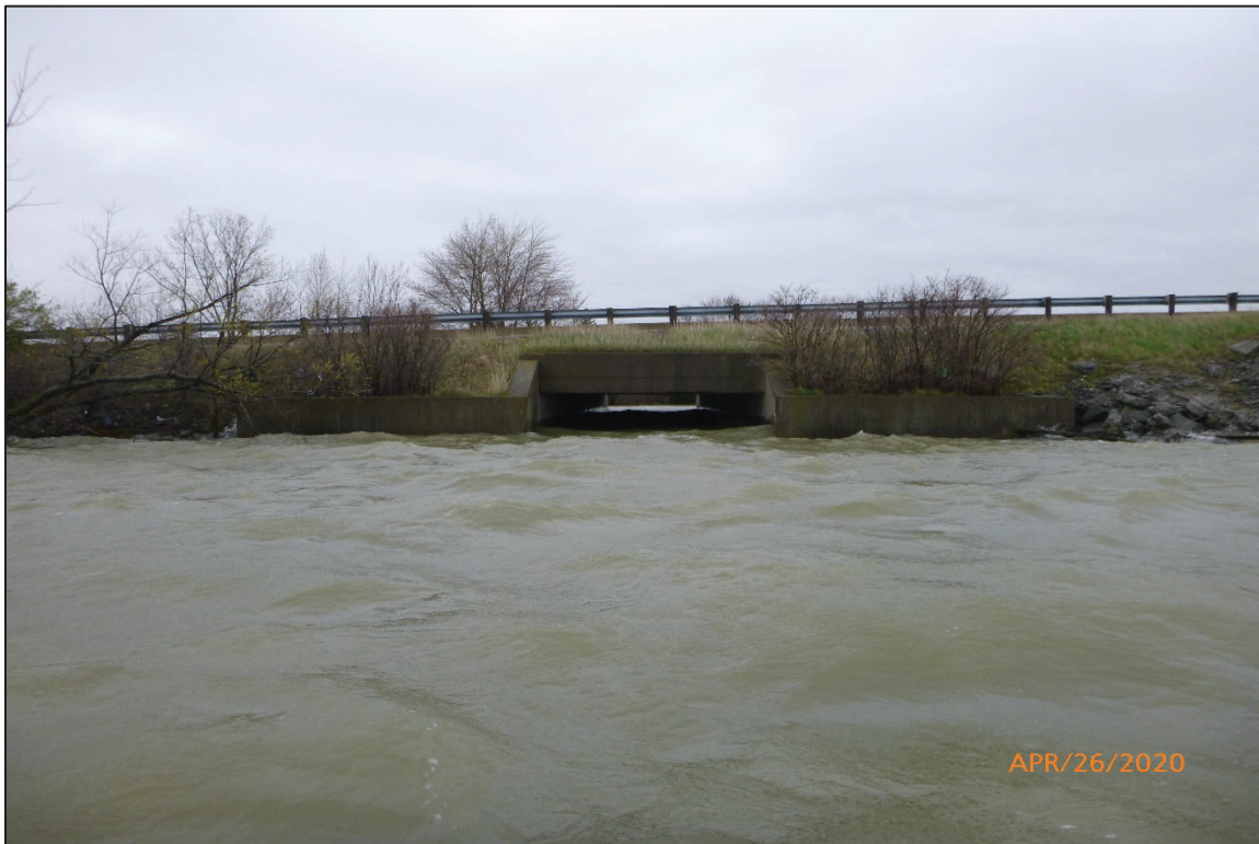
Photograph No. 2: Overall View of Structure No. 6200362 (OTT-2-1853), Looking South.
