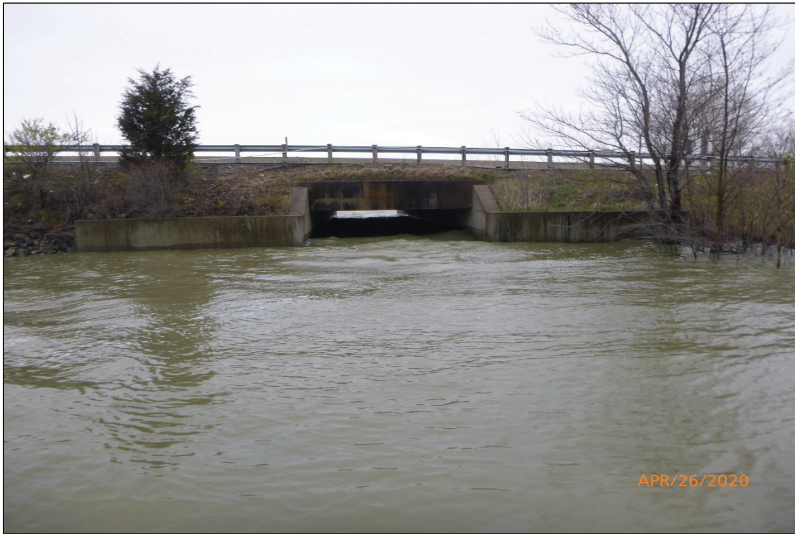
Photograph No. 1: Overall View of Structure No. 6200362 (OTT-2-1853), Looking North.
