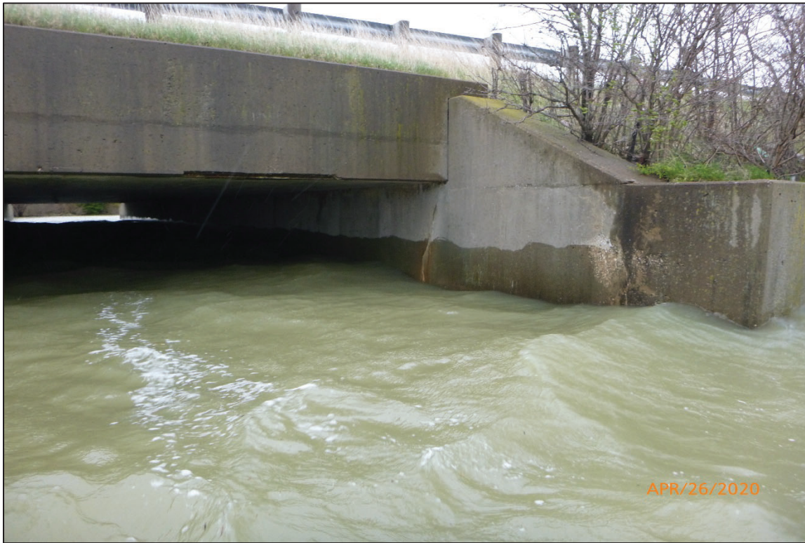
Photograph No. 7: View of the North Corner of Abutment 1, Looking Southwest.
