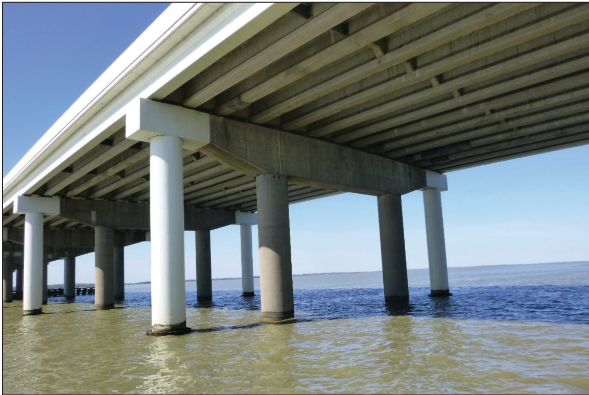
Photograph No. 21: View of the North Face of Bent 7, Looking Southwest.
