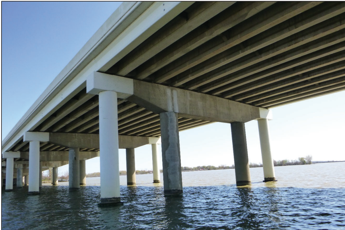
Photograph No. 22: View of the South Face of Bent 7, Looking Northeast.
