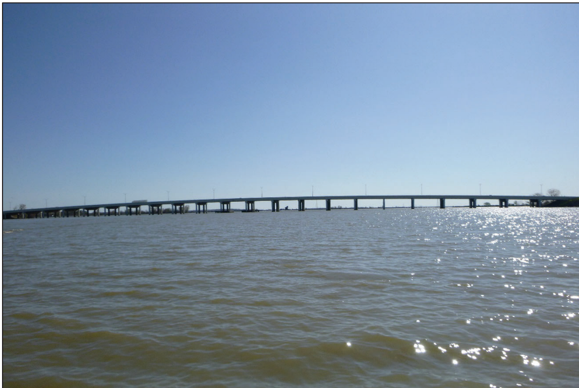
Photograph No. 2: Overall View of Structure No. 6200788 (OTT-2-2839), Looking East.
