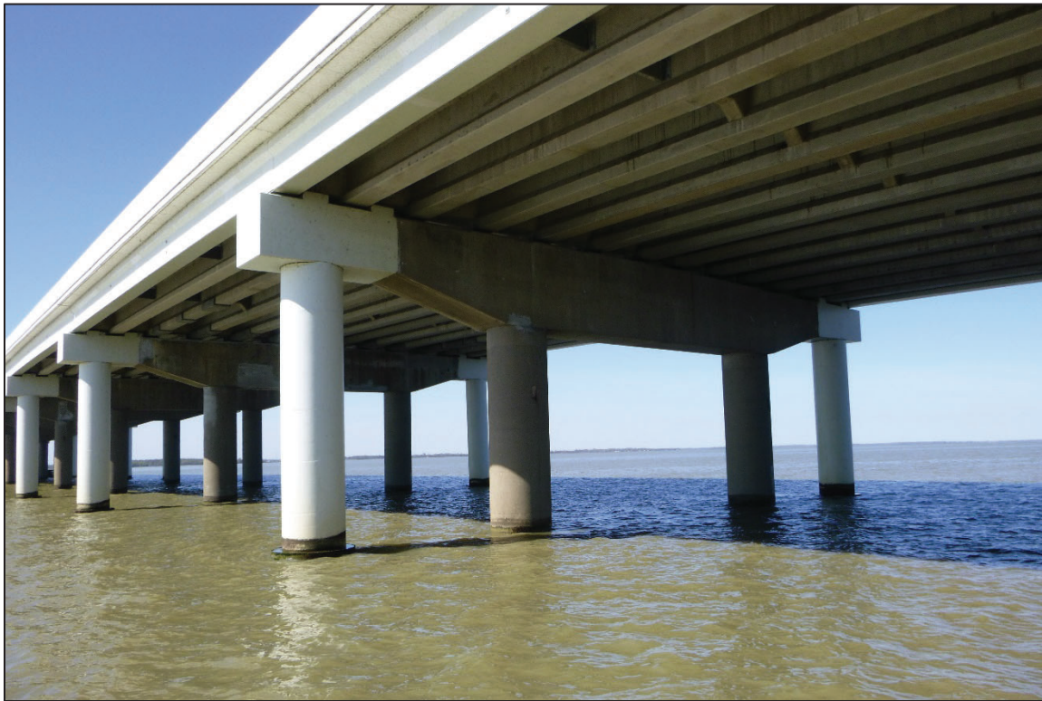
Photograph No. 13: View of the North Face of Bent 3, Looking Southwest.
