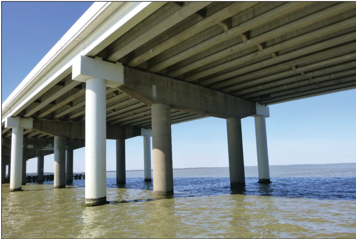
Photograph No. 23: View of the North Face of Bent 8, Looking Southwest.
