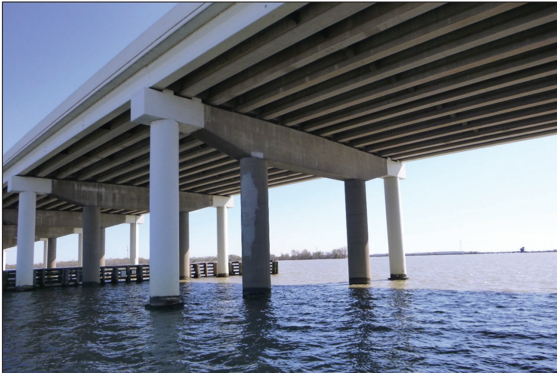
Photograph No. 34: View of the South Face of Bent 13, Looking Northeast.
