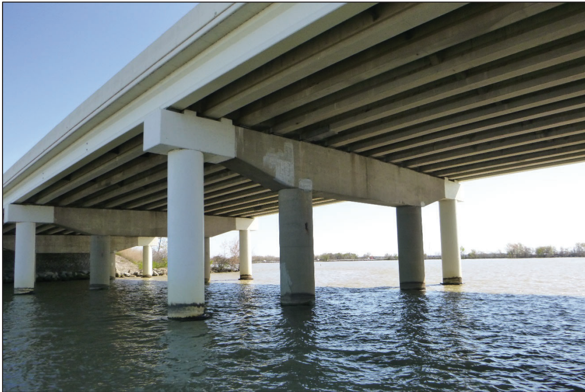
Photograph No. 14: View of the South Face of Bent 3, Looking Northeast.
