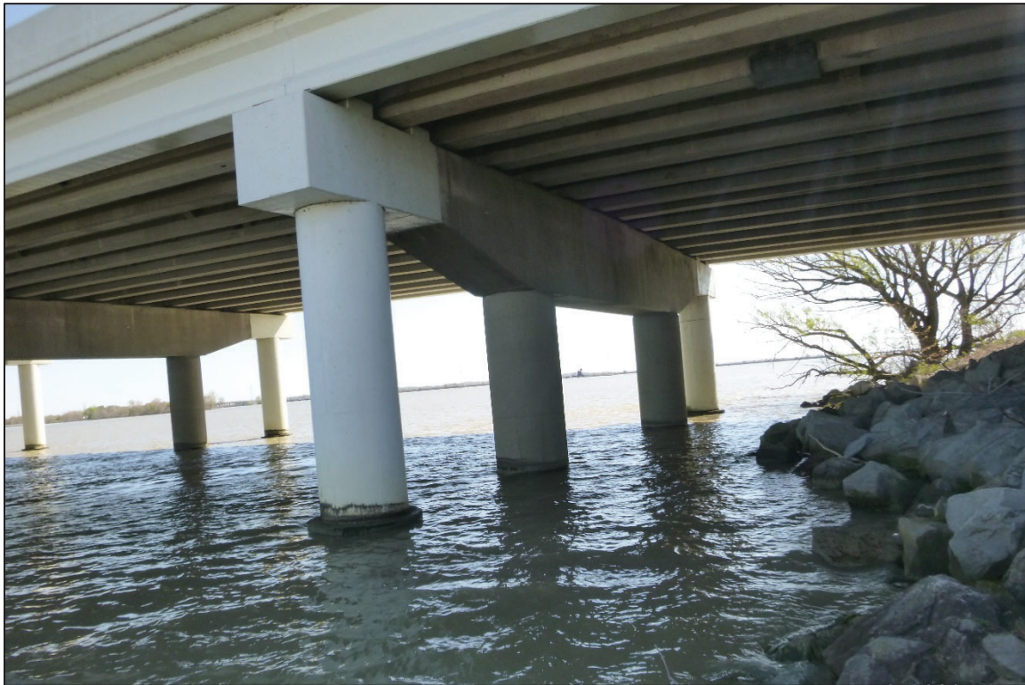
Photograph No. 52: View of the South Face of Bent 22, Looking Northeast.
