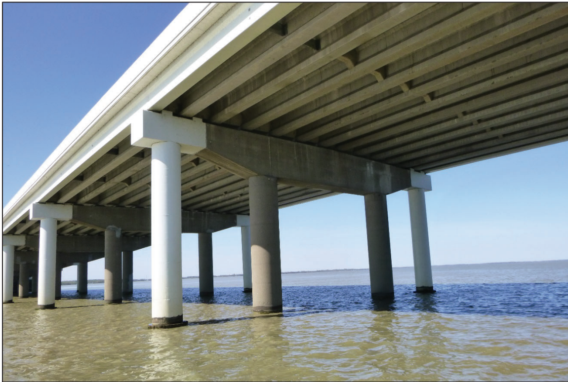
Photograph No. 37: View of the North Face of Bent 15, Looking Southwest.
