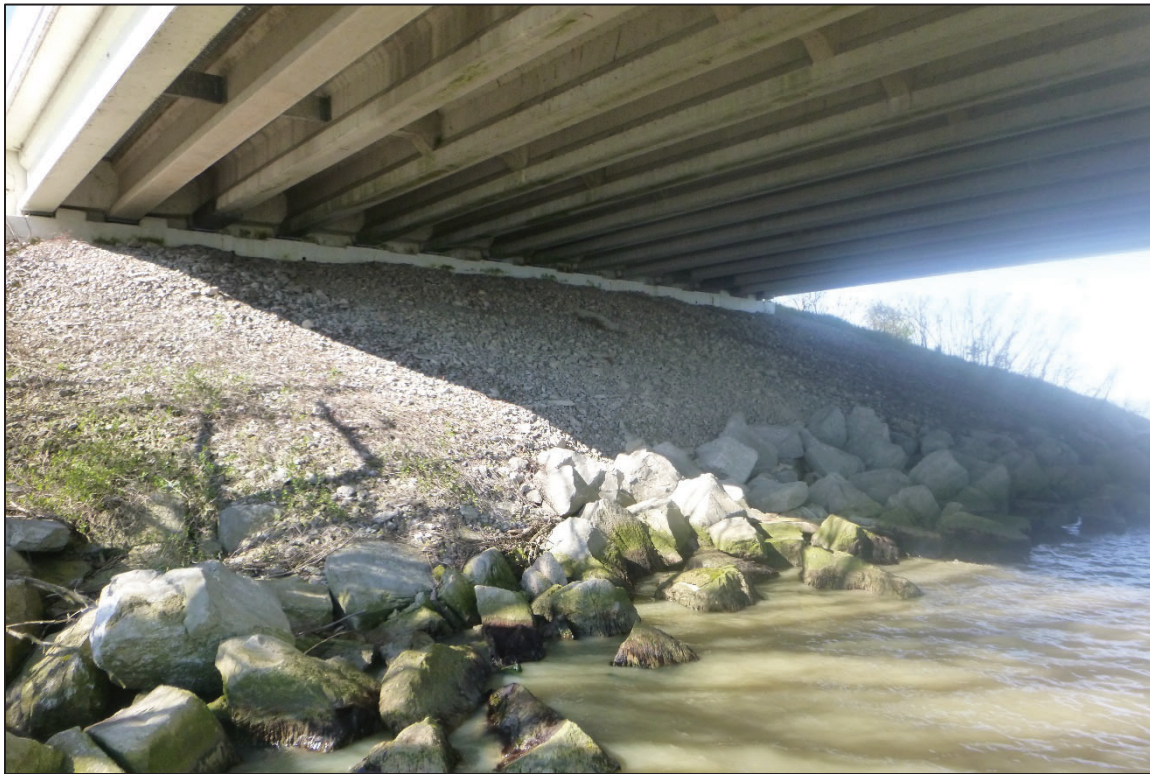
Photograph No. 7: View of the South Embankment at the Structure, Looking Southwest.
