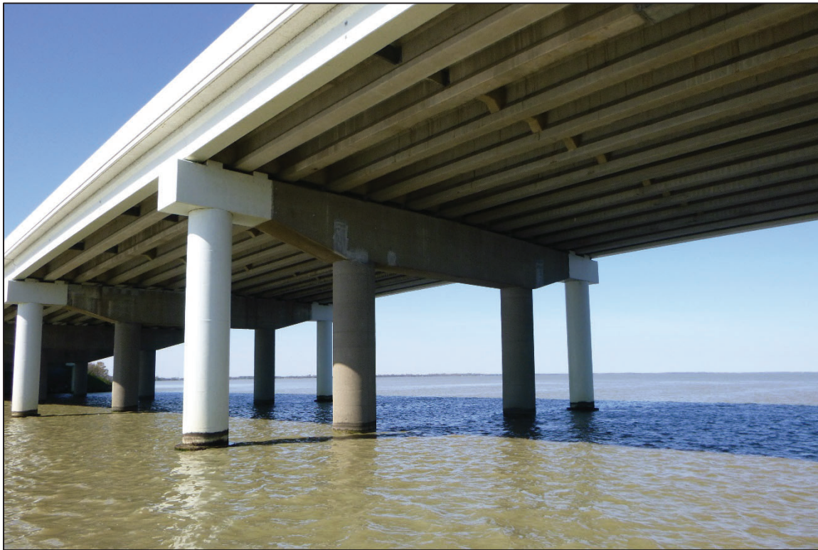
Photograph No. 43: View of the North Face of Bent 18, Looking Southwest.
