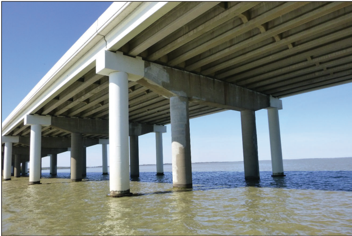
Photograph No. 35: View of the North Face of Bent 14, Looking Southwest.
