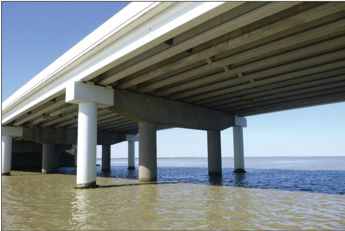
Photograph No. 47: View of the North Face of Bent 20, Looking Southwest.
