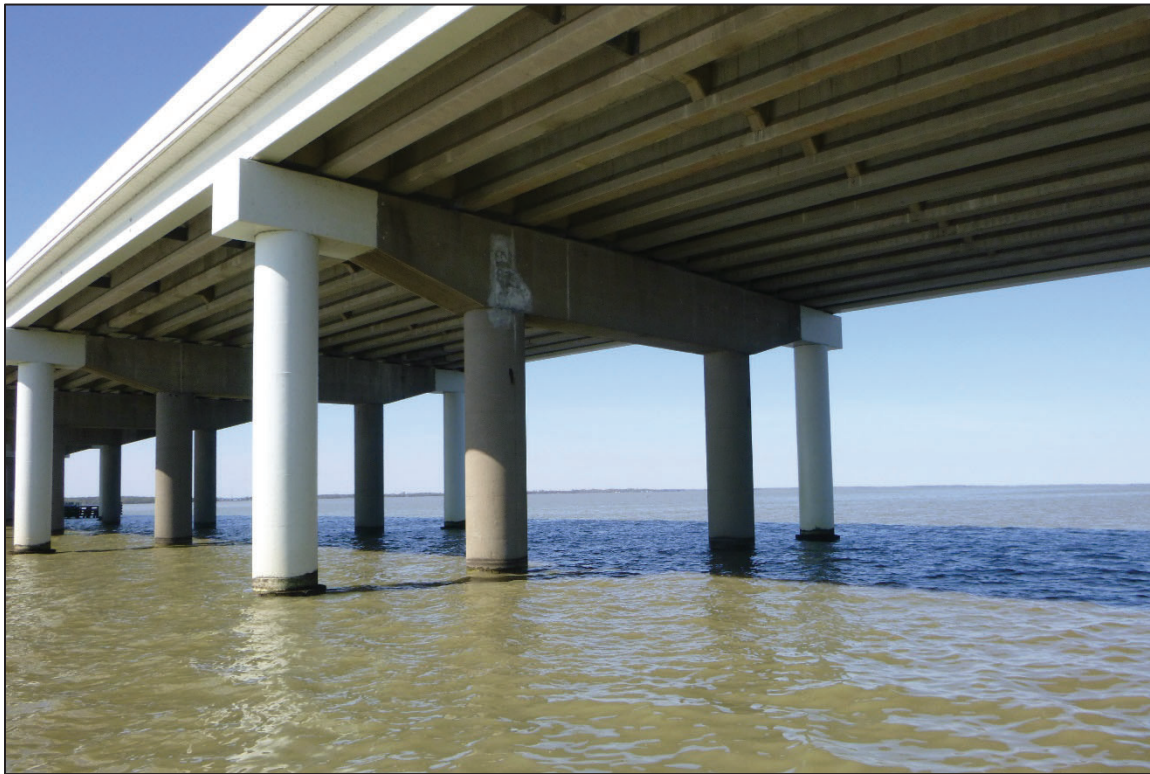
Photograph No. 19: View of the North Face of Bent 6, Looking Southwest.
