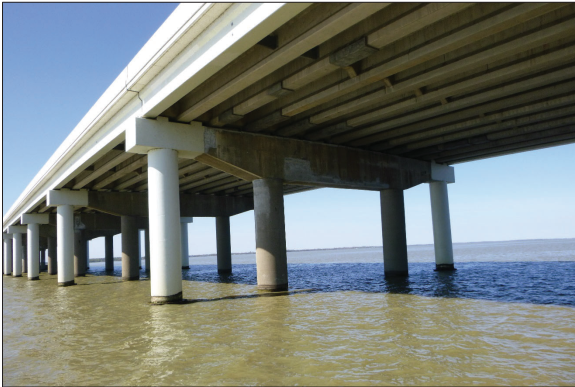
Photograph No. 15: View of the North Face of Bent 4, Looking Southwest.
