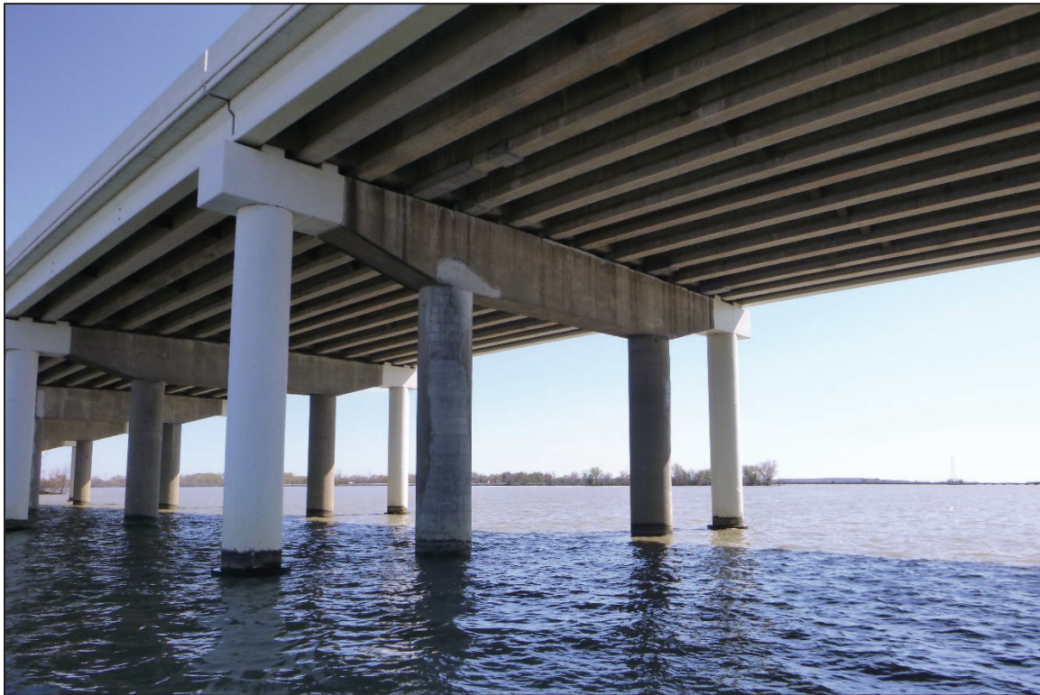
Photograph No. 26: View of the South Face of Bent 9, Looking Northeast.
