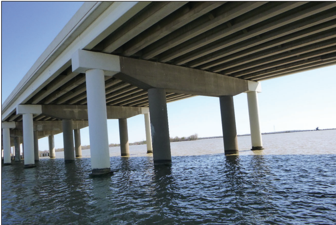
Photograph No. 42: View of the South Face of Bent 17, Looking Northeast.
