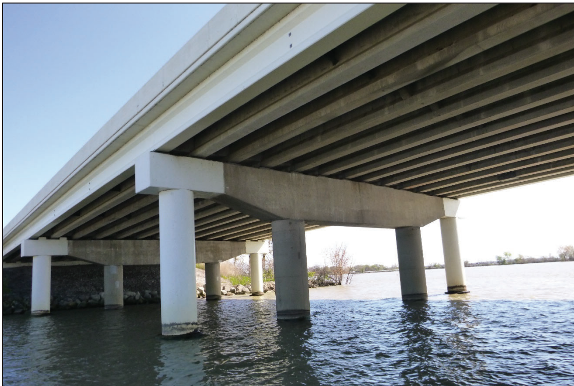
Photograph No. 12: View of the South Face of Bent 2, Looking Northeast.
