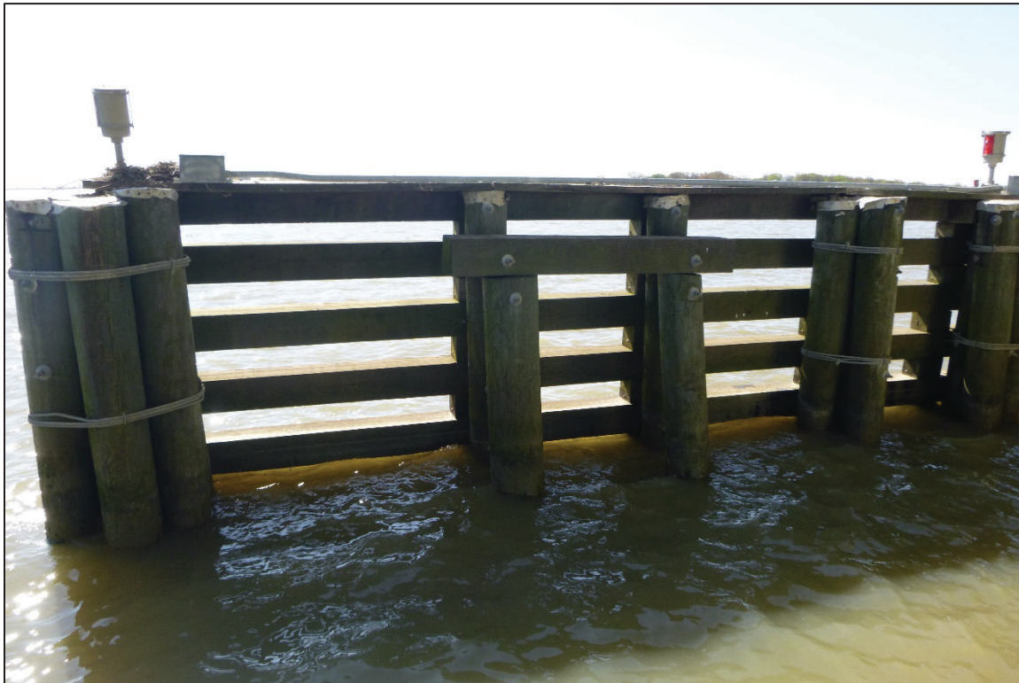
Photograph No. 56: View of the Timber Downstream Fender System, Looking Southeast.
