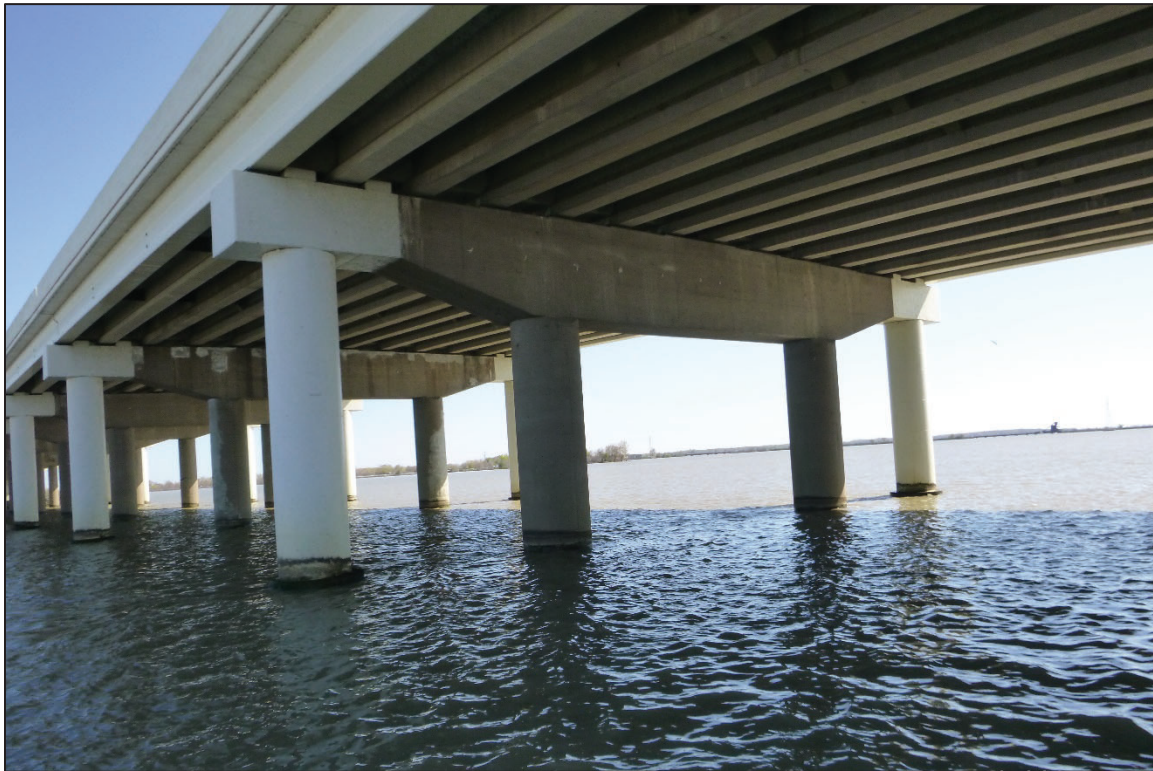
Photograph No. 48: View of the South Face of Bent 20, Looking Northeast.
