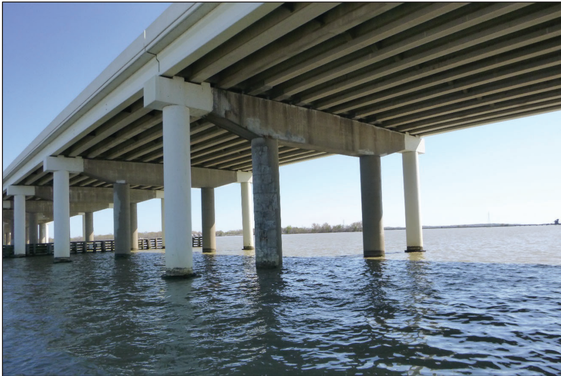
Photograph No. 36: View of the South Face of Bent 14, Looking Northeast.
