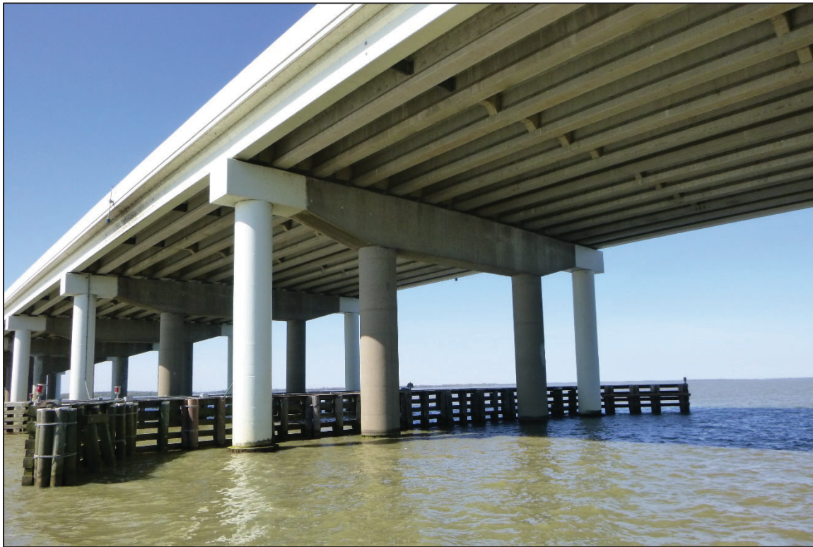
Photograph No. 29: View of the North Face of Bent 11, Looking Southwest.
