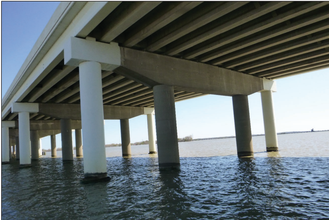
Photograph No. 44: View of the South Face of Bent 18, Looking Northeast.
