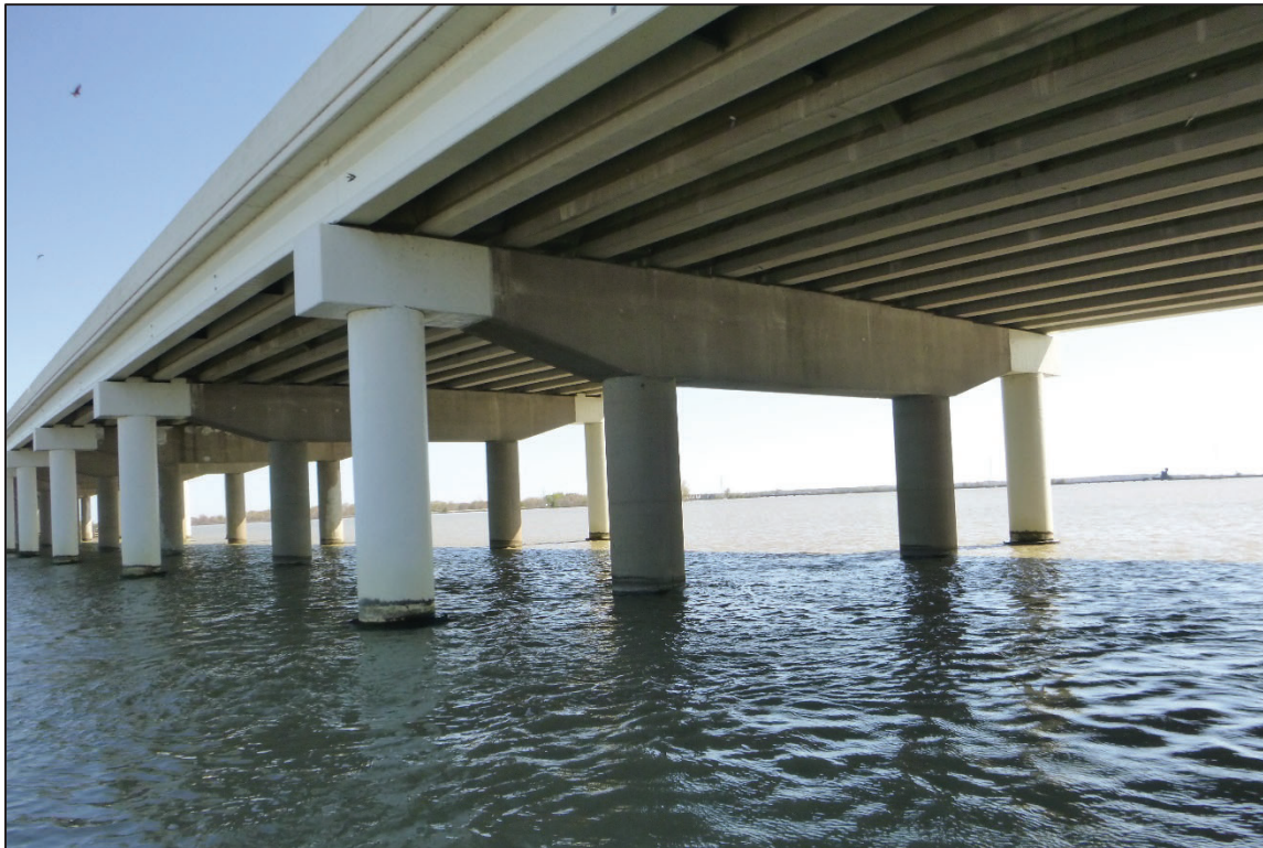
Photograph No. 50: View of the South Face of Bent 21, Looking Northeast.
