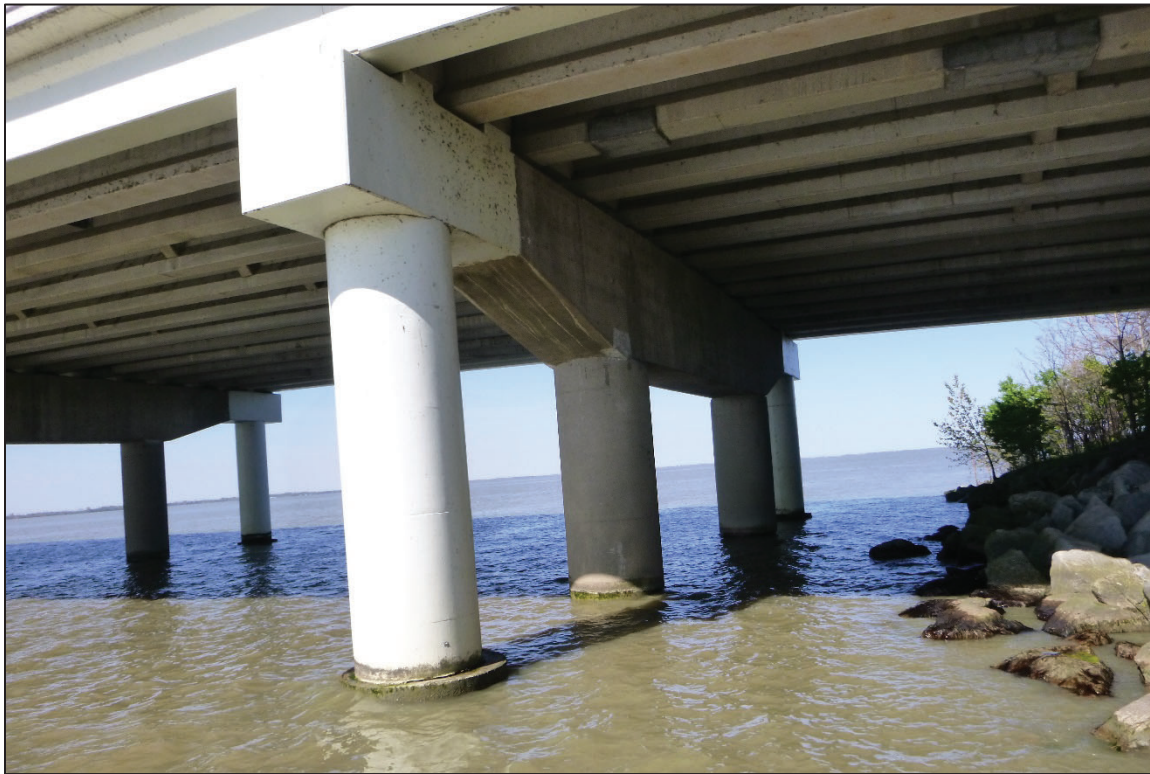
Photograph No. 9: View of the North Face of Bent 1, Looking Southwest.
