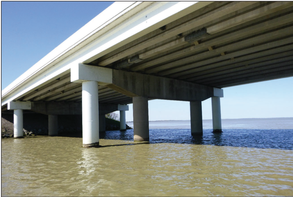
Photograph No. 49: View of the North Face of Bent 21, Looking Southwest.
