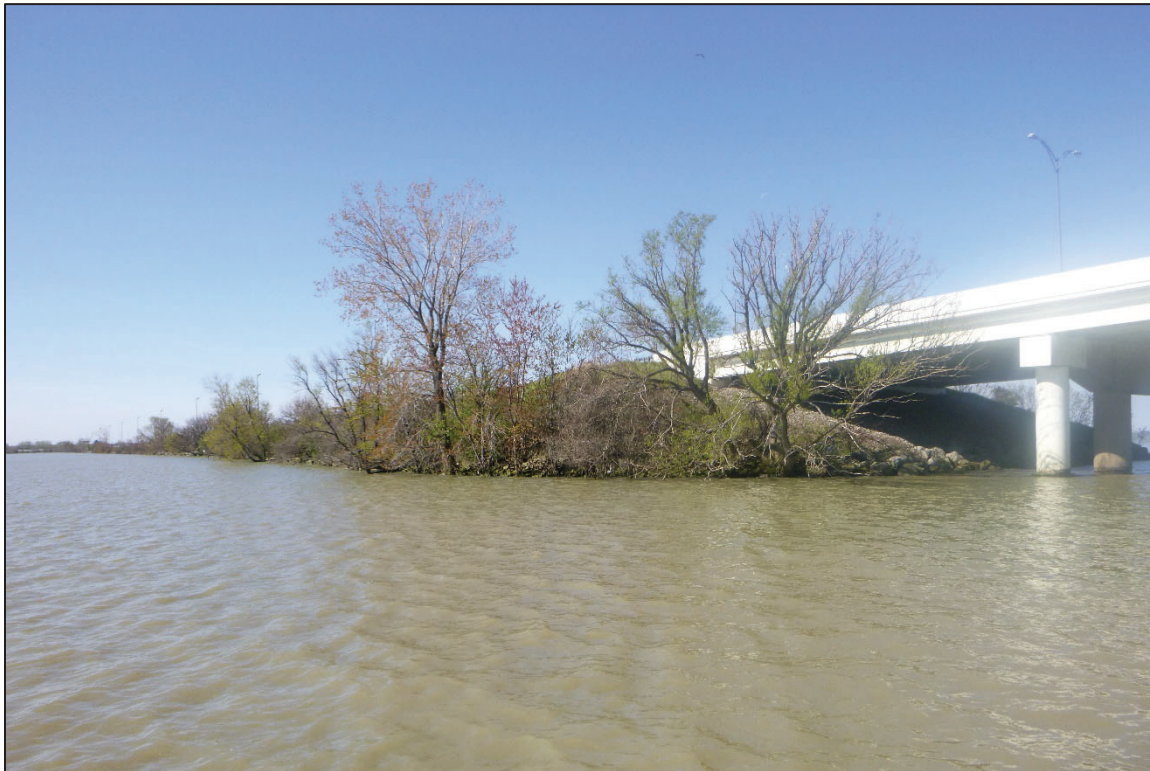
Photograph No. 8: View of the South Embankment Downstream of the Structure, Looking Southwest.
