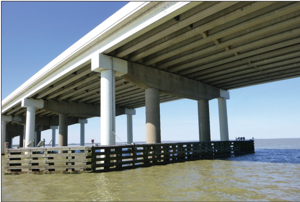
Photograph No. 31: View of the North Face of Bent 12, Looking Southwest.
