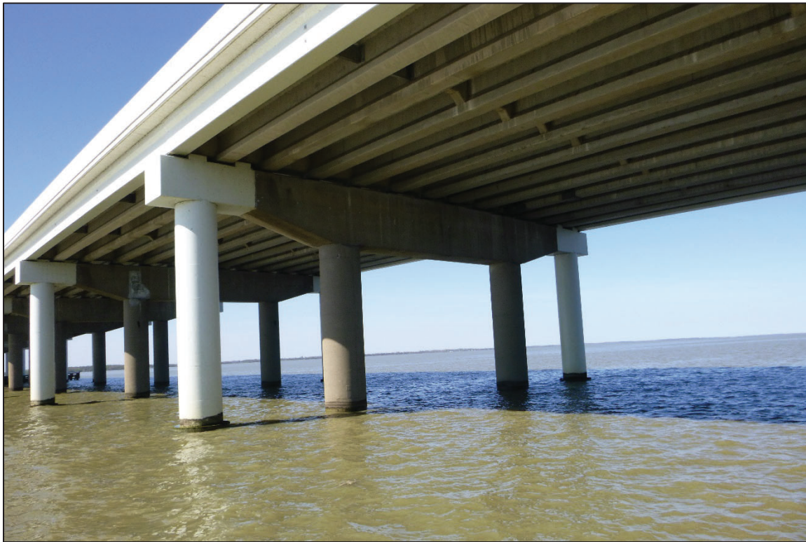
Photograph No. 17: View of the North Face of Bent 5, Looking Southwest.
