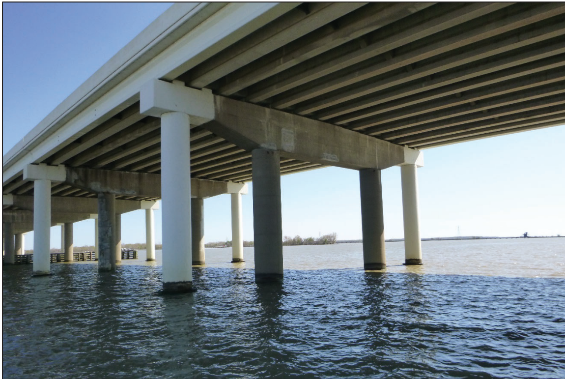
Photograph No. 38: View of the South Face of Bent 15, Looking Northeast.
