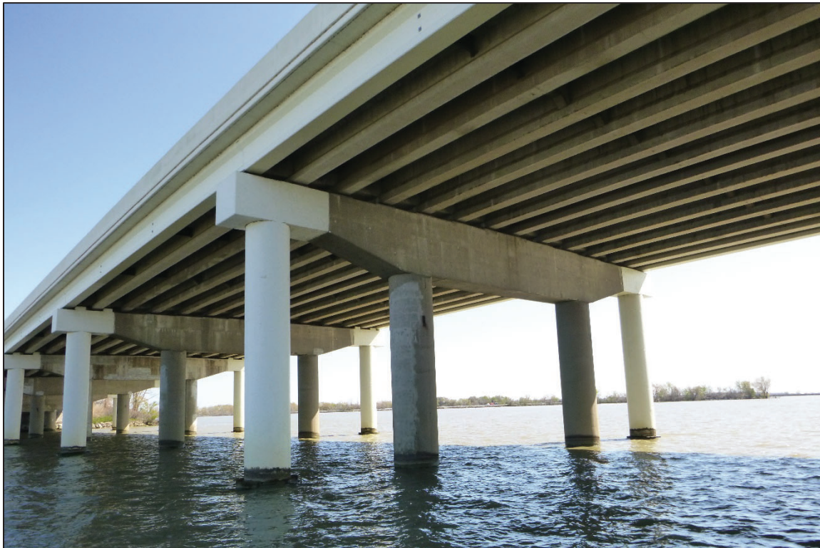
Photograph No. 20: View of the South Face of Bent 6, Looking Northeast.
