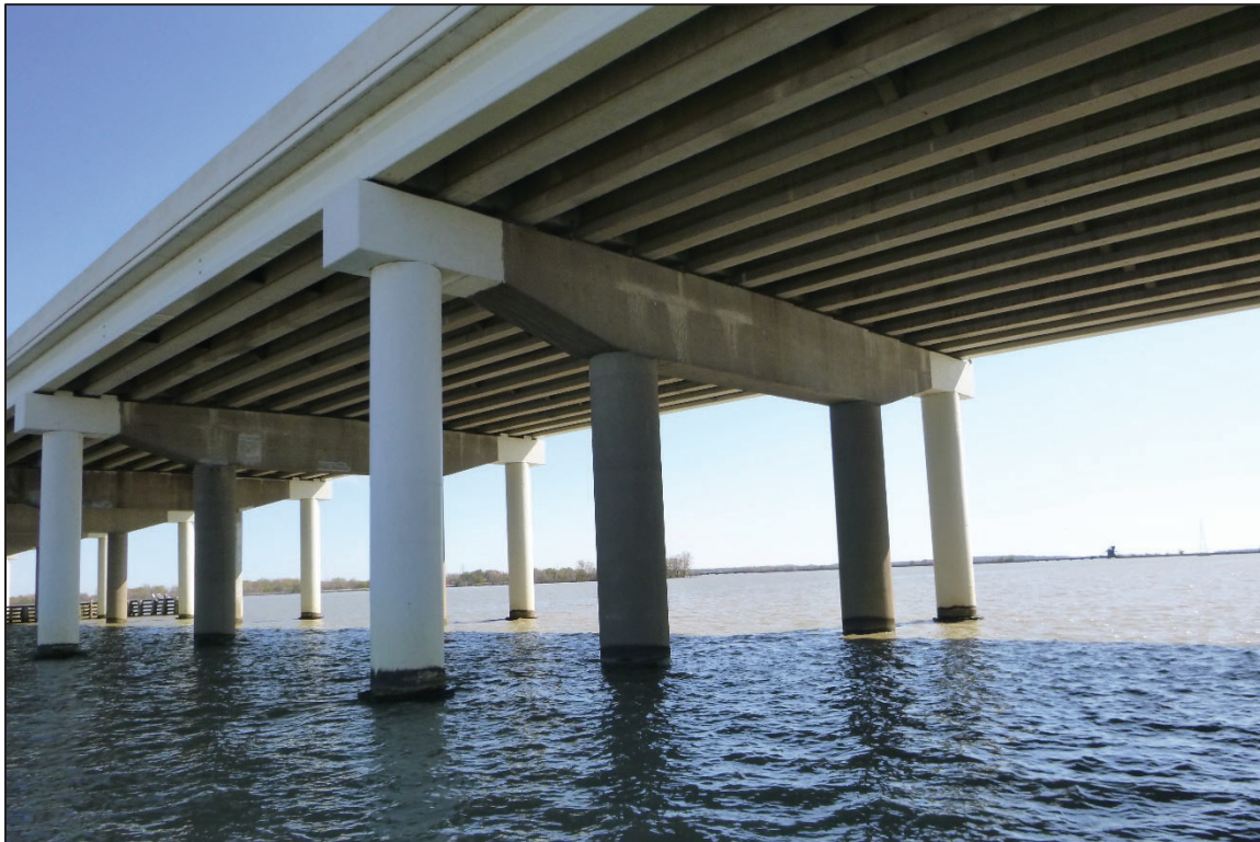
Photograph No. 40: View of the South Face of Bent 16, Looking Northeast.
