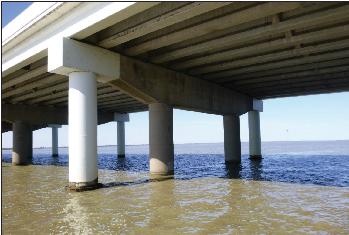
Photograph No. 11: View of the North Face of Bent 2, Looking Southwest.
