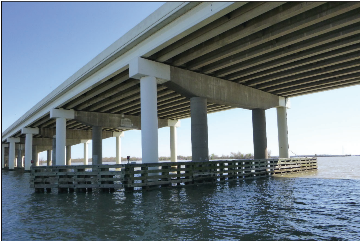
Photograph No. 30: View of the South Face of Bent 11, Looking Northeast.
