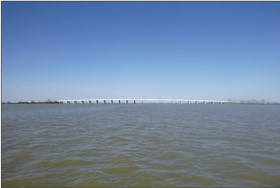
Photograph No. 1: Overall View of Structure No. 6200788 (OTT-2-2839), Looking West.
