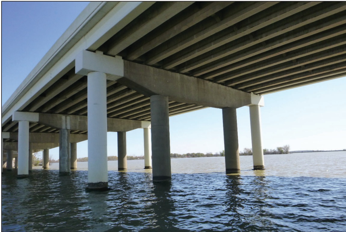
Photograph No. 24: View of the South Face of Bent 8, Looking Northeast.
