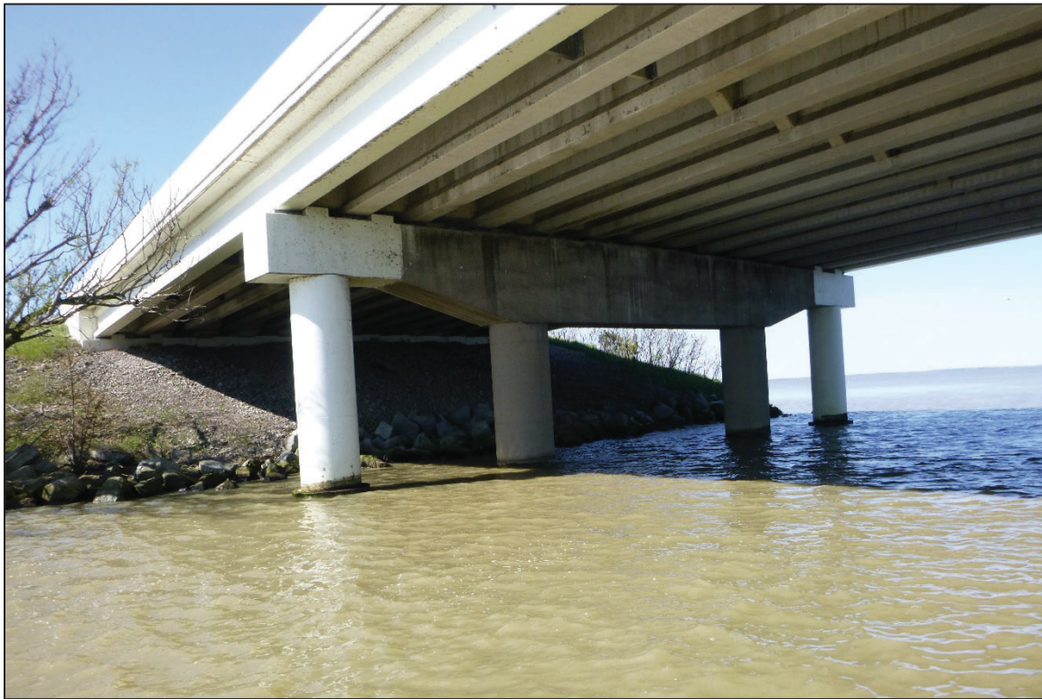
Photograph No. 51: View of the North Face of Bent 22, Looking Southwest.
