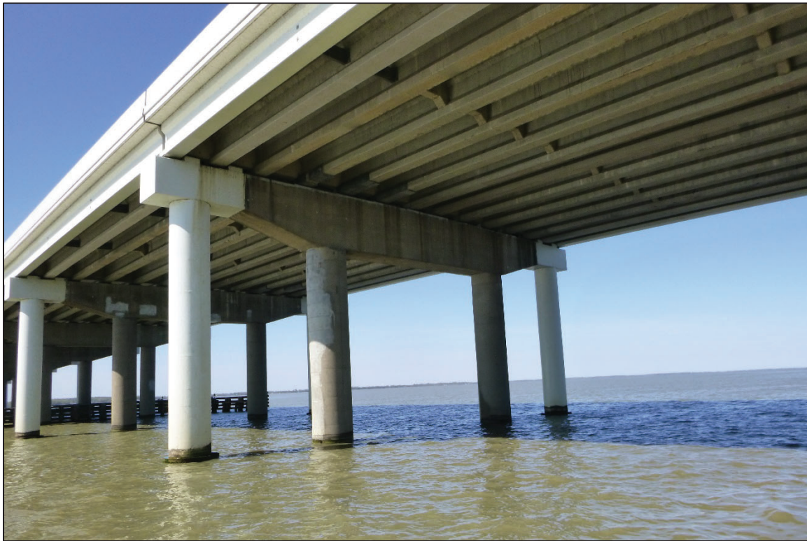
Photograph No. 25: View of the North Face of Bent 9, Looking Southwest.
