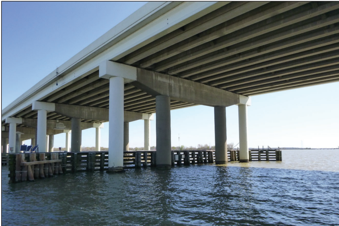
Photograph No. 32: View of the South Face of Bent 12, Looking Northeast.
