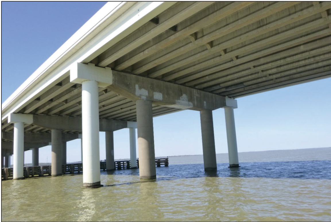
Photograph No. 27: View of the North Face of Bent 10, Looking Southwest.
