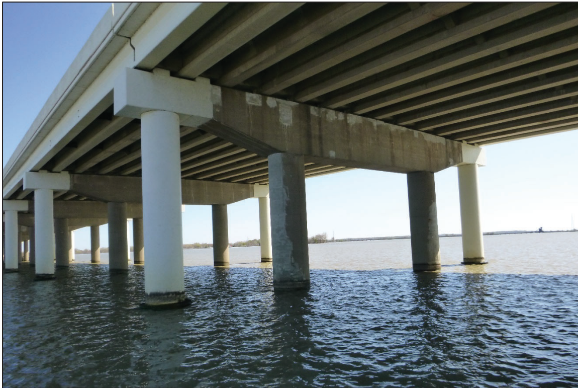
Photograph No. 46: View of the South Face of Bent 19, Looking Northeast.
