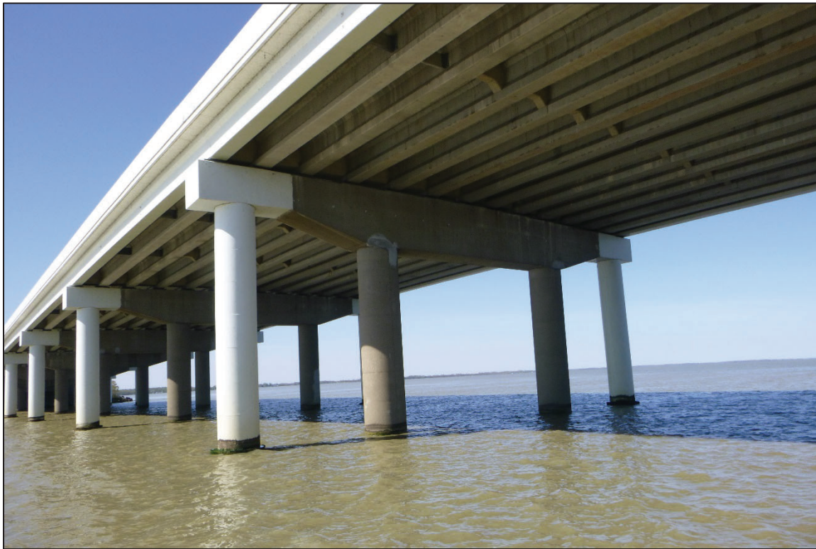
Photograph No. 39: View of the North Face of Bent 16, Looking Southwest.
