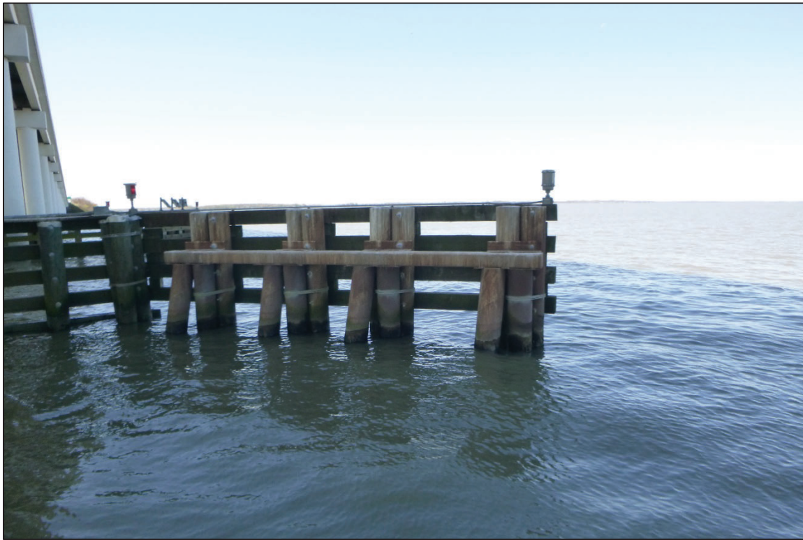
Photograph No. 55: View of the Steel Upstream Fender System, Looking Southwest.
