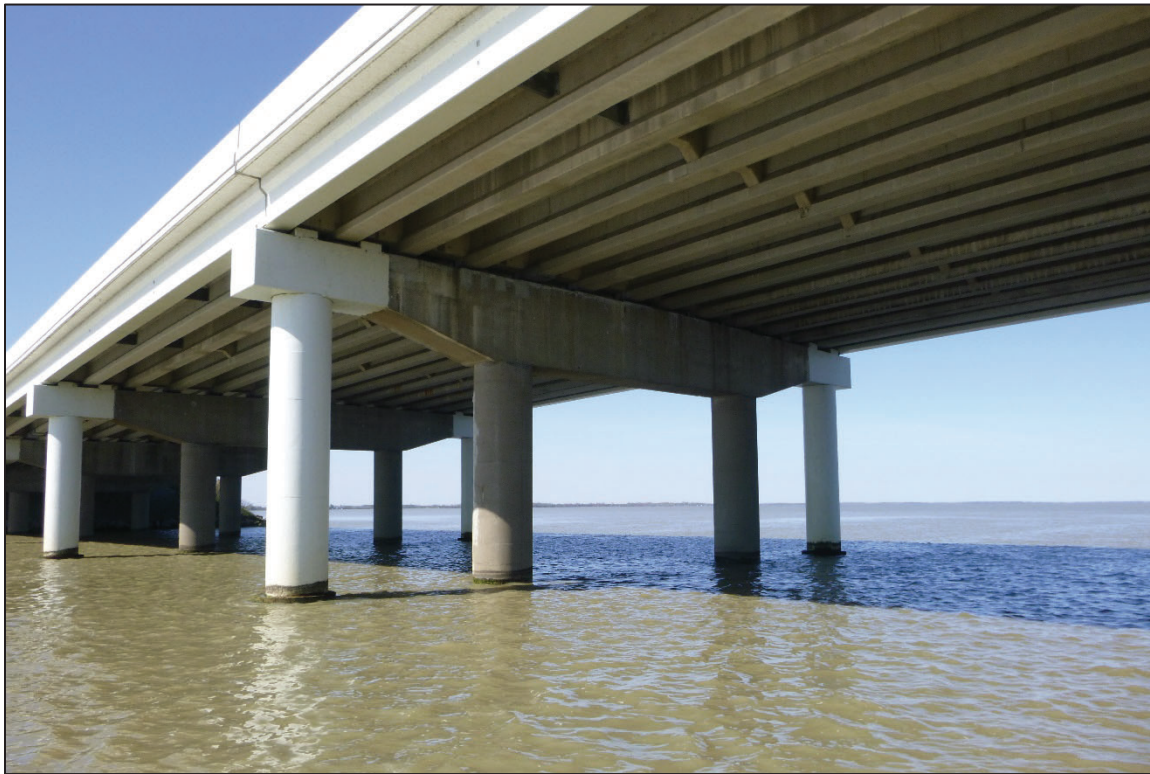
Photograph No. 45: View of the North Face of Bent 19, Looking Southwest.
