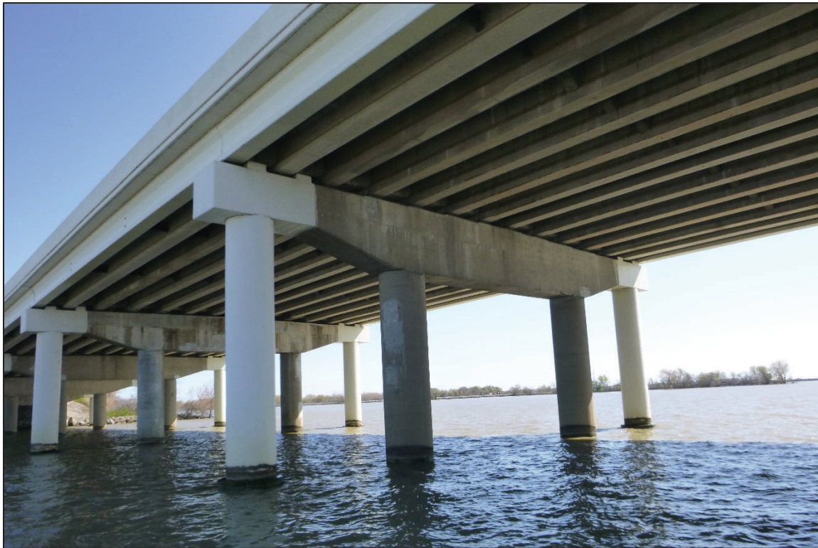
Photograph No. 18: View of the South Face of Bent 5, Looking Northeast.
