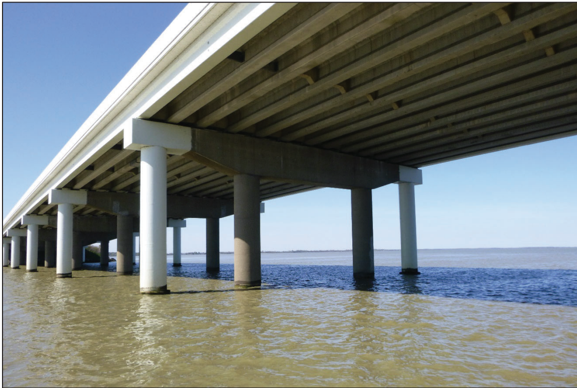
Photograph No. 41: View of the North Face of Bent 17, Looking Southwest.
