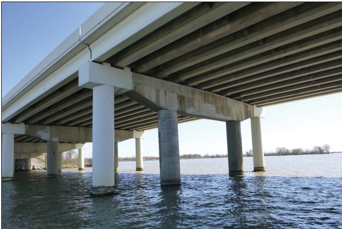
Photograph No. 16: View of the South Face of Bent 4, Looking Northeast.
