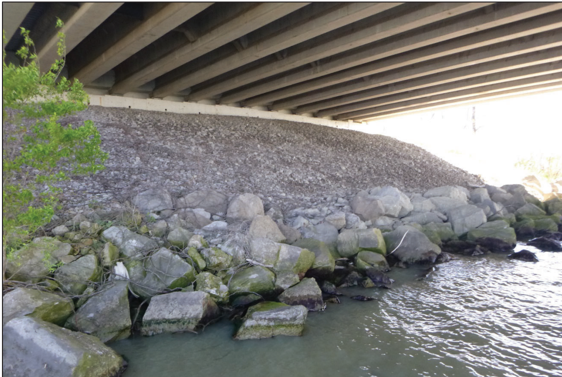
Photograph No. 4: View of the North Embankment at the Structure, Looking Northeast.
