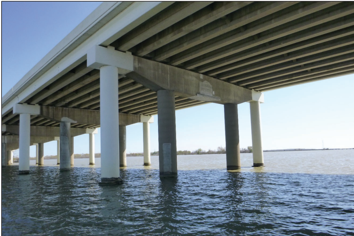
Photograph No. 28: View of the South Face of Bent 10, Looking Northeast.
