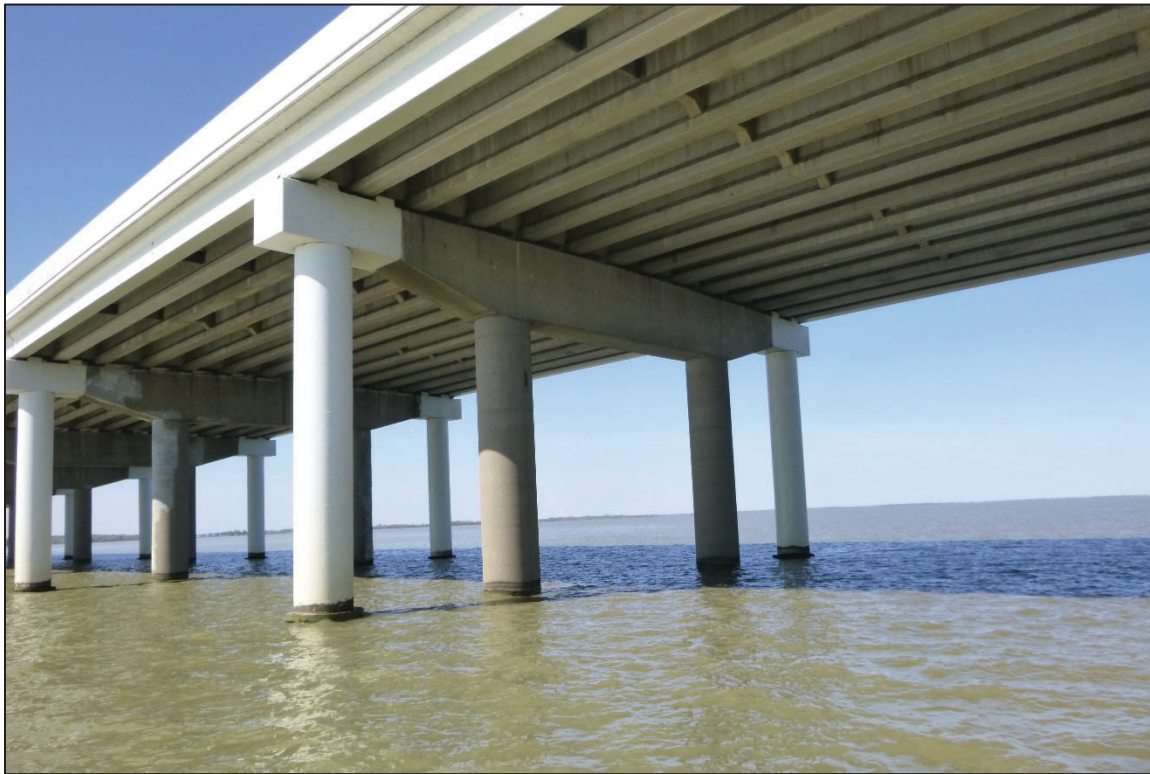
Photograph No. 33: View of the North Face of Bent 13, Looking Southwest.
