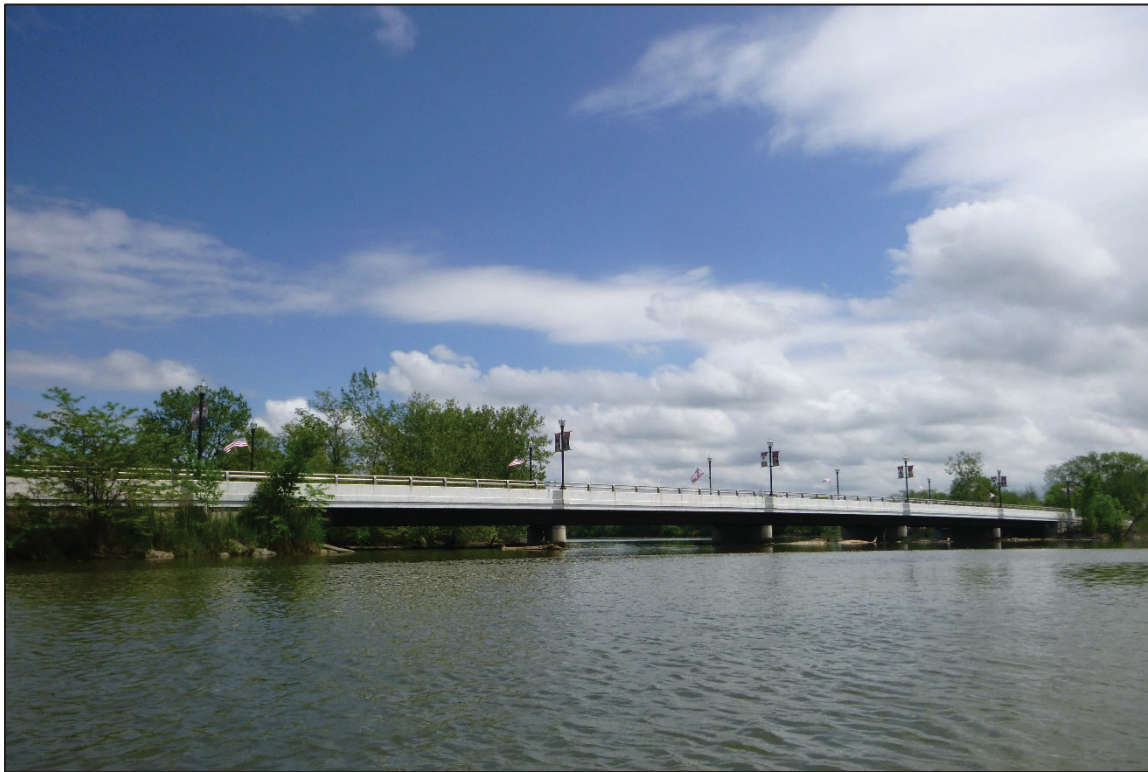
Photograph No. 1: Overall View of Structure No. 6200885 (OTT-19-0323), Looking Southeast.
