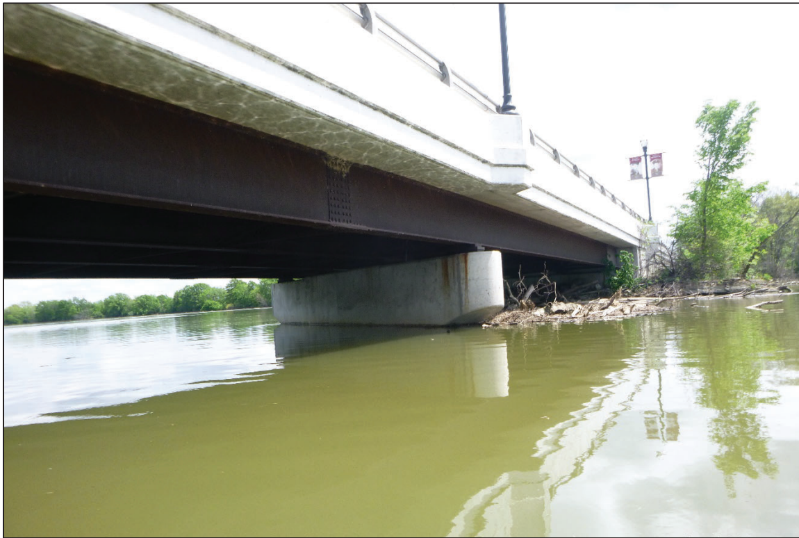
Photograph No. 9: View of the North Face of Pier 1, Looking Southeast.
