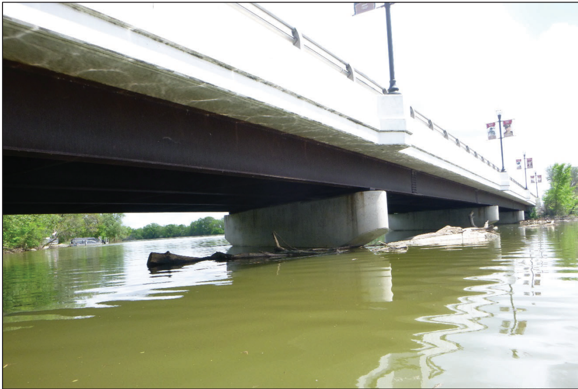
Photograph No. 13: View of the North Face of Pier 3, Looking Southeast.
