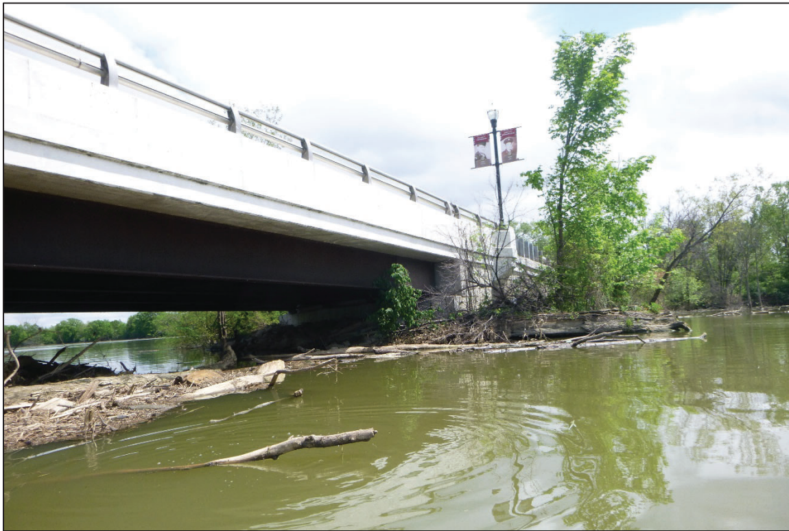
Photograph No. 7: View of the South Embankment at the Structure, Looking Southeast.
