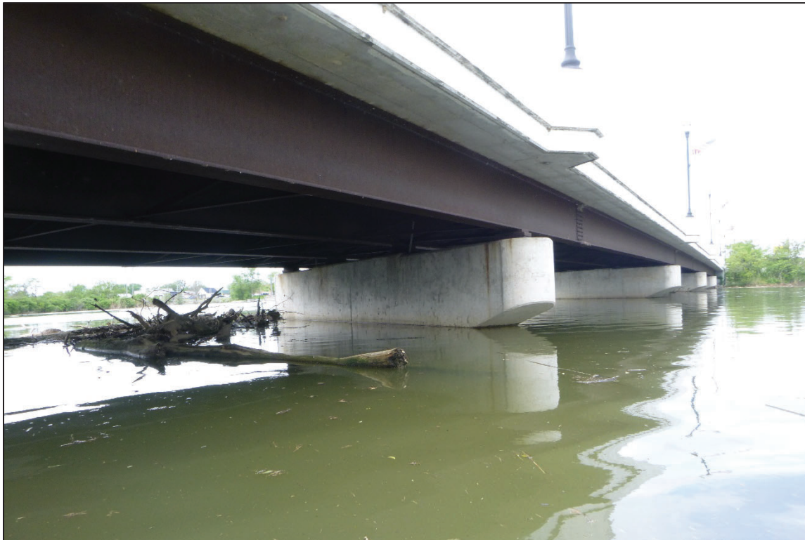
Photograph No. 10: View of the South Face of Pier 1, Looking Northwest.
