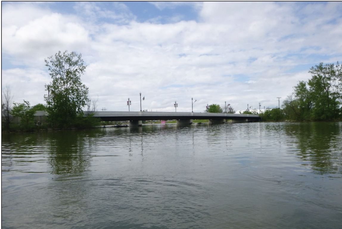
Photograph No. 2: Overall View of Structure No. 6200885 (OTT-19-0323), Looking Northwest.
