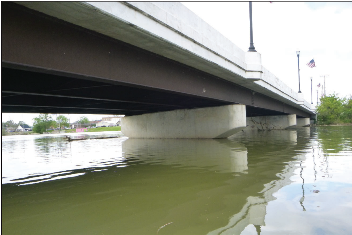
Photograph No. 12: View of the South Face of Pier 2, Looking Northwest.
