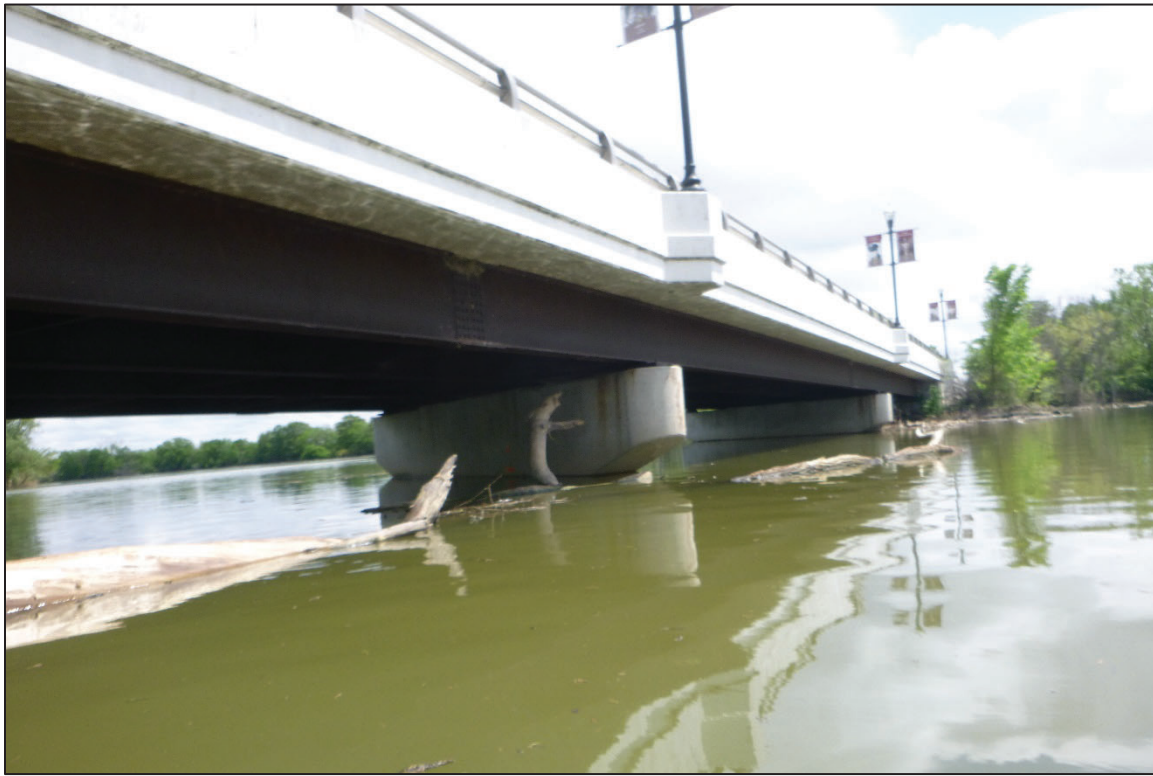
Photograph No. 11: View of the North Face of Pier 2, Looking Southeast.
