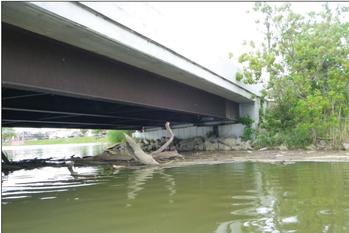
Photograph No. 4: View of the North Embankment at the Structure, Looking Northwest.
