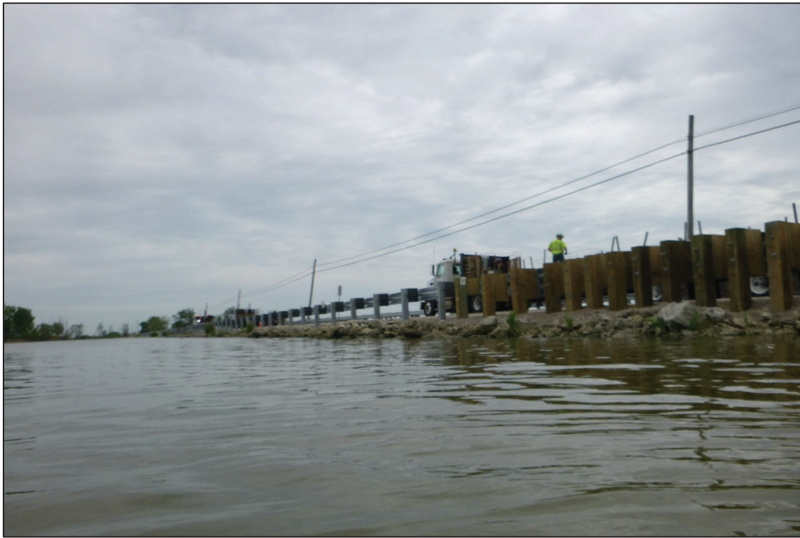
Photograph No. 3: View of the North Embankment Upstream of the Structure, Looking Northeast.
