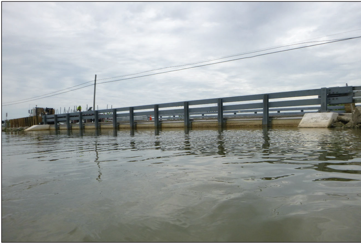
Photograph No. 1: Overall View of Structure No. 6200931 (OTT-19-0811), Looking Northeast.
