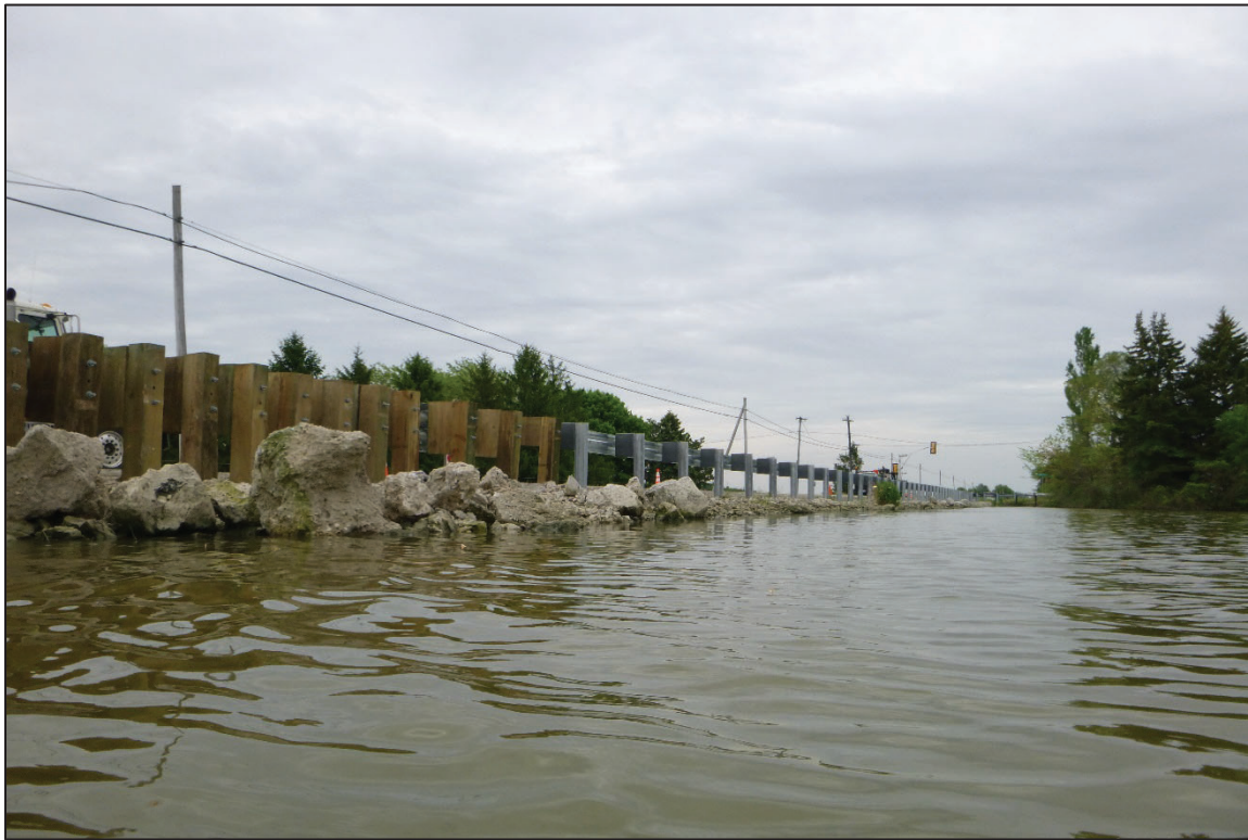
Photograph No. 5: View of the South Embankment Upstream of the Structure, Looking Southeast.
