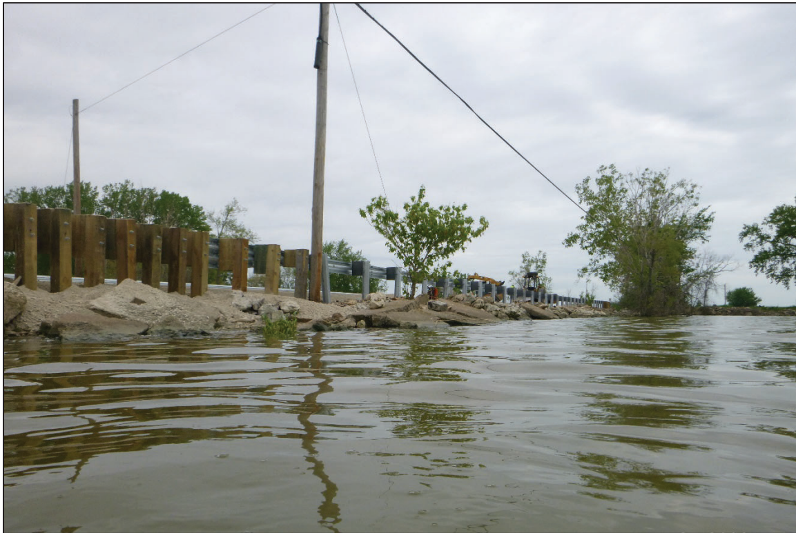
Photograph No. 4: View of the North Embankment Downstream of the Structure, Looking Northwest.
