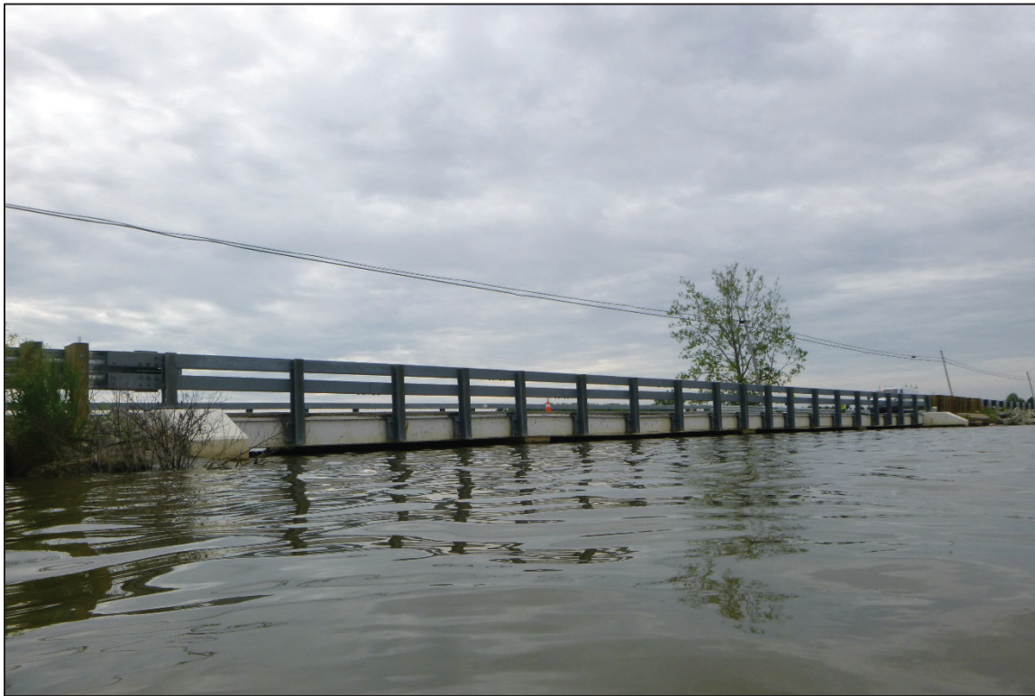
Photograph No. 1: Overall View of Structure No. 6200966 (OTT-19-0833), Looking Southeast.
