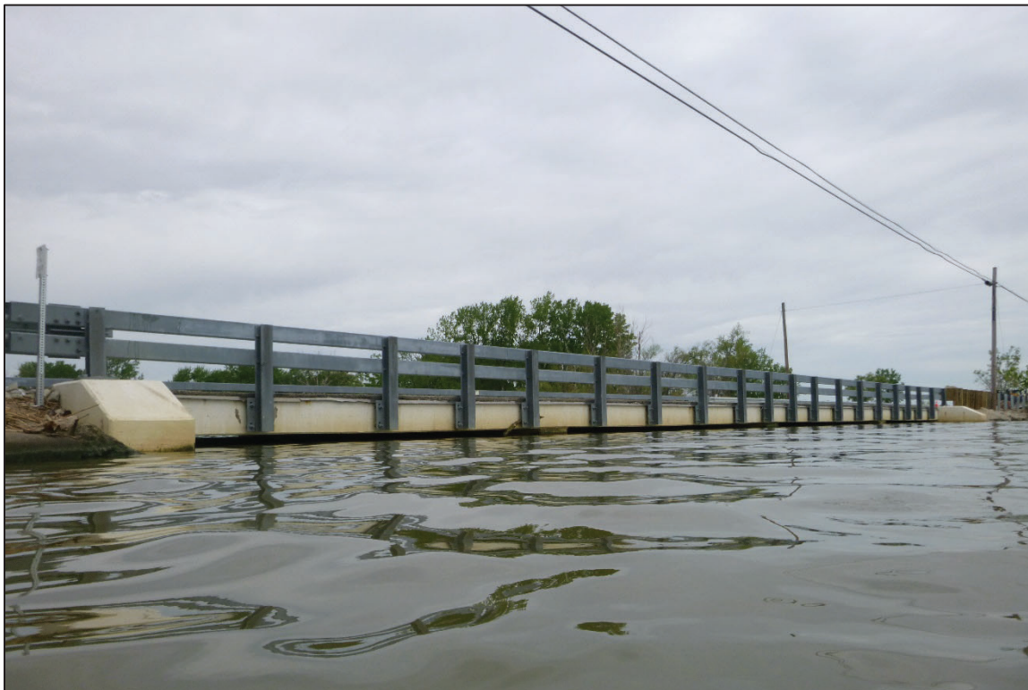
Photograph No. 2: Overall View of Structure No. 6200966 (OTT-19-0833), Looking Northwest.
