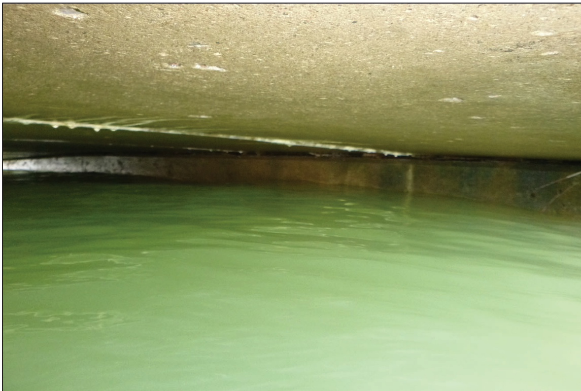
Photograph No. 10: View of Abutment 2, Looking Northwest.
