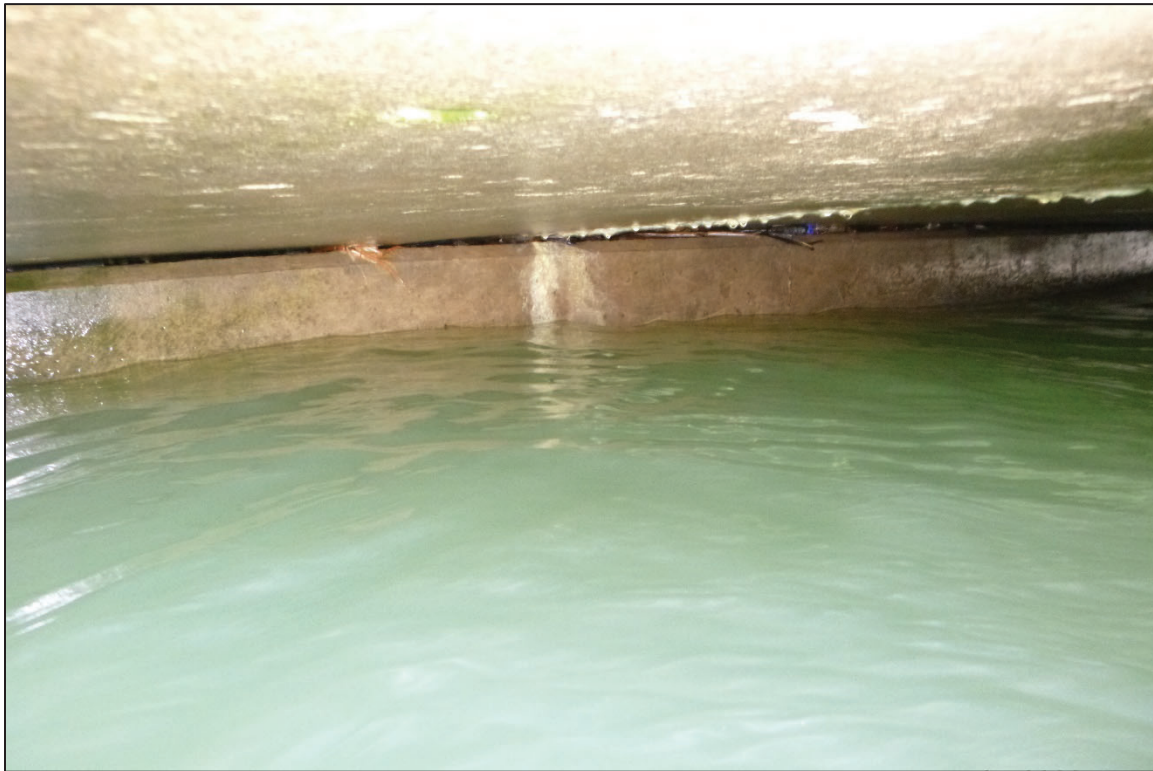
Photograph No. 8: View of Abutment 1, Looking South.
