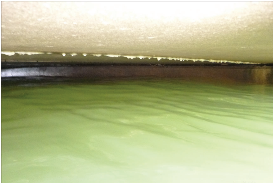
Photograph No. 7: View of Abutment 1, Looking Southeast.
