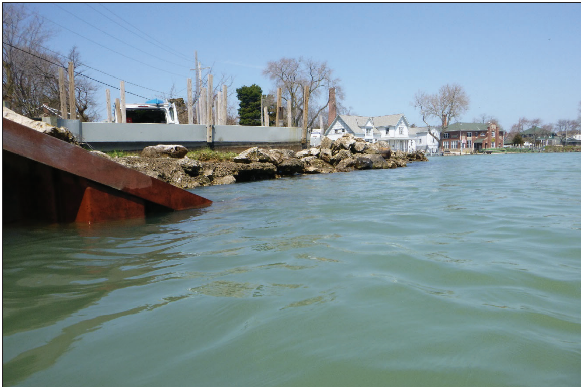
Photograph No. 4: View of the North Embankment Downstream of the Structure, Looking North.
