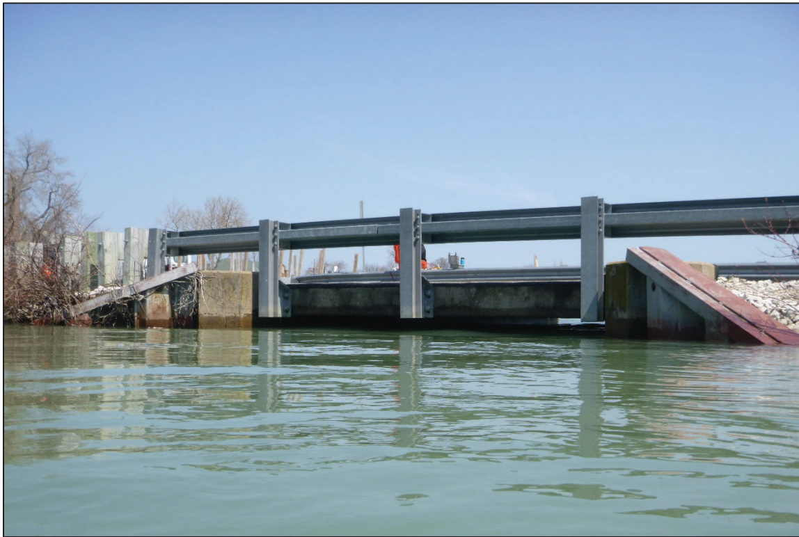
Photograph No. 1: Overall View of Structure No. 6201776 (OTT-357-0016), Looking Northeast.
