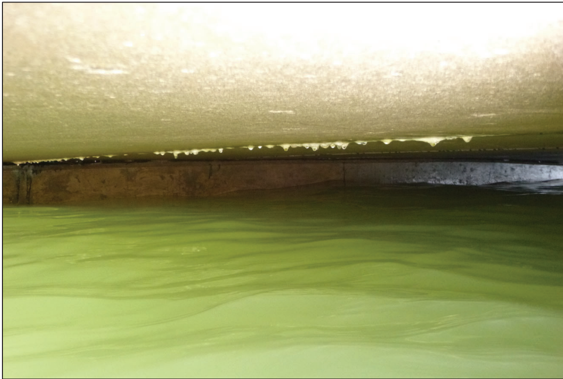
Photograph No. 9: View of Abutment 2, Looking North.
