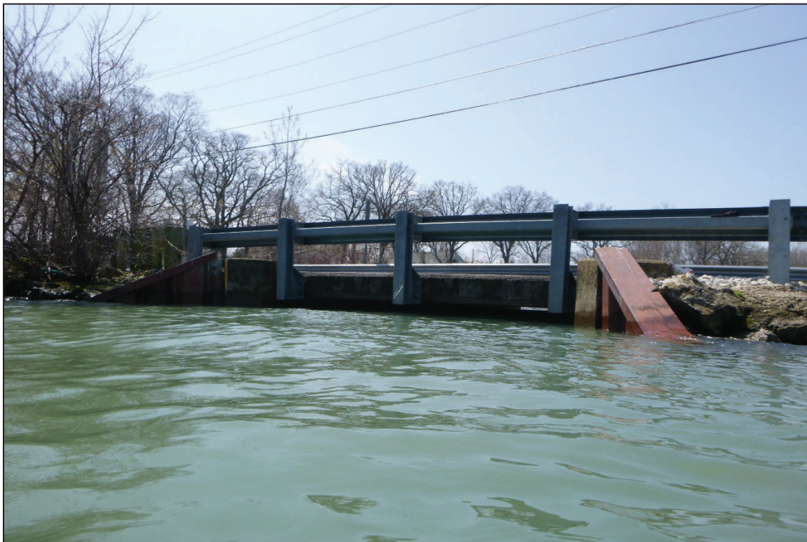
Photograph No. 2: Overall View of Structure No. 6201776 (OTT-357-0016), Looking Southwest.
