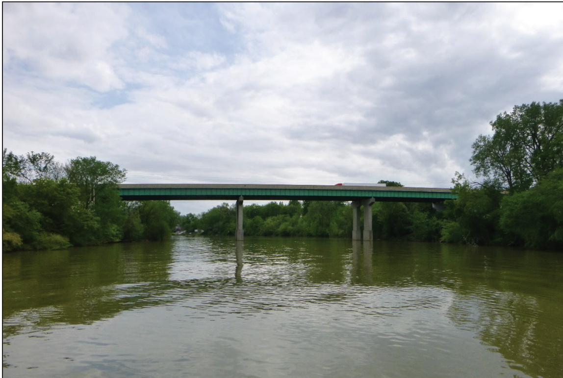
Photograph No. 2: Overall View of Structure No. 7200579 (SAN-6-1751), Looking South.
