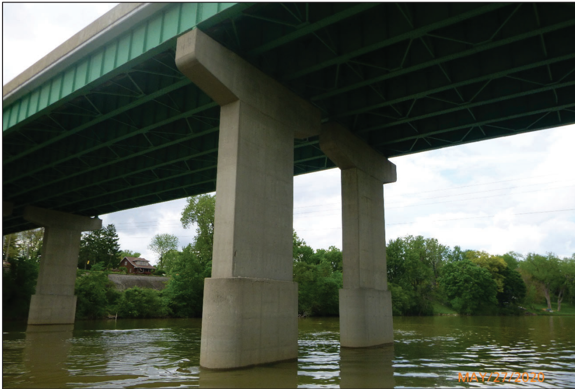
Photograph No. 13: View of the East Face of Pier 5, Looking Northwest.
