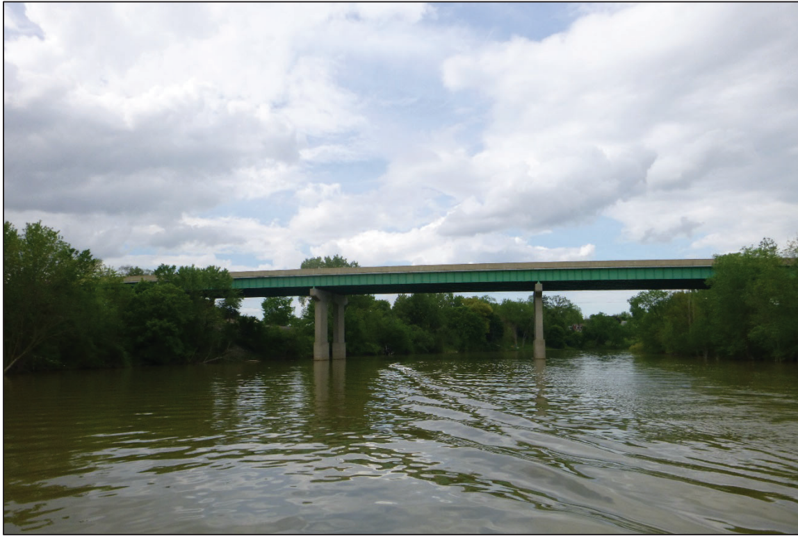
Photograph No. 1: Overall View of Structure No. 7200579 (SAN-6-1751), Looking North.
