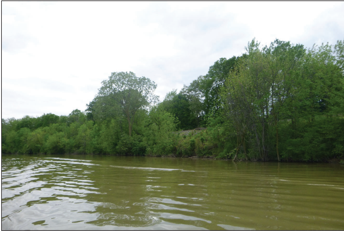
Photograph No. 3: View of the West Embankment Upstream of the Structure, Looking Southwest.
