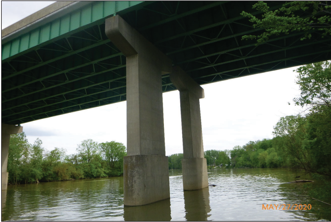
Photograph No. 9: View of the West Face of Pier 4, Looking Southeast.
