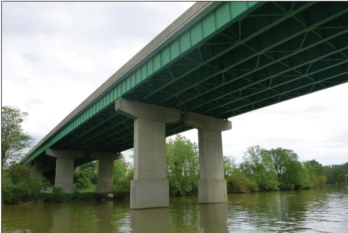
Photograph No. 12: View of the West Face of Pier 5, Looking Southeast.
