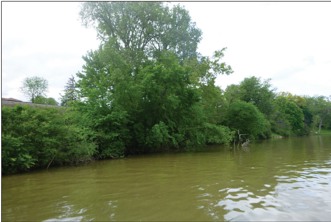
Photograph No. 5: View of the West Embankment Downstream of the Structure, Looking Northwest.
