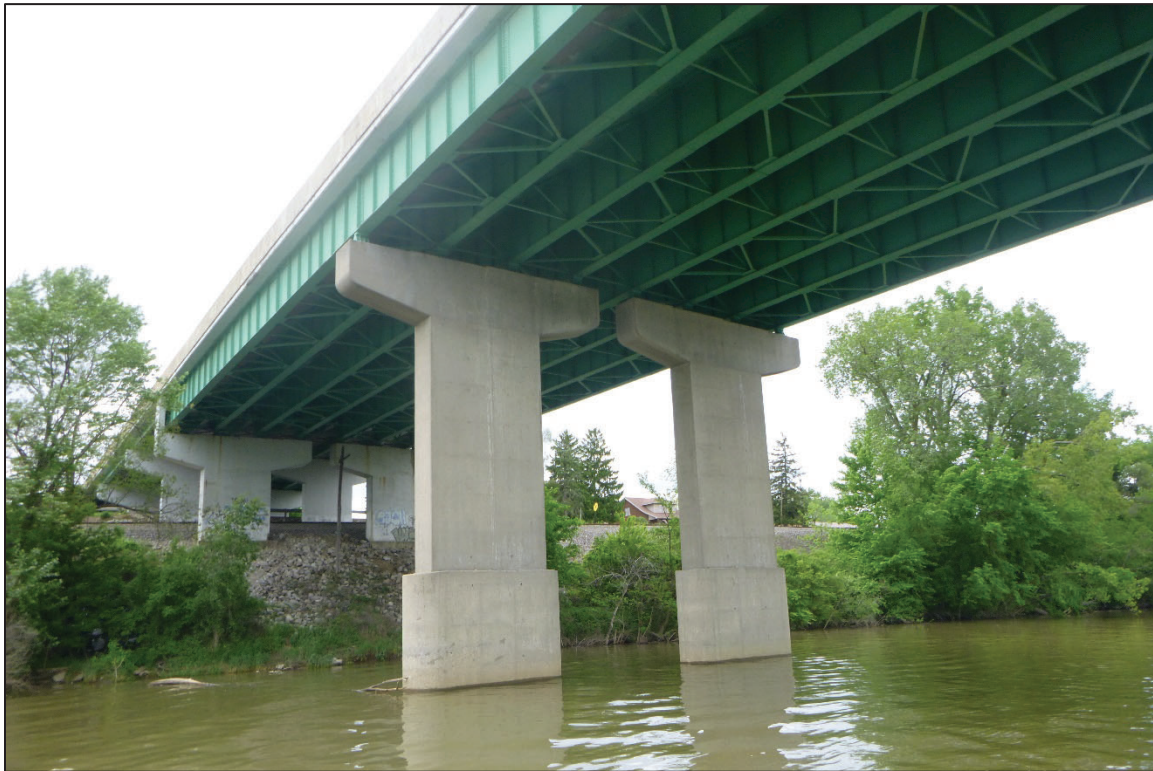
Photograph No. 10: View of the East Face of Pier 4, Looking Northwest.
