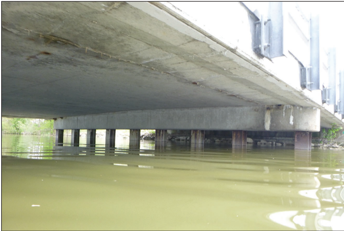
Photograph No. 9: View of the North Face of Bent 1, Looking Southeast.
