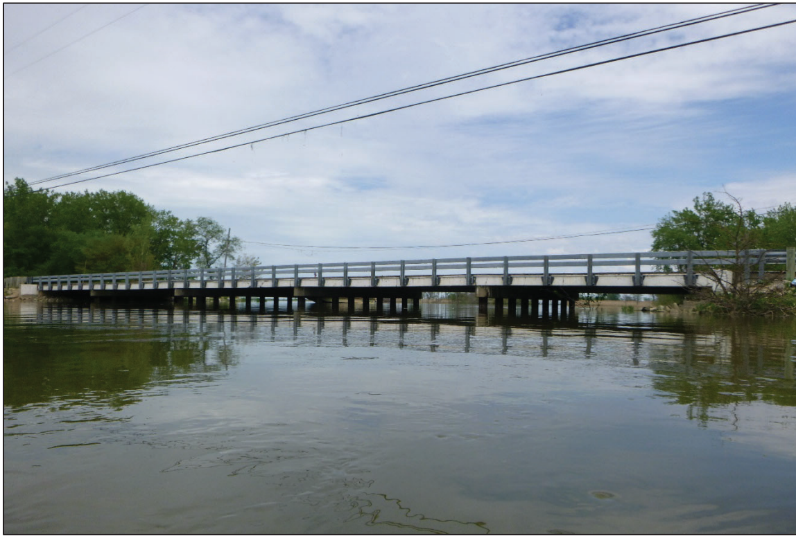
Photograph No. 1: Overall View of Structure No. 7202431 (SAN-5301745), Looking Southeast.
