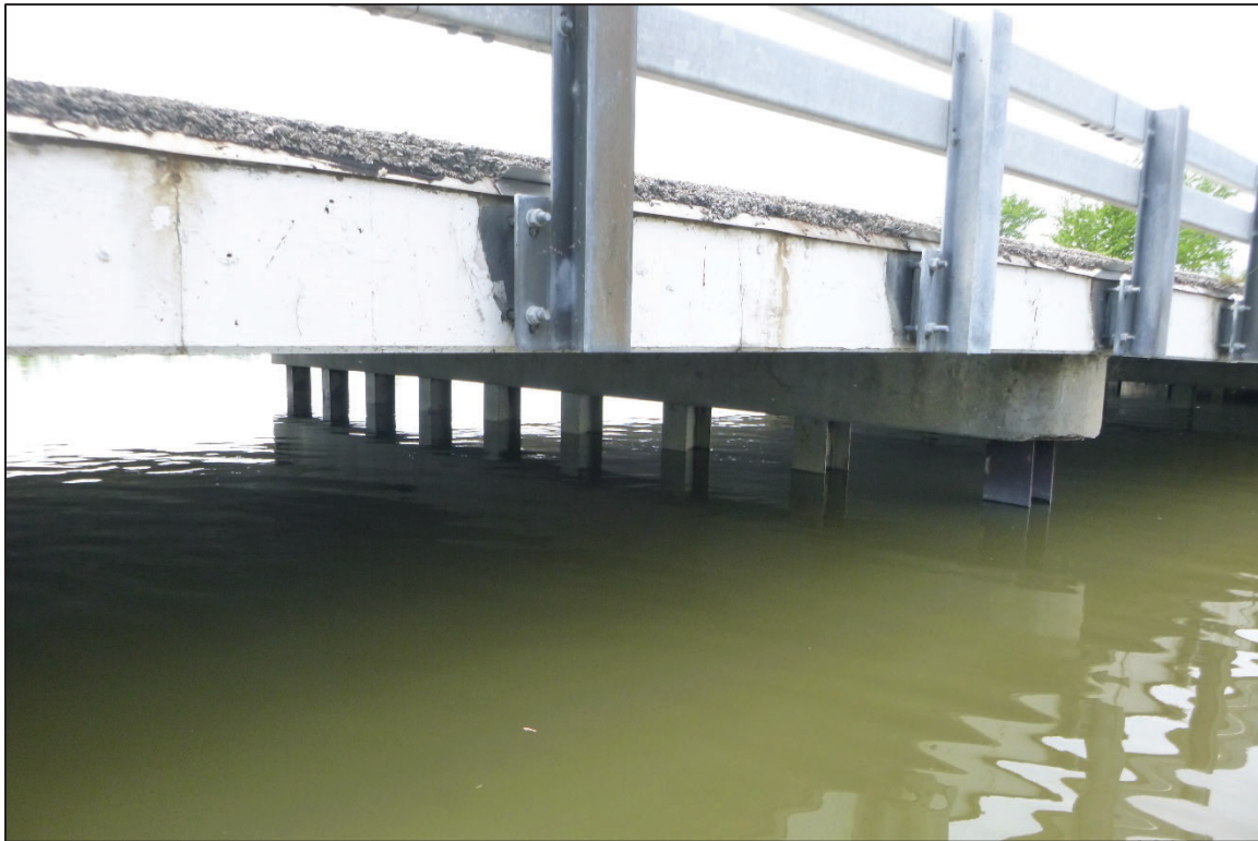
Photograph No. 12: View of the South Face of Bent 2, Looking Northwest.
