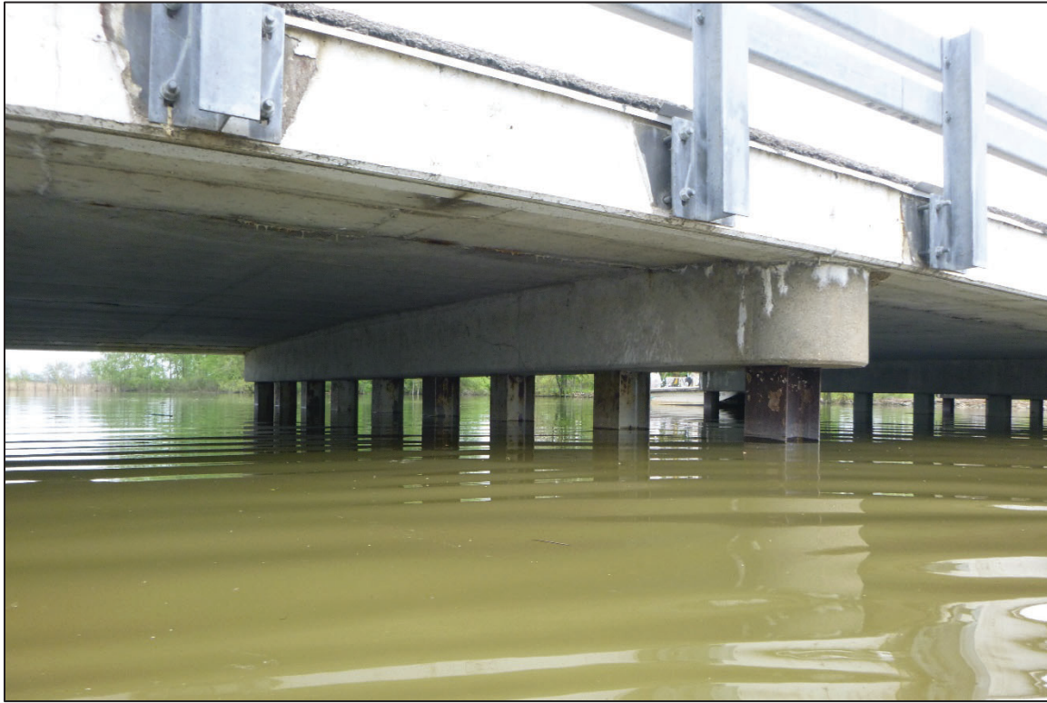
Photograph No. 15: View of the North Face of Bent 4, Looking Southeast.
