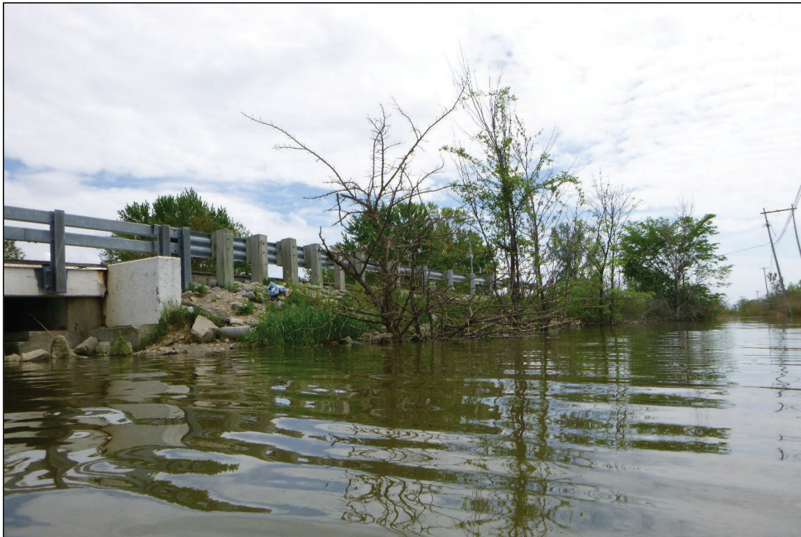
Photograph No. 6: View of the South Embankment Upstream of the Structure, Looking Southeast.
