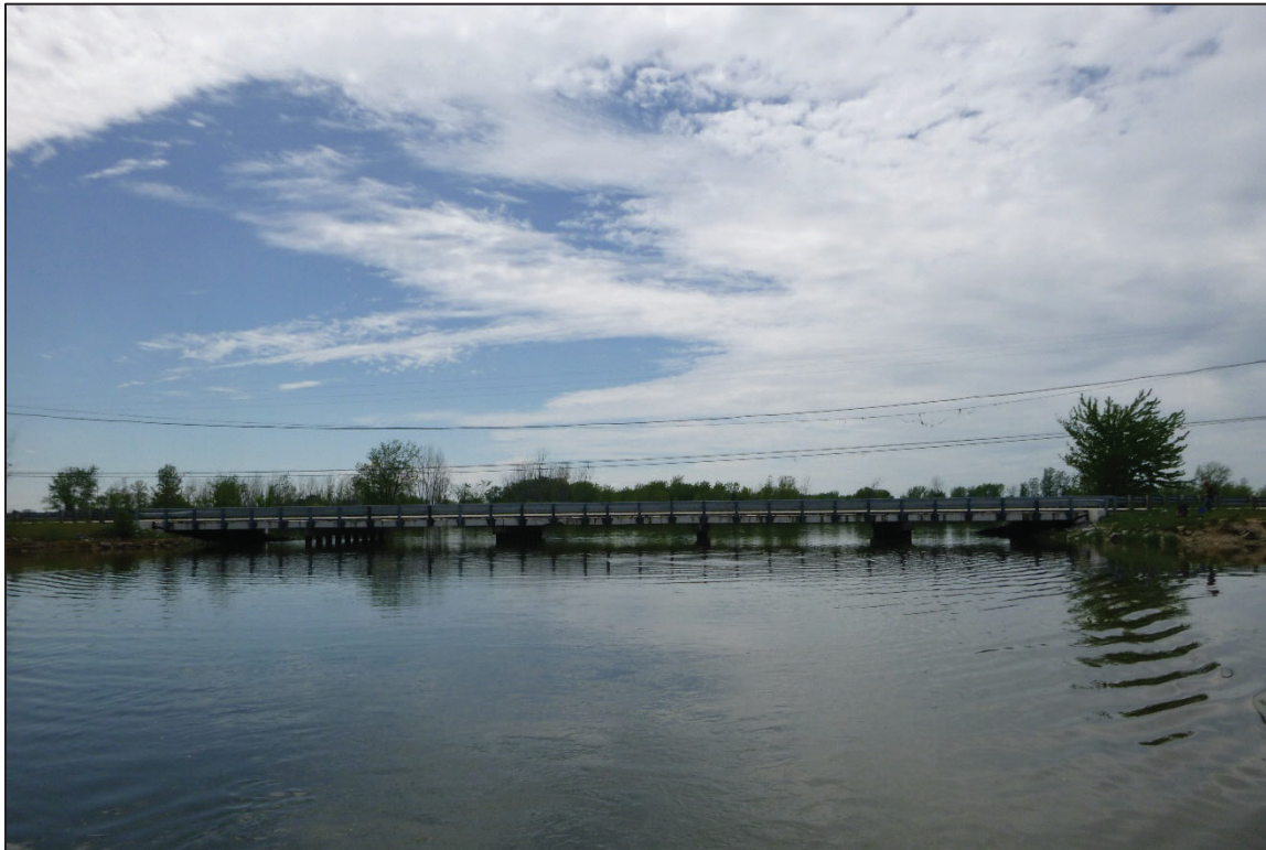
Photograph No. 2: Overall View of Structure No. 7202431 (SAN-53-1745), Looking West.
