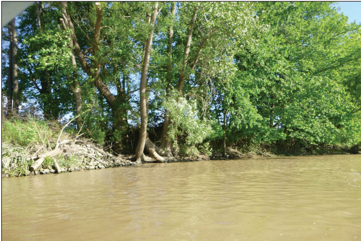
Photograph No. 6: View of the East Embankment Upstream of the Structure, Looking Southeast.
