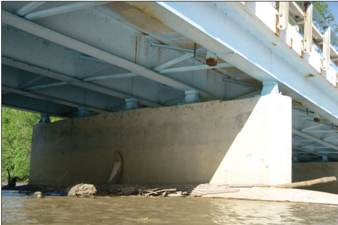
Photograph No. 14: View of the West Face of Pier 3, Looking Northeast.
