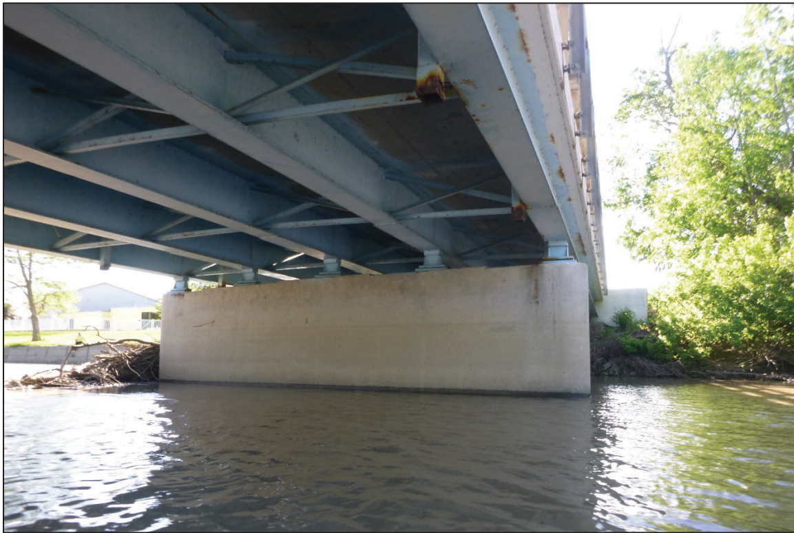
Photograph No. 9: View of the East Face of Pier 1, Looking Southwest.
