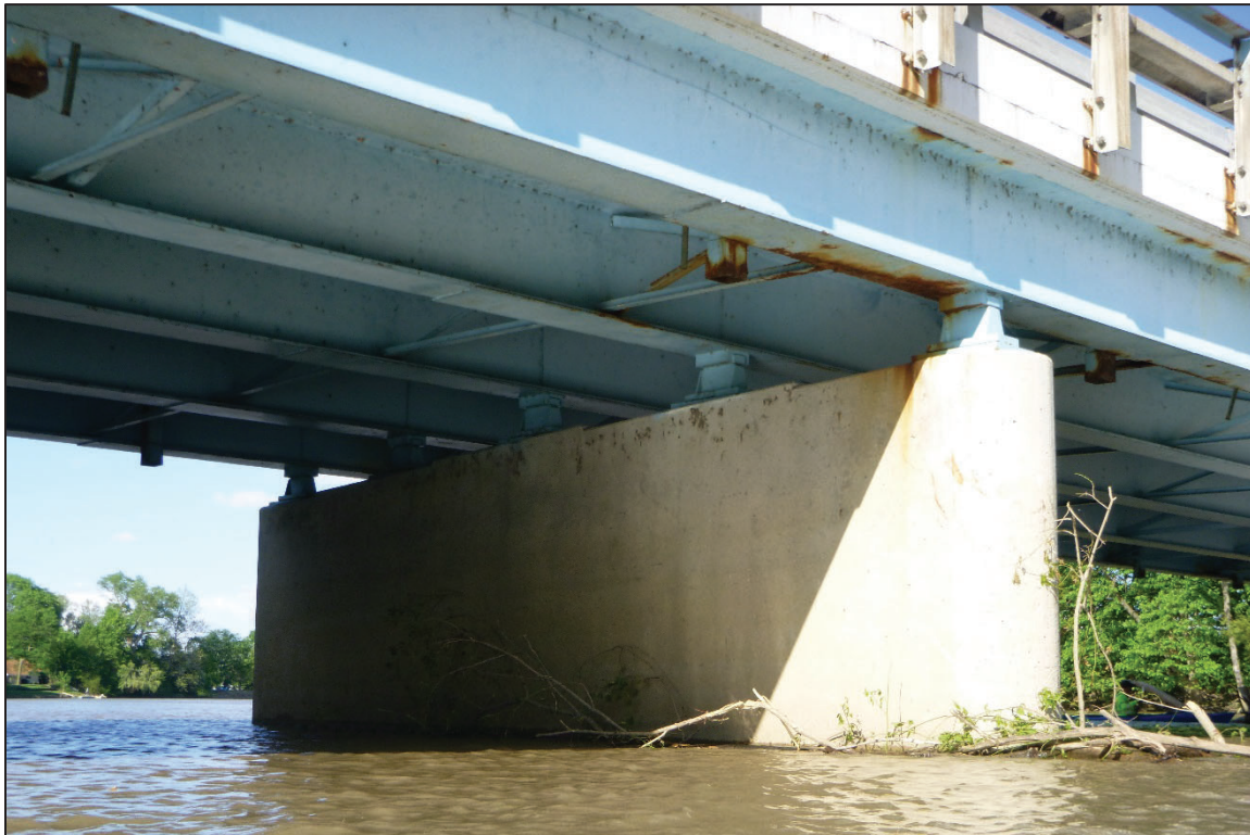
Photograph No. 12: View of the East Face of Pier 2, Looking Northeast.
