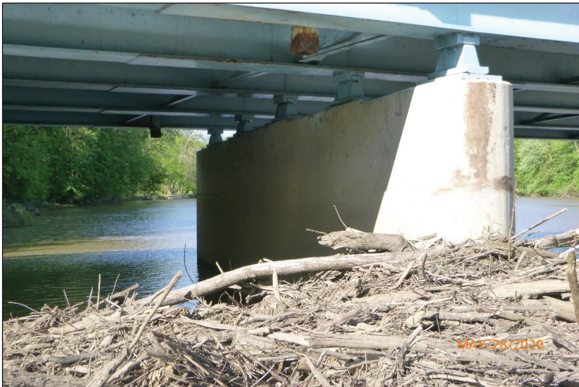
Photograph No. 10: View of the West Face of Pier 1, Looking Northeast.
