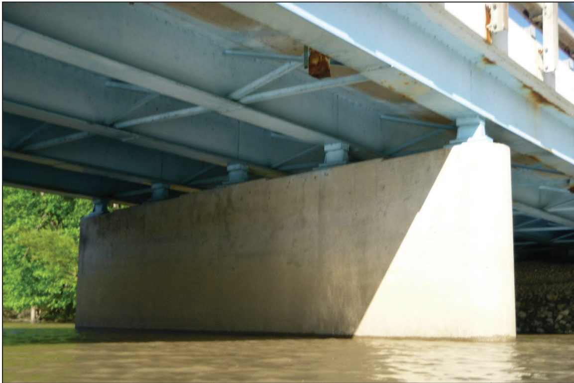
Photograph No. 16: View of the West Face of Pier 4, Looking Northeast.
