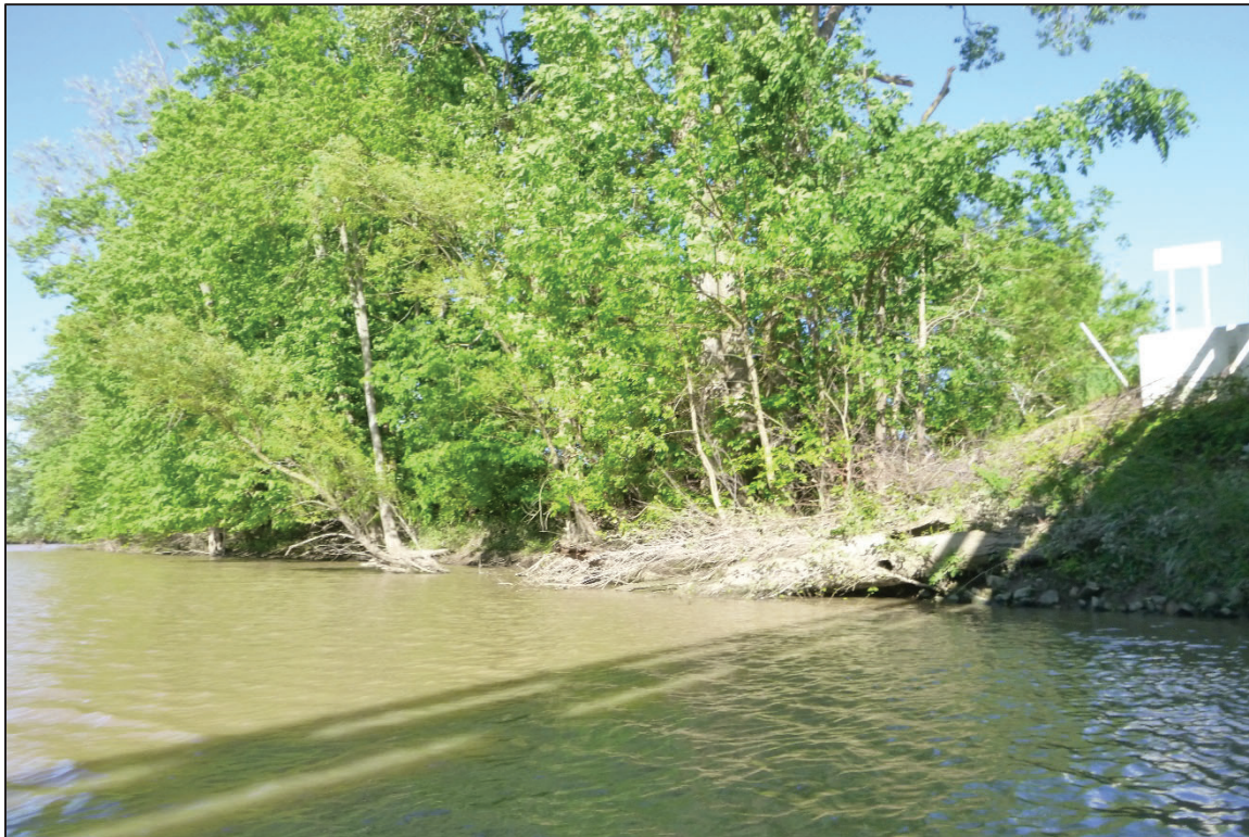
Photograph No. 8: View of the East Embankment Downstream of the Structure, Looking Northeast.
