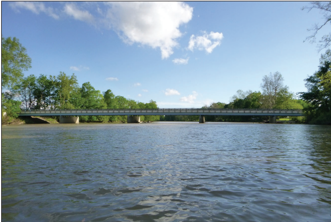
Photograph No. 2: Overall View of Structure No. 7402910 (SEN-224-1207), Looking South.
