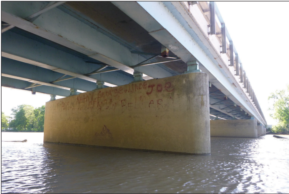
Photograph No. 15: View of the East Face of Pier 4, Looking Southwest.
