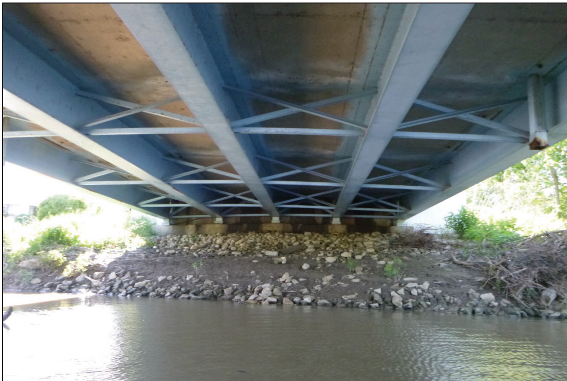
Photograph No. 4: View of the West Embankment at the Structure, Looking West.
