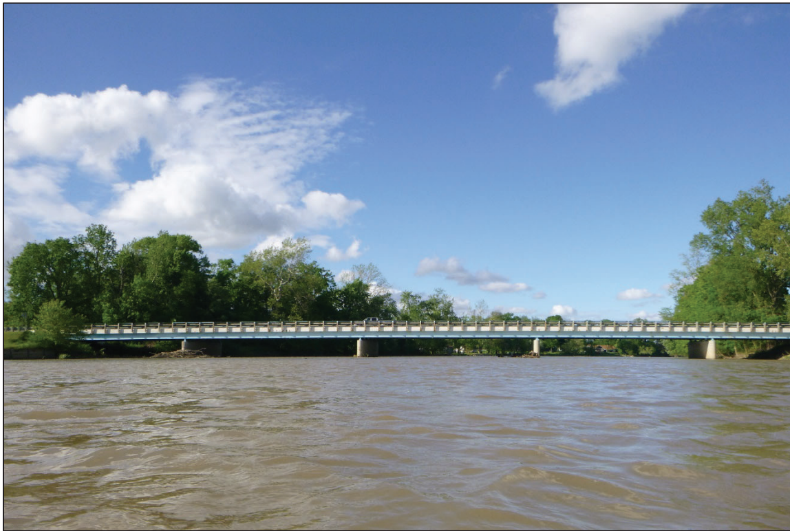
Photograph No. 1: Overall View of Structure No. 7402910 (SEN-224-1207), Looking North.
