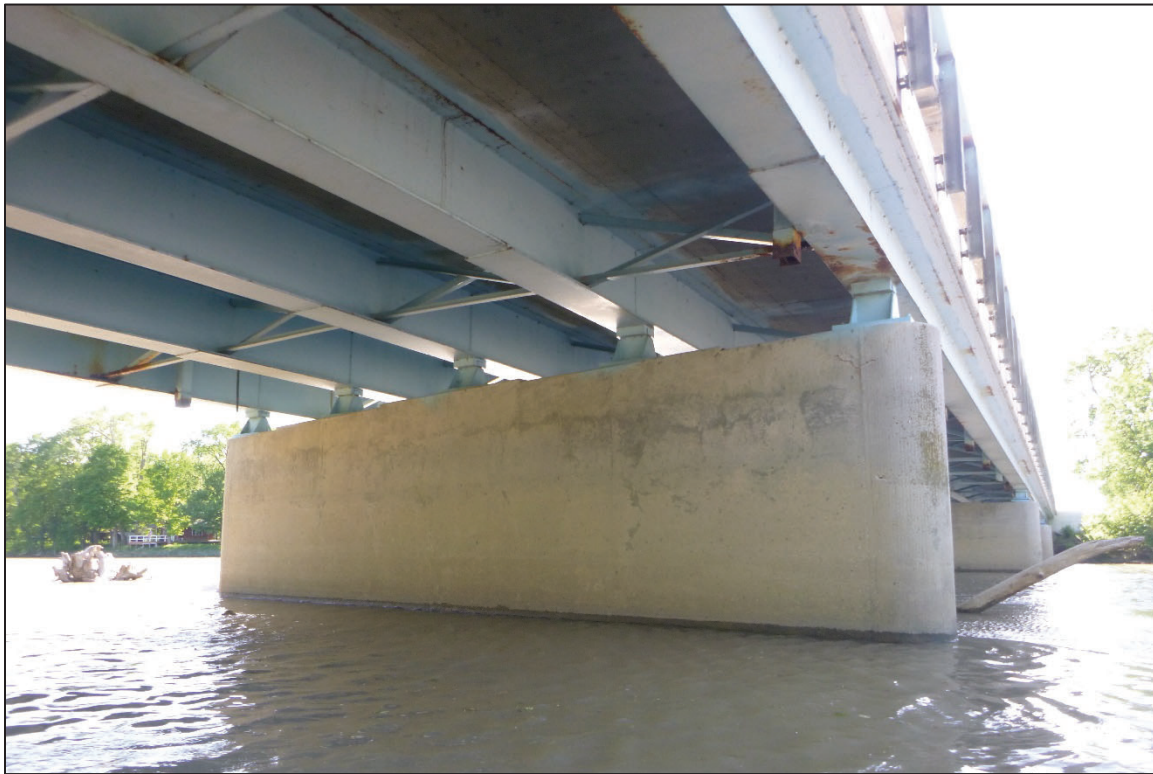
Photograph No. 13: View of the East Face of Pier 3, Looking Southwest.
