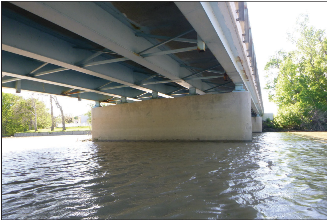
Photograph No. 11: View of the West Face of Pier 2, Looking Southwest.
