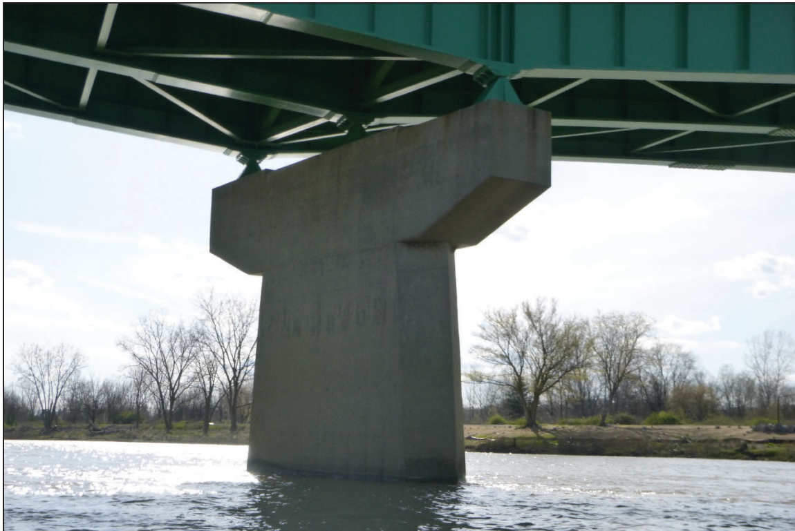
Photograph No. 14: View of the South Face of Pier 4, Looking Northwest.
