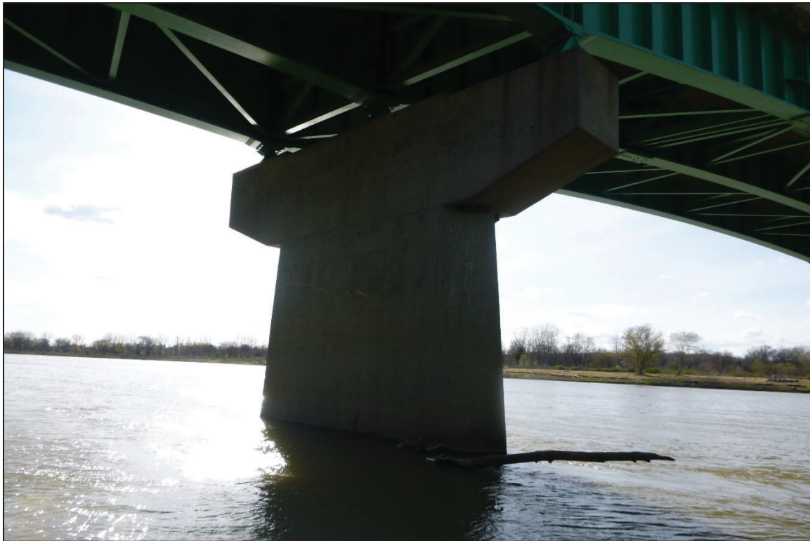
Photograph No. 10: View of the South Face of Pier 2, Looking Northwest.
