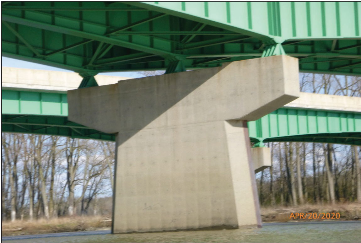
Photograph No. 13: View of the North Face of Pier 4, Looking Southeast.
