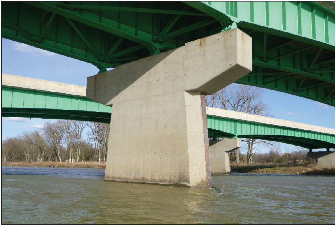
Photograph No. 11: View of the North Face of Pier 3, Looking Southeast.
