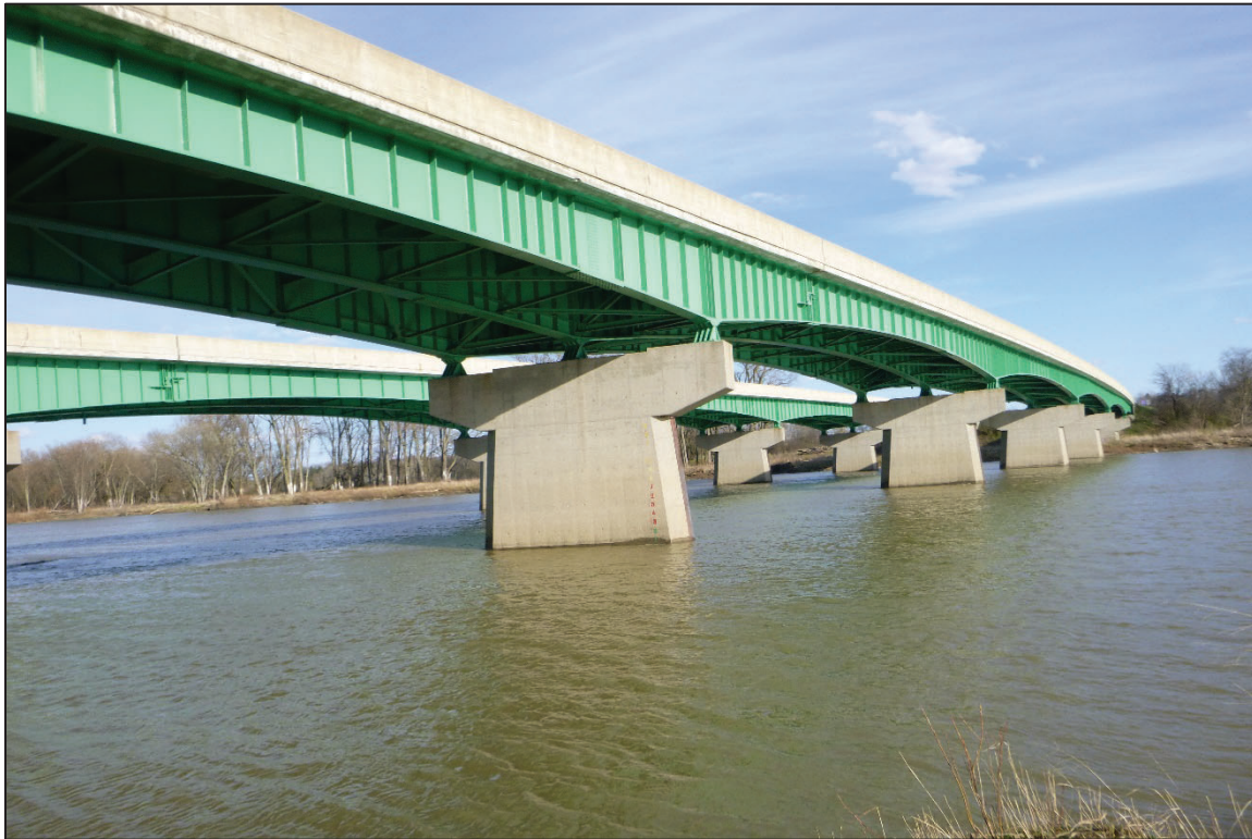
Photograph No. 2: Overall View of Structure No. 8706751 (WOO-475-0386L), Looking Southeast.
