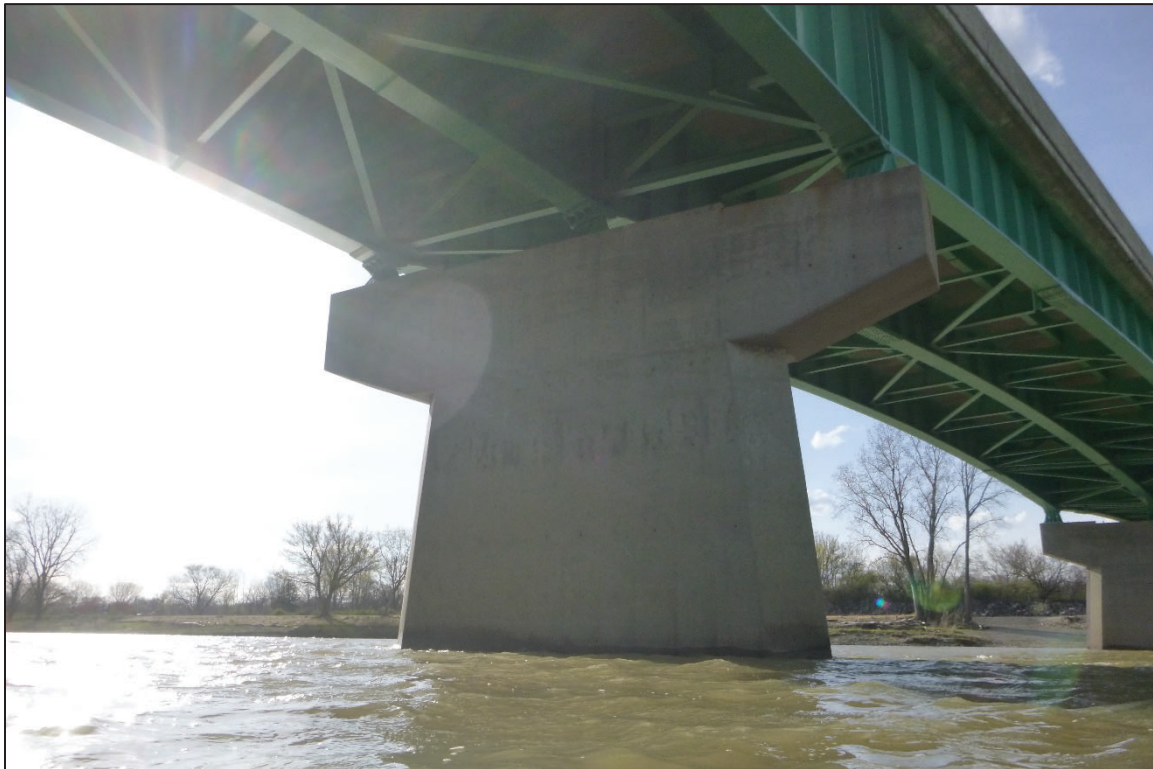
Photograph No. 12: View of the South Face of Pier 3, Looking Northwest.
