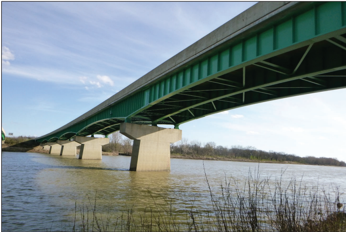
Photograph No. 1: Overall View of Structure No. 8706751 (WOO-475-0386L), Looking Southwest.
