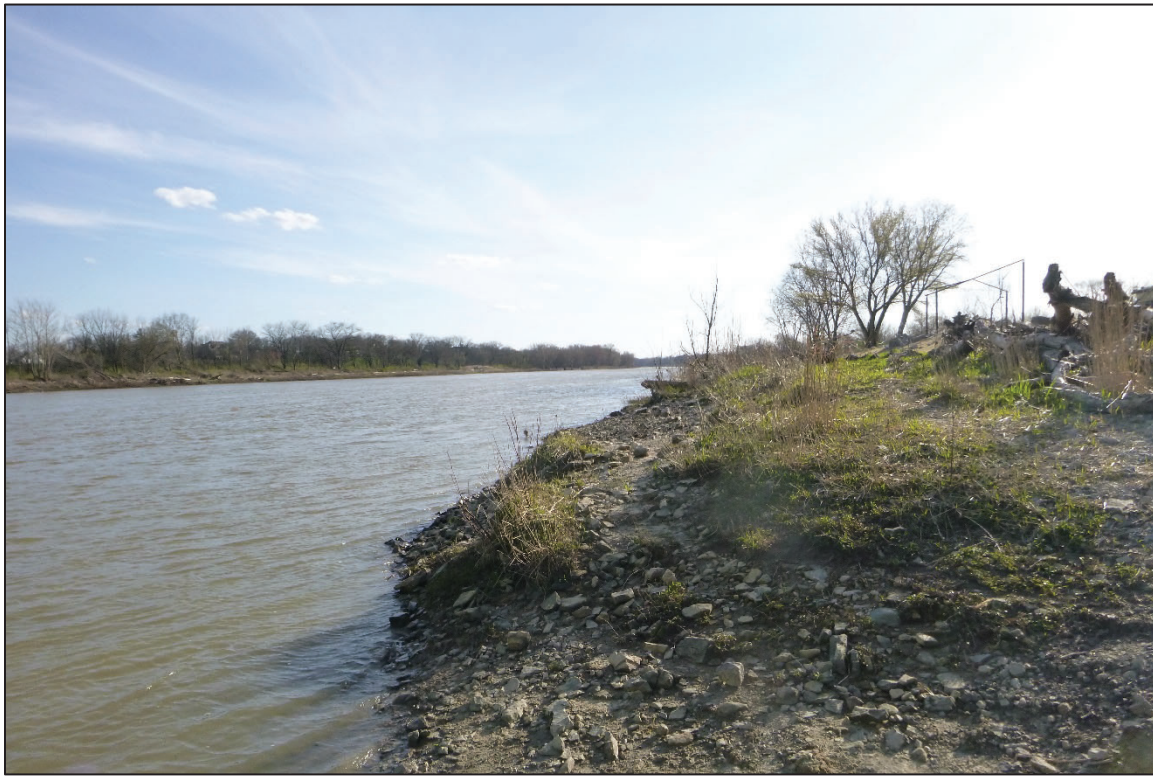
Photograph No. 3: View of the North Embankment Upstream of the Structure, Looking West.
