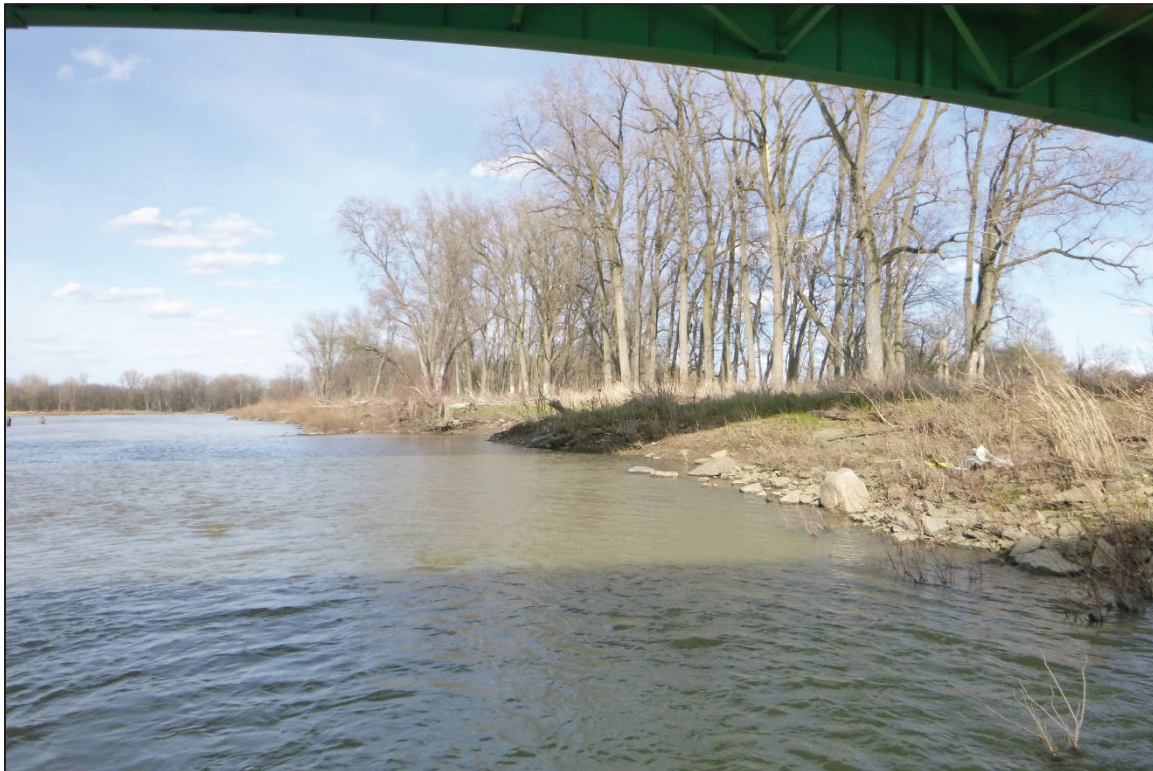
Photograph No. 8: View of the South Embankment Downstream of the Structure, Looking East.
