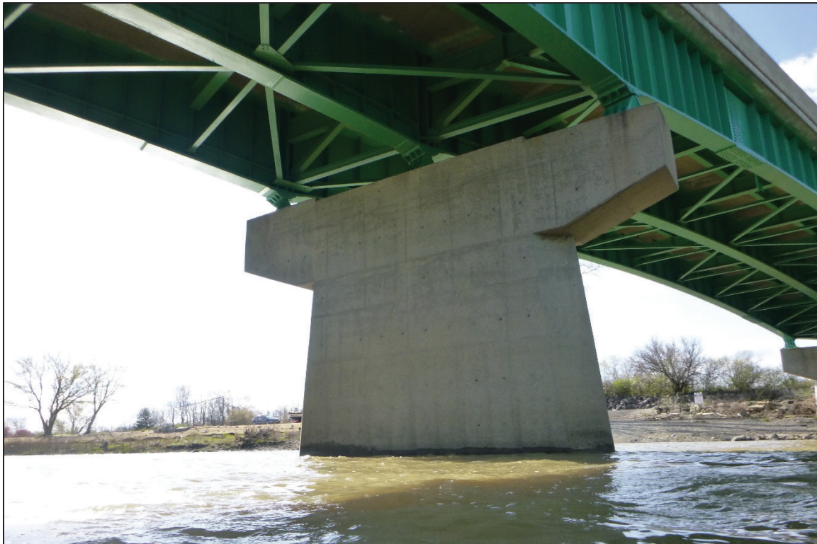
Photograph No. 16: View of the South Face of Pier 5, Looking Northwest.
