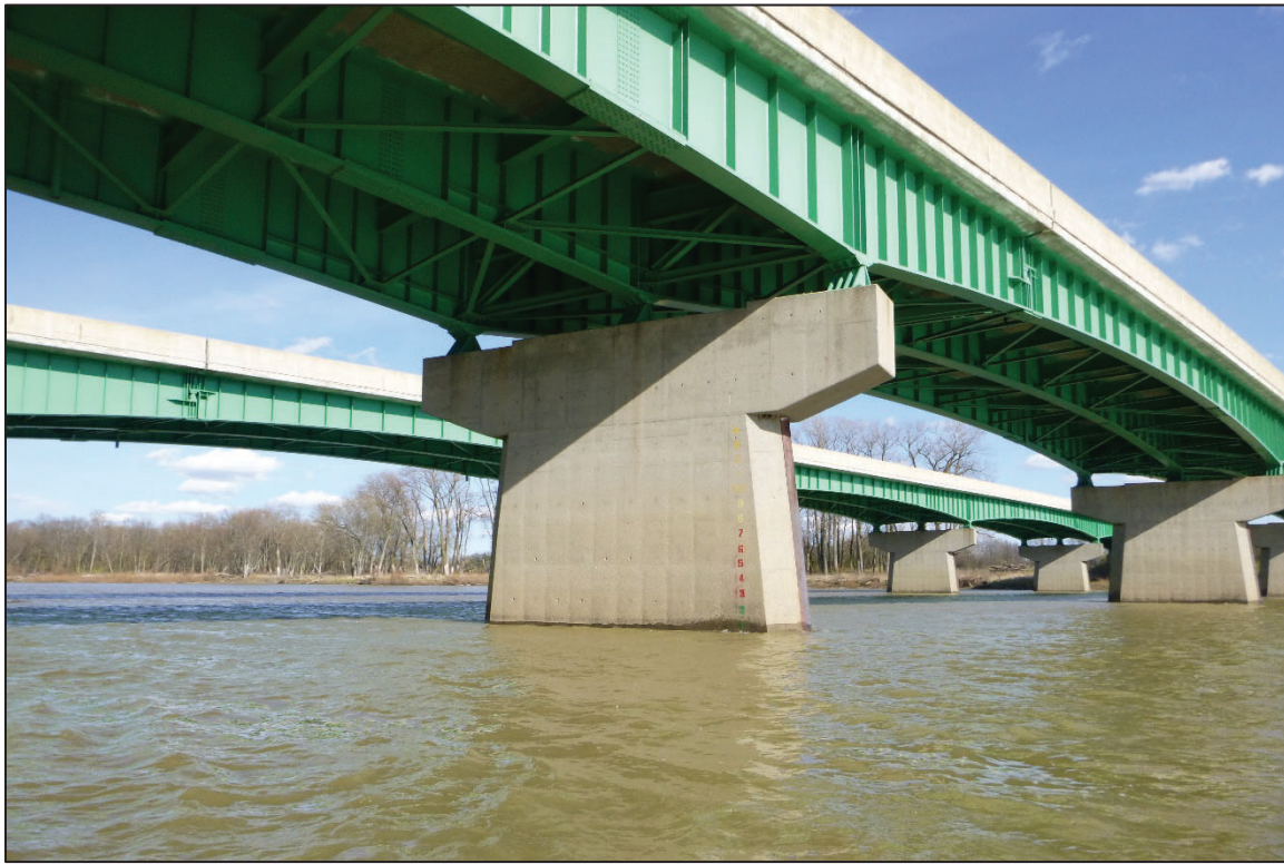
Photograph No. 15: View of the North Face of Pier 5, Looking Southeast.
