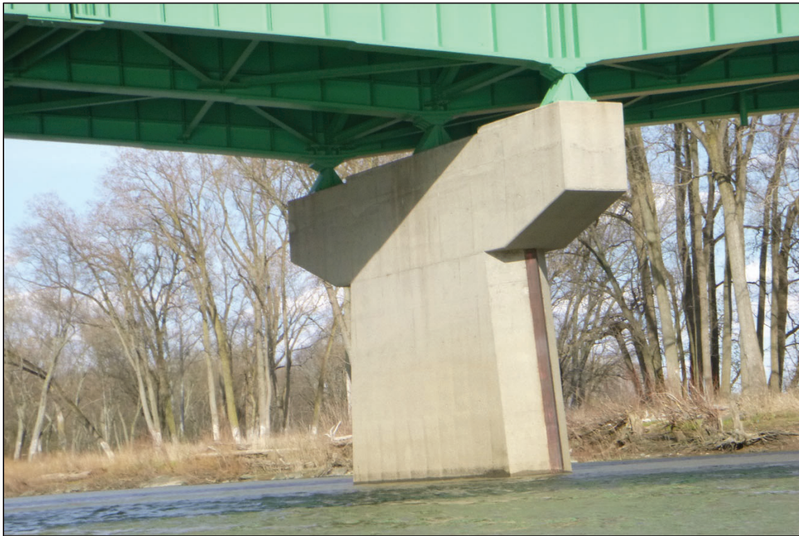
Photograph No. 9: View of the North Face of Pier 2, Looking Southeast.
