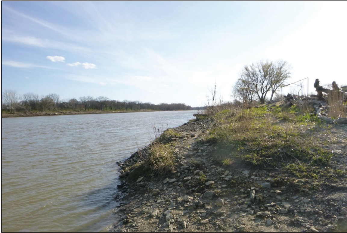
Photograph No. 3: View of the North Embankment Upstream of the Structure, Looking West.
