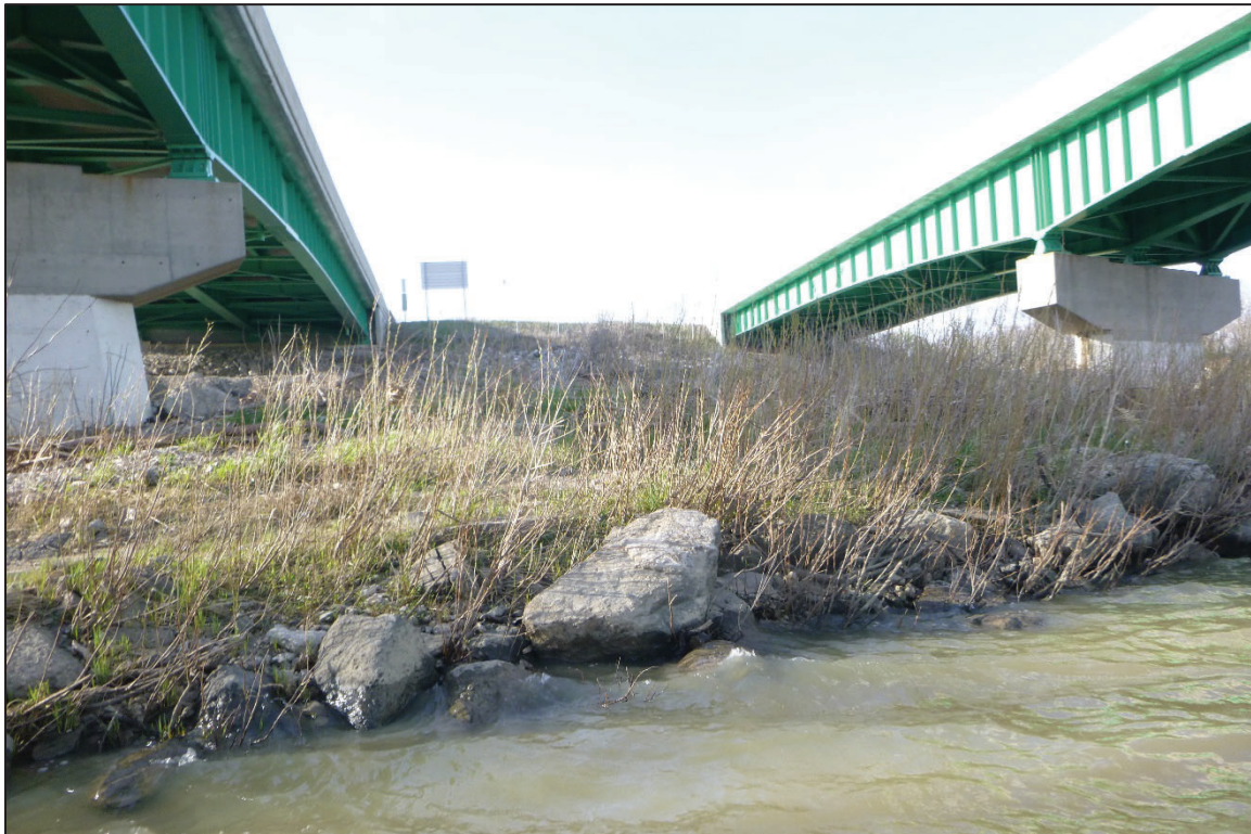
Photograph No. 4: View of the North Embankment at the Structure, Looking North.
