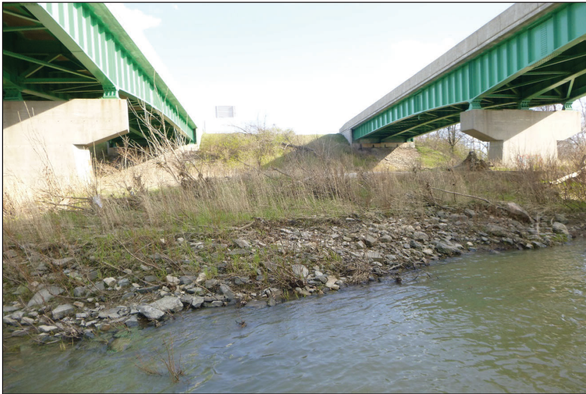
Photograph No. 7: View of the South Embankment at the Structure, Looking South.
