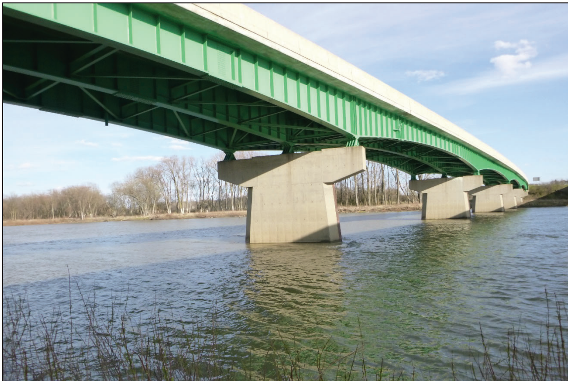
Photograph No. 2: Overall View of Structure No. 8706786 (WOO-475-0386R), Looking Southeast.
