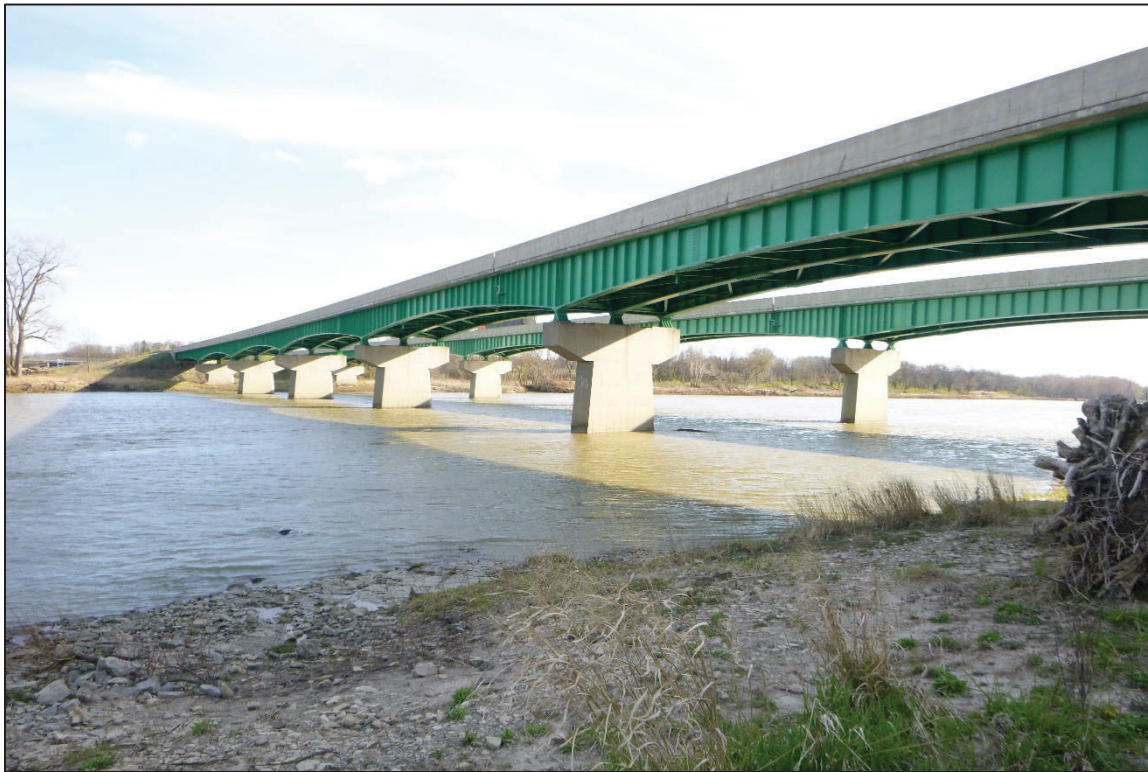
Photograph No. 1: Overall View of Structure No. 8706786 (WOO-475-0386R), Looking Southwest.
