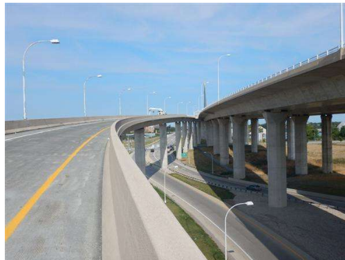
Photo 2 East elevation view of Ramp Z looking north including access equipment utilized.
