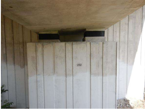
Photo 1 Typical condition of the Abutment 25Z bent and wall.
