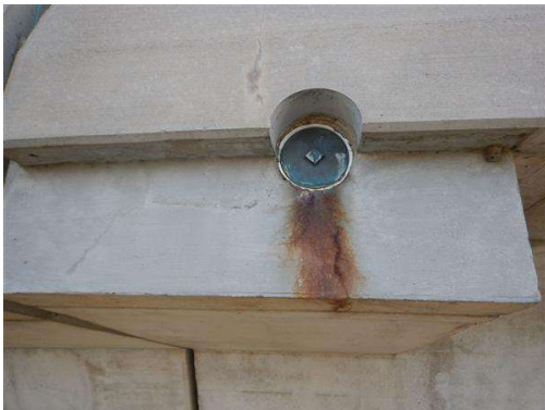
Photo 9 Typical cracking in the exterior pier segment on the edge face.
