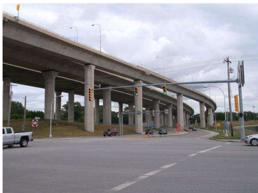
Photo 1 West elevation view of Ramp Z looking southeast.
