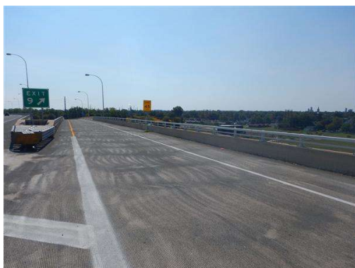
Photo 3 North end view of Ramp Z looking south.
